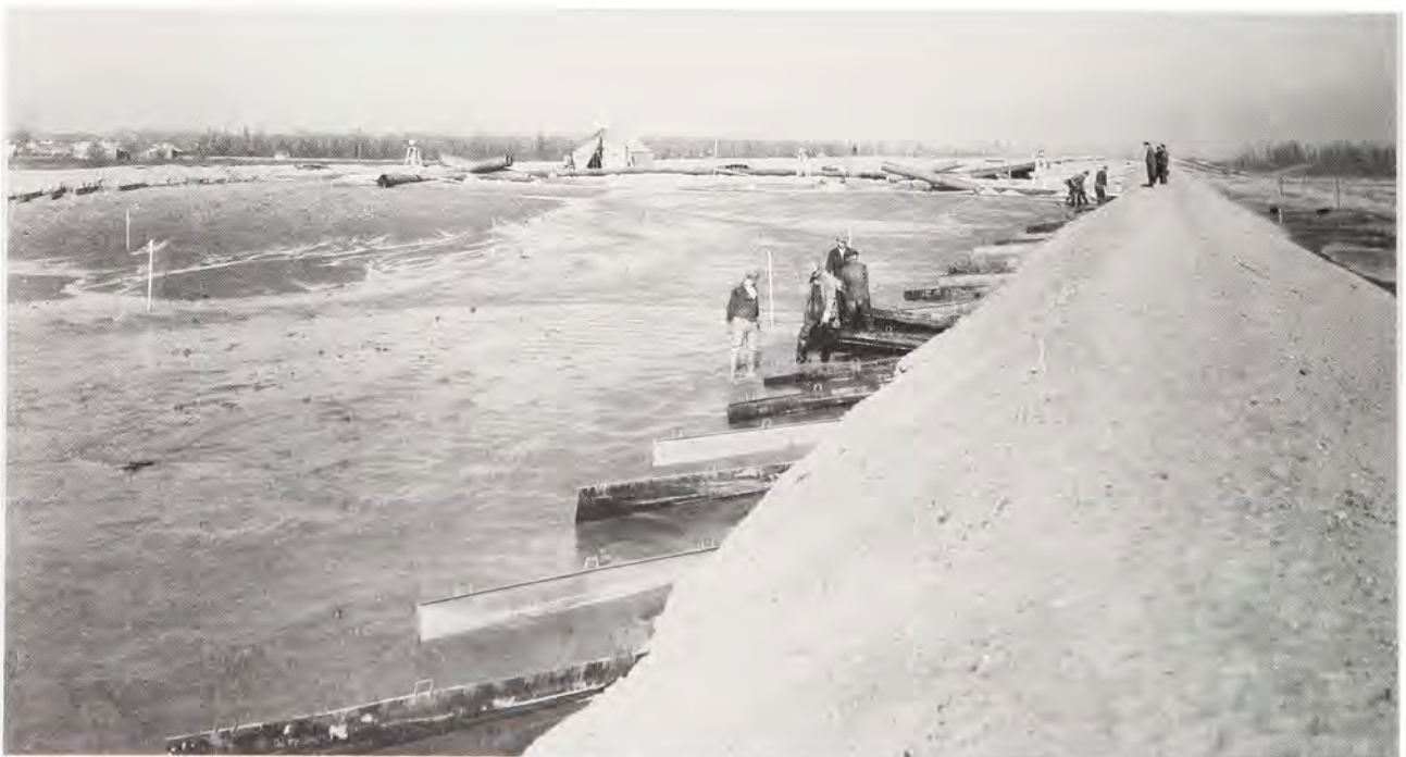
The temporary steel blades kept the water from destroying the emergency levee while it is under construction.
