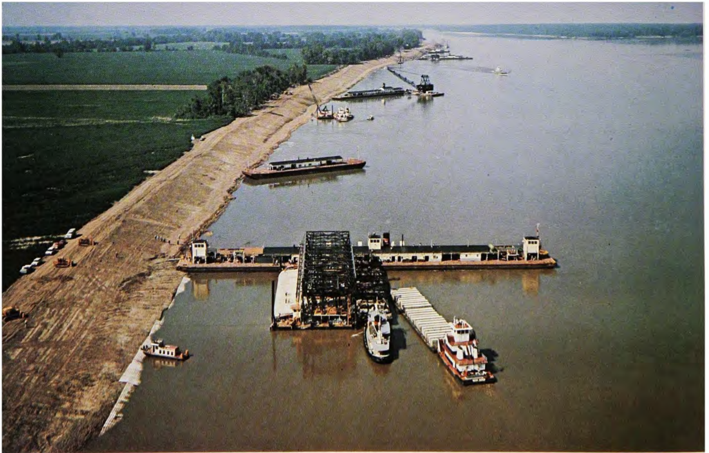
Working on the levee, today. In the background the banks are being cleared, and at mid-picture the slope is being prepared. A tug is nudging a barge of squares into position on the right side of the sinking plant, while the finished product is being rolled out and sunk to the left of the plant.
