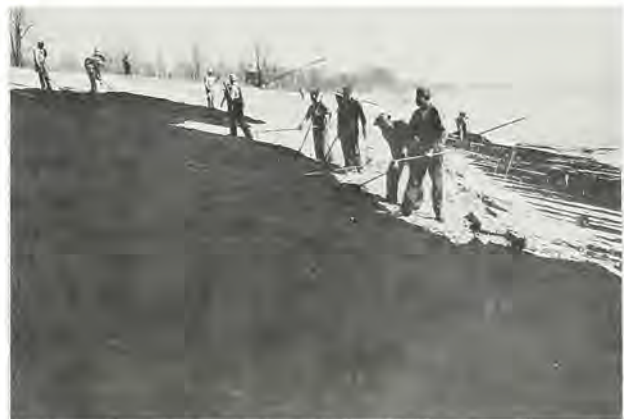
Workmen spreading hot asphalt for upper bank paving.
