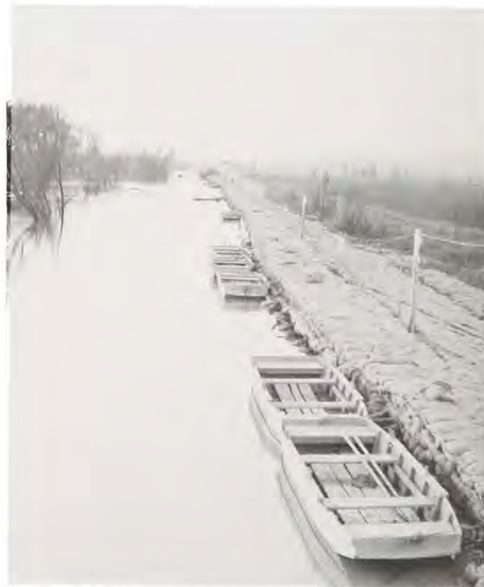
During the 1937 Flood the city of Memphis joined in with Shelby County to sustain the cost of constructing an emergency sandbag levee. The effort was successful in holding back the floodwaters of the Noncommah Creek. Feb. 10, 1937.
