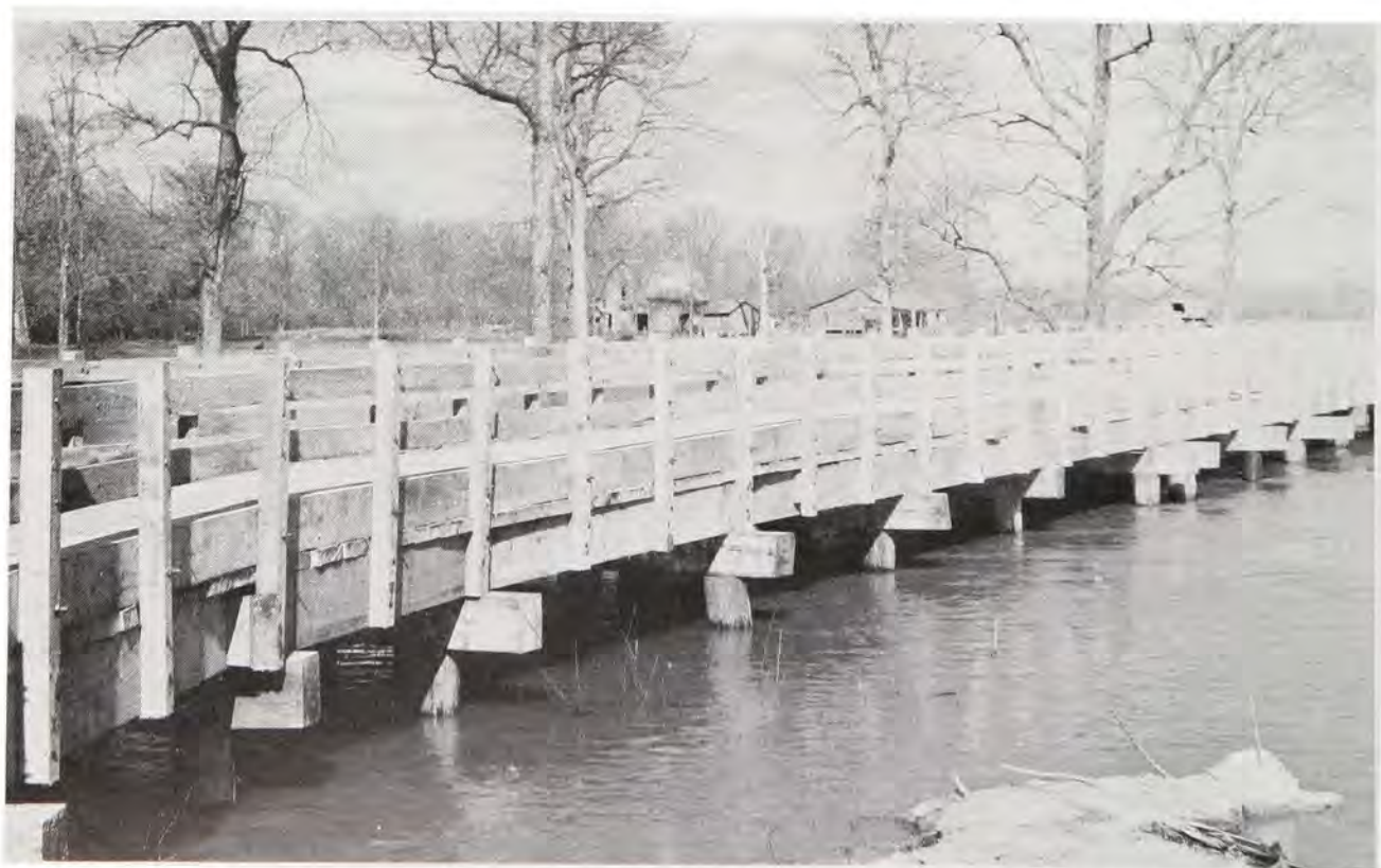
A fine example of an emergency bridge, constructed by the 129th Engineer Combat Battalion, to act as a temporary replacement for the Highway 38 bridge over the Cache River, near Cotton Plant Arkansas. White River Flood of 1945.
