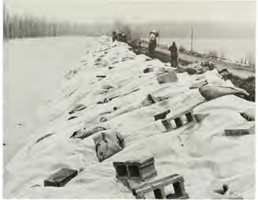
A recent development in emergency bank protection, polyethelene laid and weighted down on levee slope to minimize damage from wavewash and current erosion. Birds Point New Madrid levee, near Dorena, Missouri, during Great Flood of 1973.
