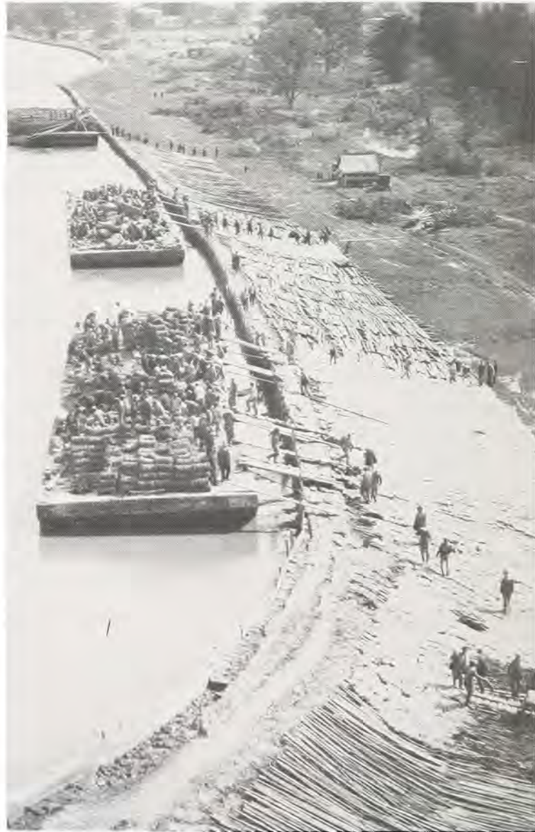
The Great Flood of 1927 created many unusual conditions that called for unusual remedies. Here we see a levee that is being paved on the landside slope, with sandbags overlaying wood and brush stabilizers. The levee has already been raised once, and is again in danger of being topped, thus it was necessary to reinforce the slope before attempting further repairs.
