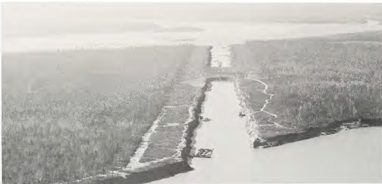
Aerial view of a cut-off nearing completion. The neck of land has been cleared of trees, and the channel has been cut to the point where only the plug remains. The plug will stay in place until river conditions are right for its removal.
