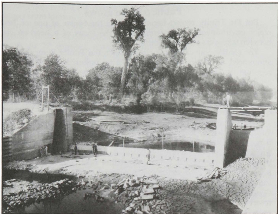
Workers labor at partially finished Lock and Dam Number 1 on the Trinity River near Dallas on Oct. 30, 1917. (Reprinted with permission of the Dallas Historical Society)
