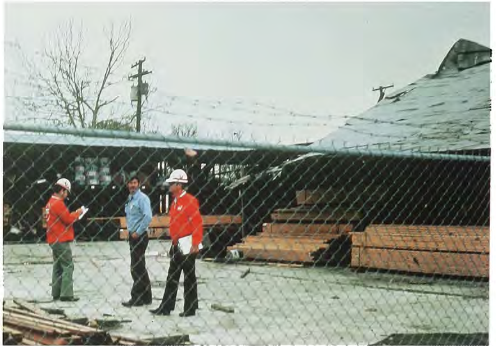
Division Emergency Operations personnel surveyed tornado damage at this lumber yard in Cabot, Arkansas, on 29 March 1976.
