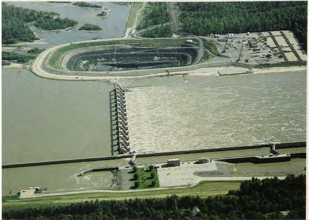
Non-federal interests now construct hydropower facilities at Corps dams, as in the excavation on the far side of the Arkansas River at Murray Lock and Dam.
