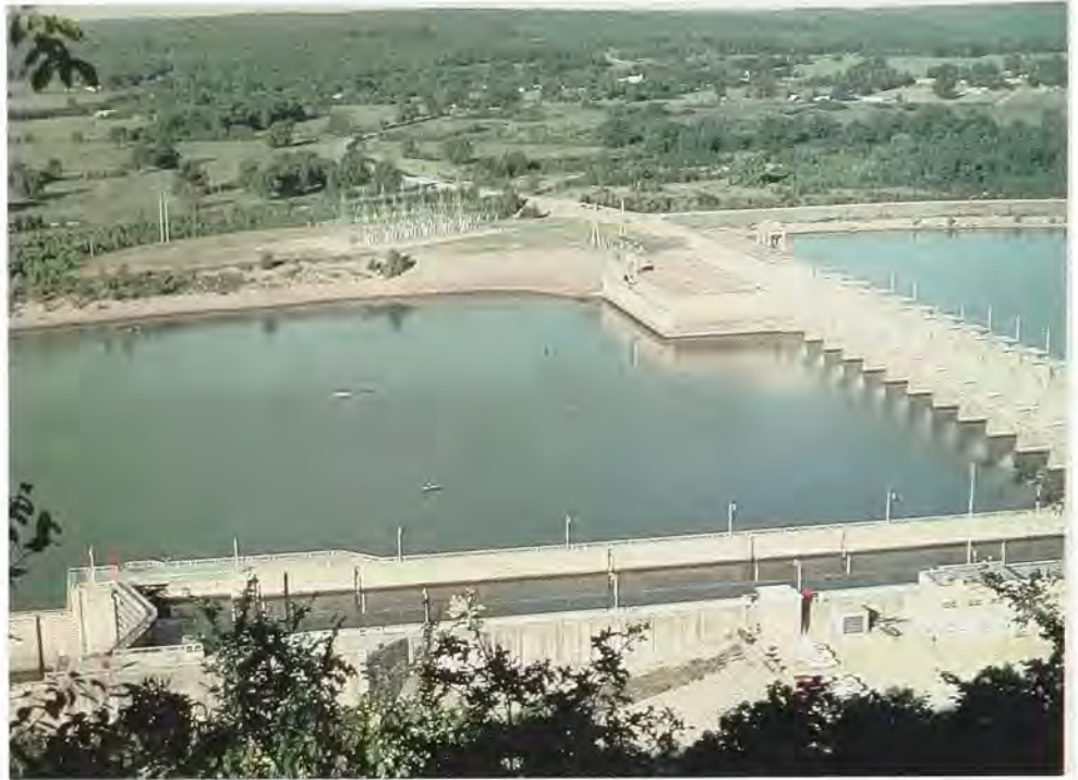
The locks at Ozark Lake, Arkansas, help make the Arkansas River navigable.
