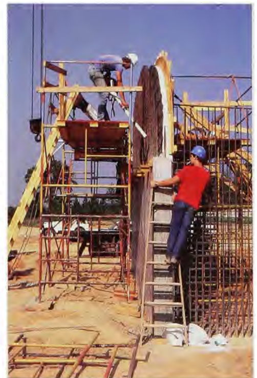
Construction workers at Fort Polk build an igloo for ammunition storage.
