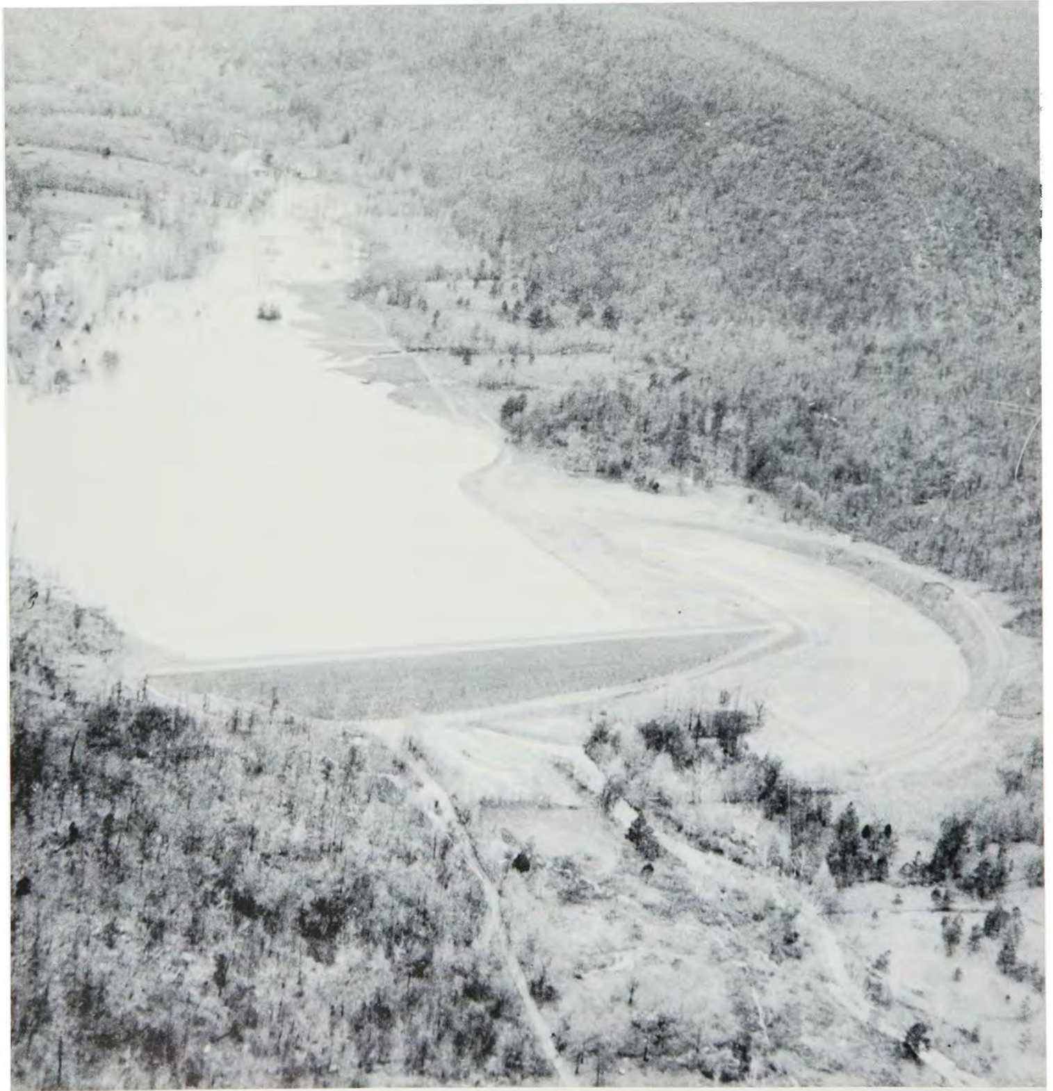
The U.S. Soil Conservation Service was one of several federal agencies that worked to prevent flood damages in the Southwest. This earthen dam is one of its projects in eastern Oklahoma. (U.S. Soil Conservation Service photo)
