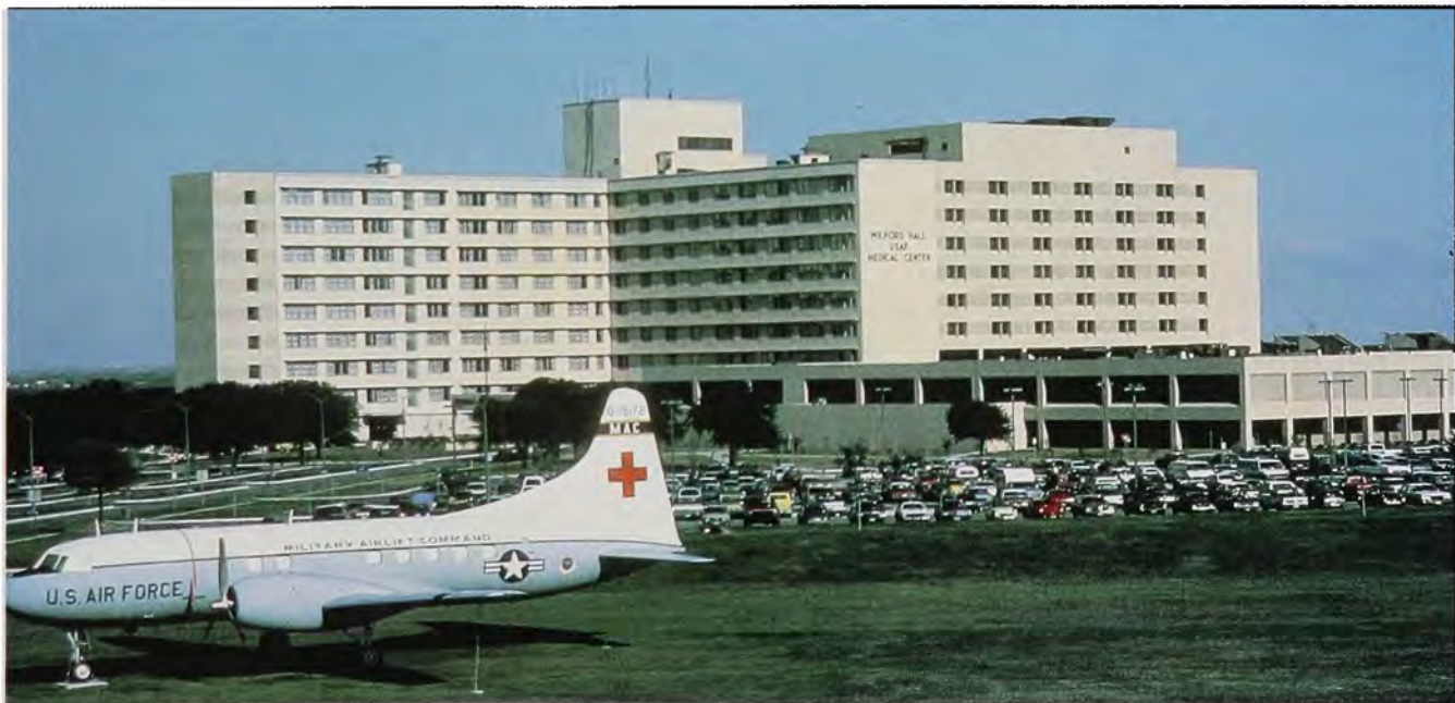
Wilford Hall Hospital, Lackland Air Force Base, Texas.
