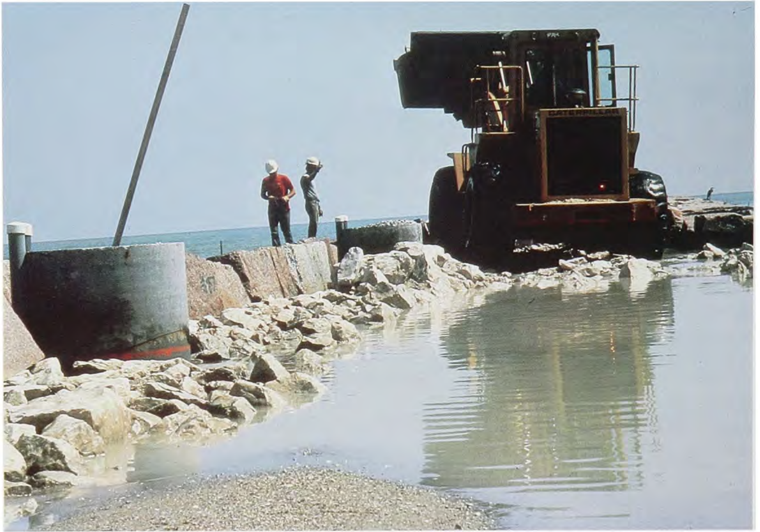
Construction at Freeport Harbor keeps its waters navigable.
