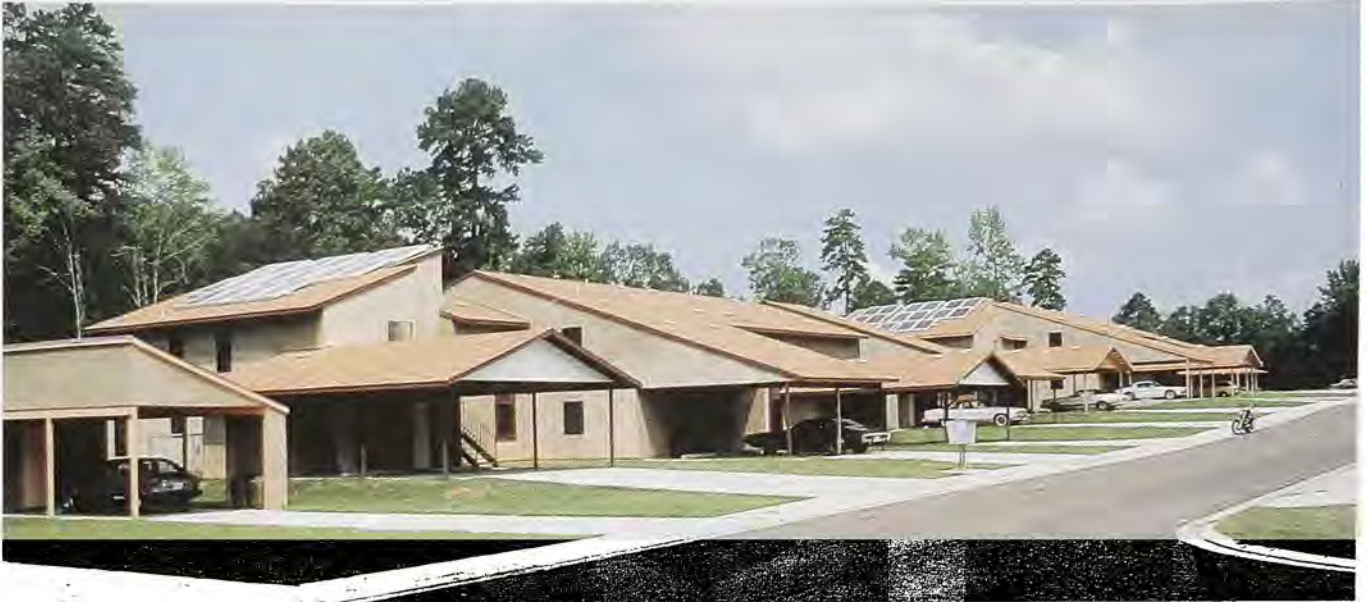
Family housing at Fort Polk, Louisiana, features solar panels to heat water.
