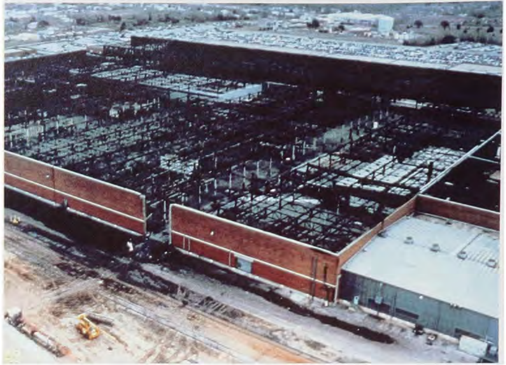
A welder's torch sparked a blaze at Tinker Air Force Base, Oklahoma, that destroyed one-third of a major aircraft repair facility in November 1984.
