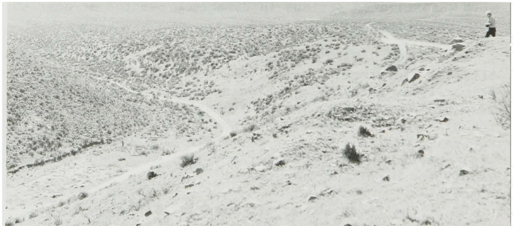
Zintel Canyon Dam Site - Looking Upstream into Reservoir Area
