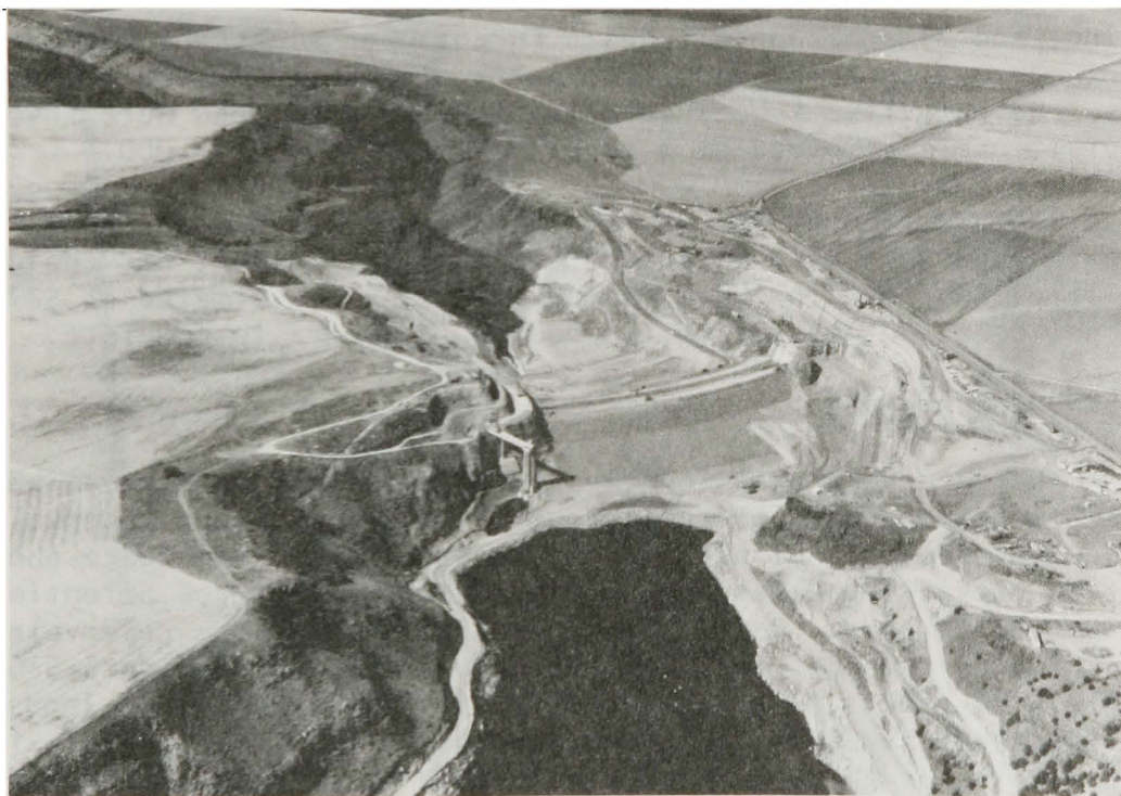
RIRIE DAM CONSTRUCTION - 1975 Spillway Channel at Right Abutment Outlet Works at Left Abutment
