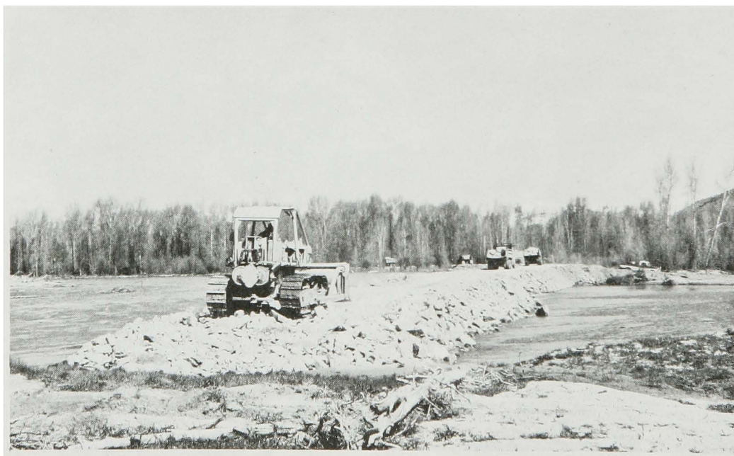
FLOOD FIGHT ACTION - JACKSON, WYOMING - 1975 Cut-off Dike to Preclude Avulsion
