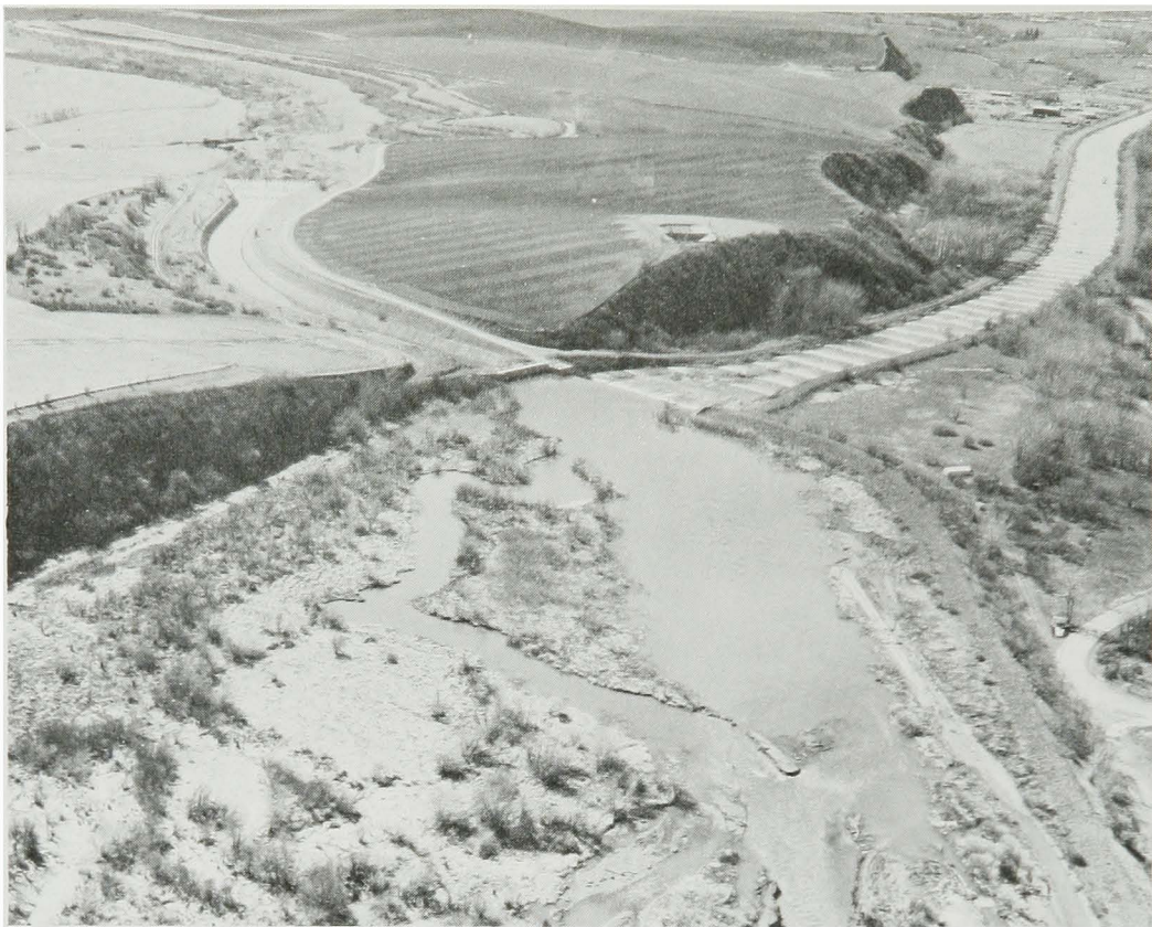
MILL CREEK PROJECT IN ACTION Offstream Reservoir at Extreme Left
