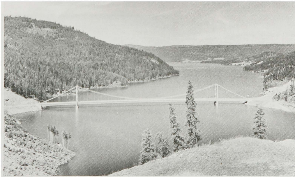
DENT BRIDGE (River Mile 17)
