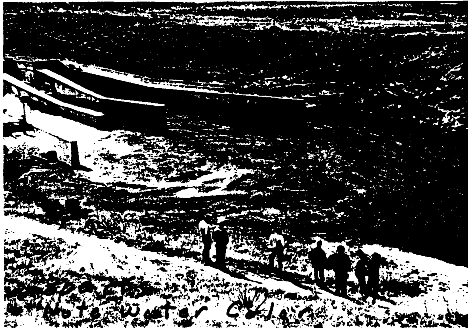
CHERRY CREEK RESERVOIR OUTLET WORKS
