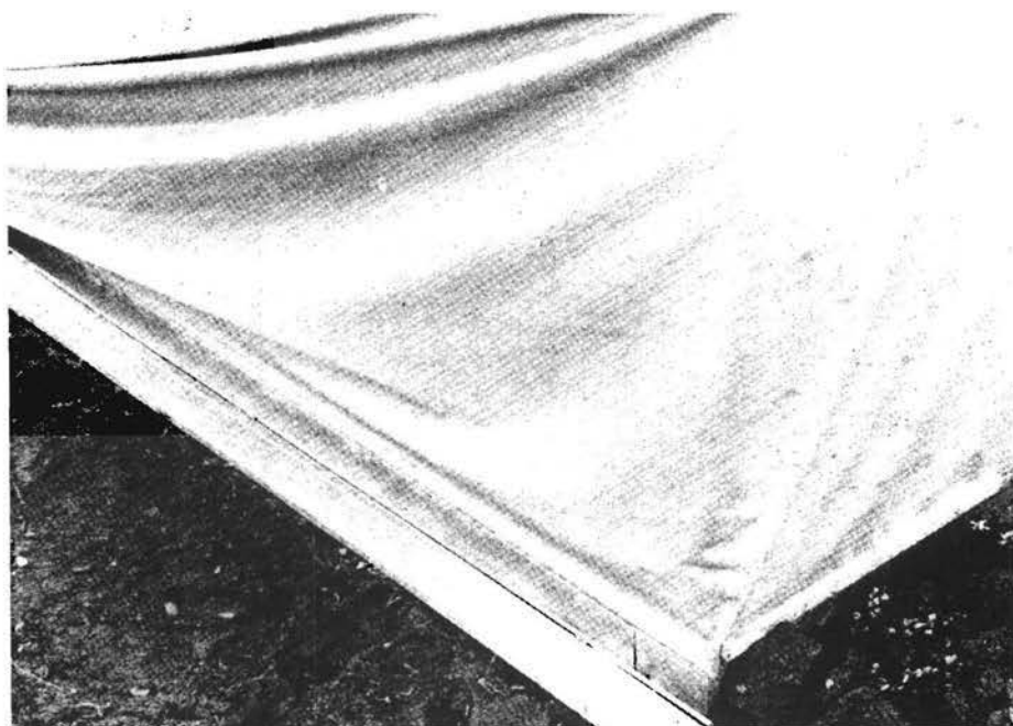
Figure 67. Protective fabric being removed from storage container and attached to the house at the desired elevation
