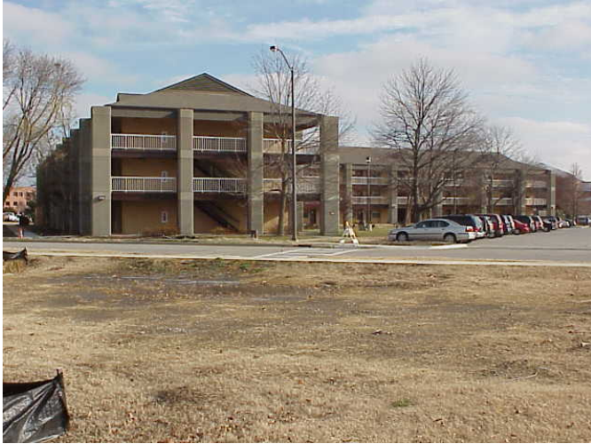
View facing northeast at Building 1912.
