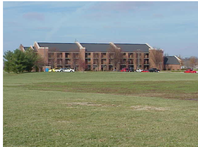
View facing east across the location of the proposed dormitory at Building 1820. The proposed dormitory would be of similar design.
