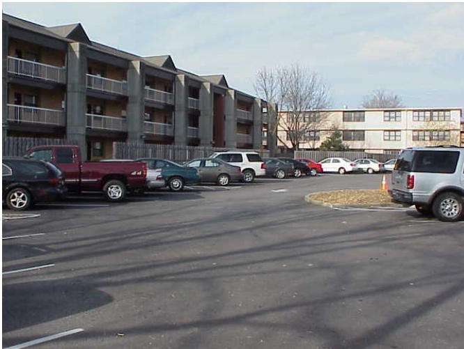
View facing west at Building 1912.
