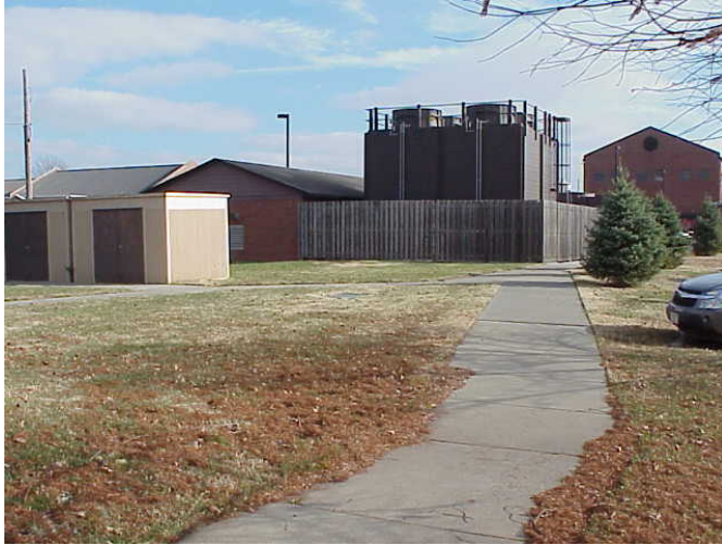
View facing northeast at Building 1899.
