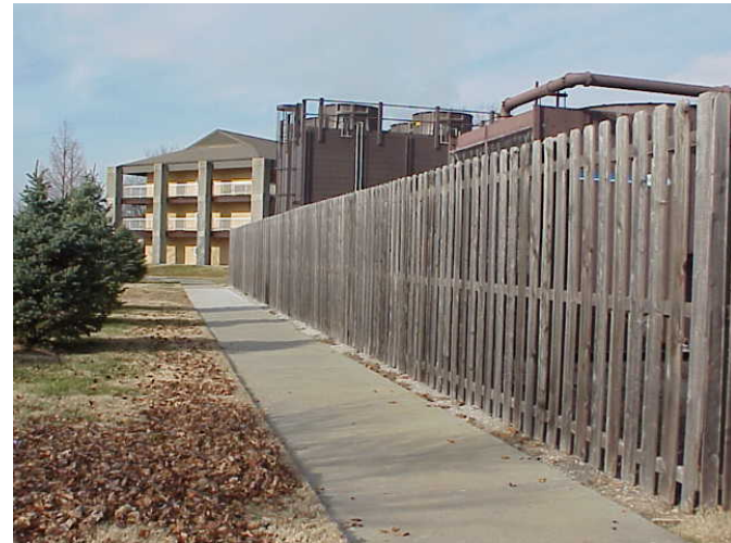
View facing northwest at Building 1899. Building 1912 is in the background.
