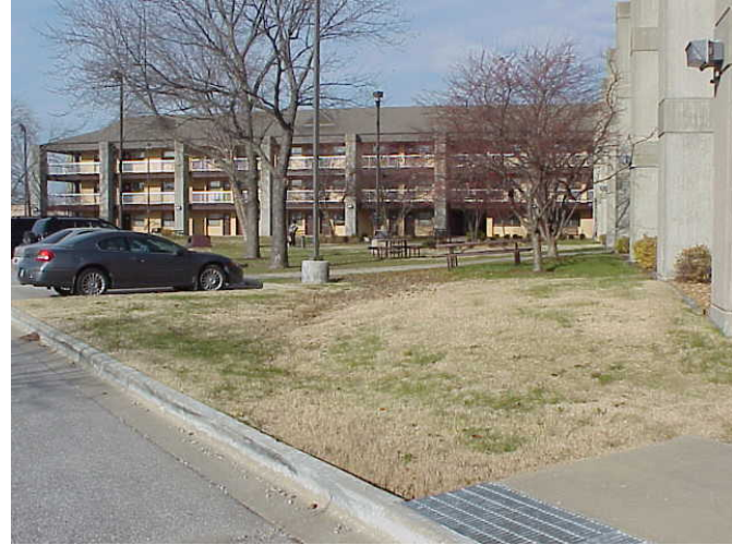
View facing north at Building 1912.
