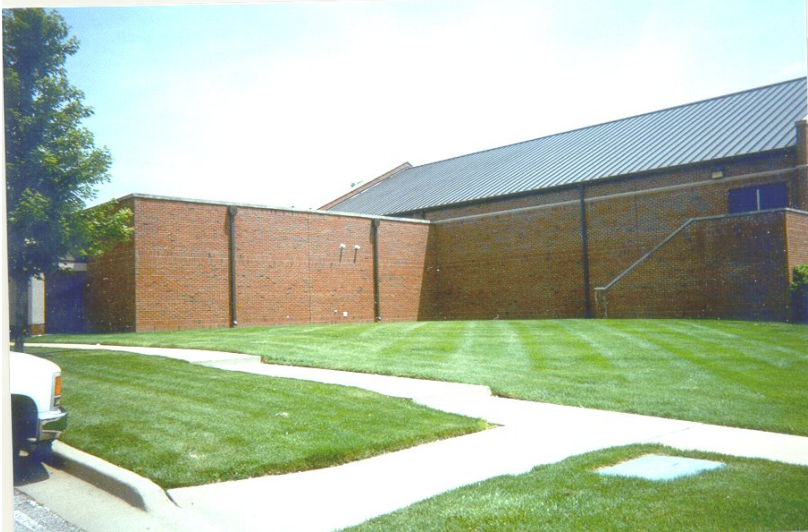
GRPC – West side of the building.
