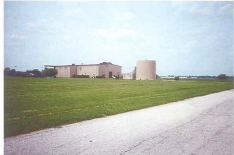
View looking northwest at the site of the Proposed Action. Building 742 is in the background.
