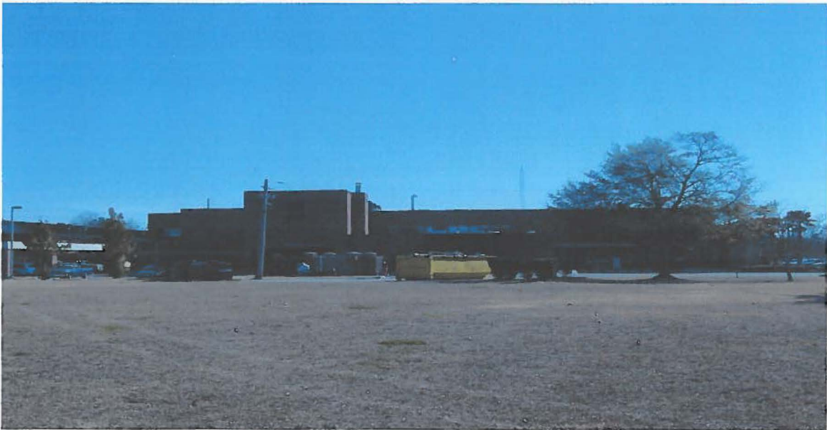
Photo 4: Looking southeast at Clinic Building 364.
