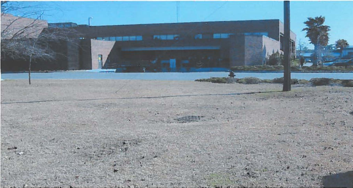
Photo 6: Looking southeast at Clinic Building 364. Stormwater drain catch basin in foreground.
