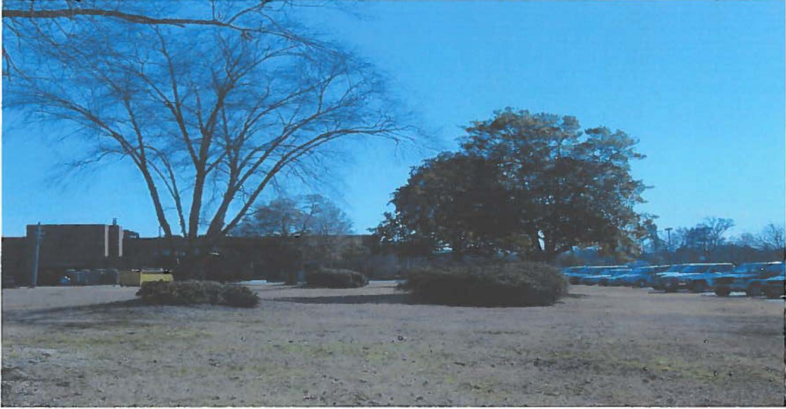
Photo 1: Looking southeast at Clinic Building 364.
