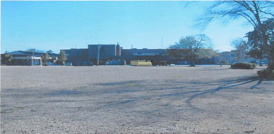
Photo 2: Looking southeast at Clinic Building 364. Proposed site is almost unobstructed.
