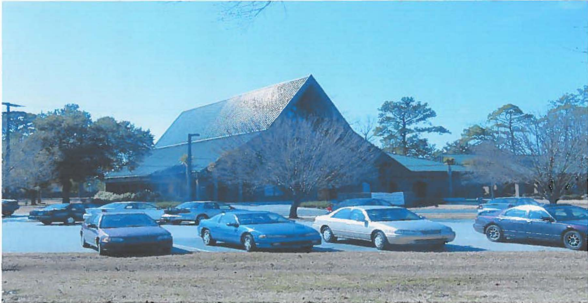
Photo 3: Looking west at Chapel Building 1005.
