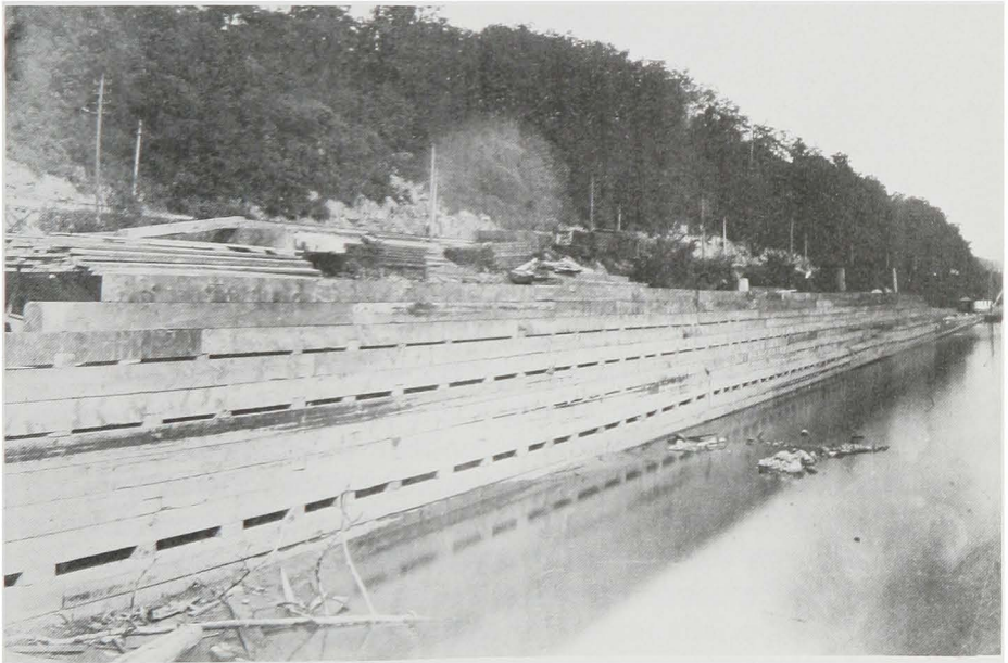
The upper guide wall was built of timbercribs along the bank upstream of the lock entrance.
