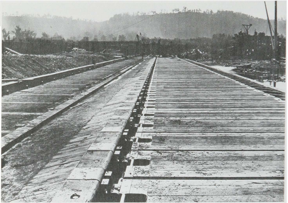
The interior of the navigable pass cofferdam in 1881 with all the wickets collapsed atop the foundation.
