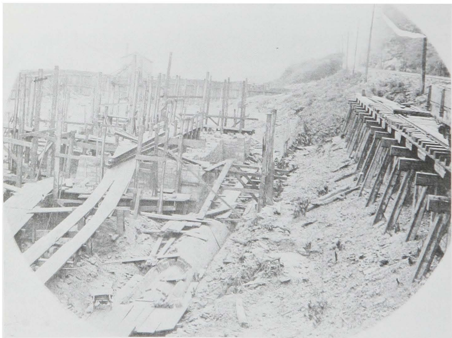
The lock house foundation was under construction in this 1878 picture with a brick sewer line behind the foundation. In the background is the wall of the cofferdam built around the lock's land wall.
