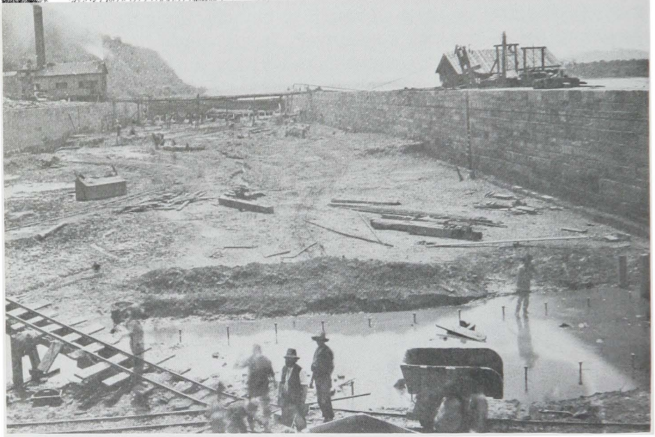
Workmen clearing the foundation inside the lock chamber.
