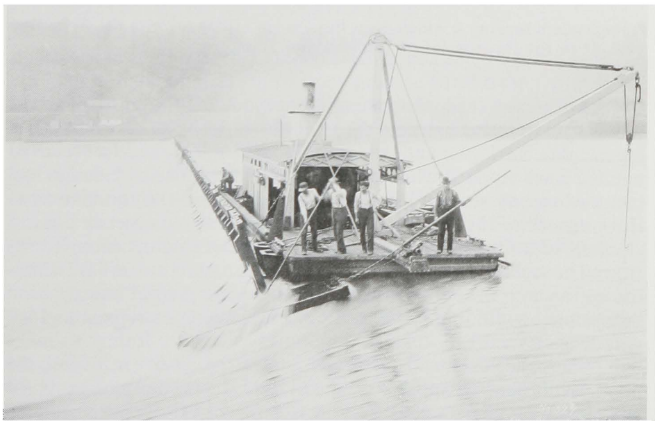
Dam tenders maneuvering the wickets at Davis Island in 1904.
