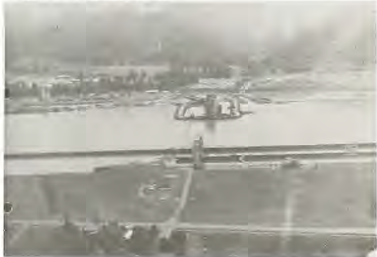
Flooded cofferdam at Hannibal
