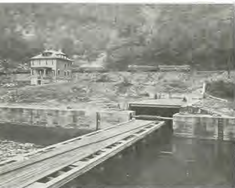
Typical rolling lock gate - Ohio River
