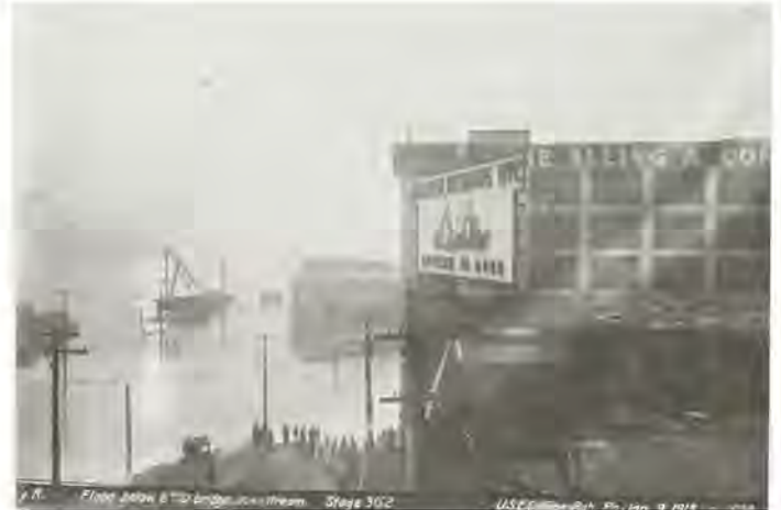
Allegheny River below Sixth Street Bridge, Jan. 9, 1913
