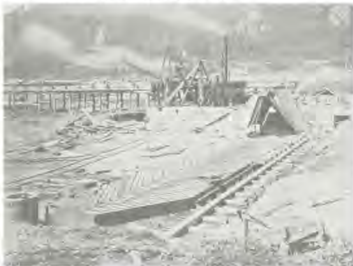
A-Frame construction - Dam 6, Ohio River
