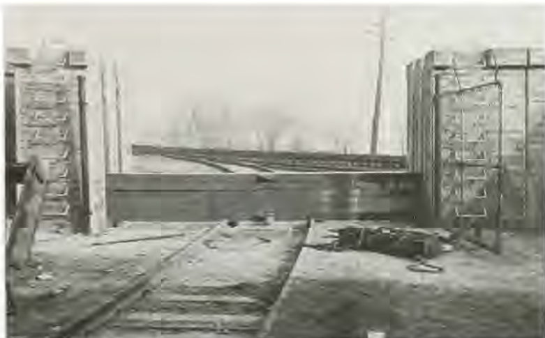
Close-up of gate closure and bulkhead timbers - Wellsville, Ohio
