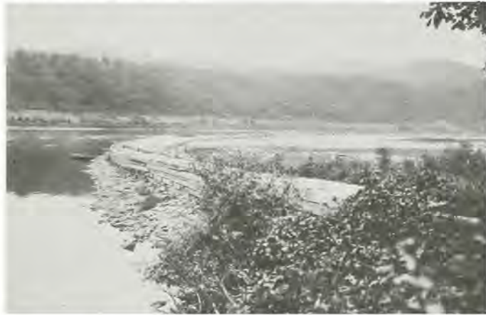
Allegheny River improvement - Redbank dike
