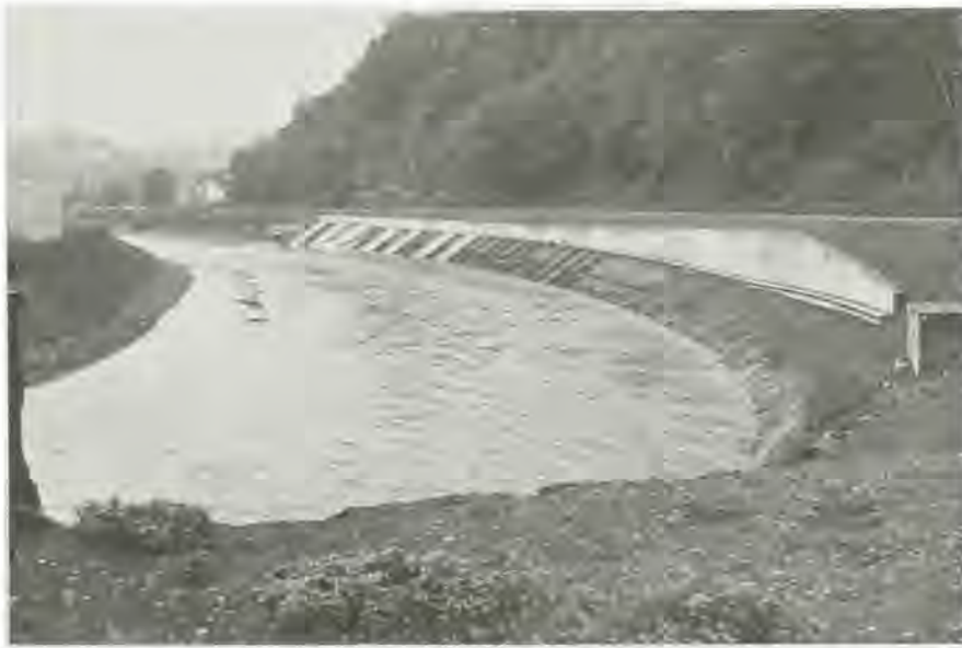
Chartiers Creek local protection project - June 1972
