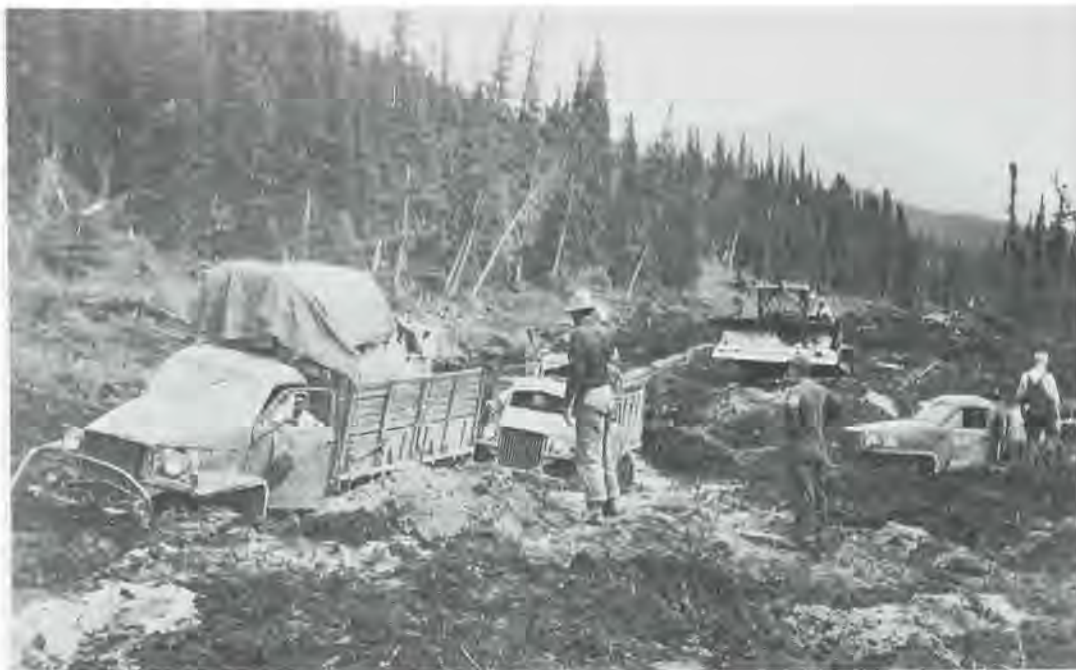
The Alaska Highway under construction.
