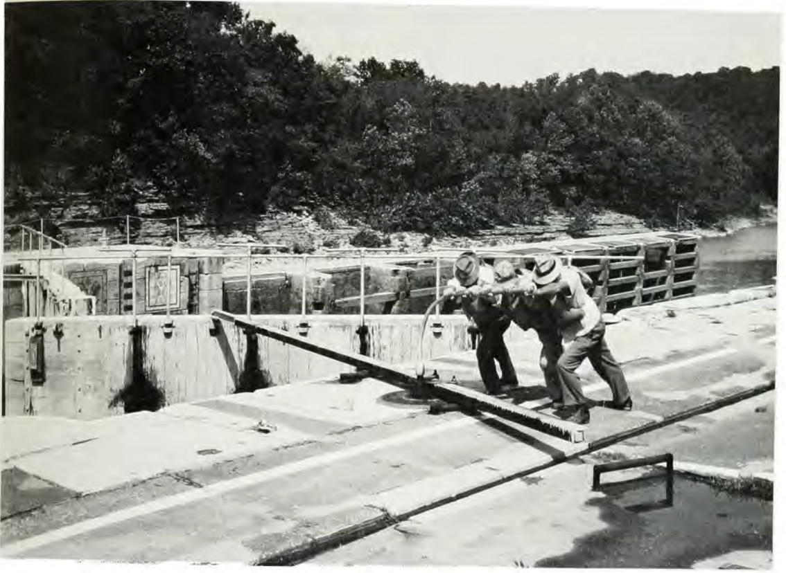
Manual operation of the lock gates on the Kentucky and Green rivers required physical strength. Walking in circles, the lockmen turned a rack and pinion to move the lock gates.
