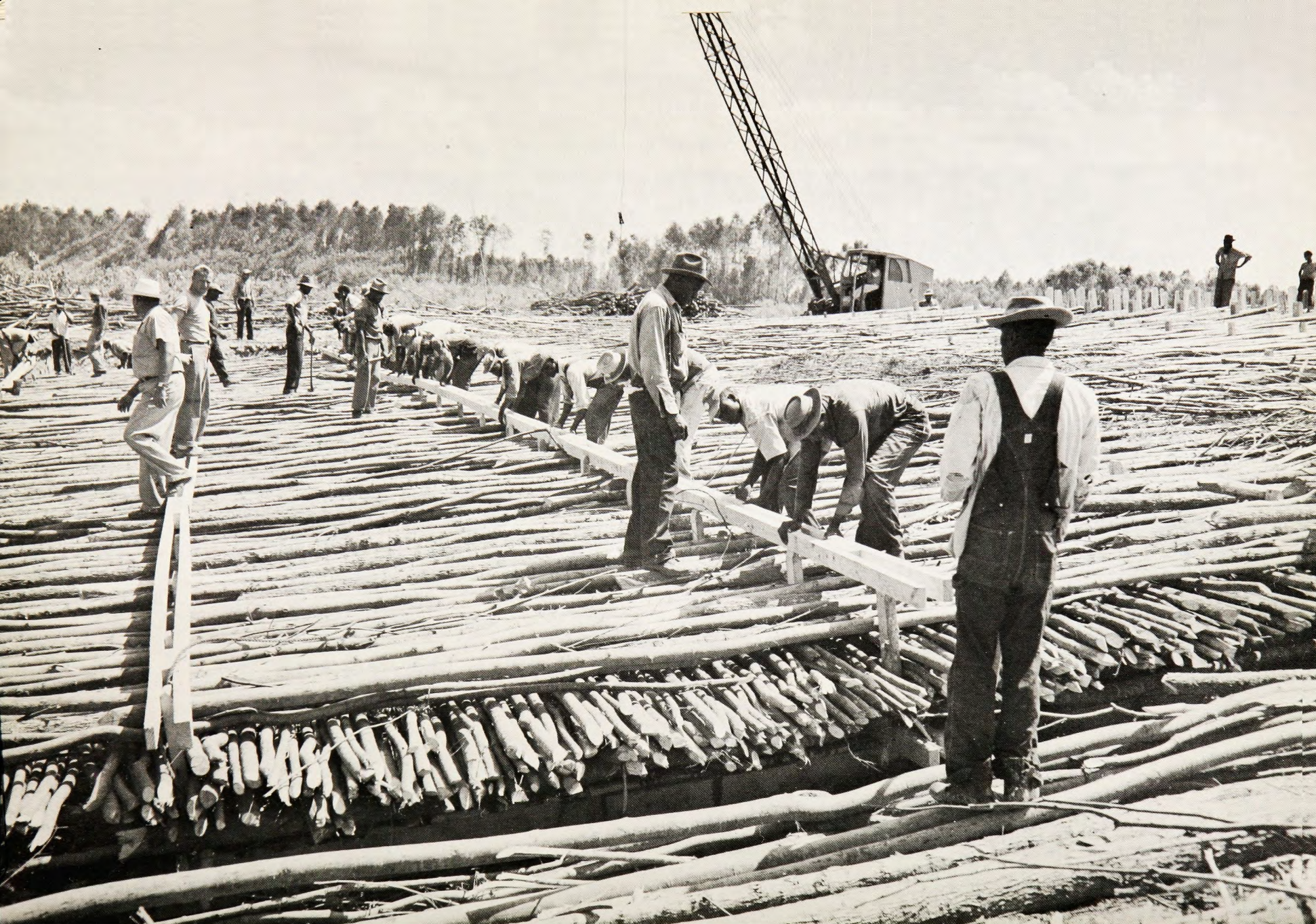
Fig. 4. Bank protection — old style. Weaving of a giant willow mattress, 1950. (Photo by C. Fortler)
