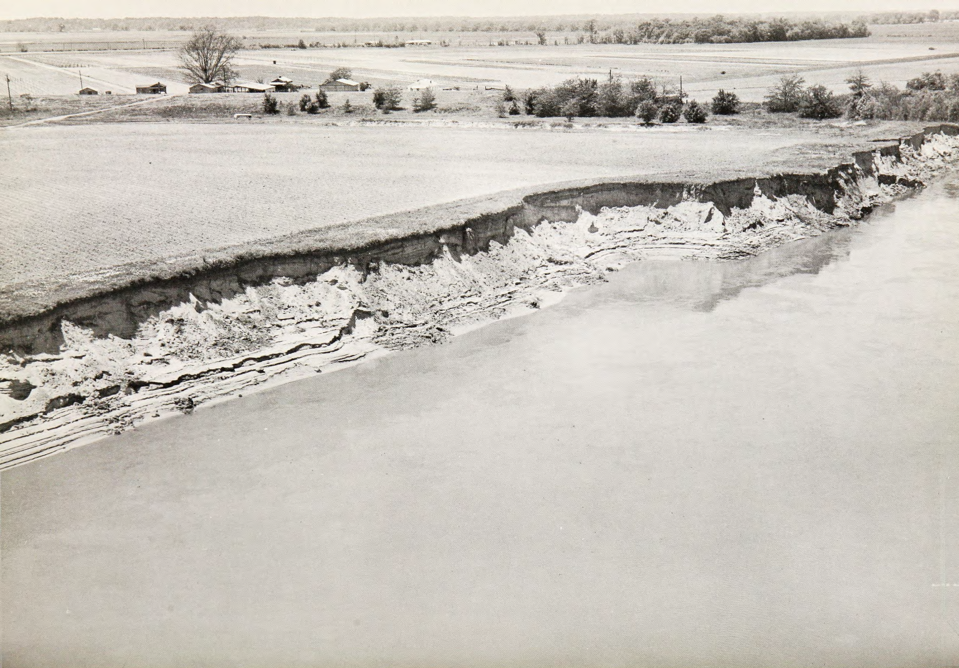
Fig. 12. The Red River problem. Erosion, destruction of farmland, the shoaling of the channel that will follow — these are the effects of the undisciplined Red. (Photo by S. R. Sutton)
