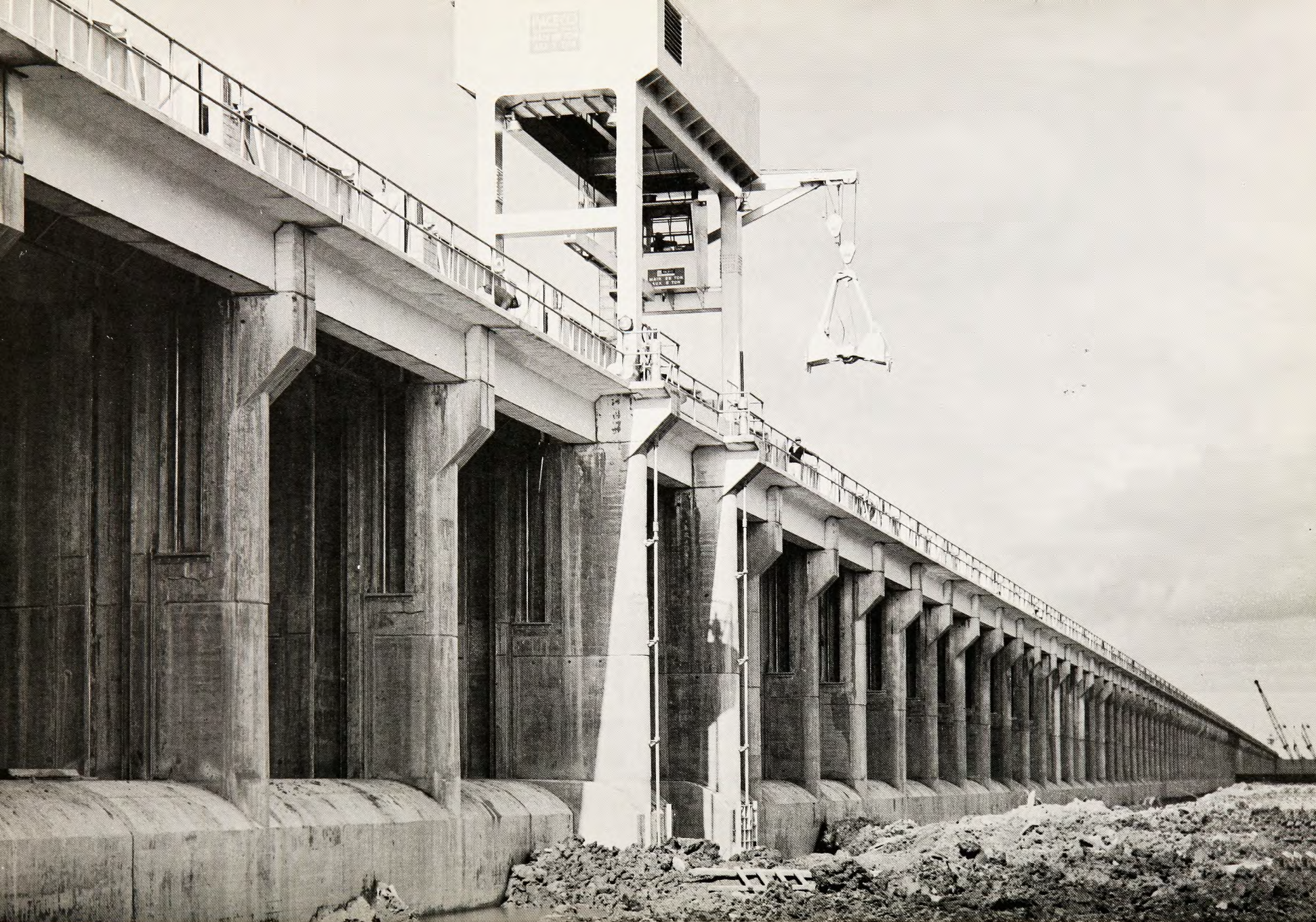
Fig. 8. Morganza Control Structure nearing completion. 1953. This structure controls the entry of water into the East Atchafalaya Floodway. (Photo by C. V. Dyer)
