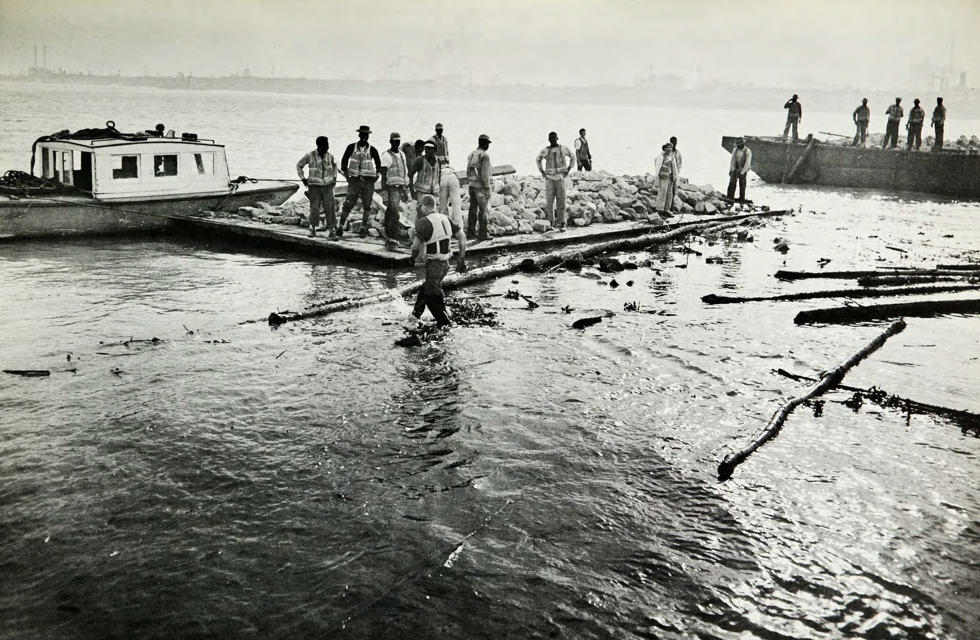
Fig. 5. "Walking on the water." Evenly distributed crushed rock gradually sinks a willow mat beneath the water. New Orleans, 1950. (Photo by C. Fortier)
