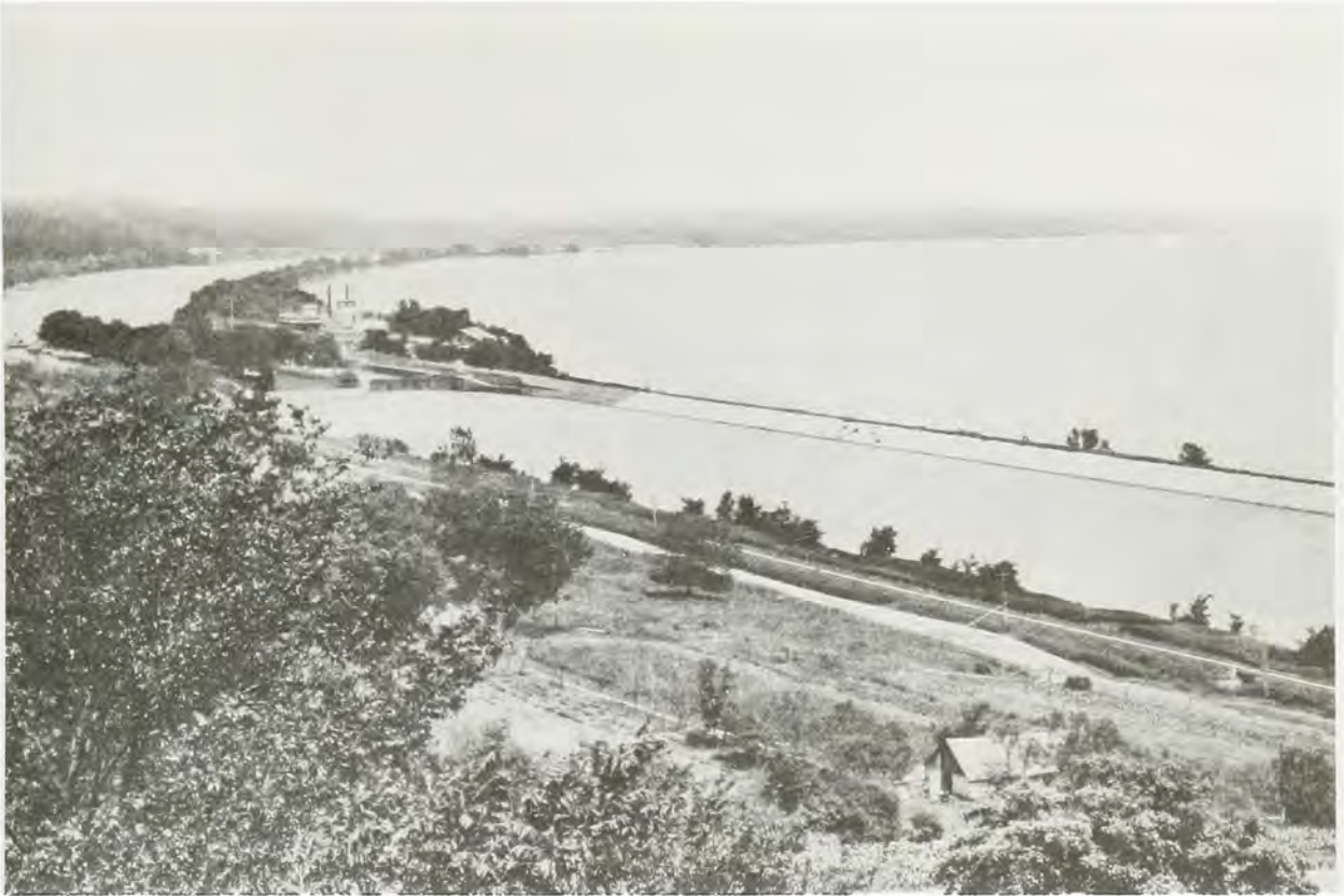
Middle lock at the Des Moines Rapids Canal, 2.5 miles above the lower lock at Keokuk, Iowa.
