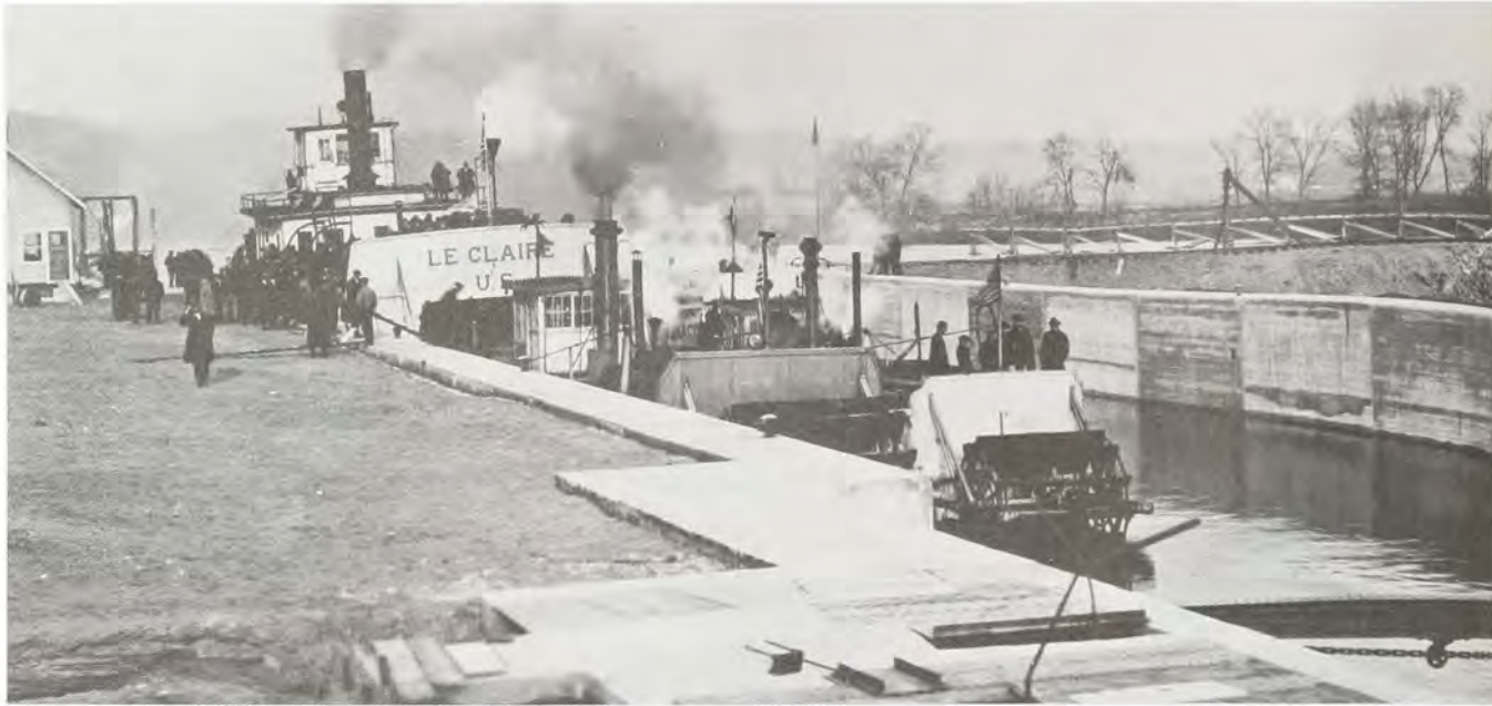
Opening day ceremonies at the new Le Claire Canal and Lock, built at the head of the Rock Island Rapids as part of the 6-foot channel project.
