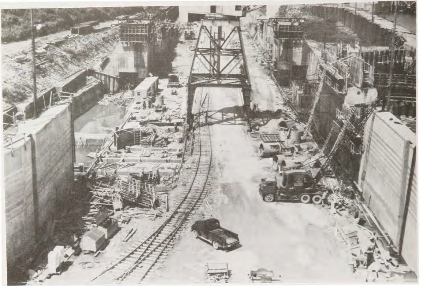
Construction at new Lock 19, taken June 1955.
