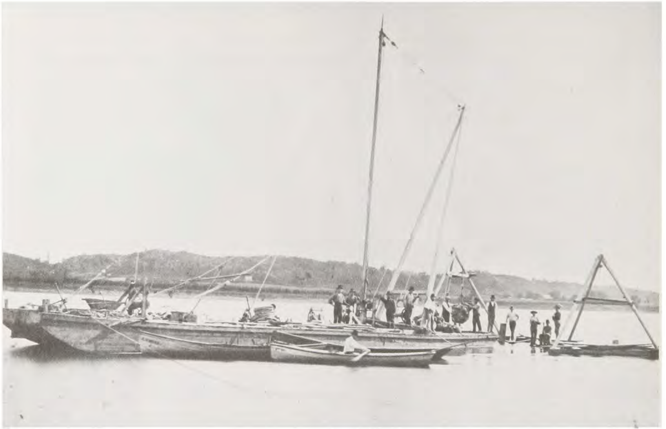
Drilling tripods and a derrickboat being used to blast and remove rock from the Rock Island Rapids. These tripods were not very different from those devised by Captain Robert E. Lee for work on the Des Moines Rapids in 1837.
