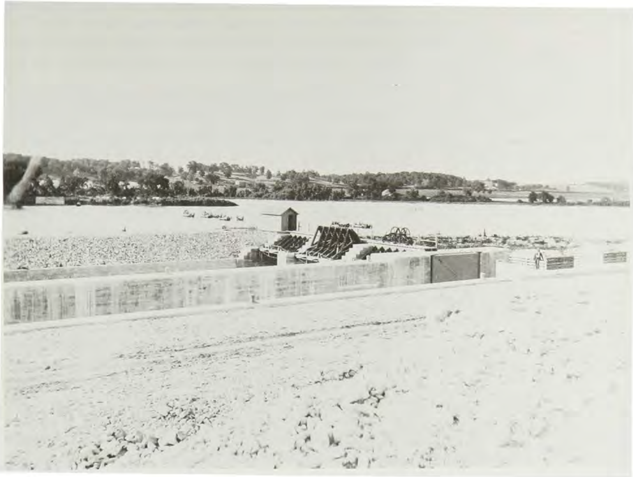
Control works and guard lock at the head of the feeder canal near Sterling, Illinois. The Rock River is in the background.
