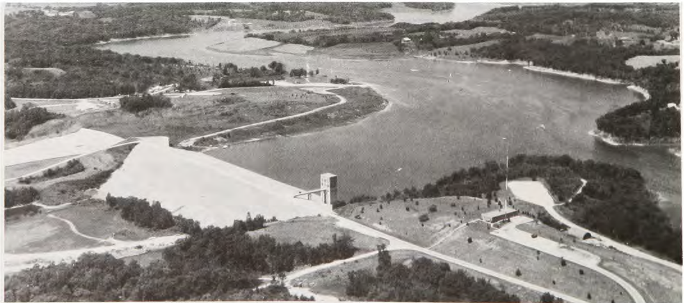
An overview of the completed facilities at Coralville.
