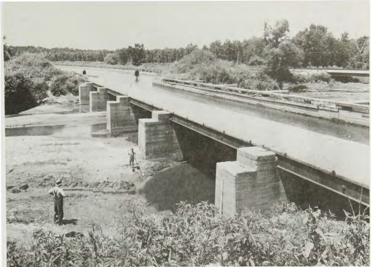
Aqueducts were needed at those places where the canal crossed another stream. This is Aqueduct No. 1.
