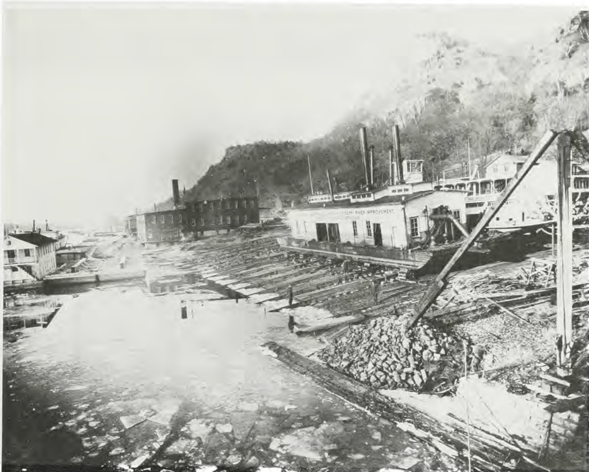
The Rock Island District Boatyard at Fountain City, Wisconsin, with the hydraulic dredge Vesuvius nearing completion on the ways.
