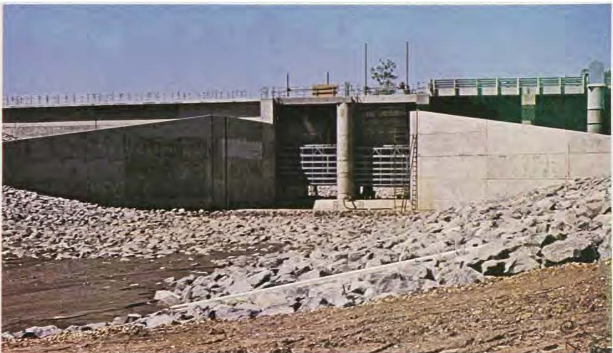
The Muddy Bayou Control Structure only a few months from completion
