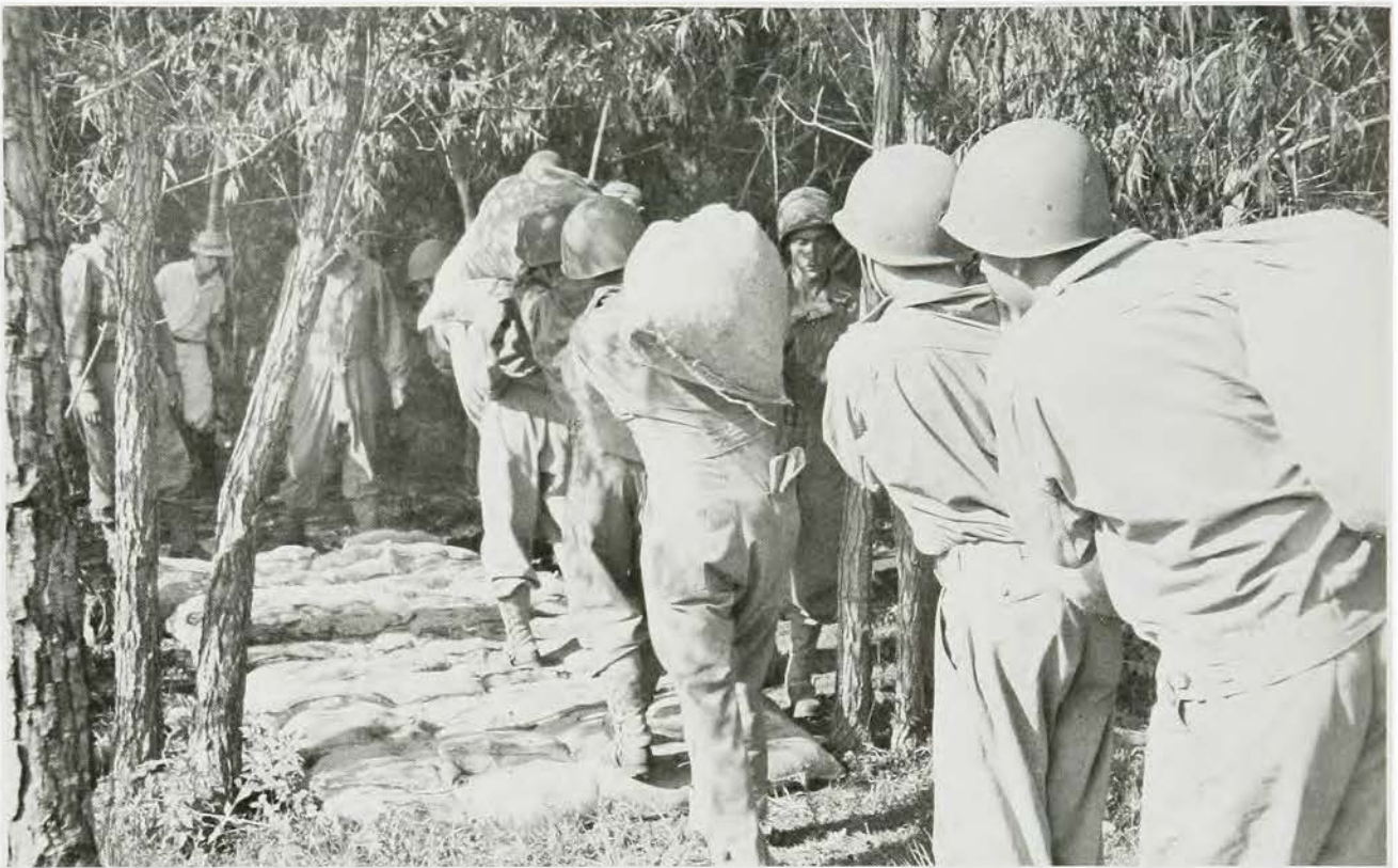
Engineer troops placing sandbags around sand boils in the dense junglelike underbrush on Arkansas River levees
