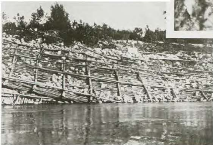
Mat in place, remainder of willows are below water level
