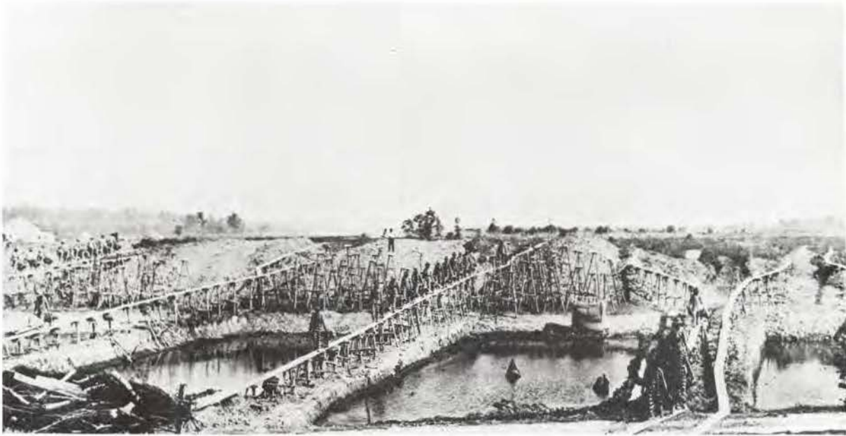
Building levee by wheelbarrow
