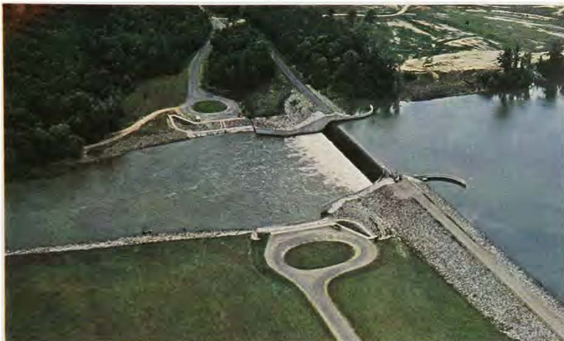
The reregulation dam at DeGray Dam, a major component in DeGray's pumpback feature
