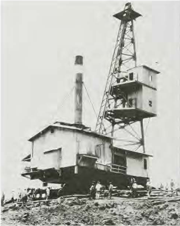
One of two giant cranes which made up a levee-raising "tower machine"
