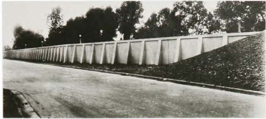
Stationary floodwall in Monroe, Louisiana, completed in 1935
