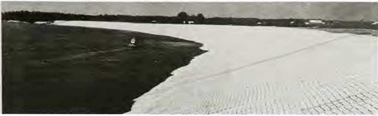
Revetment along slope of river bank. Final riprap covering traditionally placed at top of finished mat is not yet in place
