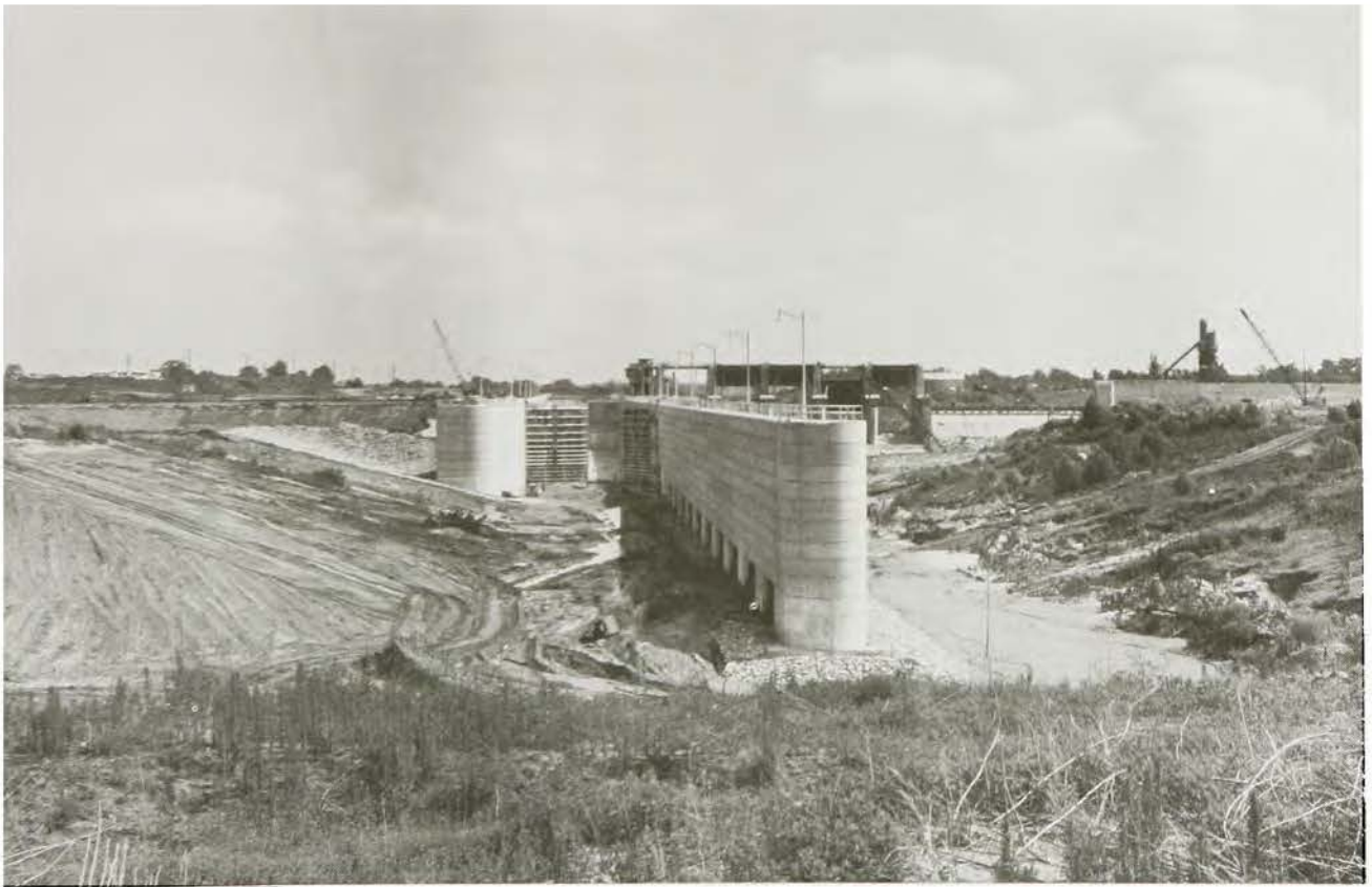
Construction of Columbia Lock and Dam
