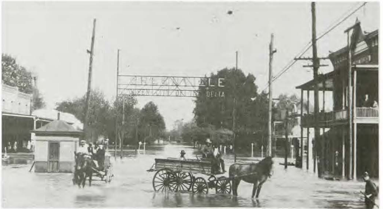
Greenville, Mississippi, the "Queen City of the Delta," took the full force of the first levee break at Mound Landing
