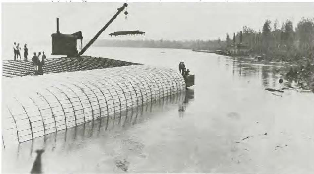
Concrete mat sinking plant in operation at Caulks Neck, Arkansas, October 1926
