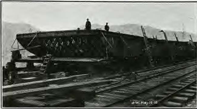
New steel barge for use in channel improvement
