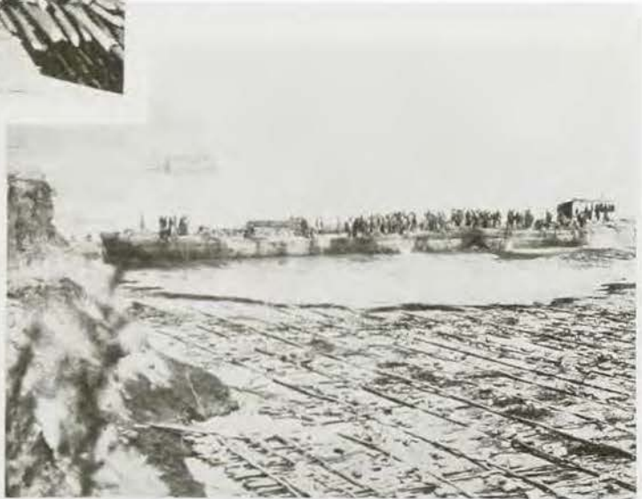
Rock is piled on floating mattress for ballast
