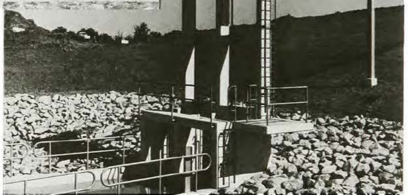
Snake Creek Drainage Structure
