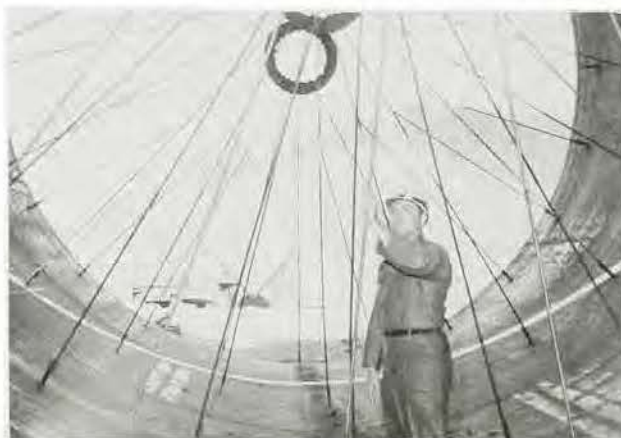
Early construction at DeGray Dam on the Caddo River
