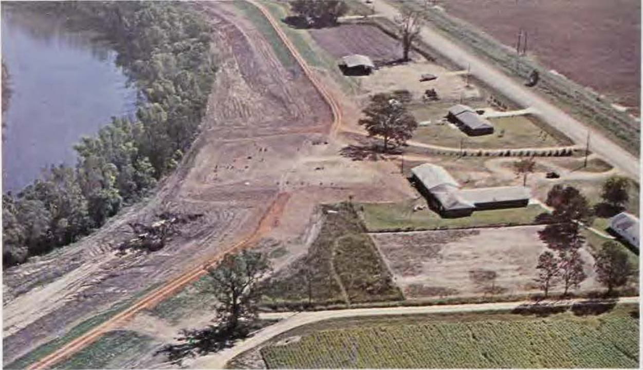
In central Louisiana, the Corps worked with the locals to put a levee through a church cemetery. The tombstones were surveyed and raised to the height of the levee, directly above their original location
