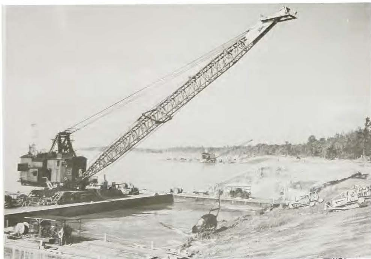
Clearing and grading operations
