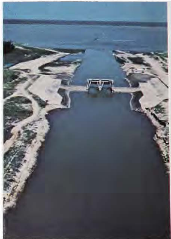
Catahoula Lake in Louisiana and water level control structure
