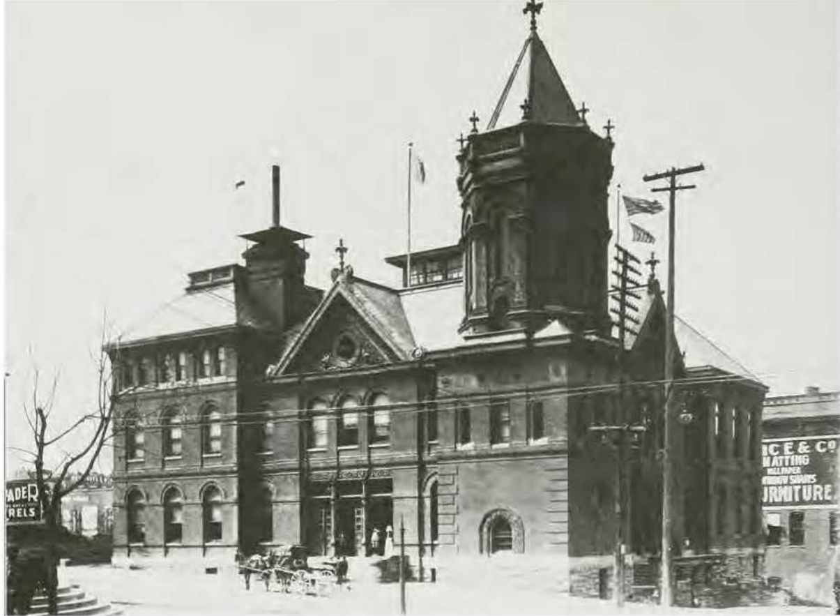
The "new" Post Office and Customs Building housed several Federal offices but the Corps of Engineers could only squeeze out attic space for their offices and working area
