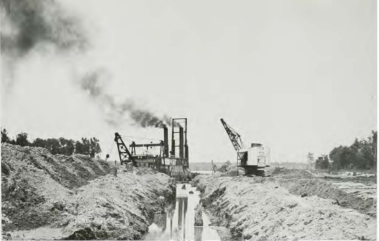
Cutterhead dredge constructing a cutoff on the Mississippi River (in background) at Caulks Neck, approximately 20 miles above Greenville, Mississippi. Dragline was also used
