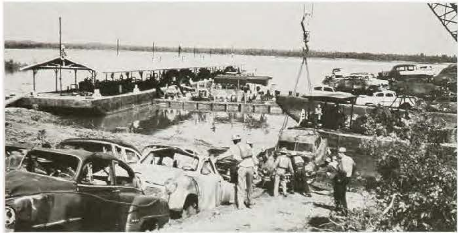
Experimental dike construction using junked automobile bodies
