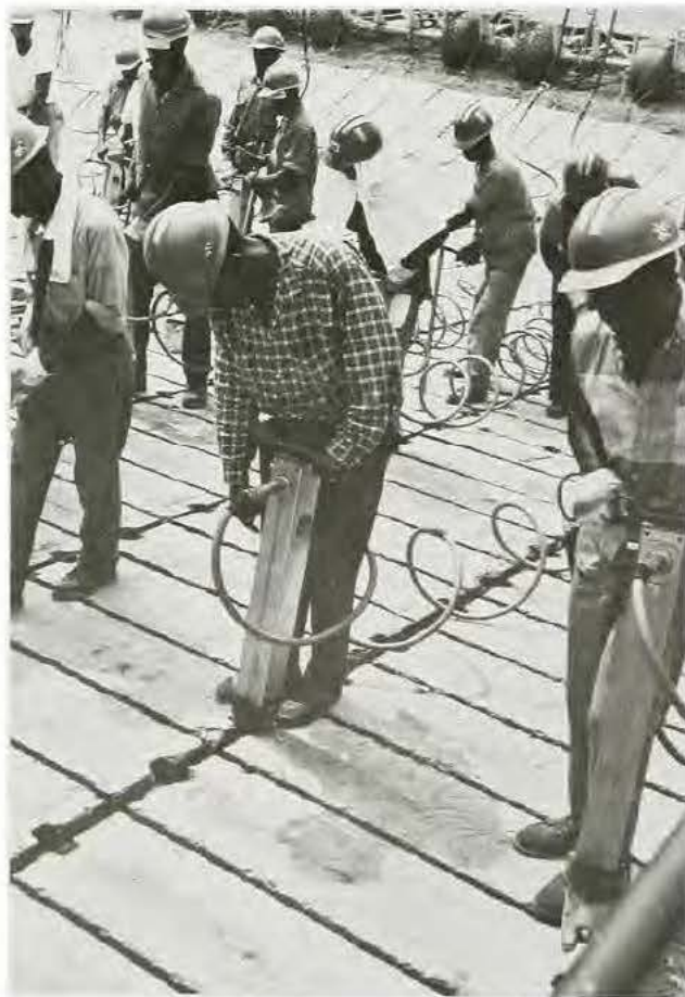
Linking concrete units by pneumatic tying machines make mat operations faster
