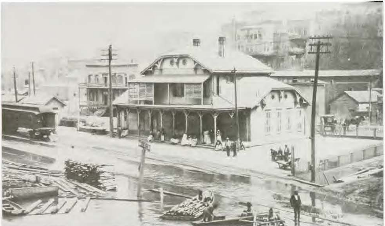
Floodwaters approach the city front at Vicksburg before construction of its first seawall
