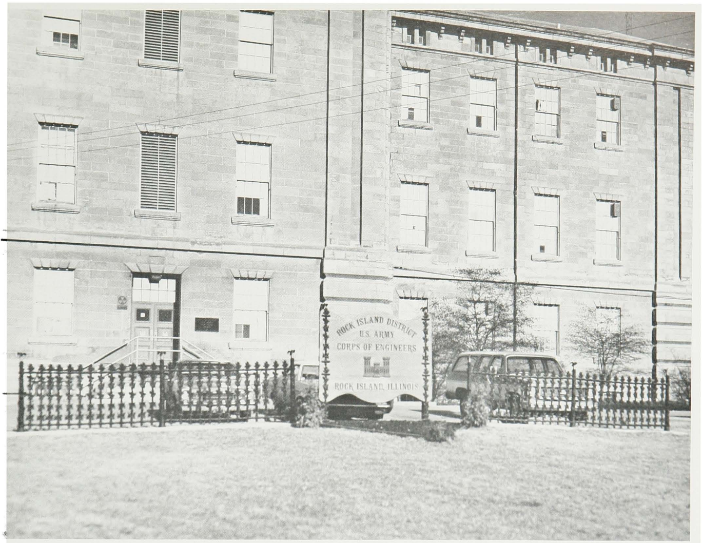
Fig. 22 Above. View of oak leaf design fence with American Eagles on top. This fence was built from Civil War cannonballs in 1870.
