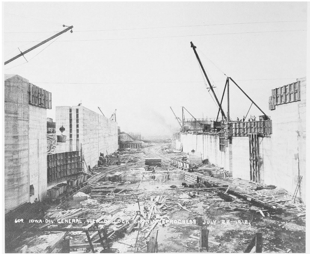
Fig. 3. Construction of Old Keokuk Lock, taken in July 1912.
