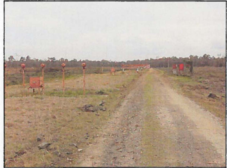
Runway 03 facing south at cleared safety zone along approach lighting to be removed as part of the 1,000 by 2,000-foot graded area.
