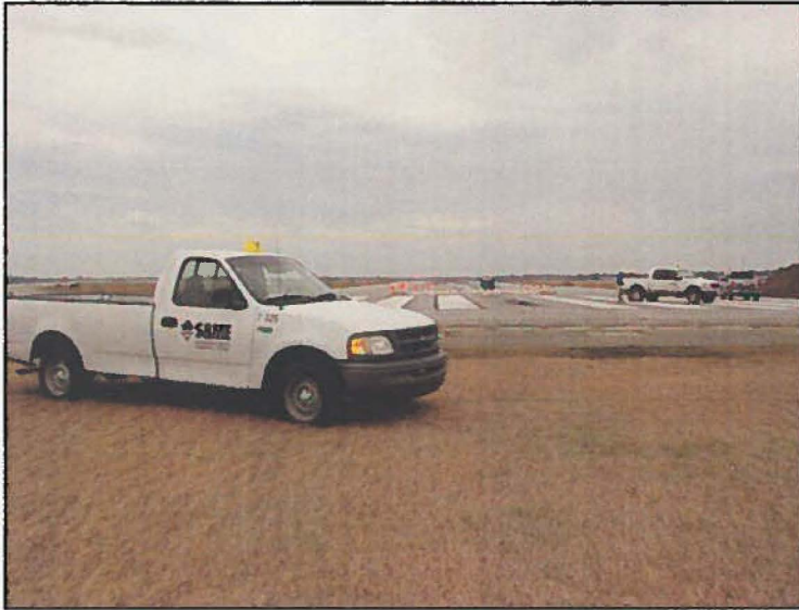
Runway 21 existing runway end.
