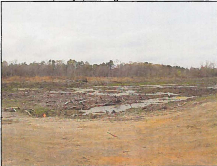
Runway 03, cleared safety zone to be graded as part of the 1,000 by 2,000-foot graded area.
