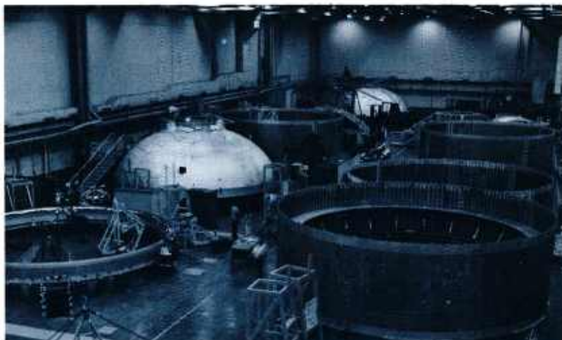
FIGURE 116 Skin sections & bulkheads
