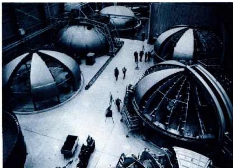
FIGURE 118 Construction of bulkheads
