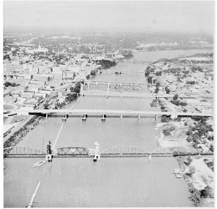
Six bridges at Little Rock needed altering or replacement to accommodate modern barge traffic on the McClellan-Kerr Arkansas River Navigation System. In all, 16 bridges in the District were to be altered or replaced.
