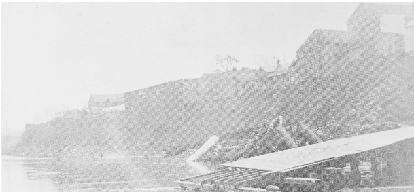
By 1900 the Arkansas River banks had eroded to the foundations of buildings in downtown Pine Bluff, Arkansas.
