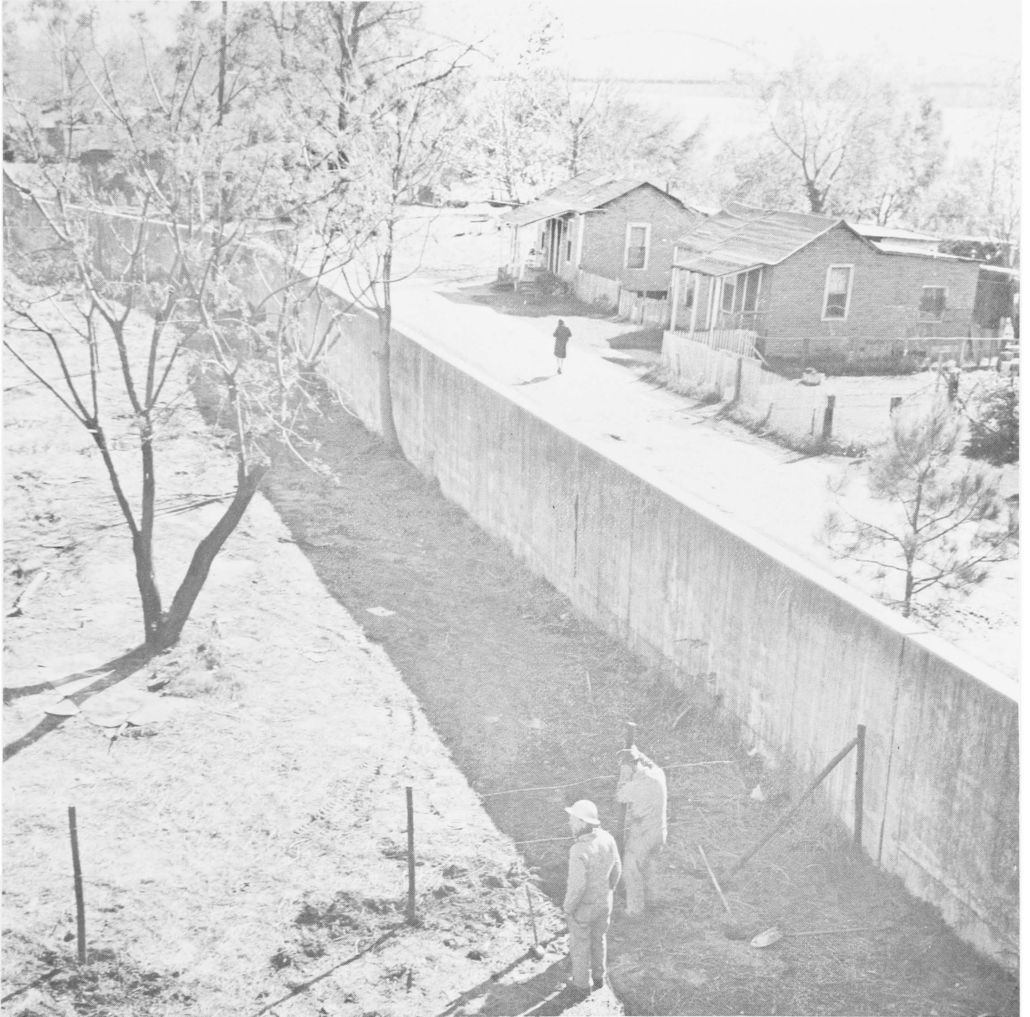
Floodwall at North Little Rock on the Arkansas River.
