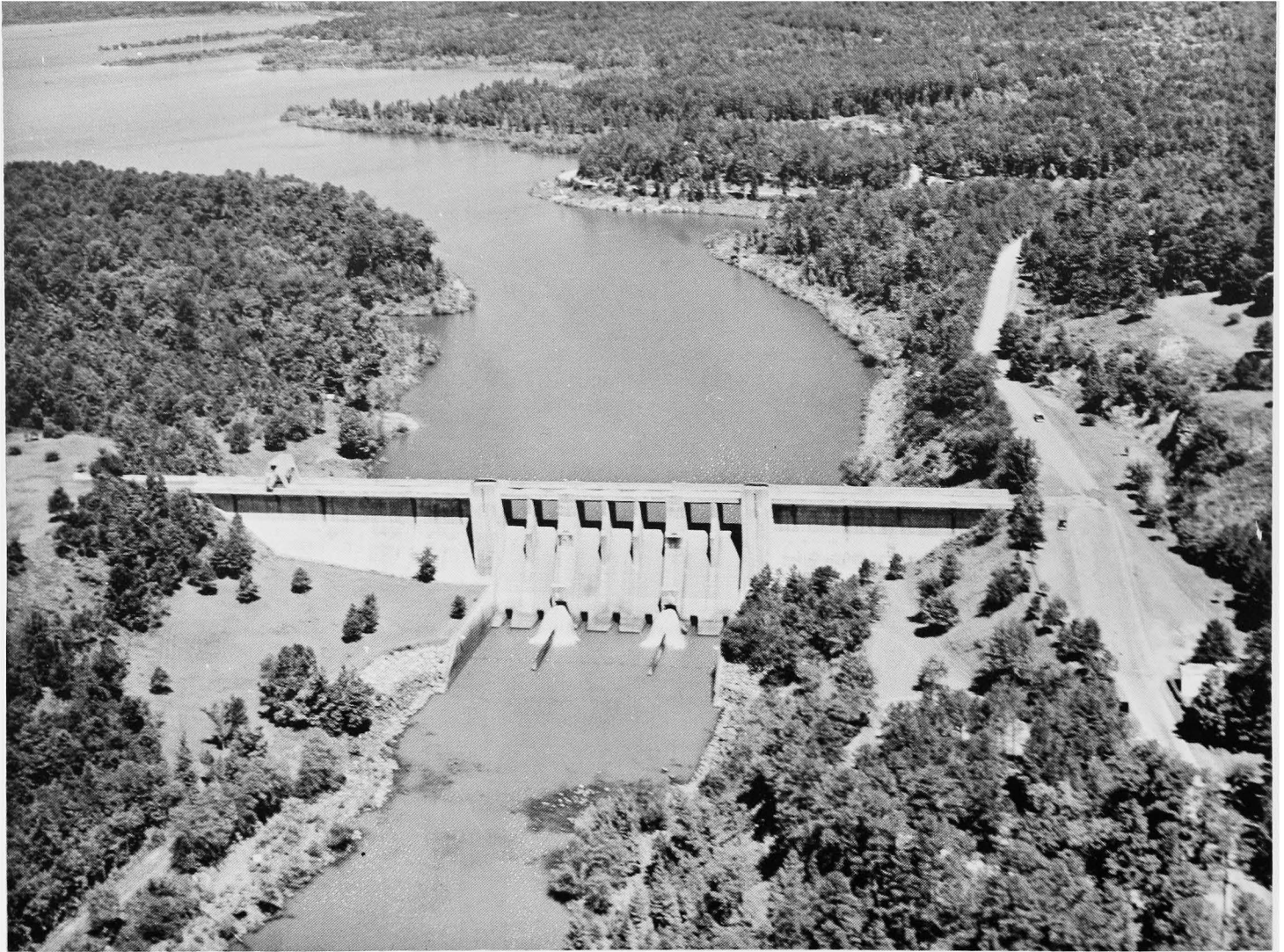
Nimrod Dam on the Fourche La Fave River near Ola, Arkansas.
