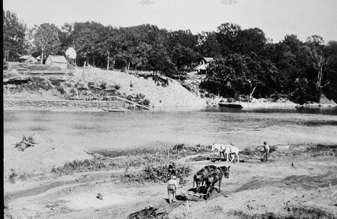
Excavation of abutment, Lock No. 1, White River.
