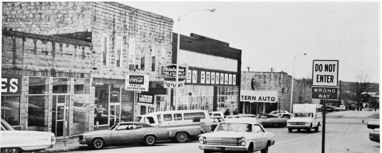
The south side of the public square, Mountain Home, Arkansas 1971.
