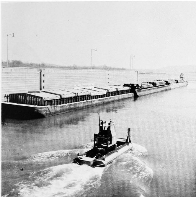
The First shipment of butyl rubber passes through Murray Lock & Dam near Little Rock on the Arkansas River in April 1971.
