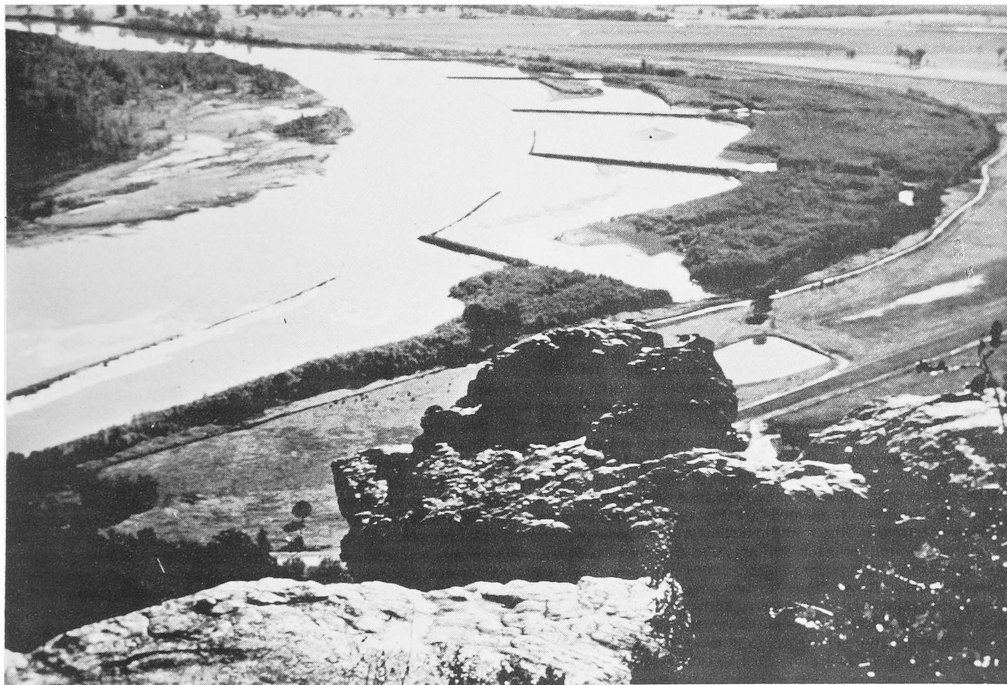
Bank Stabilization on the Arkansas River keep the meandering river within stable bounds.
