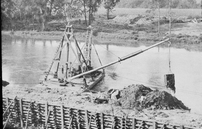
Removing excavations from lock pit, Lock No. 1, White River.
