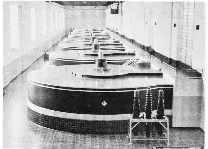
Generator Floor in Bull Shoals Dam powerhouse.
