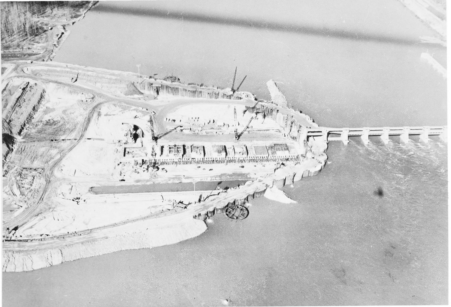
Second stage cofferdam protects construction area of Lock & Dam No. 3 on the Arkansas River near Swan Lake, Arkansas. February 1968.
