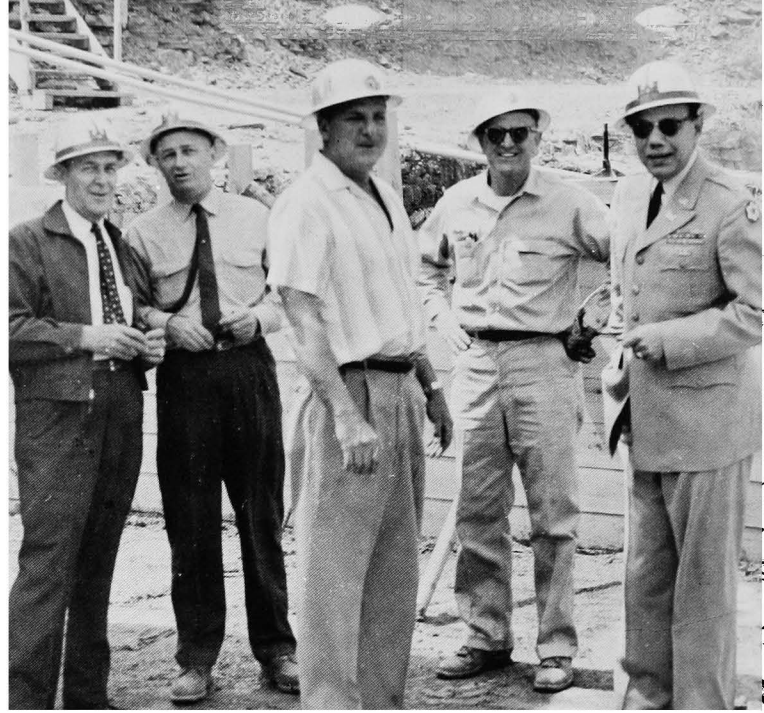
First concrete was placed in Greers Ferry Dam on April 11, 1960. Present were, left to right: W. W. Ralphe, Chief, Construction Division; Lincoln F. Sherman, Resident Engineer; P. J. Soukup, Superintendent and W. Wixon, both of Red River Builders; and Colonel A. M. Jacoby, District Engineer.
