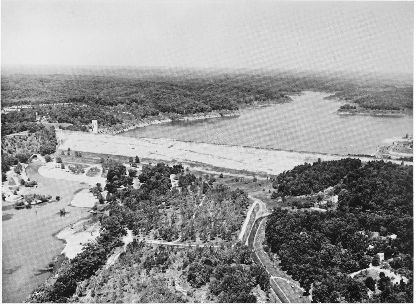
Clearwater Dam on the Black River near Piedmont, Missouri.
