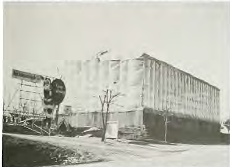
Winterization of a two-story BOQ, Camp Humphreys
