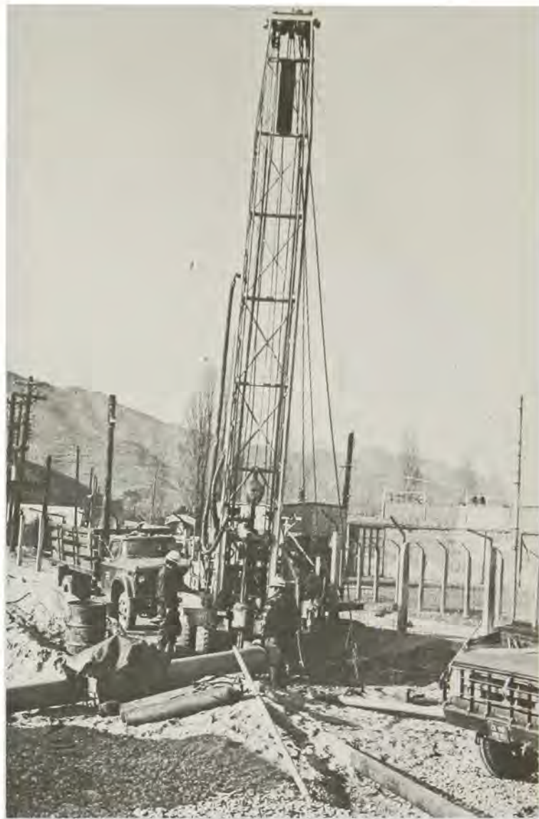
New well at Camp Casey
