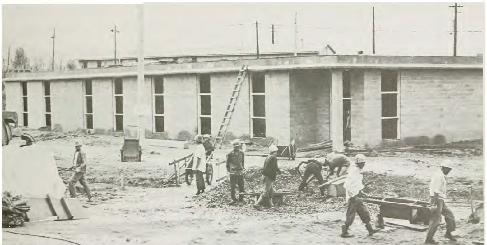
500 man mess hall project, Camp Red Cloud
