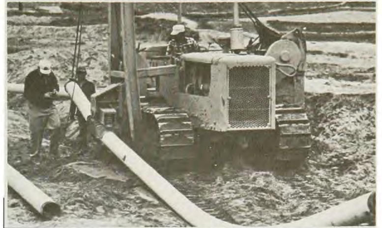
Bending coated pipe to conform with variations in the course of the pipeline
