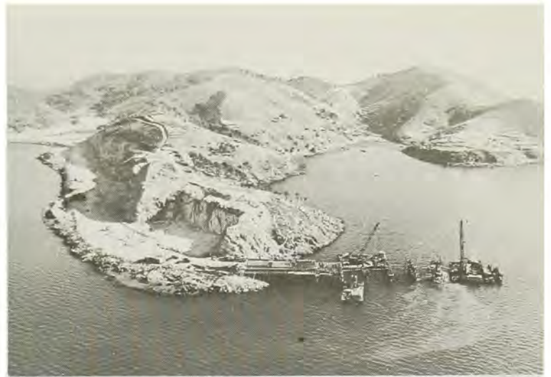
Chinhae ammunition pier project underway, significant amounts of rock have already been blasted and tons of fill added to create a work area adjacent to the wharf
