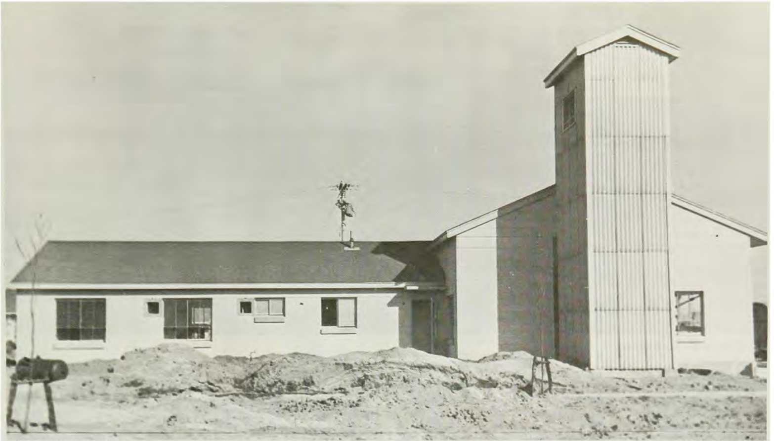
Fire station, Chitose
