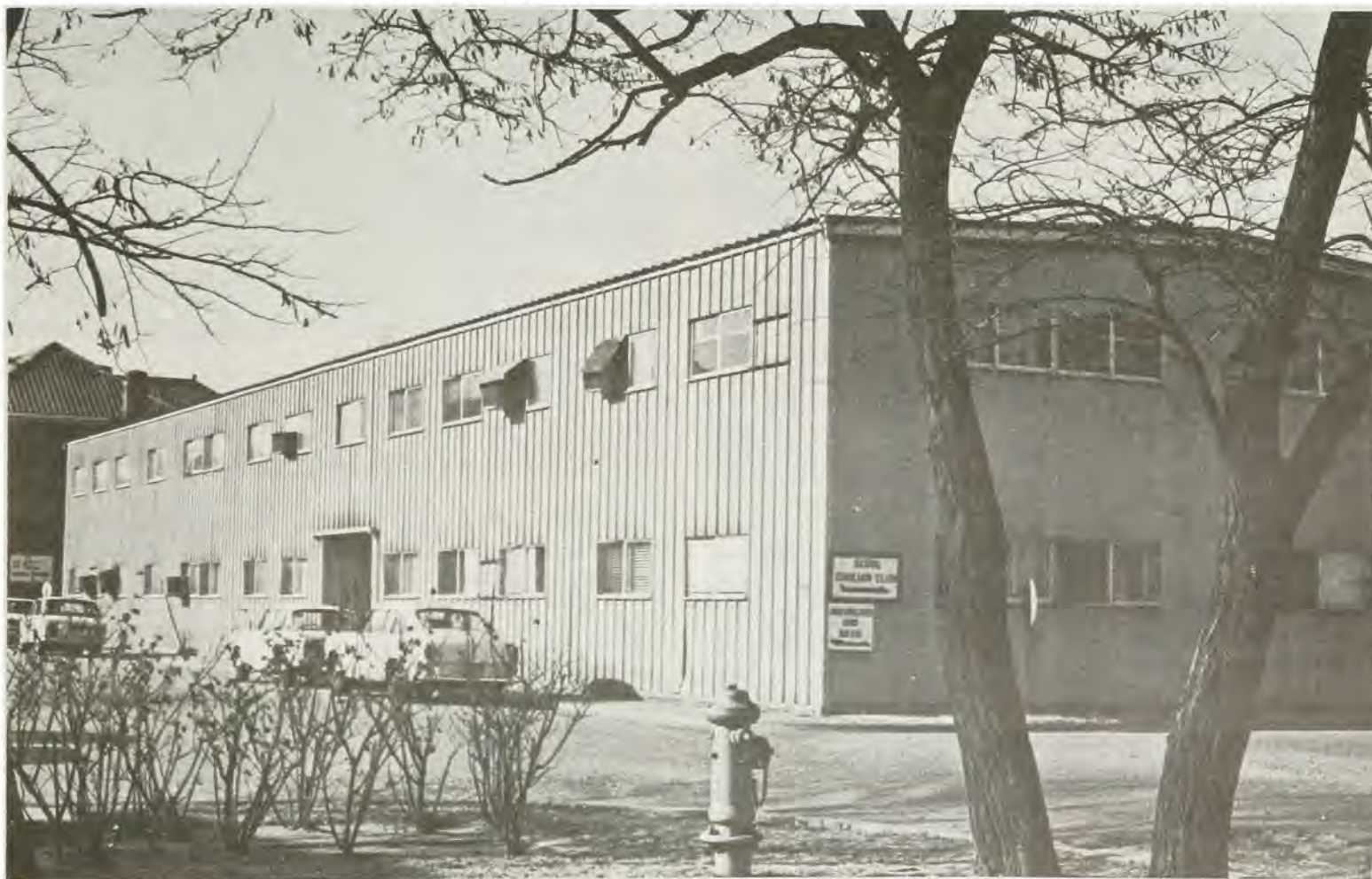
Pre-engineered office building, FED Compound, Seoul
