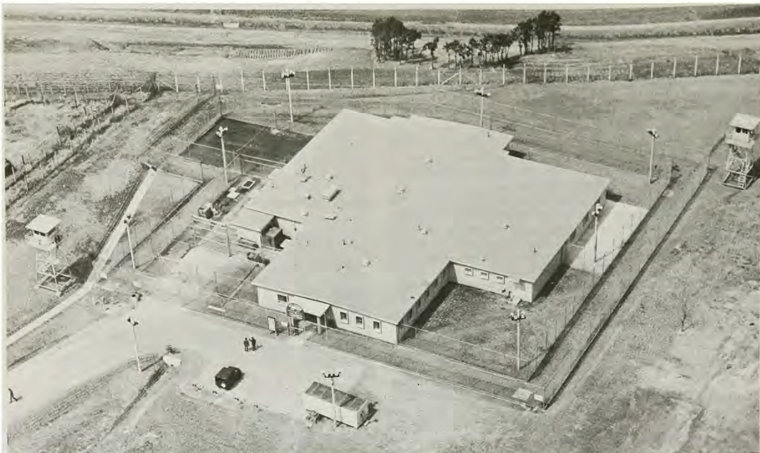
Recent view of Camp Humphreys confinement facility
