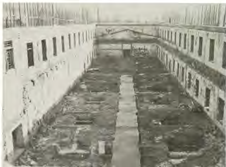
Fire-gutted Building 2212, Seoul
