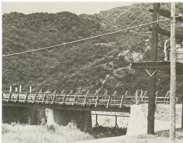
Camp Hovey bridge scheduled for replacement
