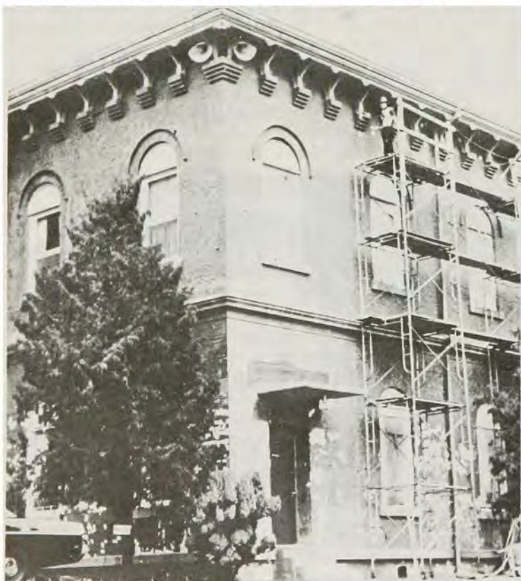
Exterior segment of JUSMAG-K building renovation, Seoul
