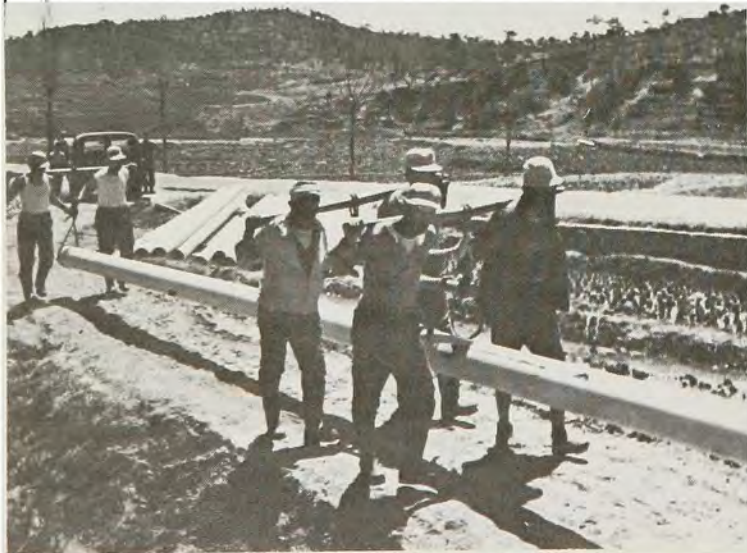
Laborers transporting the easily damaged pipe
