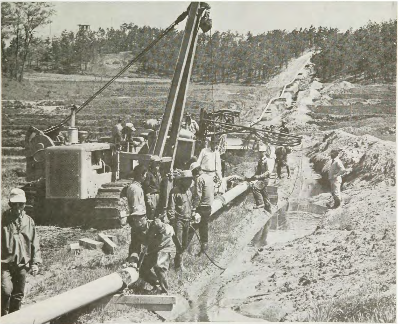
Laying of pipe for trans-Korea POL pipeline
