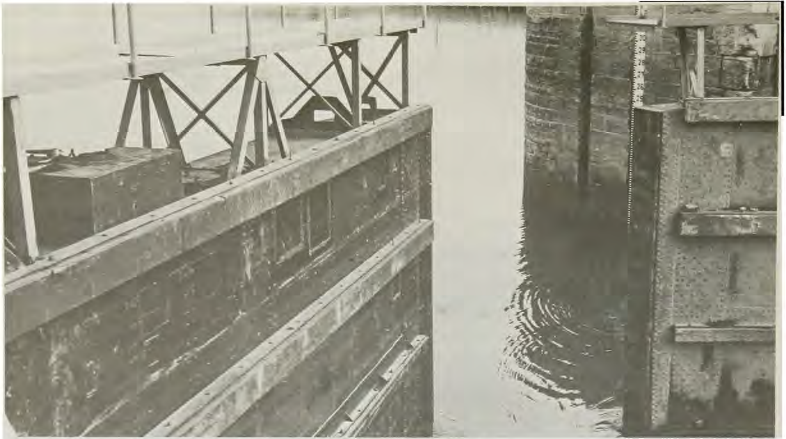
Completed Inchon Tidal Basin rehabilitation as seen through partially open mitre gates
