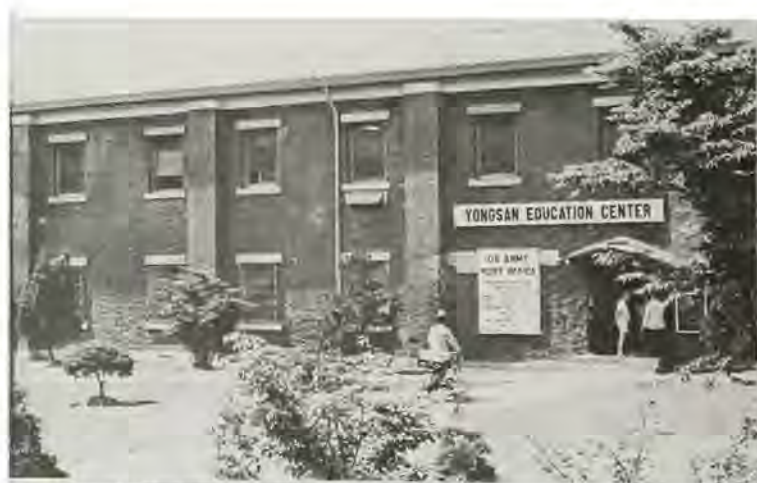
Building 2212 after restoration, Seoul
