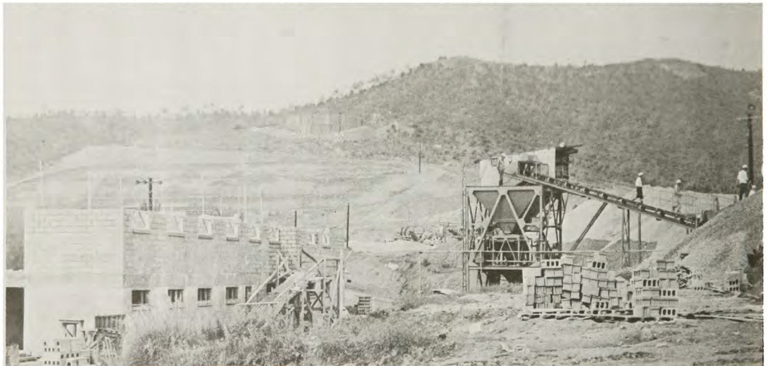
BOQ under construction, S&T Battalion, contractor's central concrete batch plant on right
