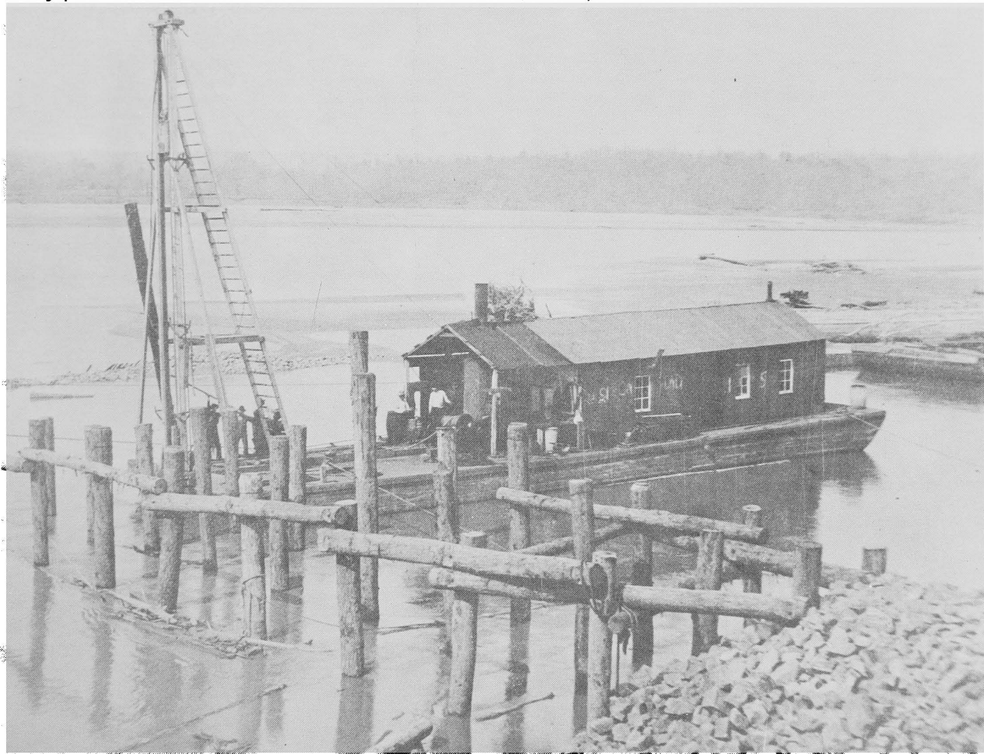
Driving pile on the Arkansas River at Lower Greathouse Bend near Little Rock, March 1900.
