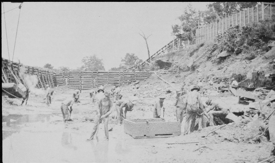
Excavation of Lock No. 1 near Batesville on the White River in 1900.
