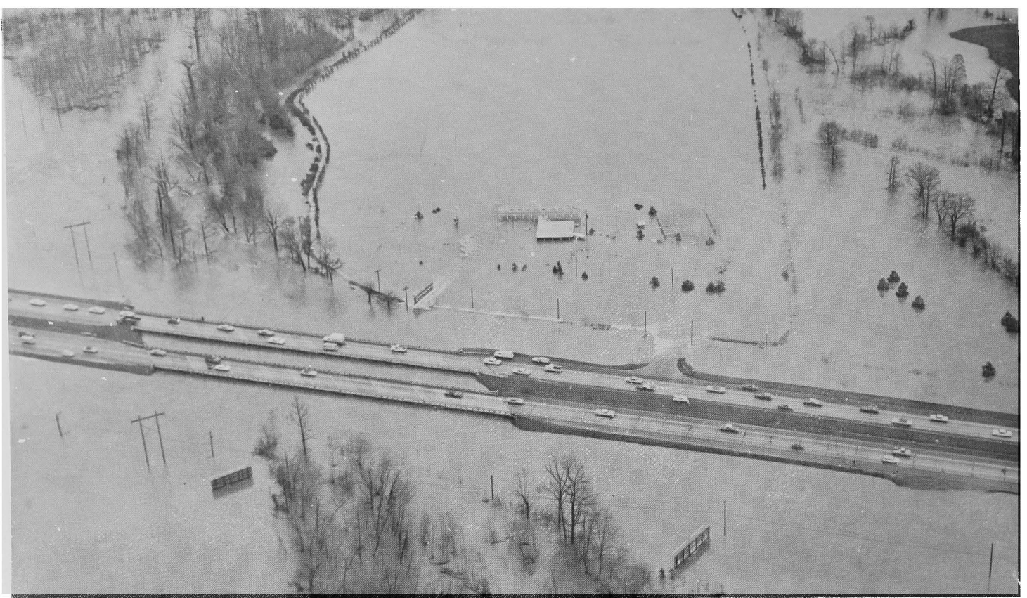
Fourche Creek floods at Little Rock in January 1969. City and county officials called upon the District for assistance.
