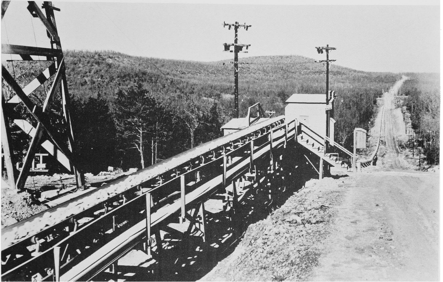
Seven-mile long conveyor system supplied material from quarry to Bull Shoals damsite. December 1948.
