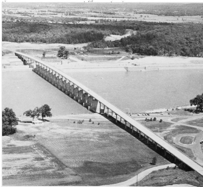
Toad Suck Ferry Lock and Dam, near Conway, Arkansas. A bridge was built over this dam in 1971, similar to the structure completed over Lock and Dam 13 in 1978.
