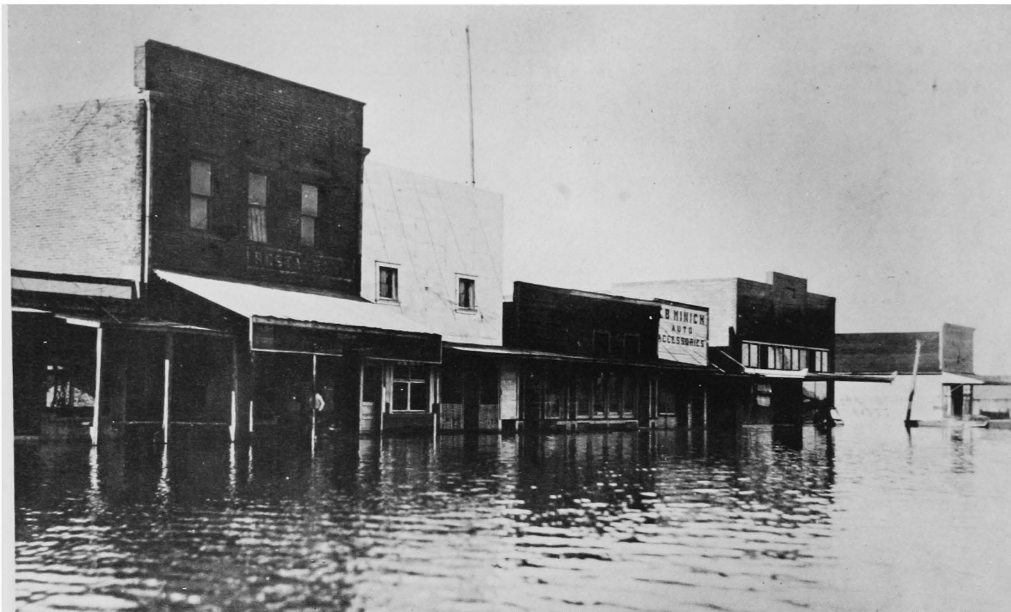
1927 Flood of the Arkansas River covered Main Street of Gillette, Arkansas. Gauge was 28.9 feet on April 27.
