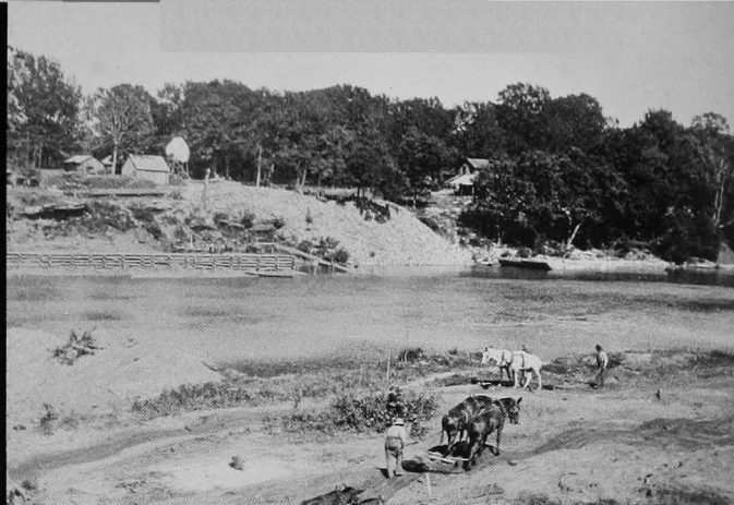
Excavation of abutment, Lock No. 1, White River.
