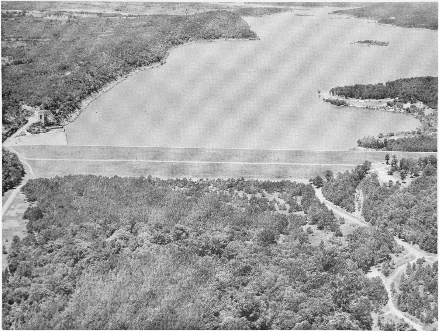
Blue Mountain Dam on the Petit Jean River near Waveland, Arkansas.
