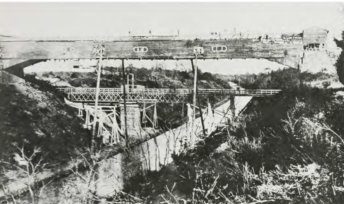
The original Summit Bridge was built in 1826 before the channel cutting was made. It spanned the canal across the "Deep Cut," 247 feet between abutments, 90 feet above the canal bottom. In this 1872 photograph the first Summit Bridge is being dismantled and its replacement is nearing completion just beyond.
