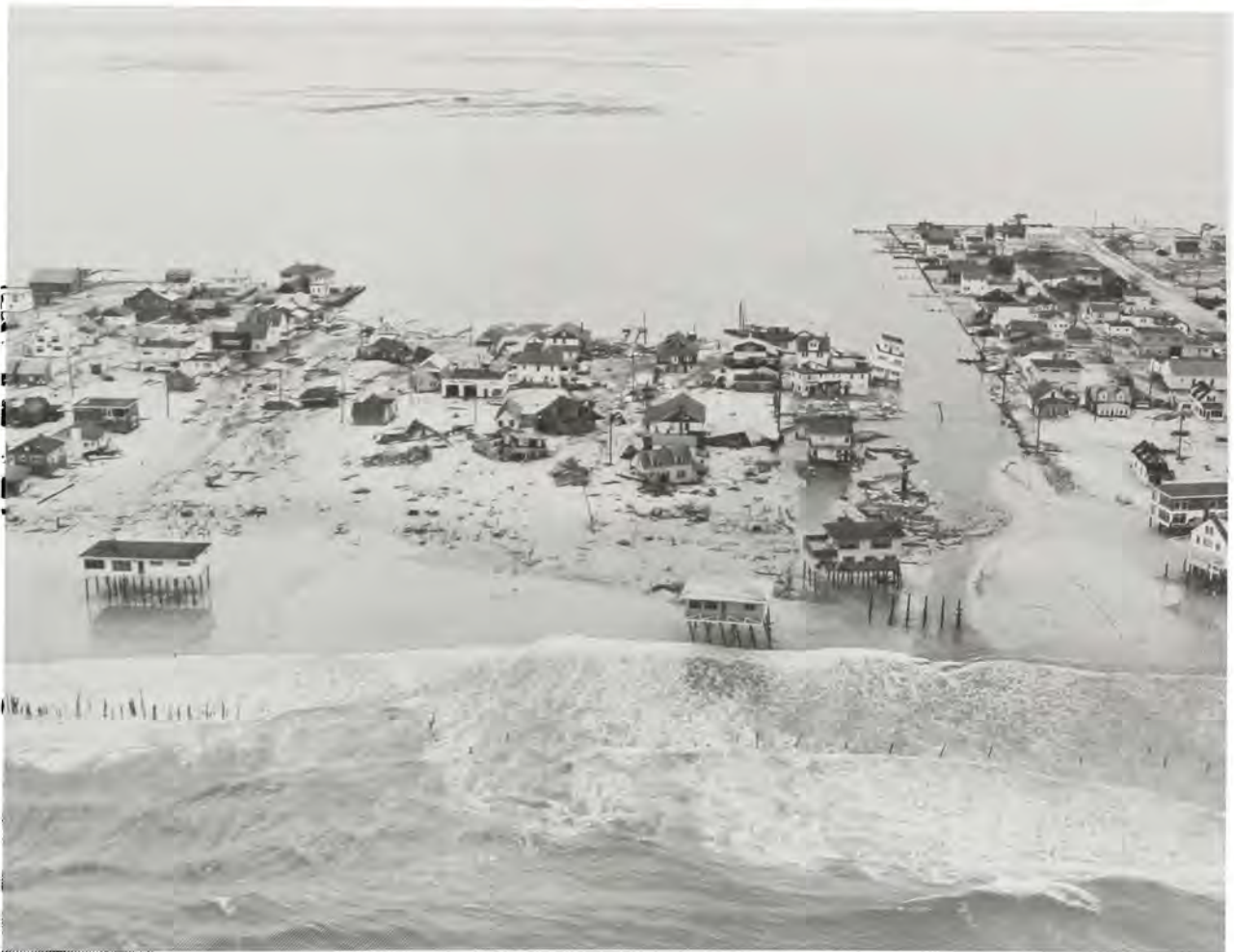
Major breach at Harvey Cedars. "Five-High" storm.
