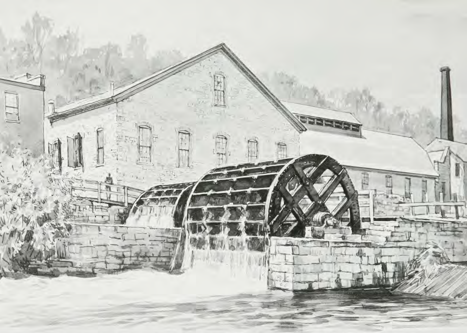
In 1830 power and lift wheels were installed at Union Mill to take water from the river and feed it into the Delaware Canal. Wells Falls was at this point, one mile below New Hope.
