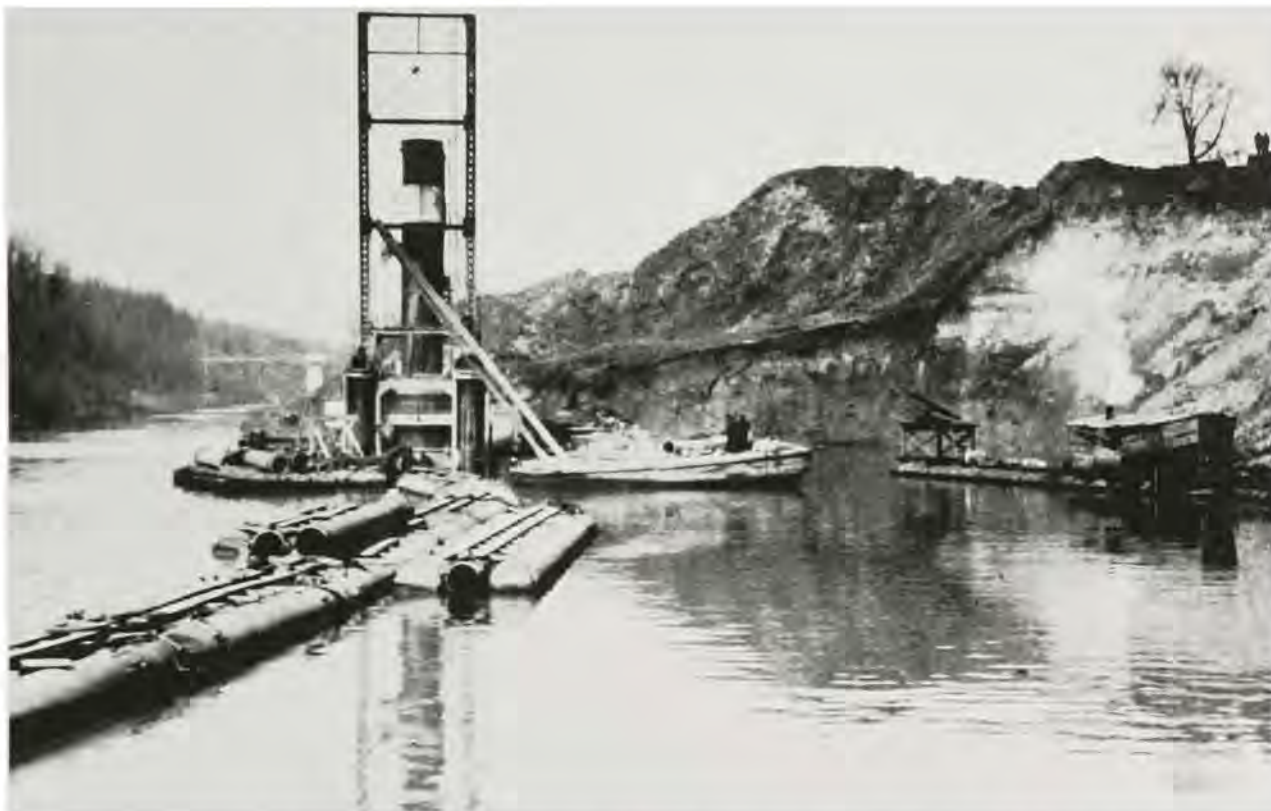
Chesapeake and Delaware Canal conversion to sea-level waterway, 1924. Hydraulic pipeline dredge is excavating in the Deep Cut east of Summit Bridge.
