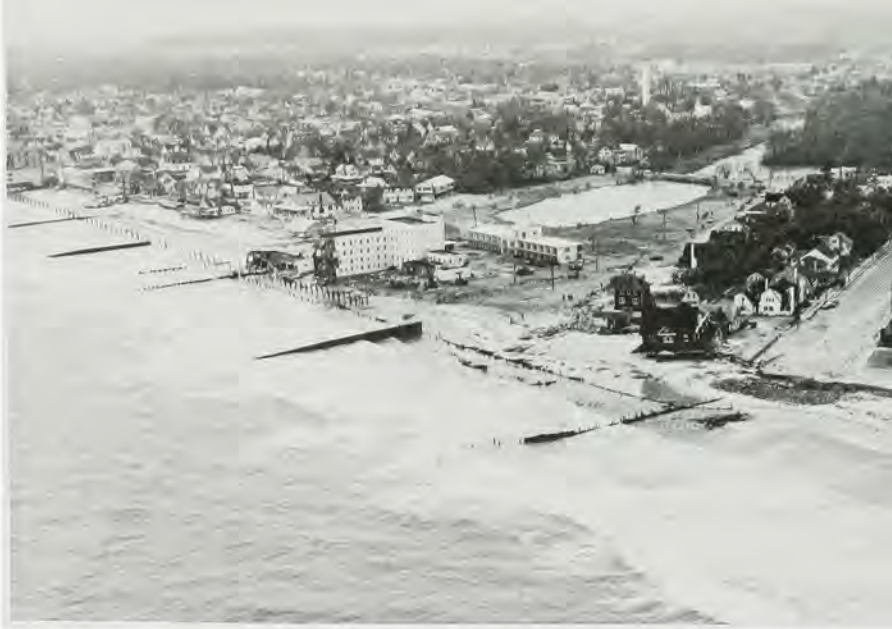
Timber groins at Rehoboth Beach, Delaware. Damage to shore-front properties was caused by the "Five-High" storm of March, 1962.
