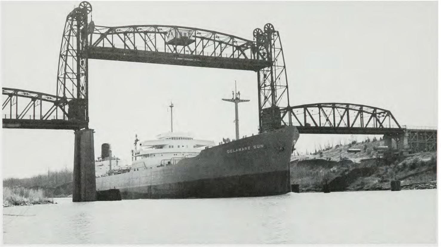
The third bridge at Summit, Delaware was a vertical lift iron bridge with a horizontal clearance of 190 feet between piers and 140-foot vertical clearance at mean low water, span up. Its design was similar to that of four other lift bridges, constructed when the Chesapeake and Delaware Canal was converted to a sea level waterway.
