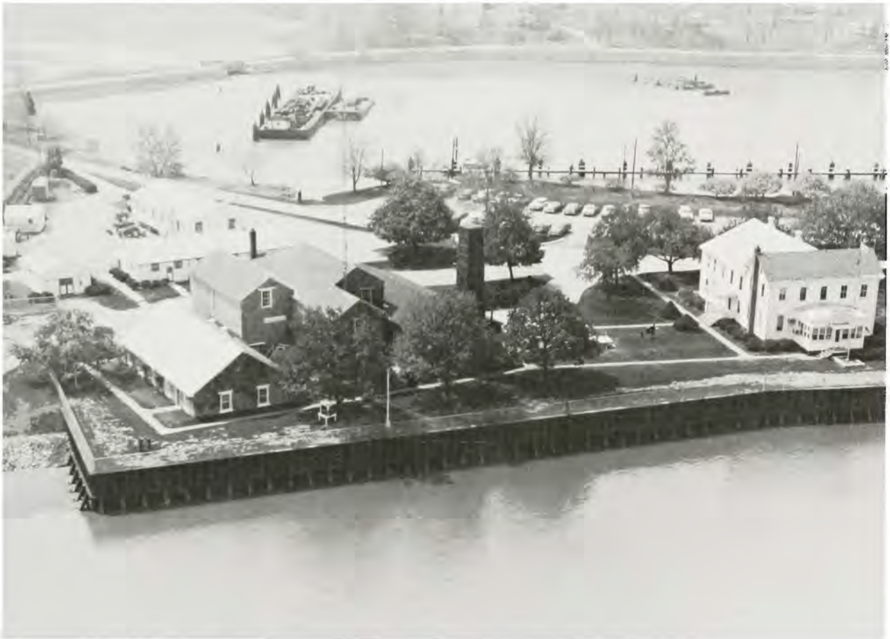
1969 view shows the edge of the sea-level canal within 40 feet of the pumphouse, its surface 14 feet lower than the old lock canal. The waters of Back Creek in the background which were once channeled into the wheelhouse and pumped up to the canal's summit level, now serve as a depot anchorage. The buildings have been designated a National Historic Site and function as a museum, in which the old liftwheel and beam engines are preserved.
