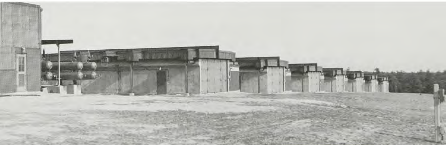
Bomarc installation at New Egypt, New Jersey, with missile launching structures and powerplant.
