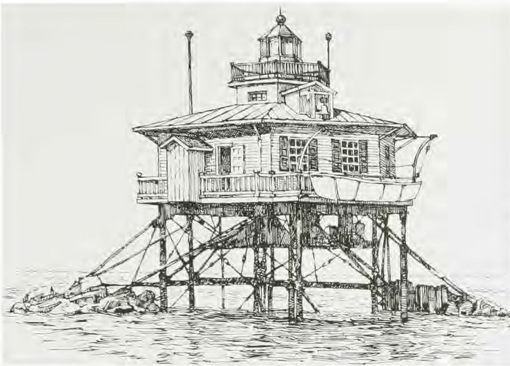
Wrought iron screw pile construction was typical for lighthouses in Chesapeake and Delaware Bays. This is Windmill Point Light at the mouth of Rappahannock River.
