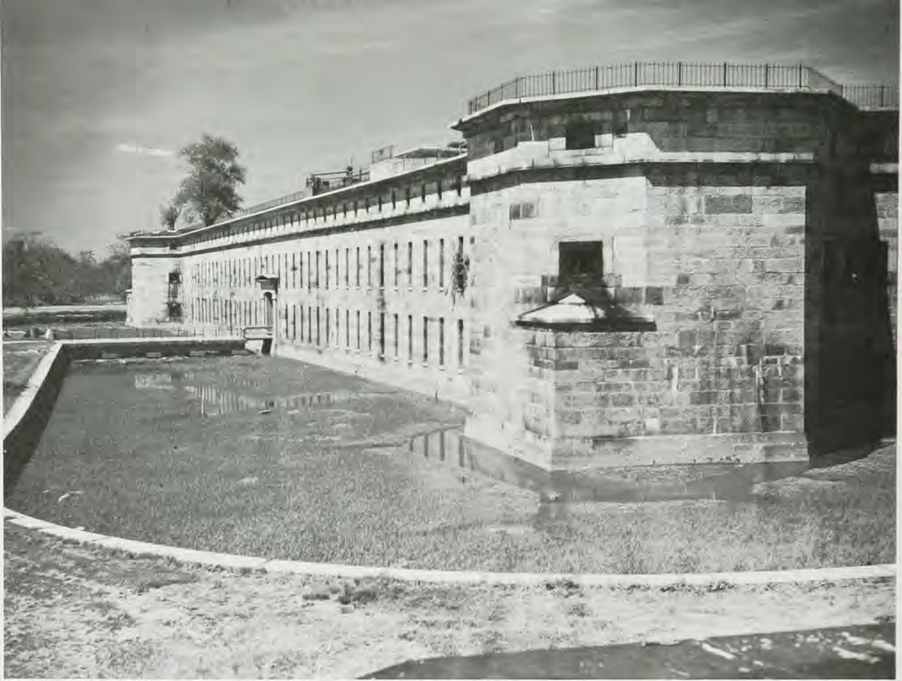
In Fort Delaware's twelfth decade, marsh grass chokes the moat and trees flourish on the ramparts, but the masonry shows signs of only minor subsidence. The superb mitering of the stone work is observable in this view of Front 5, with the permanent bridge, drawbridge and sally port. The State of Delaware and the Fort Delaware Society have begun restoration of the fort as a military museum.
