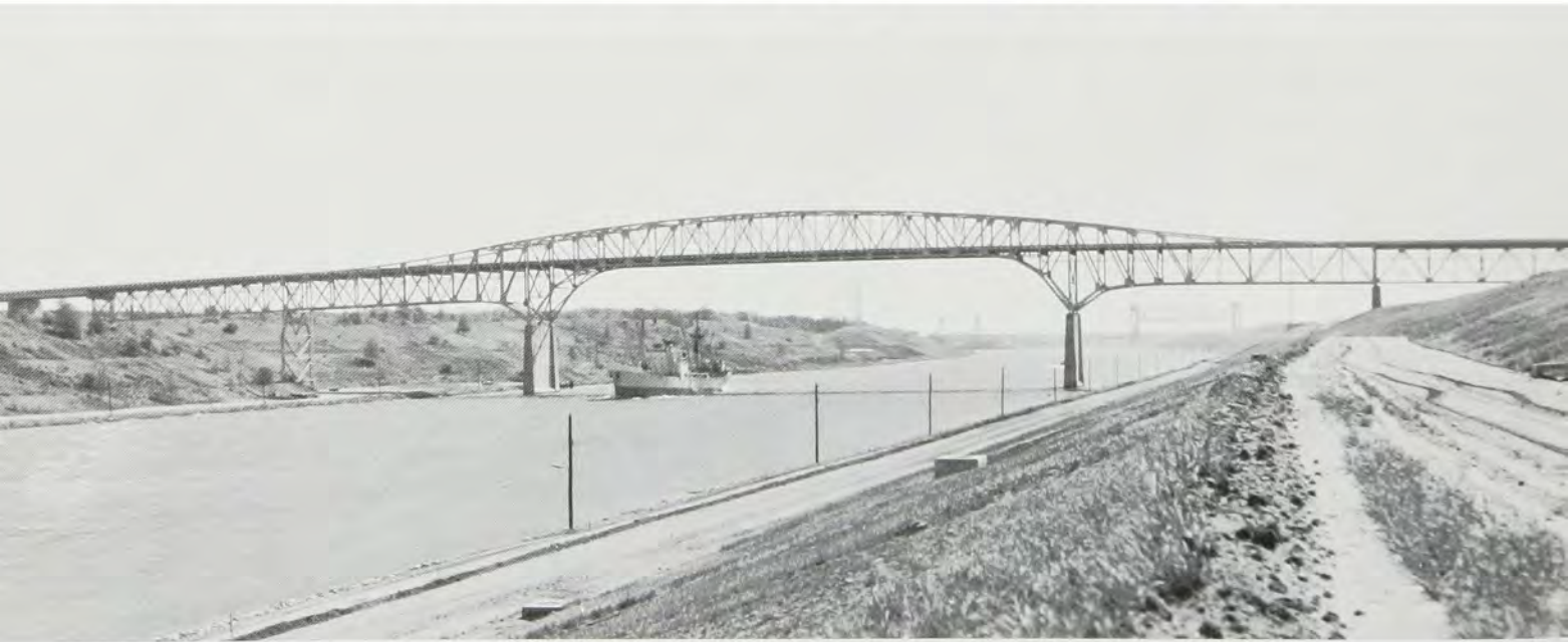
The high level Summit Bridge was opened to traffic in 1960. That year it received the “most beautiful bridge” award from the American Institute of Steel Construction. This fourth Summit Bridge spans the canal near the “Deep Cut” site of the original bridge, but the cut seems shallow with its terraced embankments and new width of 450 feet at the water line.
