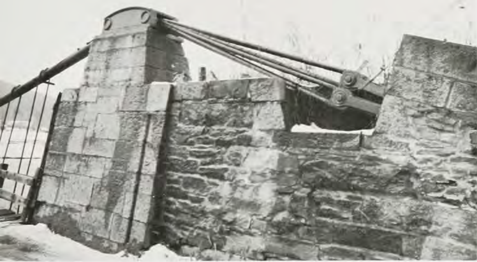
John Roebling designed the suspension aqueduct which carried the Delaware and Hudson Canal across the Delaware River at Lackawaxen, Pa. Built in 1847, it bore boat traffic until the canal was abandoned in 1898. Today, stripped of its wooden trunk, it serves as a link for vehicular traffic between New York and Pennsylvania.
