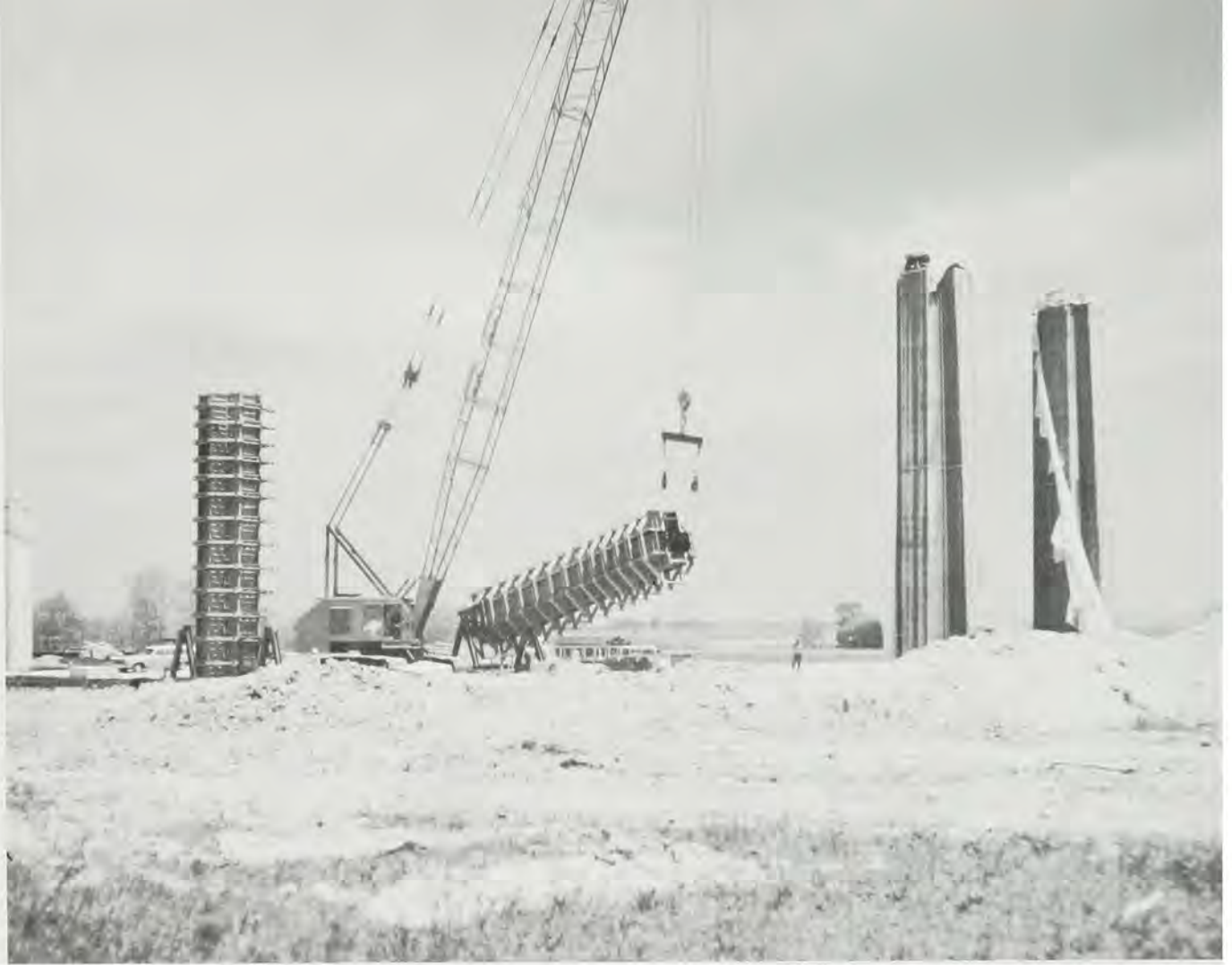
Construction of piers for Reedy Point high level bridge.
