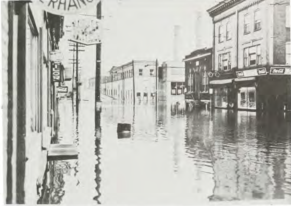
Waters of the Lehigh River in the streets of Bethlehem, Pa. Flood of May, 1942.
