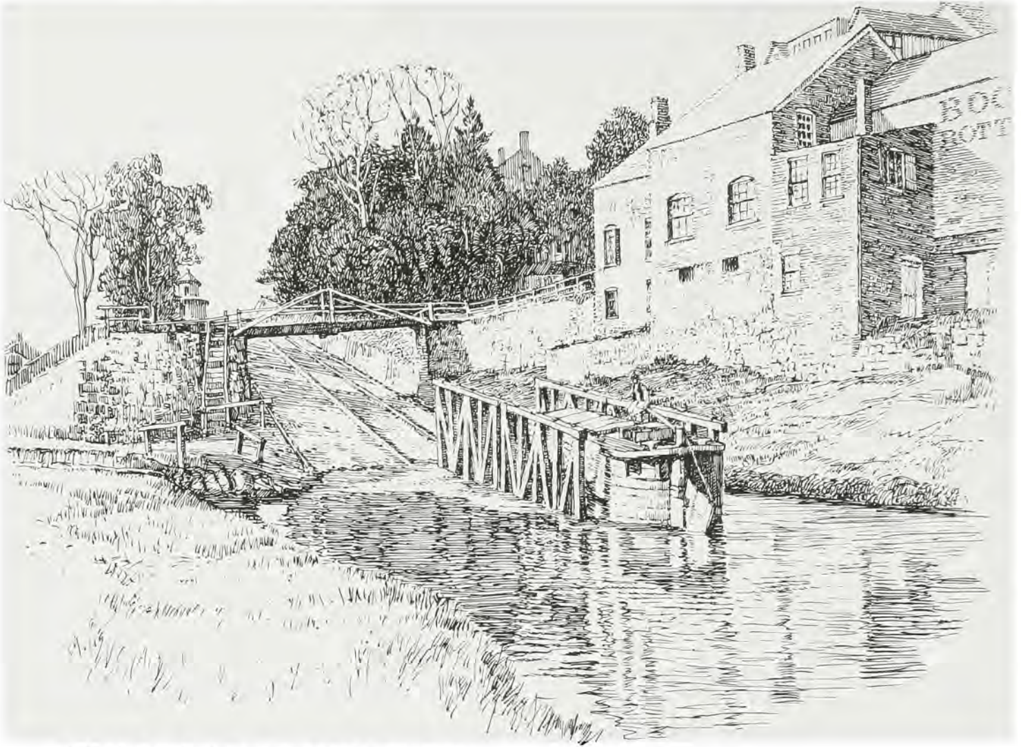
A freight boat begins the ascent of an inclined plane on the Morris Canal at Boonton, New Jersey. As an alternative to surmount this lift of 82 feet, nine or ten locks would have been required.
