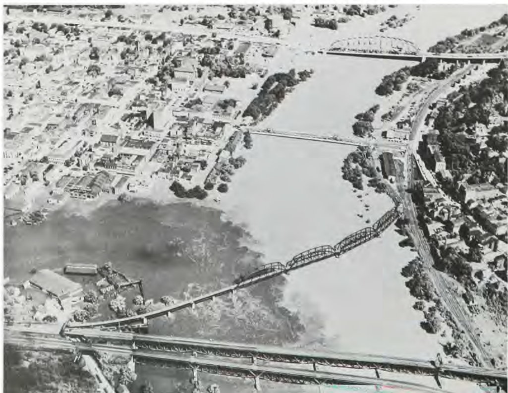
Flood of August 1955. Confluence of Lehigh and Delaware Rivers at Easton, Pa. and Phillipsburg, N.J.
