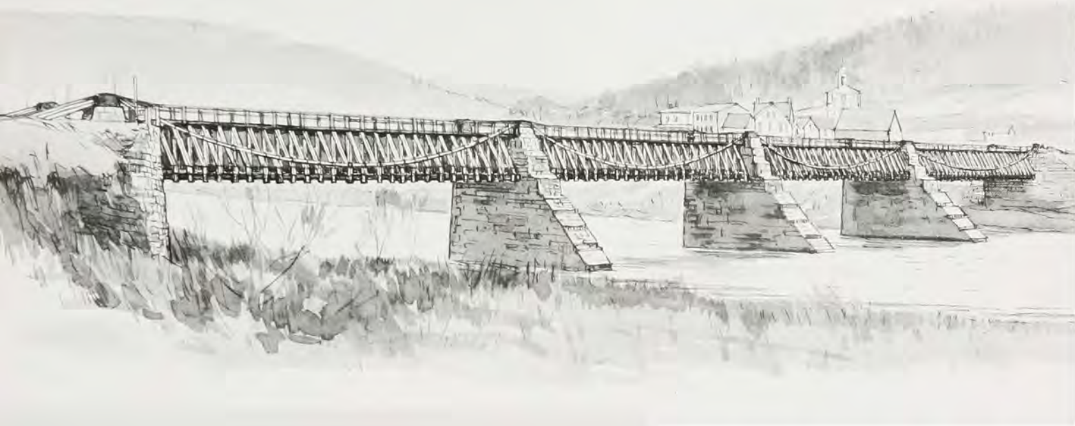
John Roebling designed the suspension aqueduct which carried the Delaware and Hudson Canal across the Delaware River at Lackawaxen, Pa. Built in 1847, it bore boat traffic until the canal was abandoned in 1898. Today, stripped of its wooden trunk, it serves as a link for vehicular traffic between New York and Pennsylvania.
