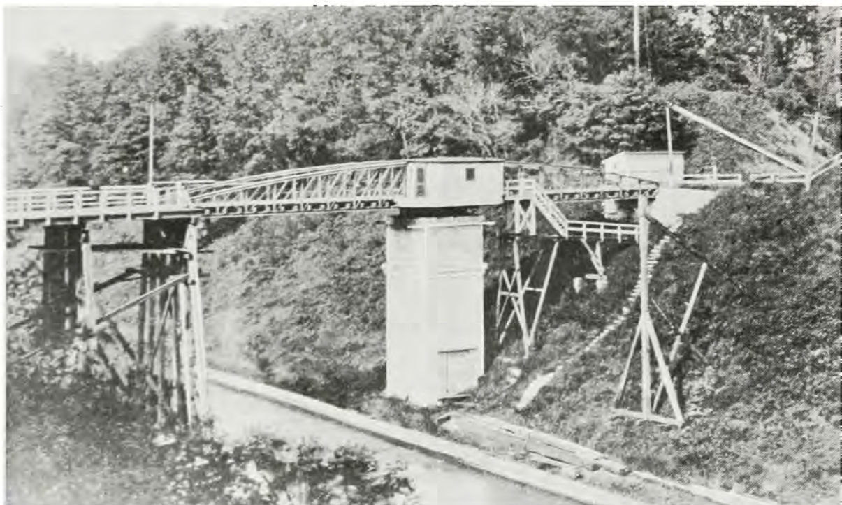
Summit Bridge No. 2 was this pivoting span, located a short distance eastward of the old covered bridge site. Also known as Buck Bridge, the structure was in service 55 years before giving way to the canal enlargement project of 1921-1927.
