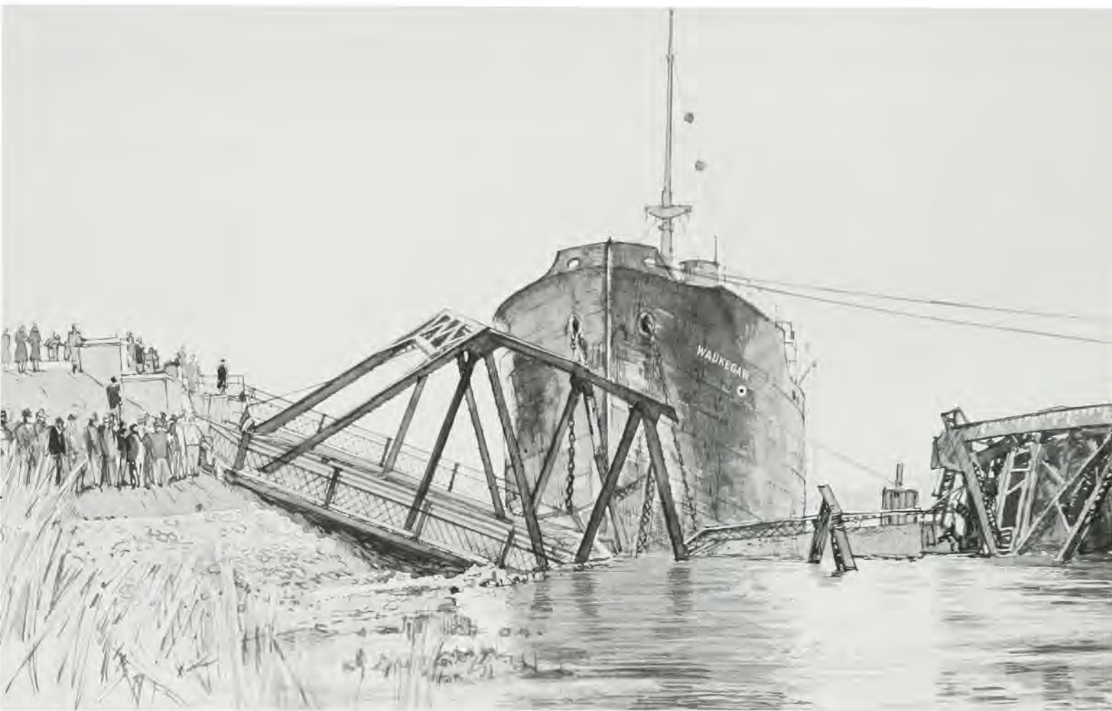
The S.S. Waukegan aground and jammed in the wreckage of St. Georges Bridge.
