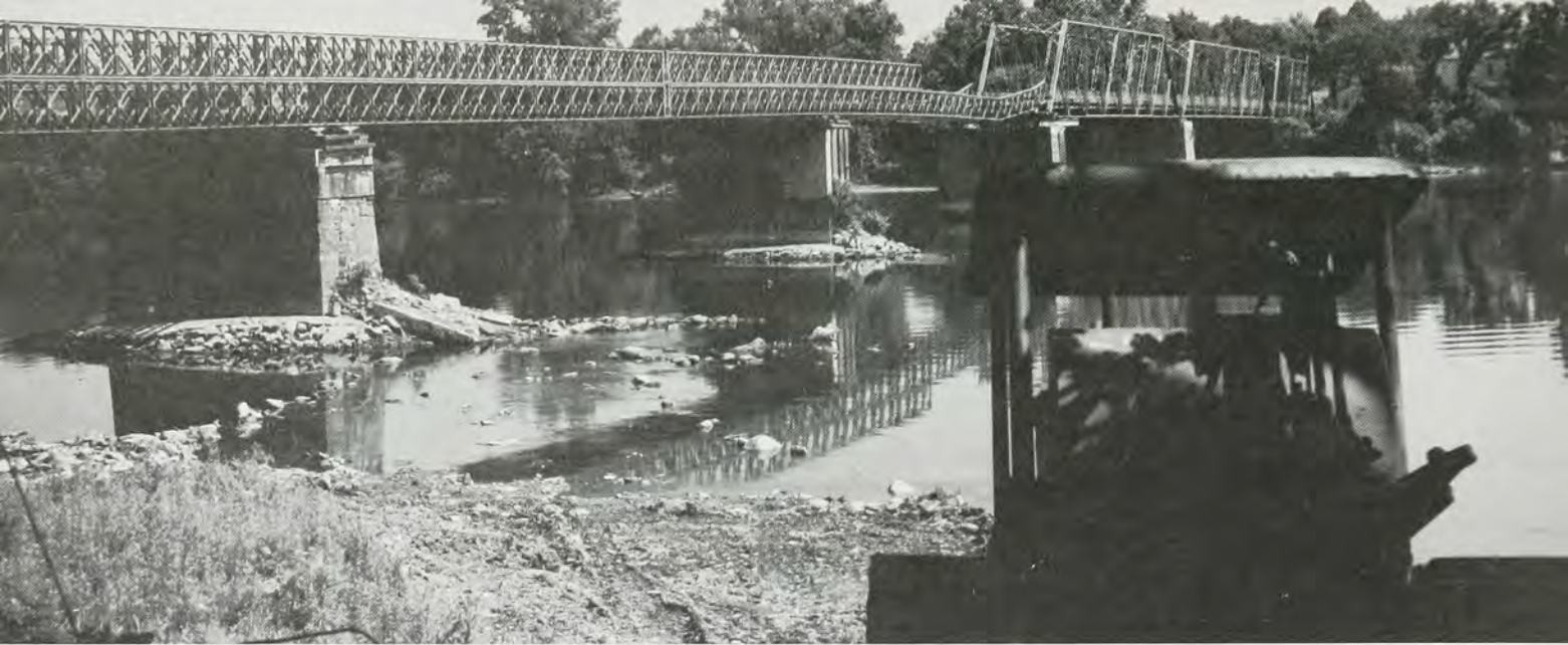
Two-lane Bailey Bridge constructed on piers of destroyed Yardley span.
