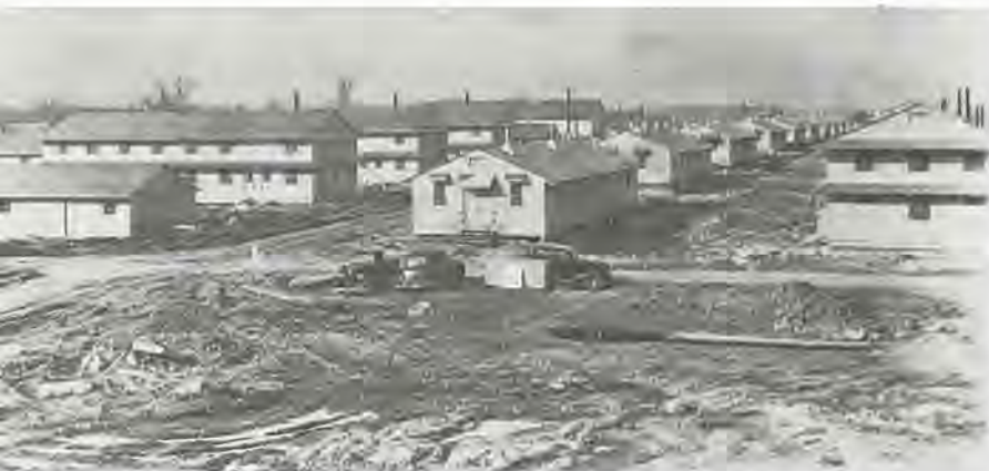
Wooden barracks construction, Fort Dix, New Jersey.
