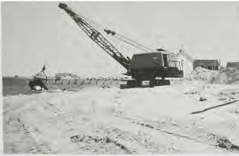
Dragline moving sand at Harvey Cedars. "Five-High" storm.
