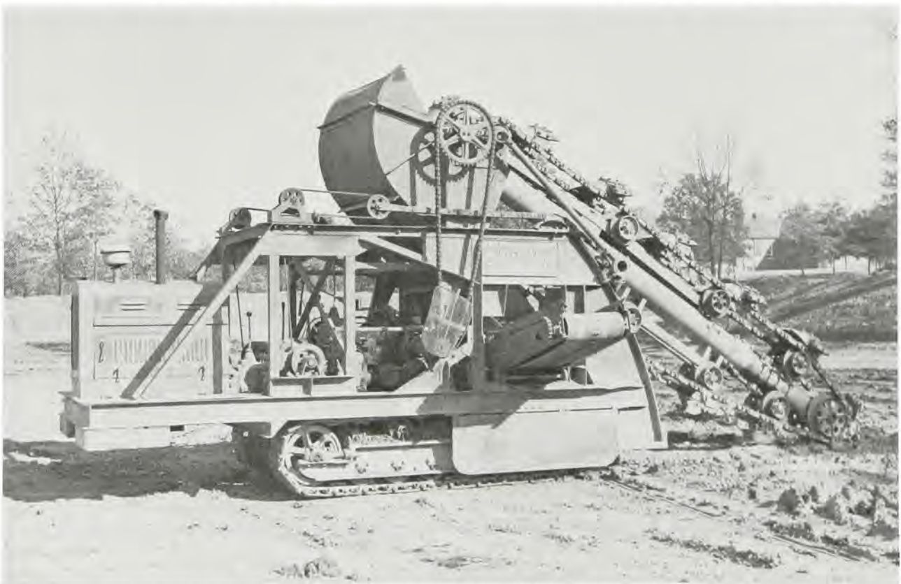
Experimental traction ditch digger weighed 20,000 lbs. and made 18-inch cut.
