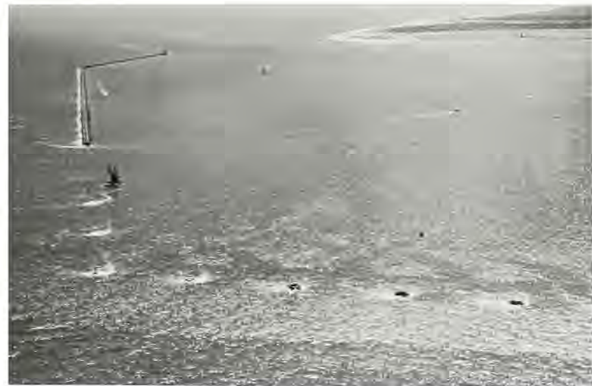
View southward of National Harbor of Refuge with its dog-legged breakwater at left and row of ice piers in the foreground. Distantly, to the right, Cape Henlopen and the old breakwater seem striving to meet.
