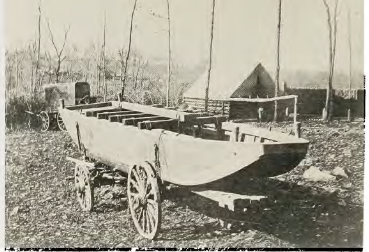
Ponton boat and wagon, 50th N.Y. Engineers, Rappahannock Station, Va. March 1864.
