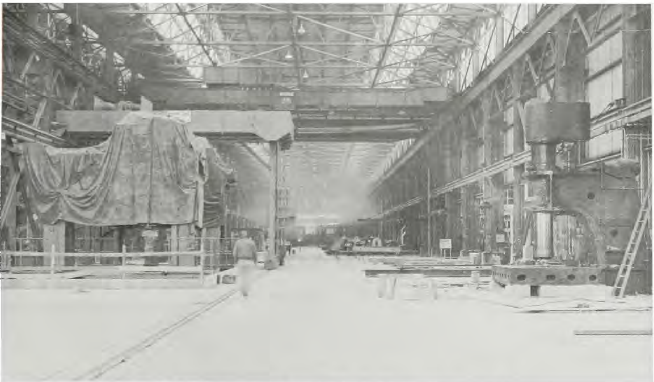
Birdsboro Foundry, the east bay looking west, January 1954.
