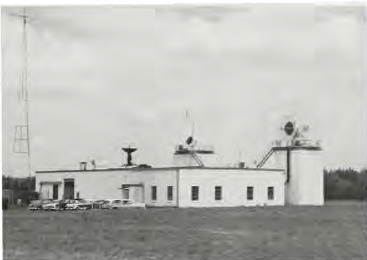
The D.A.M.P. (Downrange Army Missile Program) building at Moorestown, New Jersey.
