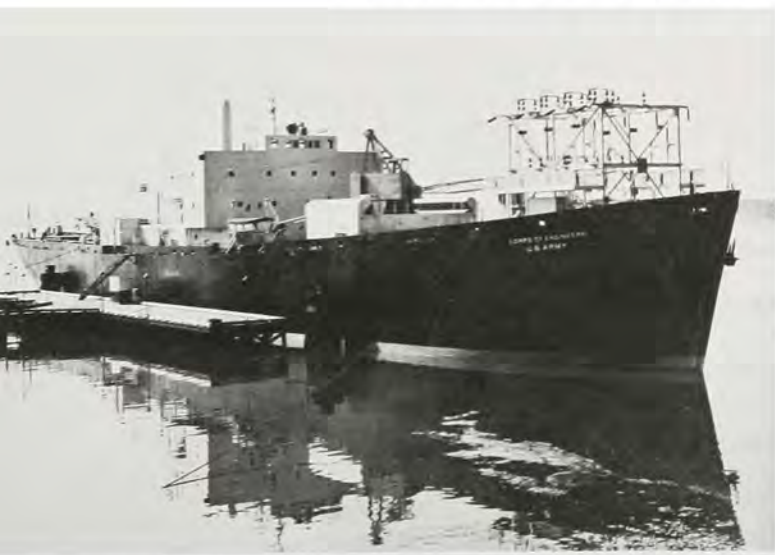
The Sturgis (MH1A), first floating nuclear power plant.
