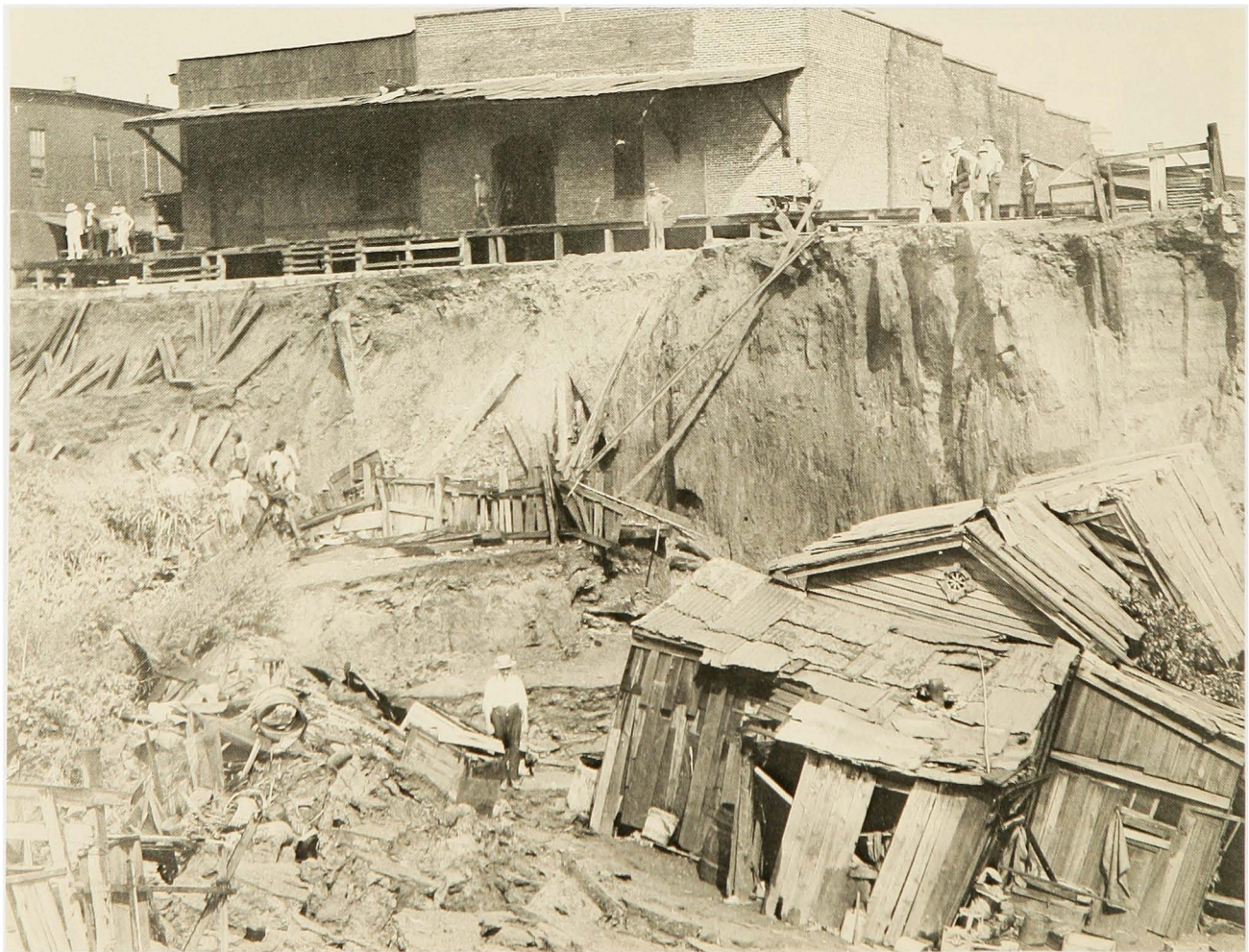
Severe bank caving in Memphis, July 26, 1926.
