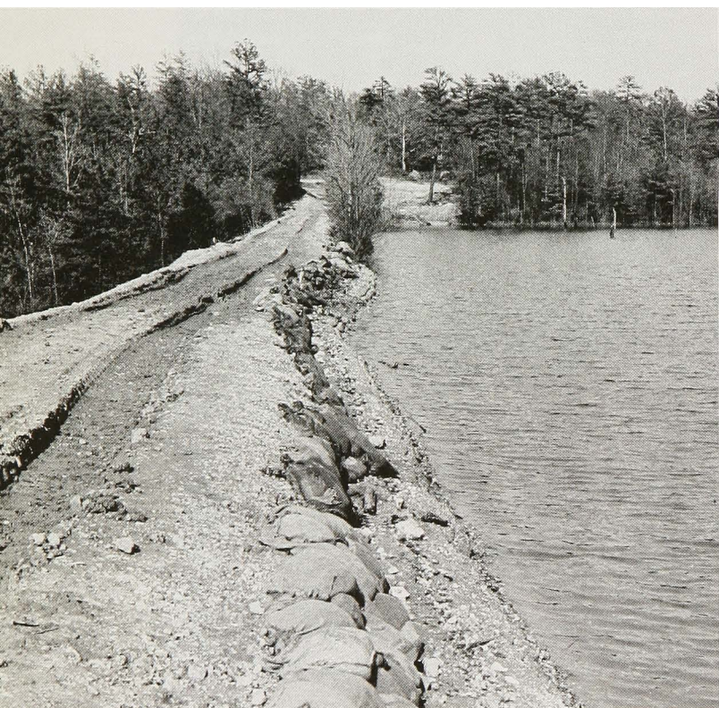
Emergency levee at Fredricktown, Missouri, 1979.
