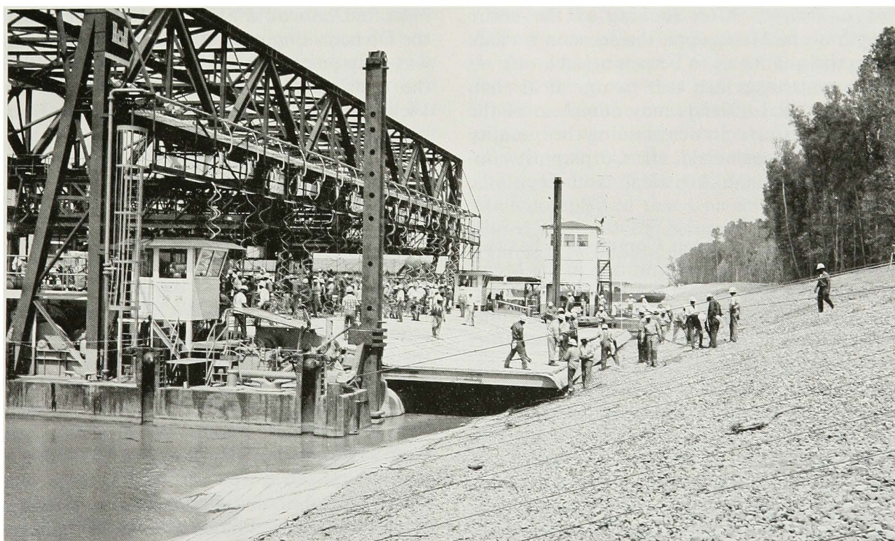
A Corps mat sinking unit at work laying articulated concrete mattresses.
