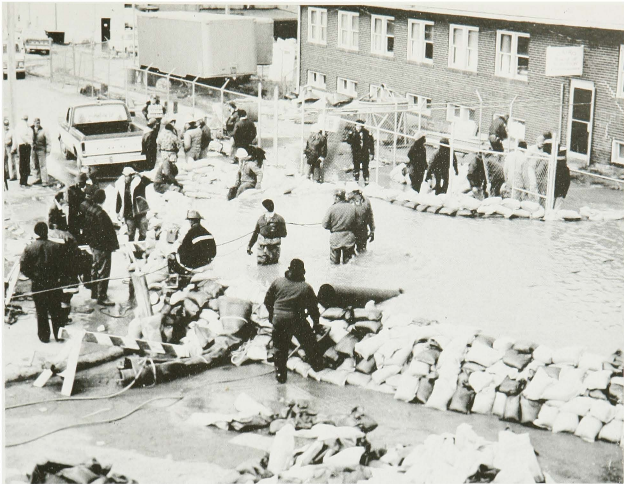
Emergency work at Cairo, Illinois, 1979.
