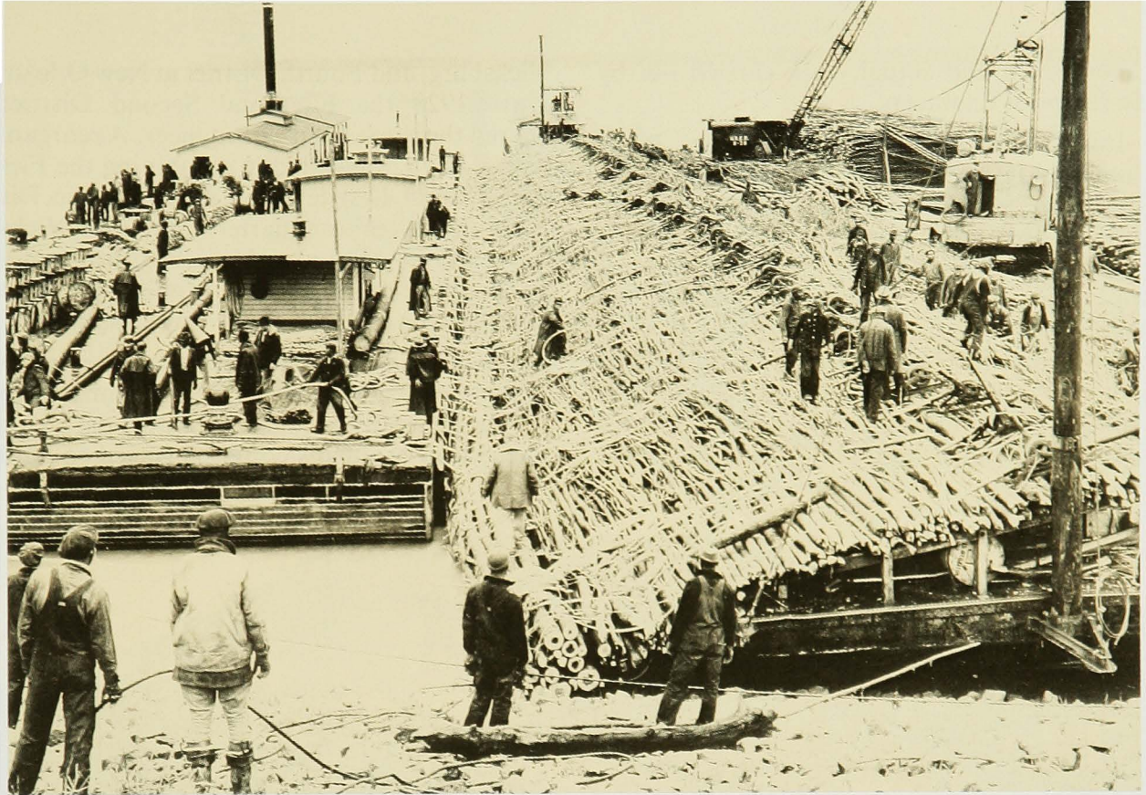
Willow mattress plant and mooring barge being swung into position.
