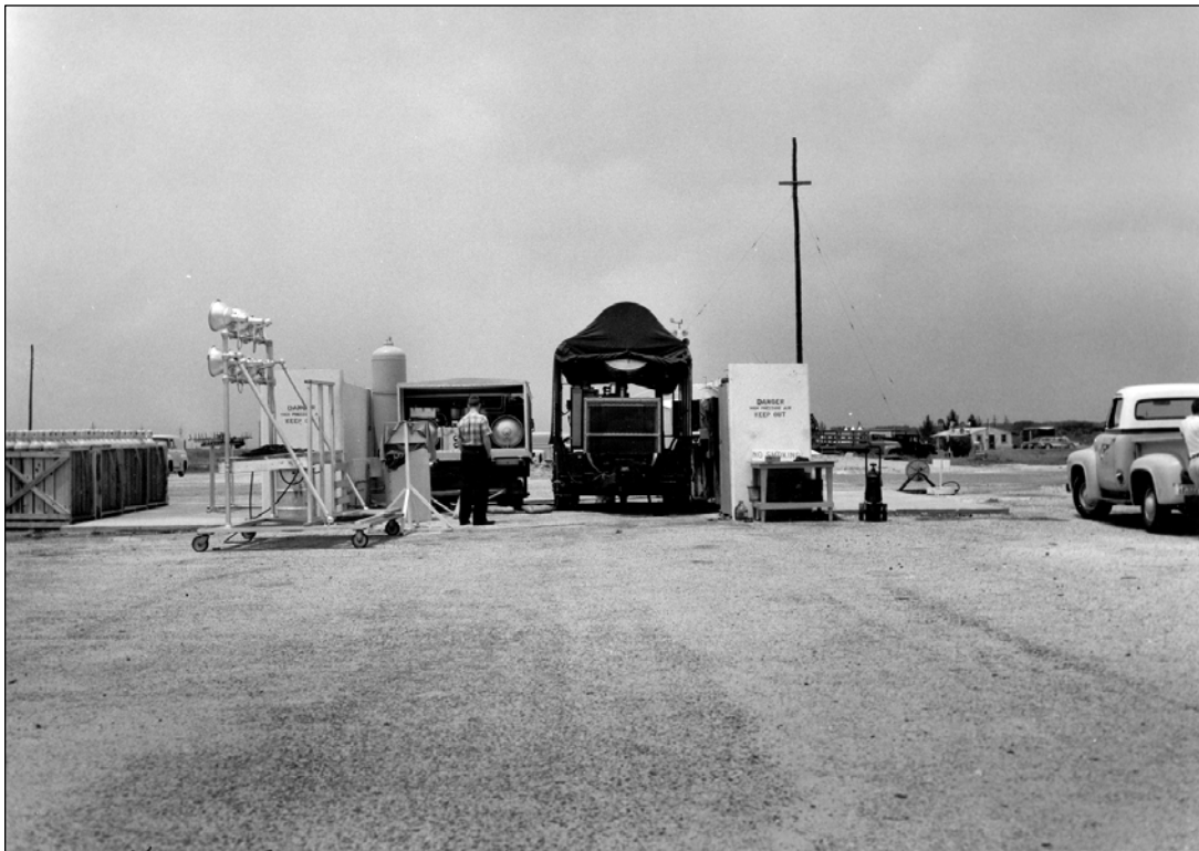
Figure 19. High Pressure Air Facility, date unknown. Photograph located at University of Central Florida, Florida Space Coast History Project.
