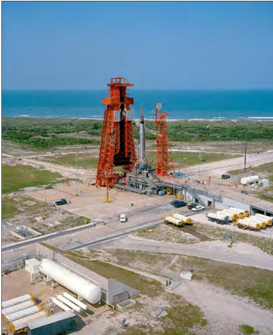
Figure 8. Mercury-Atlas 9 in preparation for launch, May 15, 1963. Note Launch Stand and Ramp, Umbilical Mast behind Ramp, Service Structure to left of Ramp, and LOX and GN2 Storage Area in foreground. Photograph located at San Diego Aerospace Museum.
