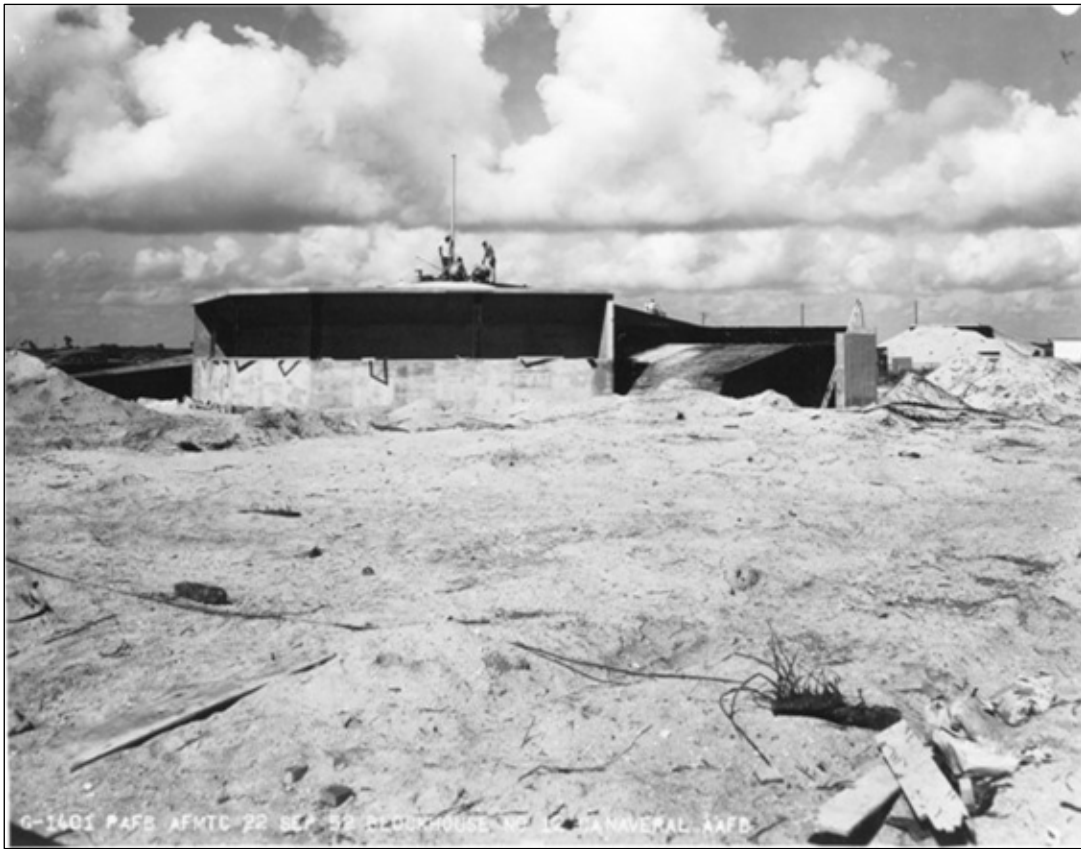
Figure 6. Complex 1/2 Blockhouse during construction, September 22, 1952. Photograph 52-g-1401, 45th Space Wing History Office, Patrick Air Force Base.
