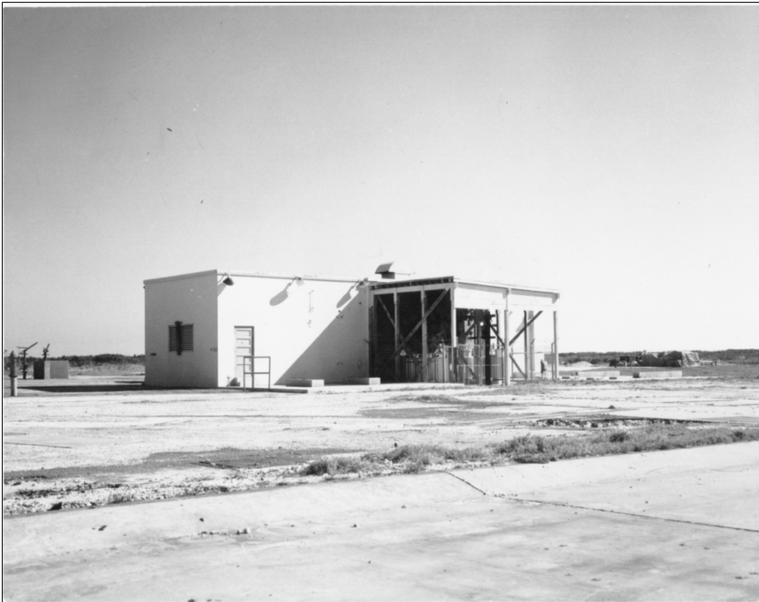
Figure 20. High Pressure Air Building and Electric Substation, date unknown. Photograph located at University of Central Florida, Florida Space Coast History Project.
