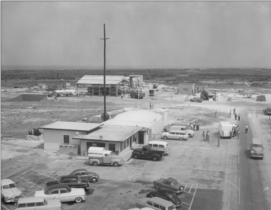
Figure 22. Launch Complex 3/4, ca. 1956. Blockhouse and Ready Room in foreground. Launch Shelter No. 2 over missile at Launch Pad 4 in center background. Bomarc Launching Building under construction behind Pad 4. High Pressure Air Building and High Pressure Air Facility in background on right. Photograph a089703, A series Boeing Photographs, located at University of Central Florida, Florida Space Coast History Project.
