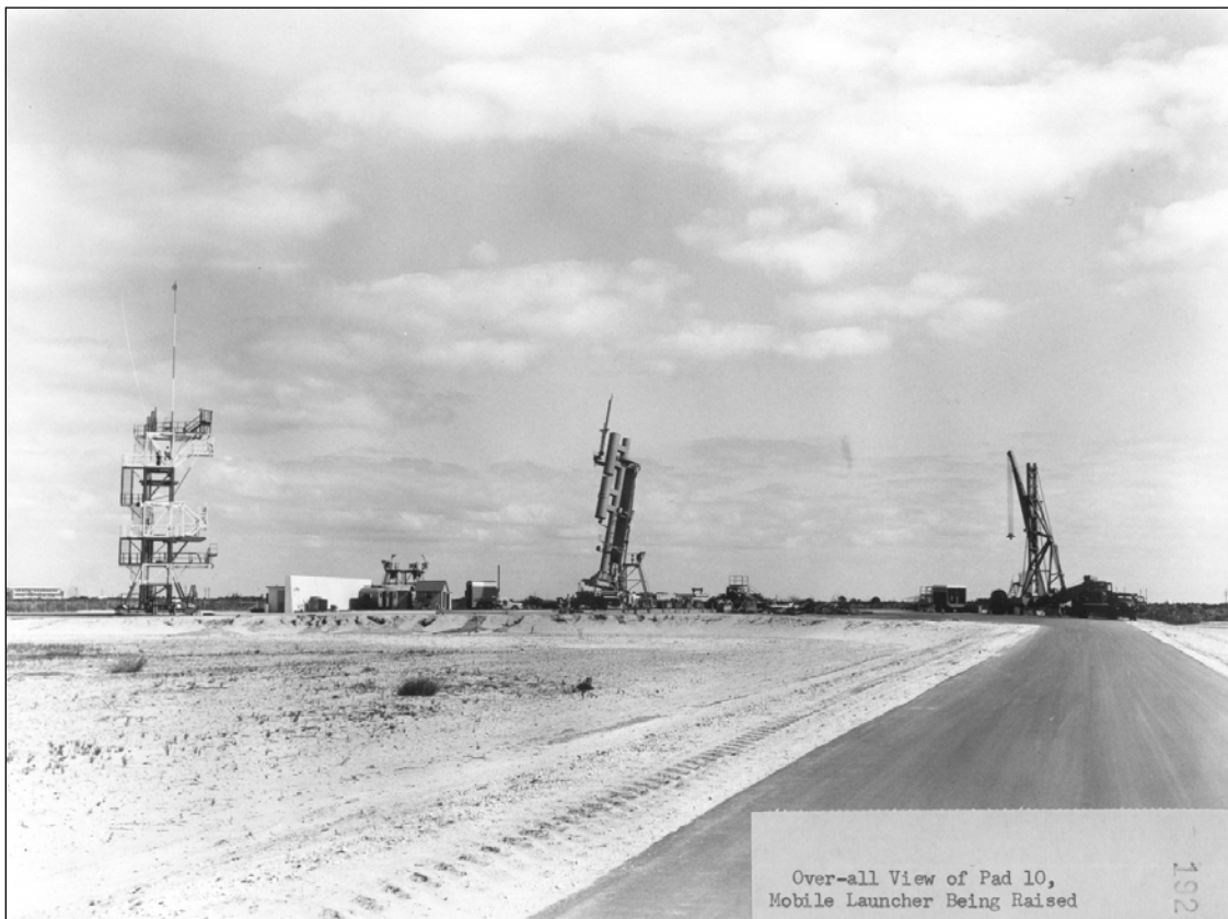
Figure 11. Overall view of Pad 10, date unknown. From left to right: Navaho Service Tower, Blast Wall, and Restroom Building, Mobile Launcher, and Test Navaho. Photograph 16989, RCA, U.S. Air Force. Photograph located at 45 th Space Wing History Office, Patrick Air Force Base.
