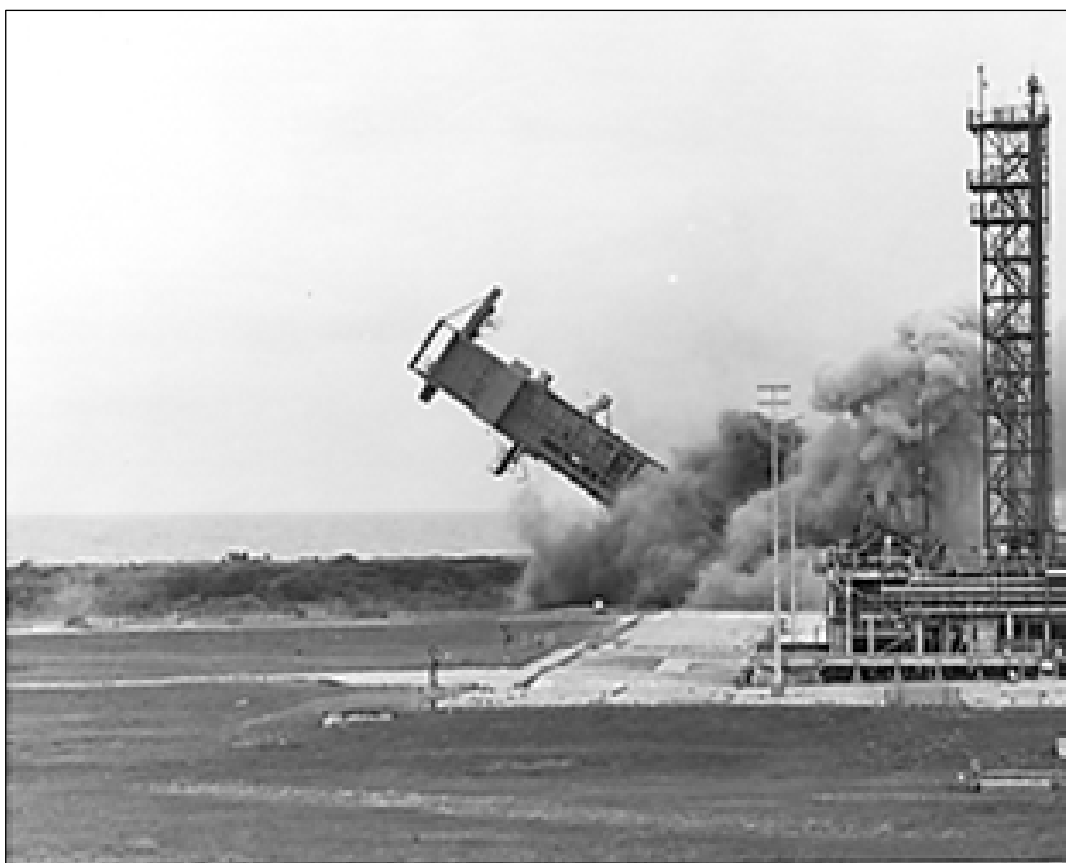
Figure 5. Demolition of Service Structure, December 1, 1976. Photograph 76-PL-76-37401.4, U.S. Air Force, located at University of Central Florida, Florida Space Coast History Project.
