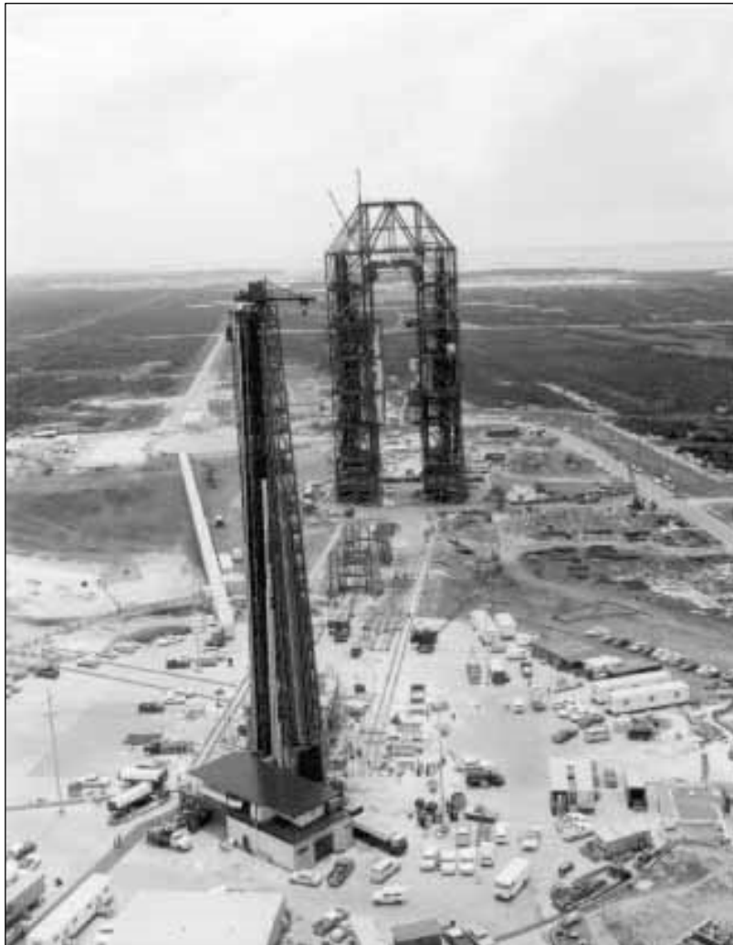
Figure 16. Launch Pad, Umbilical Tower, Environmental Control System Building, and Mobile Service Structure 1965. Figure 239, NASA History Office, http://history.nasa.gov/MHR-5/Images/fig239.jpg .
