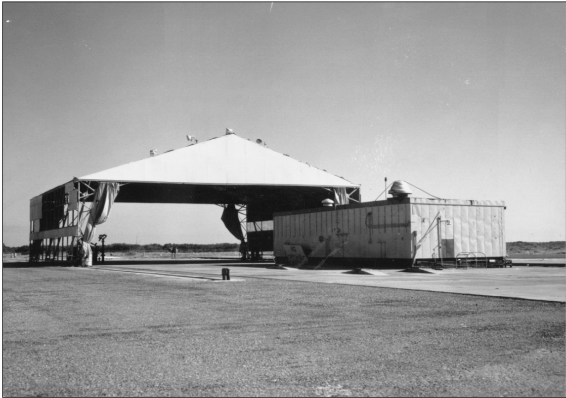
Figure 21. Launch Shelter No. 2 (left) and Launch Support Building at Launch Pad 4, date unknown. Photograph located at University of Central Florida, Florida Space Coast History Project.
