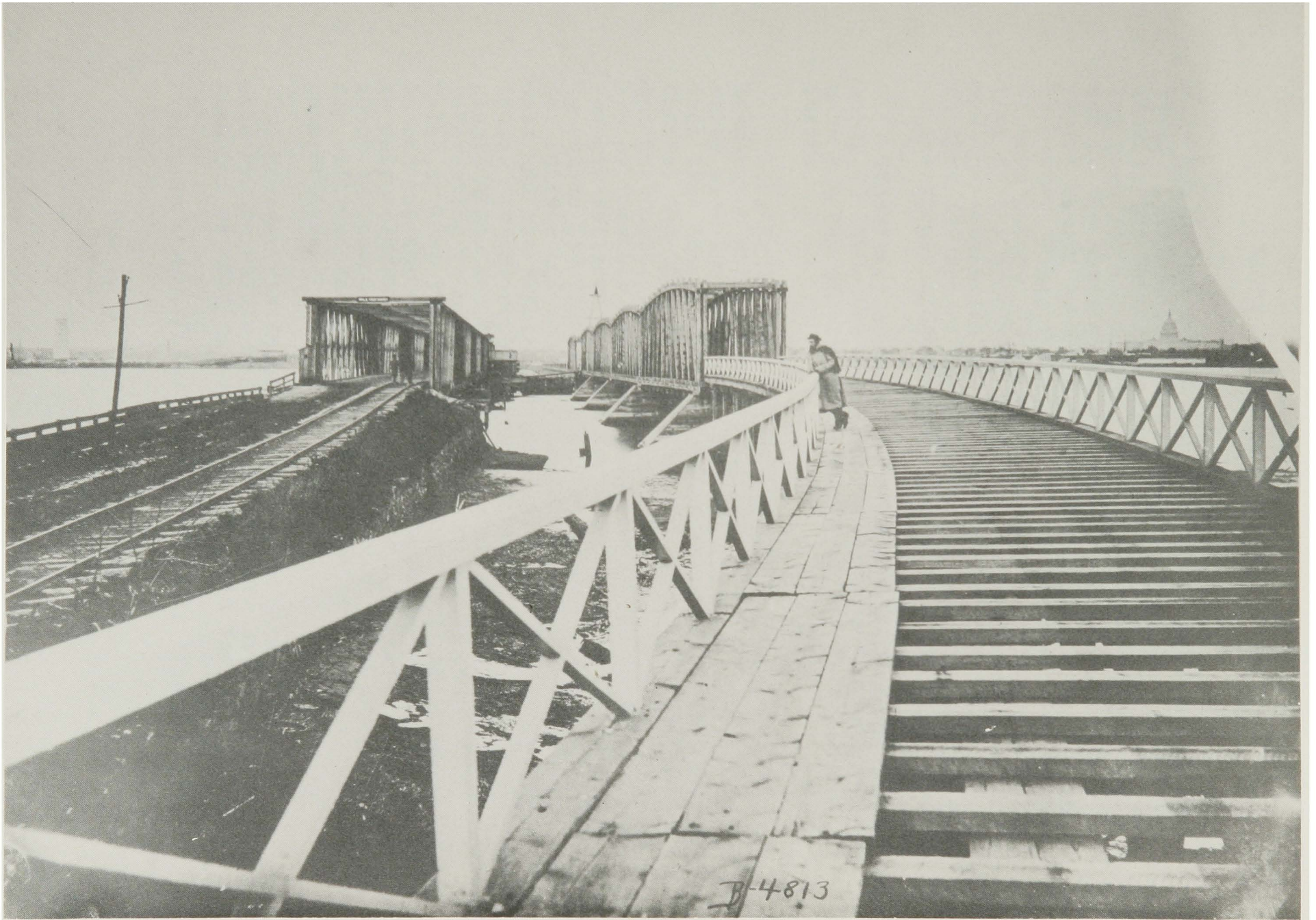
Old Long Bridge
