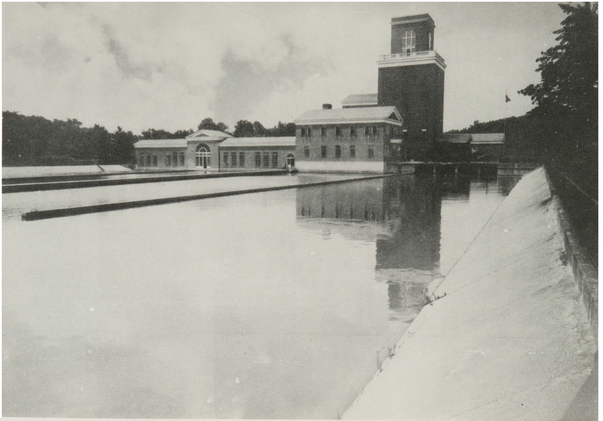
Dalecarlia Filtration Plant
