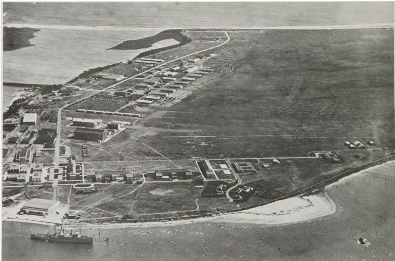
Fill on North Island, San Diego Bay, by Navy Department with authorization by permit from LAD, August 29, 1921.
