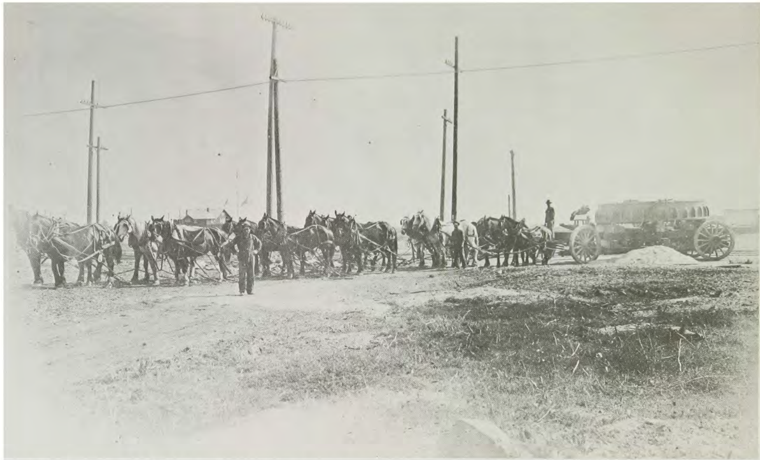
Hauling a base ring for 12-inch mortar with teams of horses by Pioneer Truck Company, Ft. MacArthur, California, September 23, 1916.
