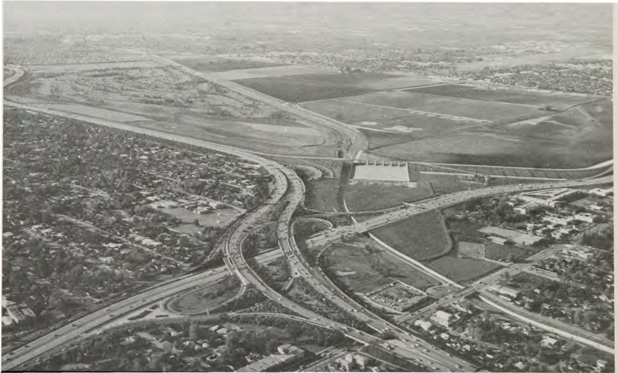
Sepulveda Dam affords protection against floods for considerable residential, urban, and commercial development in the communities of Van Nuys, North Hollywood, Sherman Oaks, and Studio City. (Photo taken c. 1965.)
