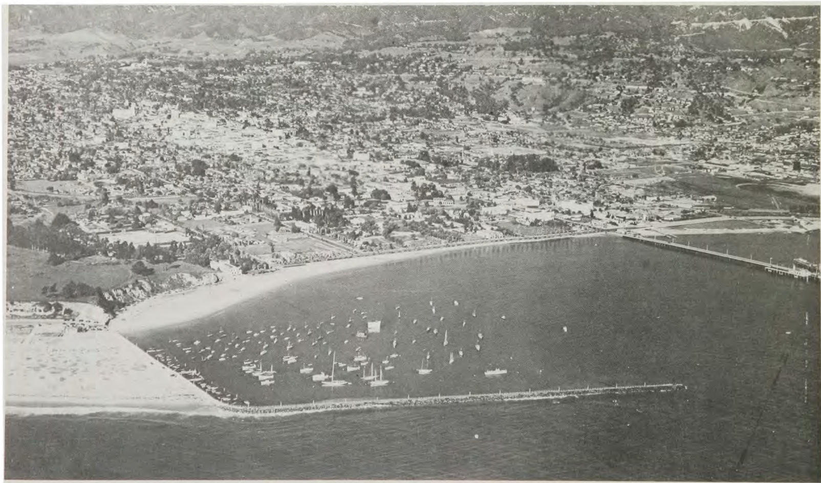
Santa Barbara Harbor dredging by engineers to maintain depths, Dec. 23, 1934.
