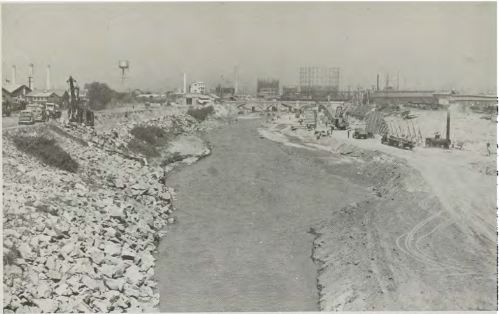
Upstream view of Los Angeles River channel above Soto St. bridge at start of construction.
