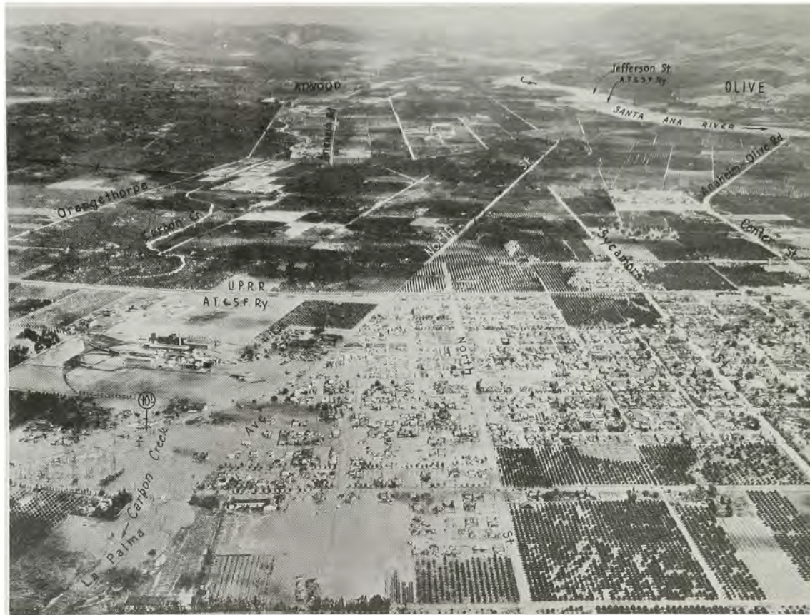
Aerial view of Anaheim, Calif., showing vast area of inundation from overflow of Santa Ana River during flood of March 1938.
