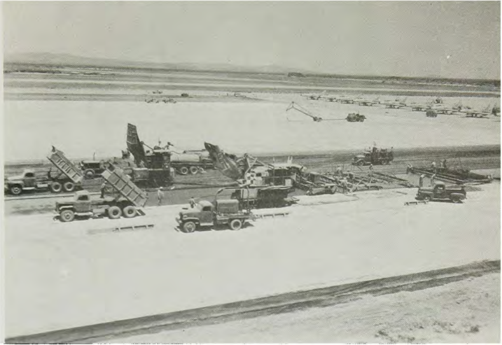
Pouring concrete for taxiway, Edwards Air Force Base, California, August 1955.
