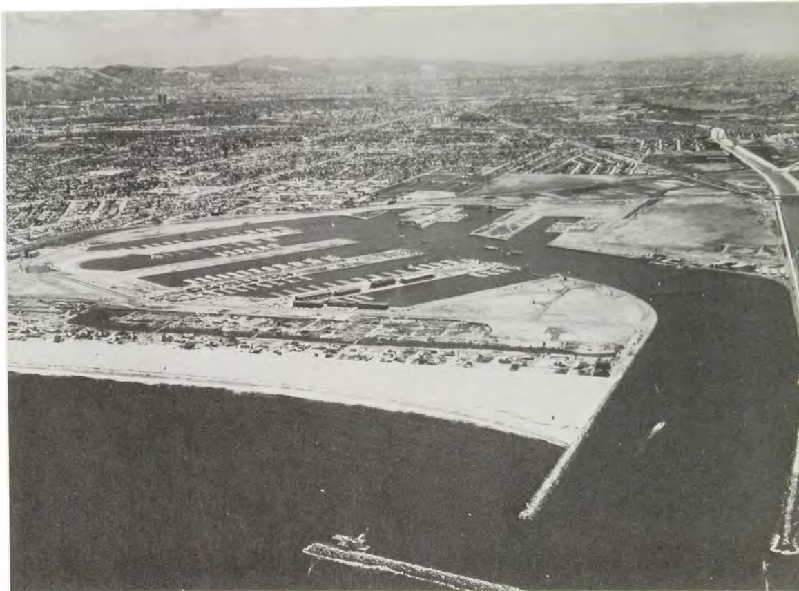
Marina del Rey Harbor. Dredging and construction of entrance channel, jetties and offshore breakwater by Los Angeles District. Project completed in 1962.
