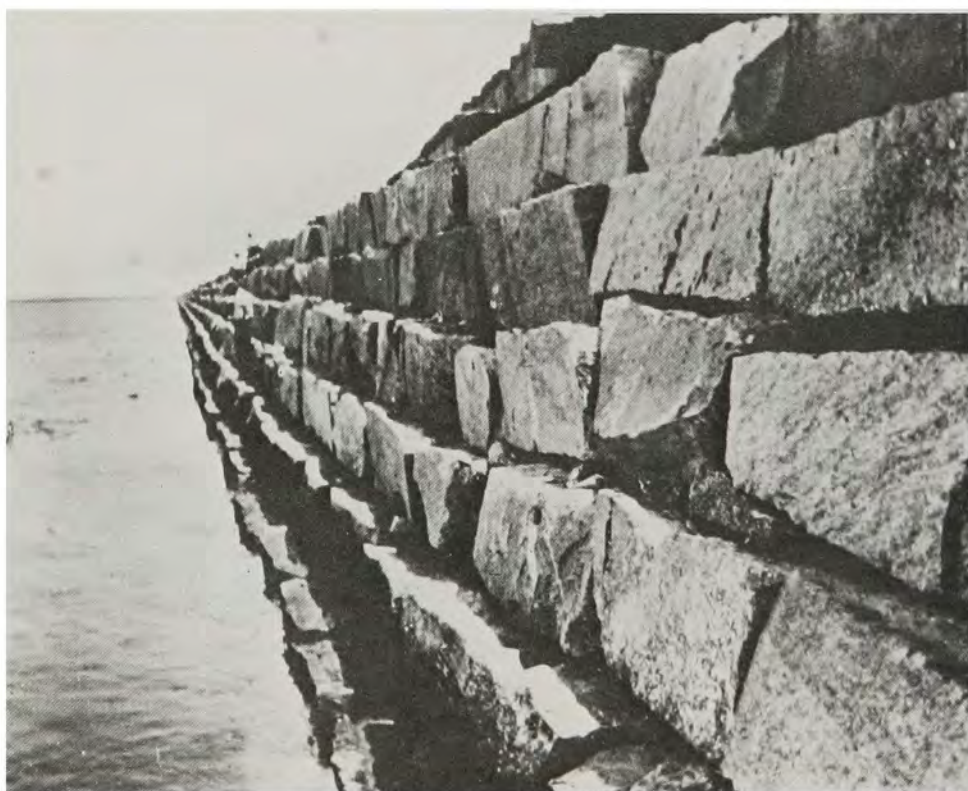
San Pedro Harbor, completed breakwater. (Title Insurance)
