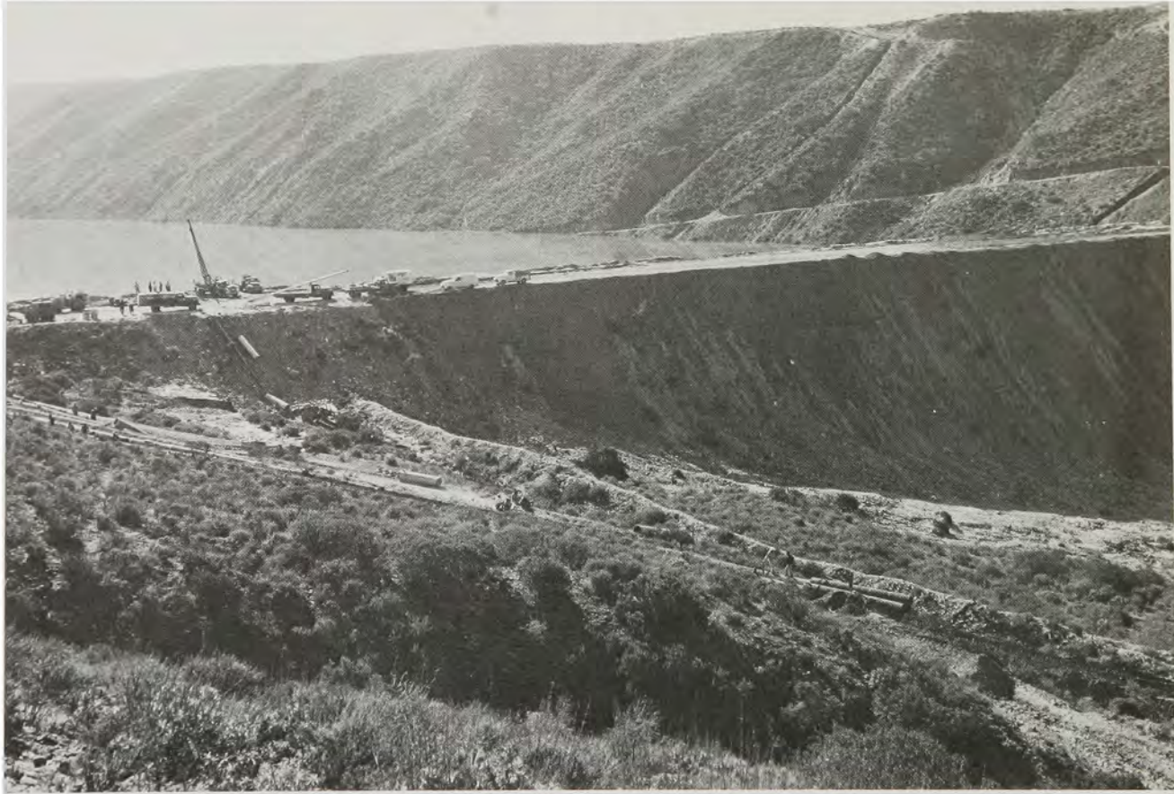
Construction on Tijuana Dam, Mexico, for the International Boundary and Water Commission (1968).
