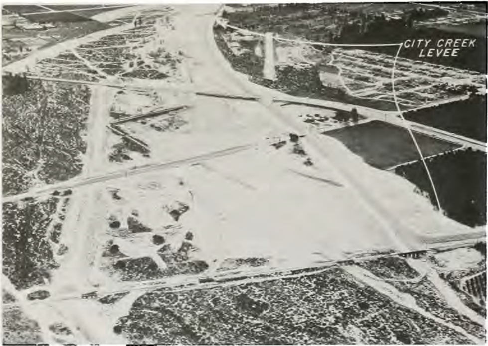
City Creek levee, a small flood control project in San Bernardino County, Calif., is at the right. The levee-like structure at the left is a spoil-bank area used for the disposal of excess channel-excavation material.
