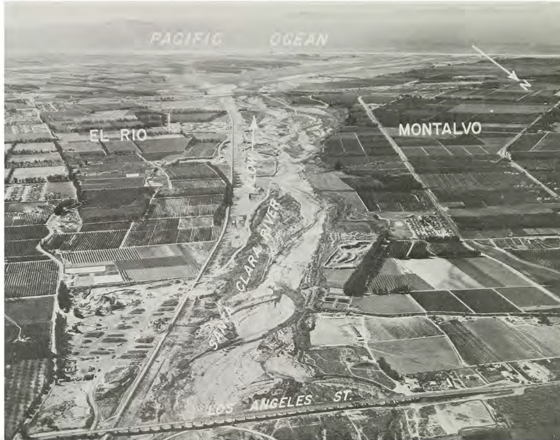
Santa Clara River levee. View of nearly completed levee looking downstream from the upper end of the project (1960).
