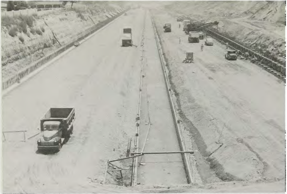
Los Angeles River channel improvement, Tujunga Wash channel. View shows graded channel with wall footings on the left and low water channel complete. The forms and steel for the right wall footing are in place and concrete is being poured. To the left filter material is being dumped and spread preparing the invert sub-grade.
