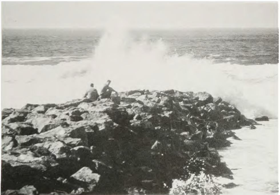
Waves breaking on groin, Imperial Beach (1961).
