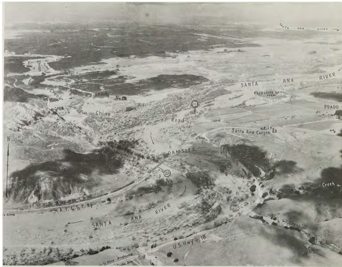
Prado dam site after 1938 flood.
