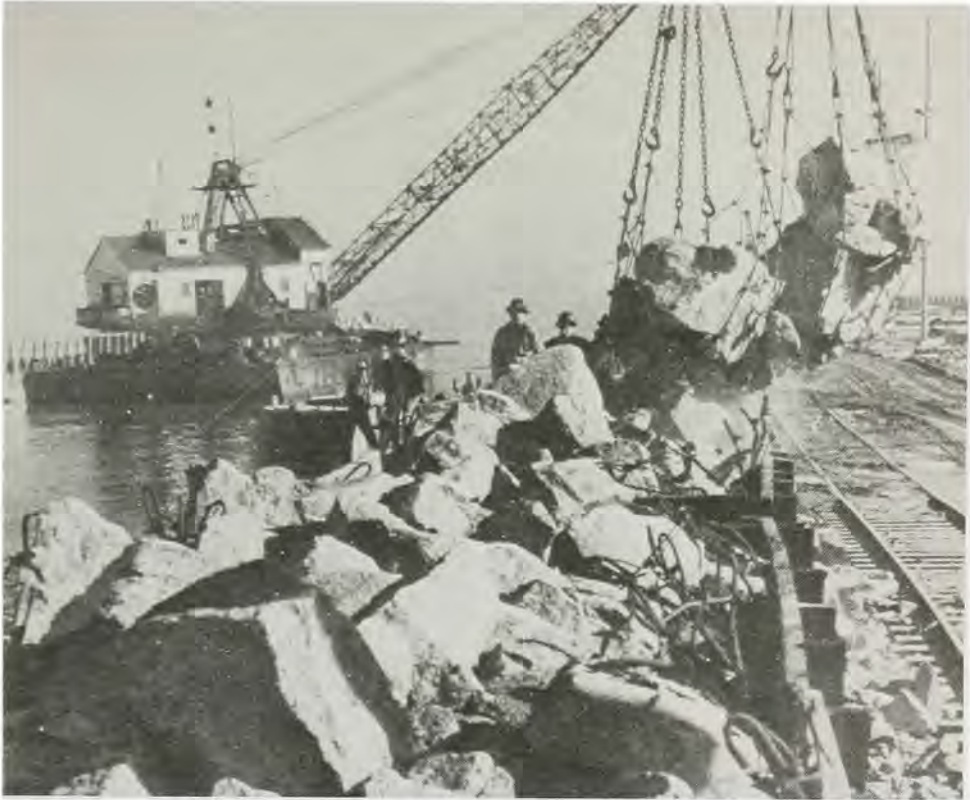
Long Beach Harbor, constructing Pier A to serve as an ammunition dock, 1943.
