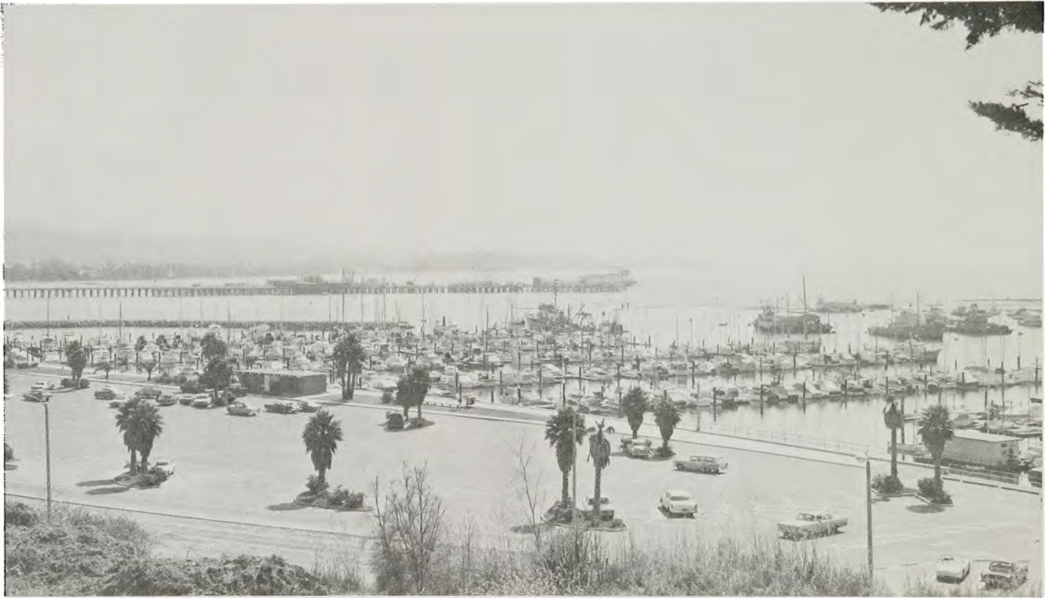
Crowded conditions and constant buildup of sand in the Santa Barbara Harbor requiring constant dredging (shown in the middle background) led to planning a project to eliminate those conditions.
