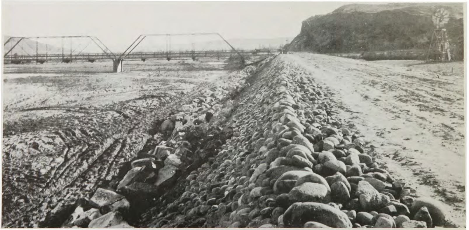
San Diego River Dike, Jan. 20, 1897. Repair work of raising crest and revetting face with riprap nearly completed.
