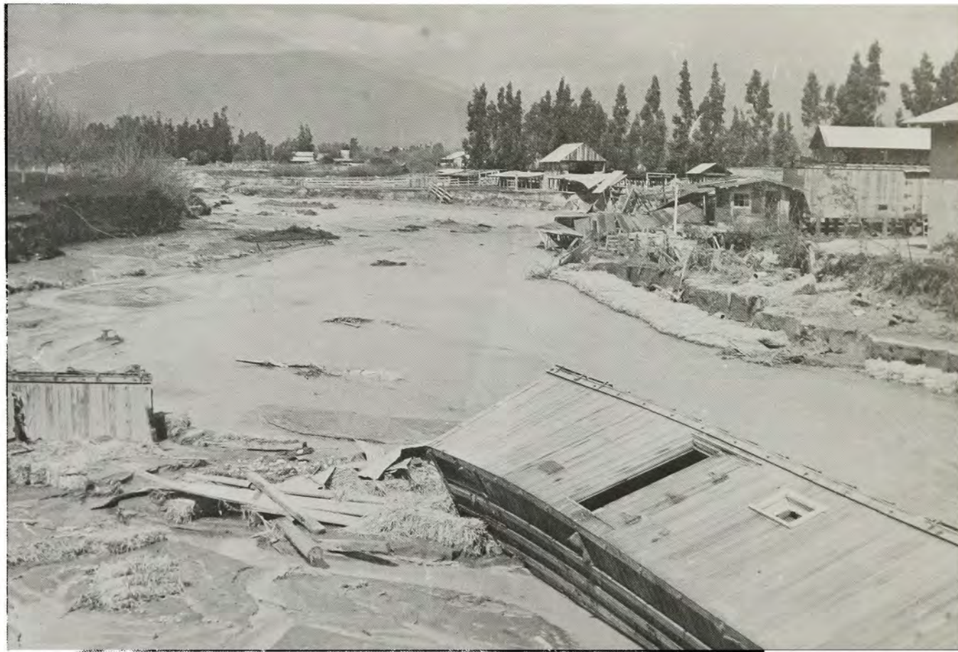
Damage from the March 1938 flood on San Antonio Creek.
