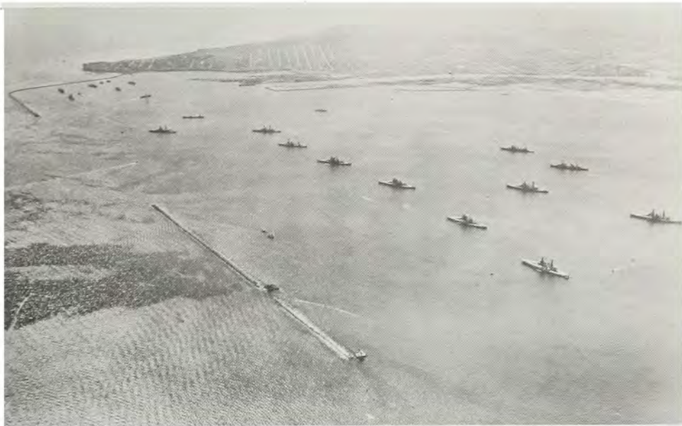
This is a view from offshore looking up the coast toward San Pedro which shows the partially completed detached section of the breakwater in the foreground with work in progress at two points.
