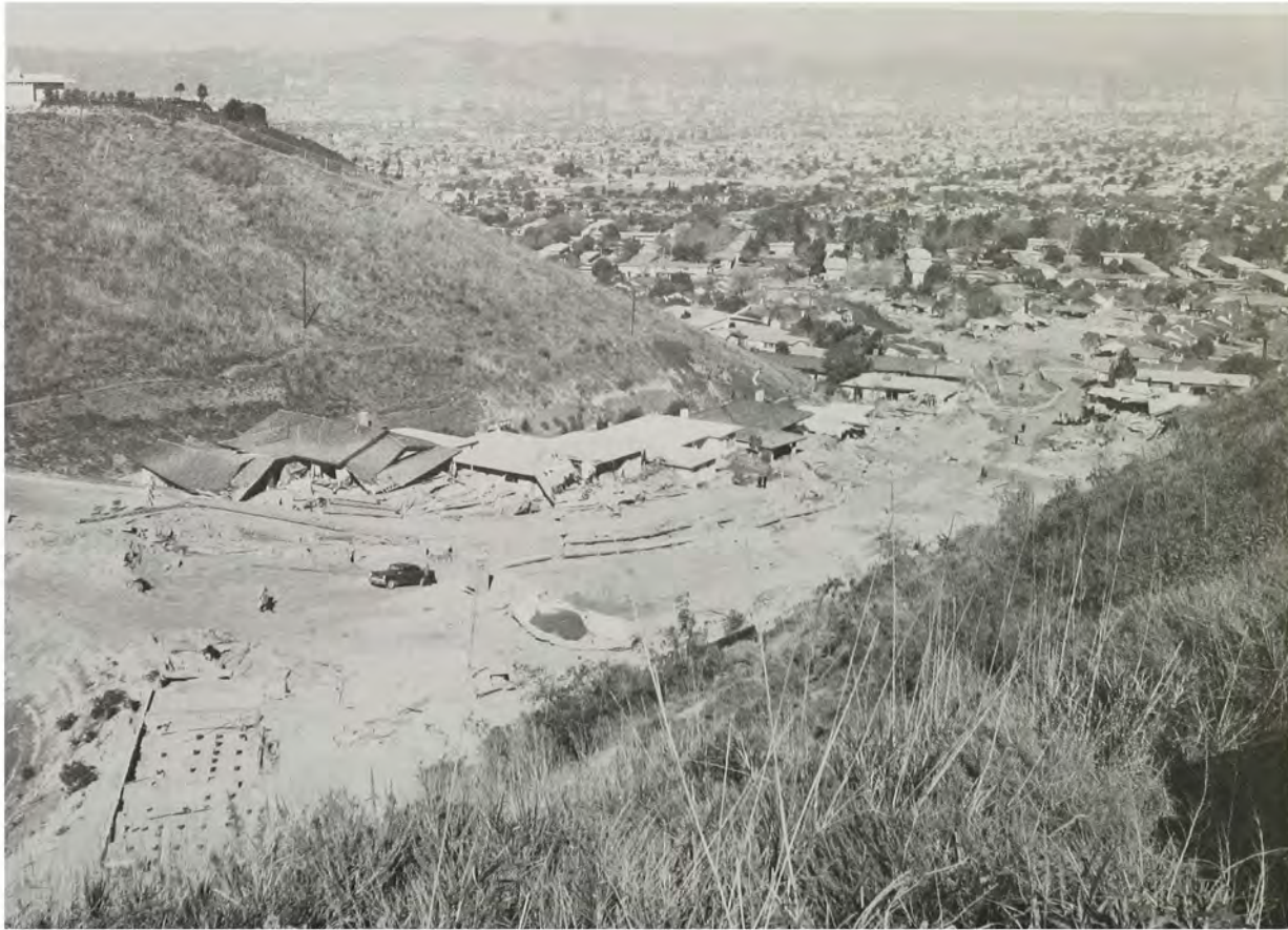
Same view as previous photograph. Sidewalks, curbs, and gutters restored subsequent to Corps of Engineers work.
