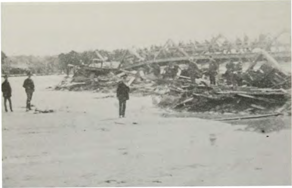
First St. bridge over Los Angeles River after the flood of 1884.
