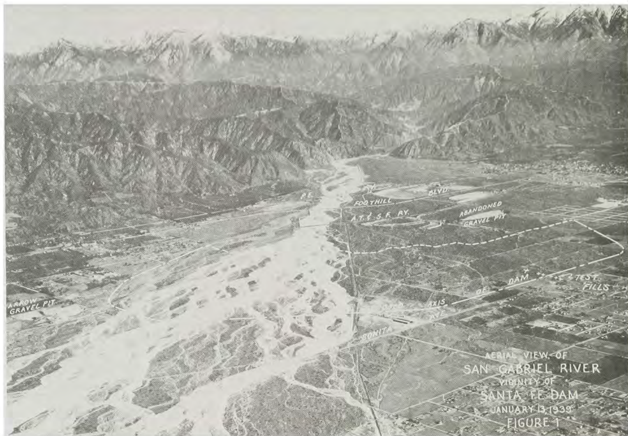
Upstream view of San Gabriel River shows the site of Santa Fe flood control basin prior to construction, January 13, 1939.
