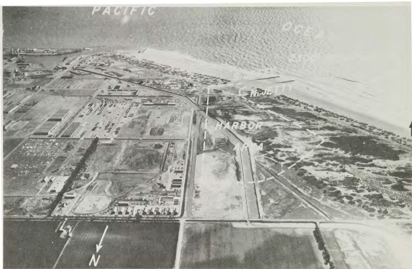
Site for Channel Islands Harbor prior to start of construction. In the upper left background is Port Hueneme whose shoaling problem led to a solution which included a new harbor.
