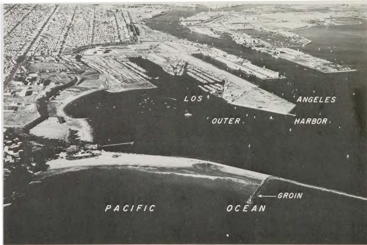
Stone groin at harbor breakwater to combat erosion at Cabrillo Beach, Los Angeles Harbor (1962).
