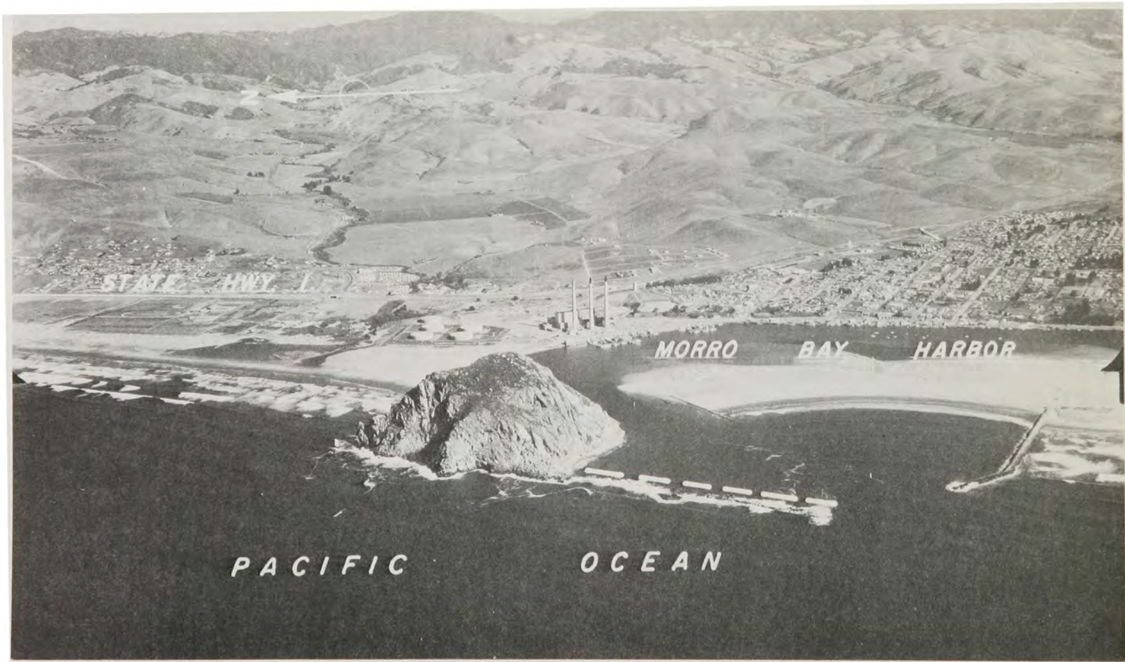
Rehabilitation of north breakwater in progress in 1962.
