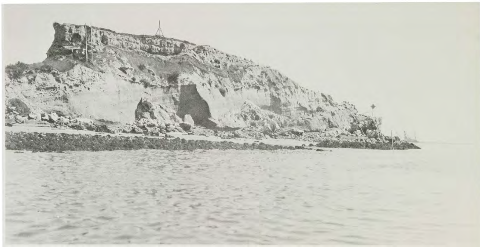
Los Angeles Harbor, Main Entrance. Widening channel to 1,000 feet and 35-foot depth; Deadman's Island; removal of reclamation of Reservation Point, March 30, 1927.
