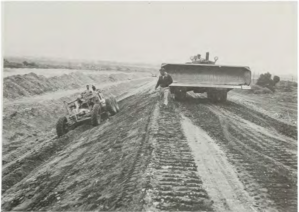
Placing and compacting embankment fill on Sepulveda Dam.
