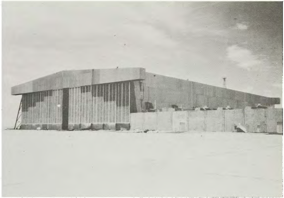
Completed hangar, Edwards Air Force Base, California, August 1955.
