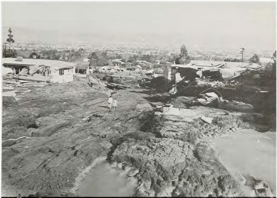
Downstream view of Cloverdale Avenue, showing typical damage to residential property after dam break.
