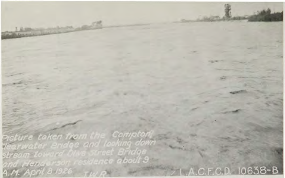
Flood of April 8, 1926. Downstream view of the Los Angeles River at Mile 1.9. (LACFCD photo)
