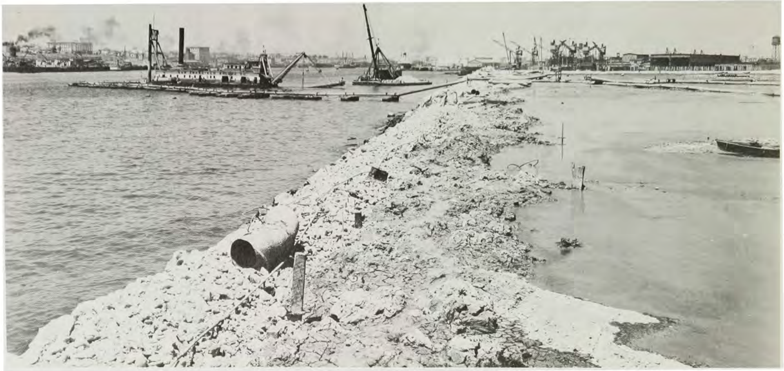
Same project. The view is northwesterly. In the right foreground is the west bulkhead and fill, and in the left foreground is a new water area, site of former Deadman's Island. In the left middleground is the new channel area with dredge McMullen and pipeline to fill, clamshell dredge, and barges for obtaining project depth and clean-up, May 5, 1929.
