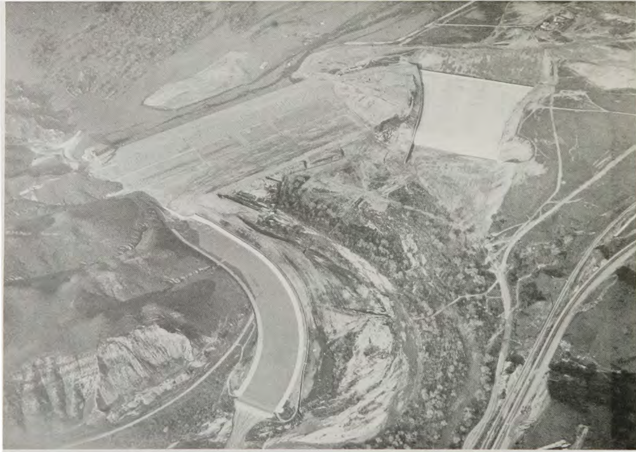
Prado Dam at Santa Ana River mile 31.5, the major flood control work (1941).
