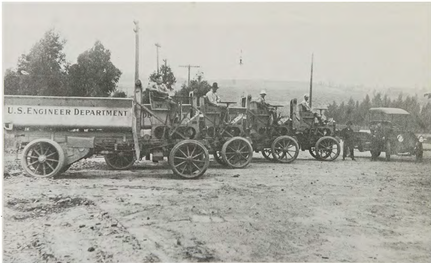
Trucks used by Los Angeles District to supplement horsedrawn equipment, Ft. MacArthur, California, 1916.
