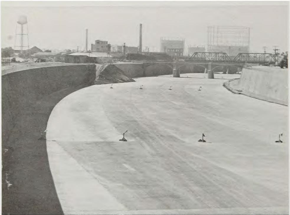
Upstream view of completed Los Angeles River channel above Soto St. Bridge.
