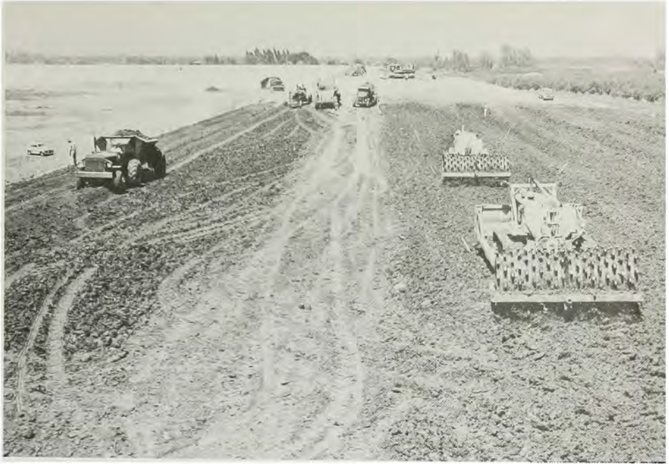
Slope grading, Lytle Creek.
