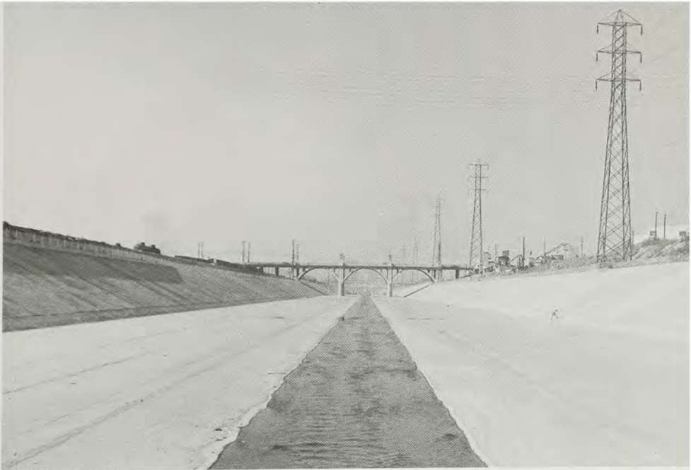
Completed Los Angeles River channel upstream from Butte St. bridge.
