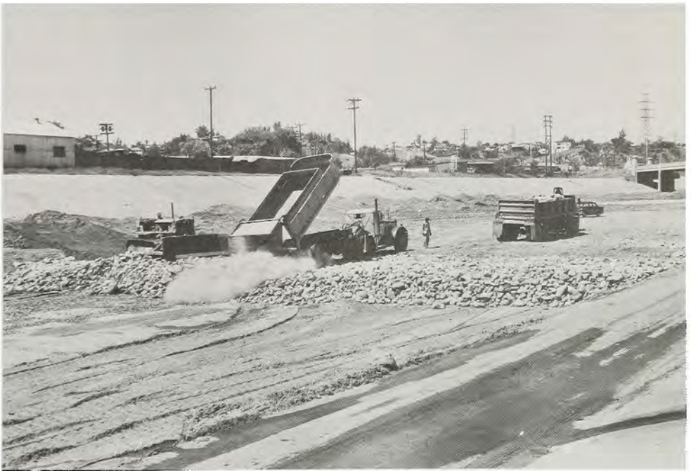
Placing cobblestone between toes of levees.
