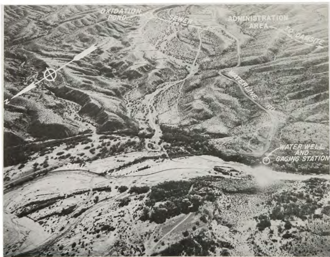
Alamo Reservoir, Bill Williams River, Arizona. View showing administration area under construction (1963).
