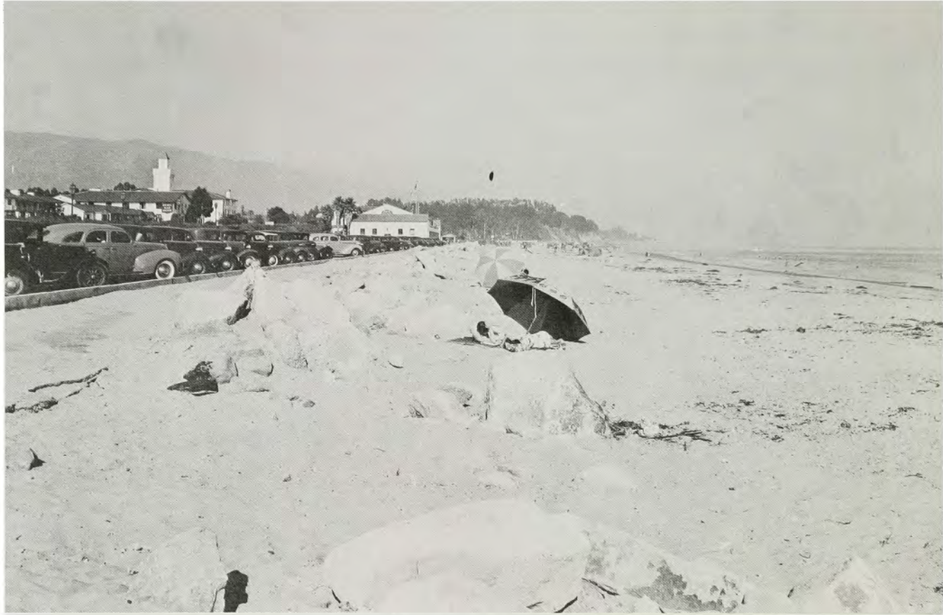
Dredged sand covers the revetment and makes the beach usable again (1938).
