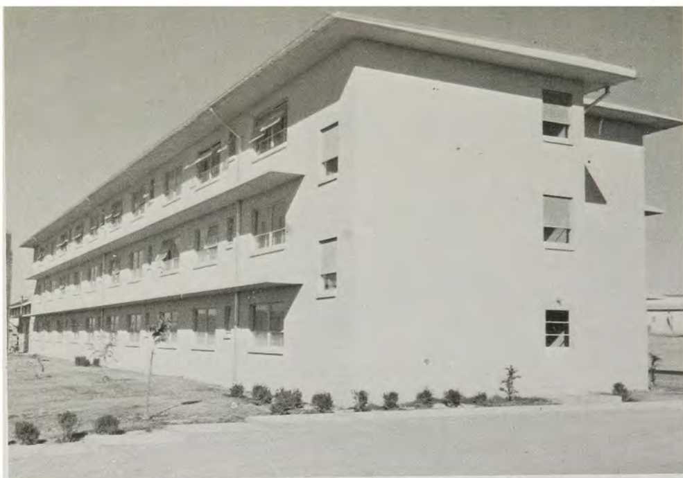
Bachelor Officers' Quarters, Yuma Test Proving Grounds, Arizona.
