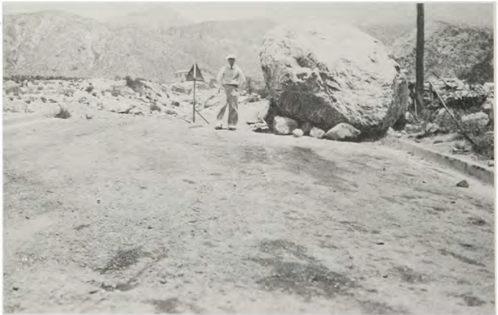
Granite boulder, about 9 feet in diameter, washed onto the pavement at the end of New York Ave. Dunsmuir Canyon flood of January 1, 1934.
