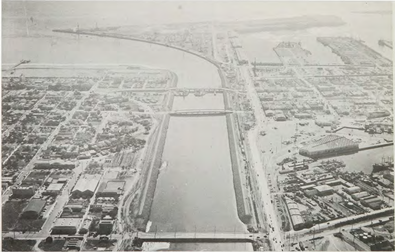
Lower Los Angeles River channel, 7th St. to Pacific Ocean. Levees in this section were rebuilt and raised. Completed 1953.
