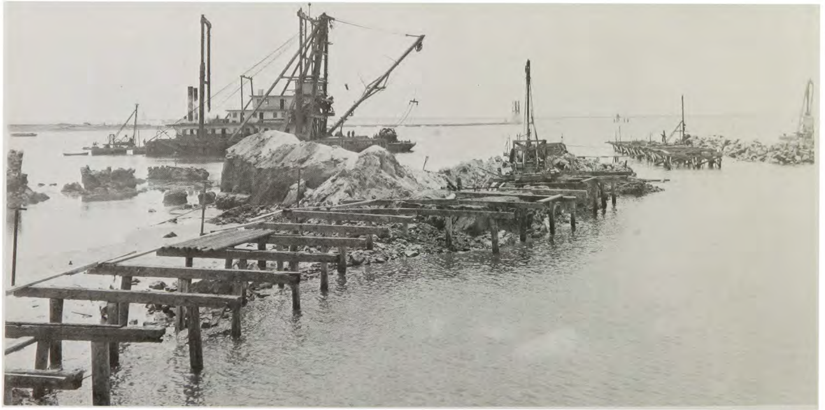
Los Angeles Harbor. In the foreground are the remainder of Deadman's Island, the dredge, San Francisco No. 2 , and trestles supporting boring rigs for blasting holes and jetty; in the distance the southeasterly corner of fill pipe line, the suction dredge, and the government breakwater, June 9, 1928.
