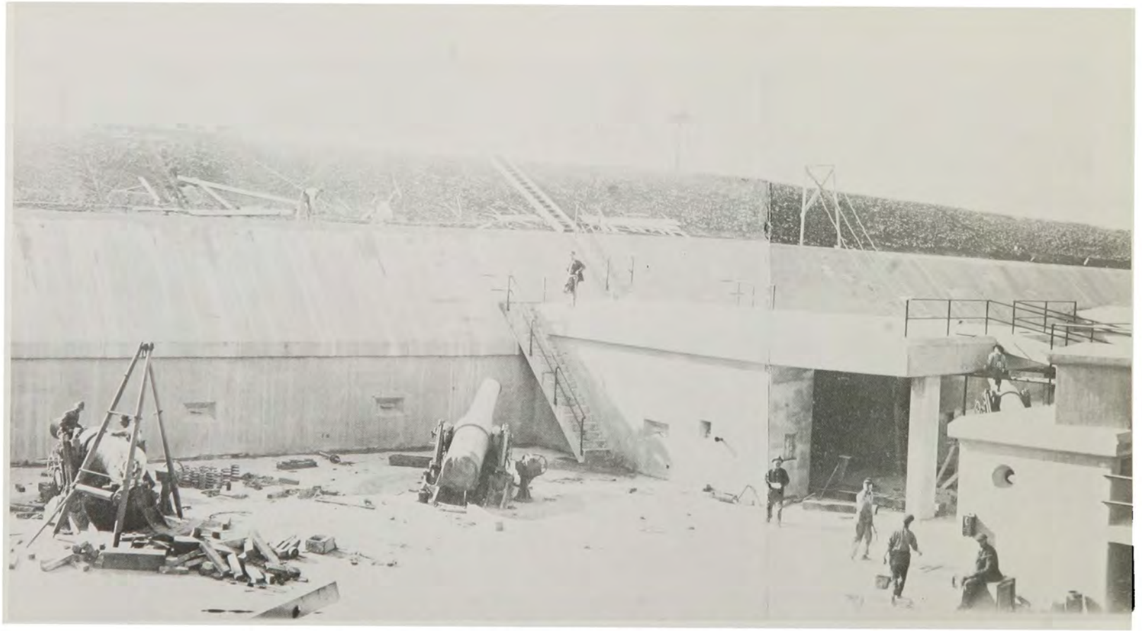
Construction in progress for mortar battery, Ft. MacArthur, California, December 16, 1916.
