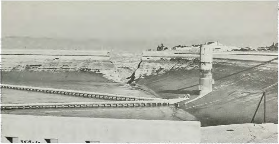
Baldwin Hills Dam and Reservoir, looking downstream. Note break in dam and in asphalt lining along length of reservoir.
