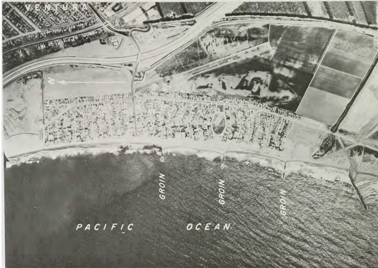
Completed construction of three groins, Phase One, Shore Protection, Ventura-Pierpont Area.
