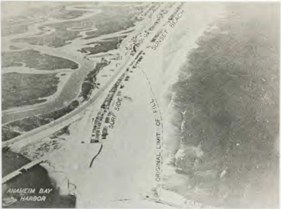
View of temporary fill at Surfside, March 18, 1948, about three months after completion of dredging.
