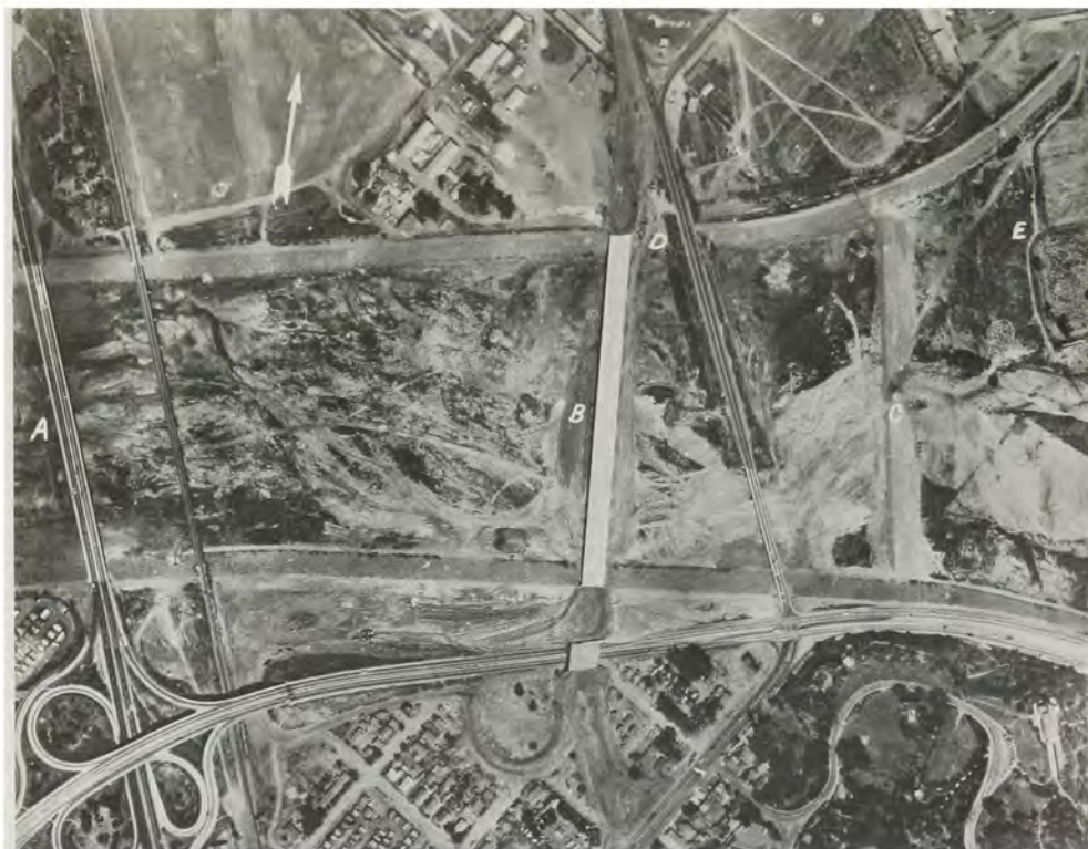
Aerial view of flood control portions of the project displays the completed new U.S. Highway 101 Bridge at "A", the new Moreno St. Bridge at "B", and stabilizer at "C", with still uncompleted portion of levee at "D", and upper limits of the project at "E", December 31, 1951.
