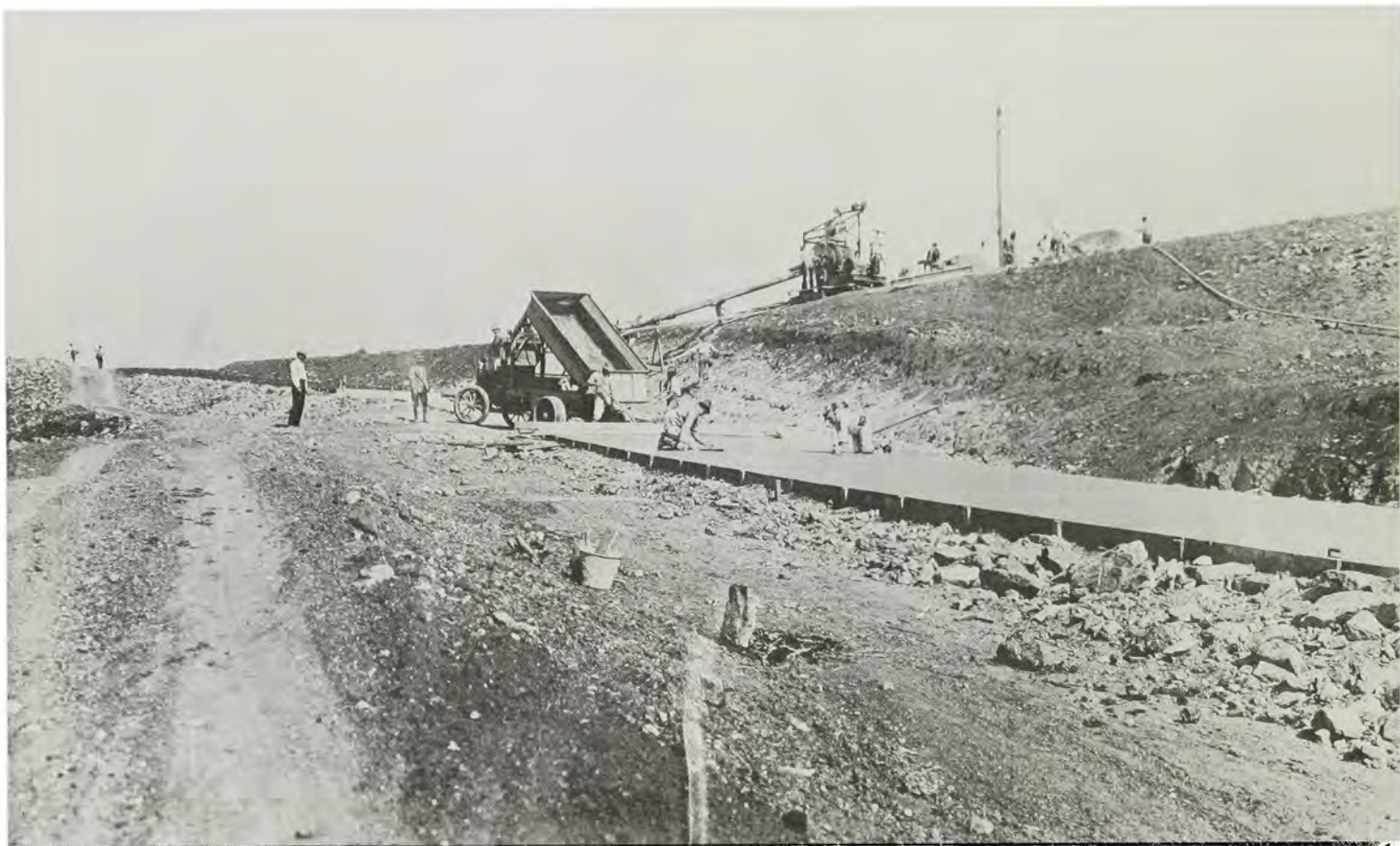
Pouring concrete, mixer and 6-ton Locomobile truck in use, Ft. MacArthur, California, October 28, 1916.
