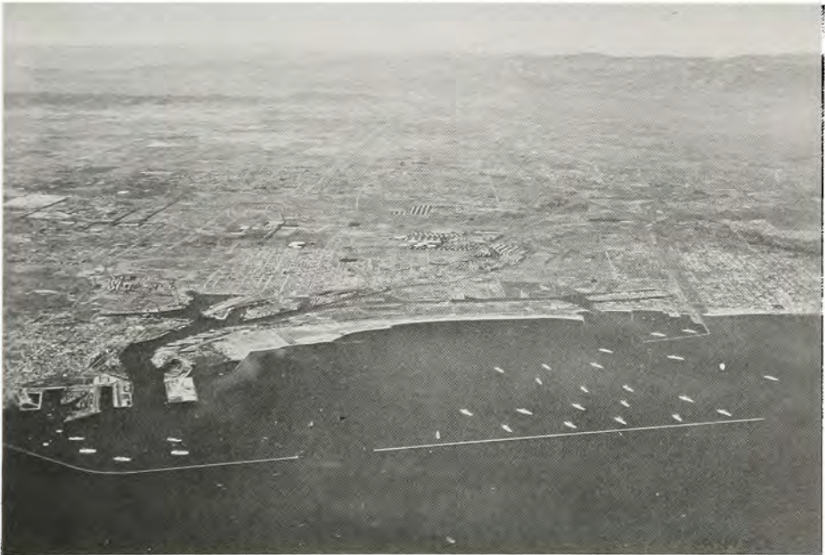
A view of the Los Angeles-Long Beach Harbors and the completed breakwater. At anchor in the area protected by the improvement lies part of the United States fleet (1938).
