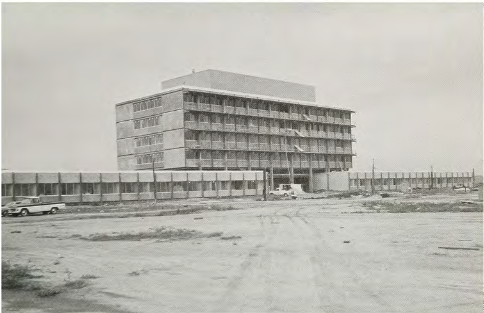
Two-hundred bed hospital, March Air Force Base, California (1964).
