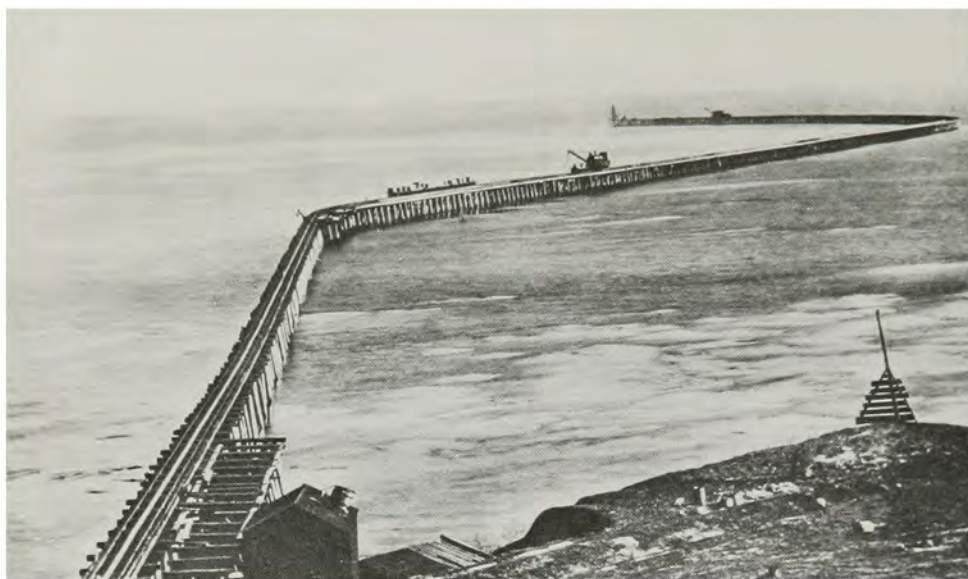
San Pedro breakwater under construction, 1902. (Title Insurance)
