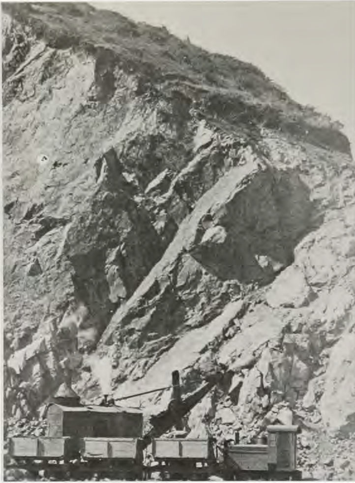
This is a view of operations and the face in the quarry near Avalon on Catalina Island, the source of stone for the breakwater, October 26, 1932.
