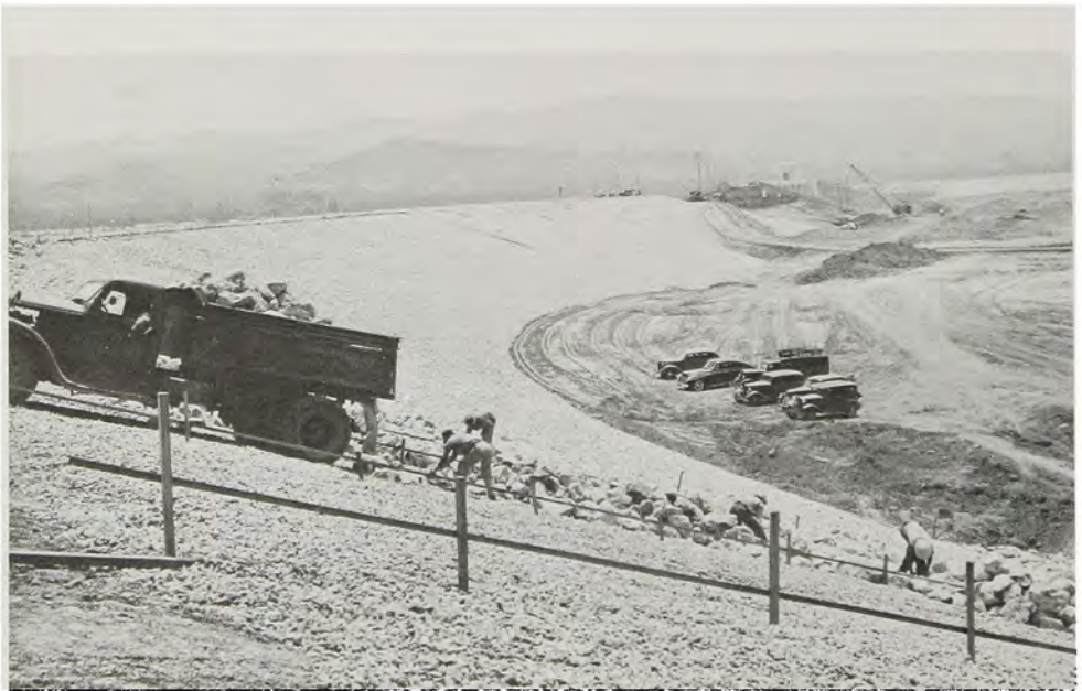
Placing stone blanket on upstream slope of Sepulveda Dam.
