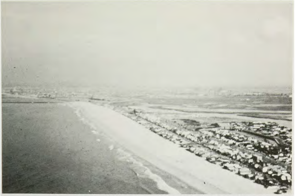
Completed fill project for Surfside-Sunset Beaches (1965).
