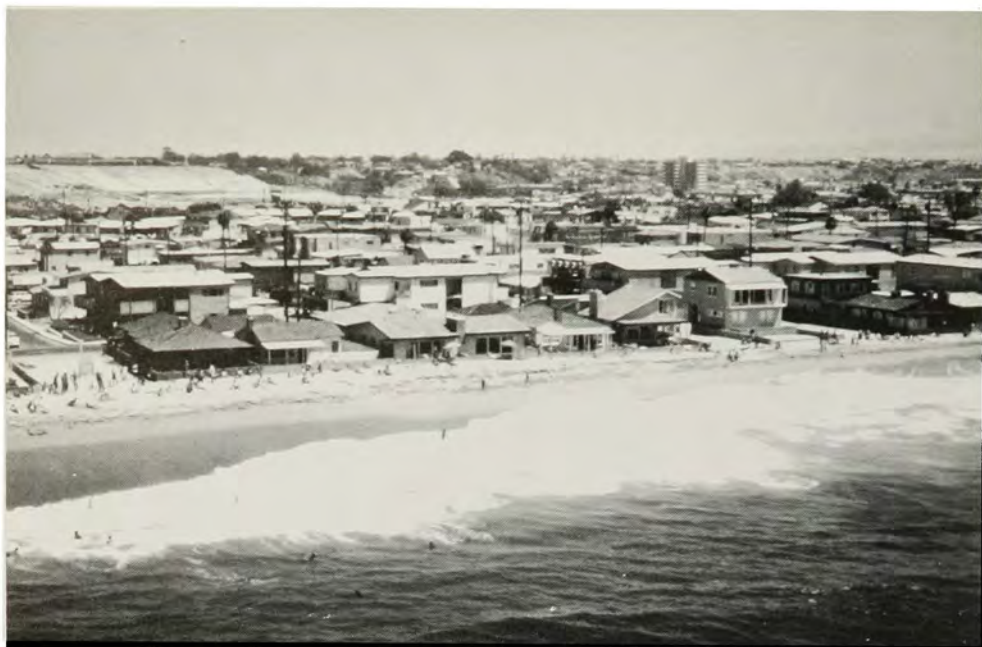
Eroded area between 48th and 38th Sts., Newport Beach, 1965.
