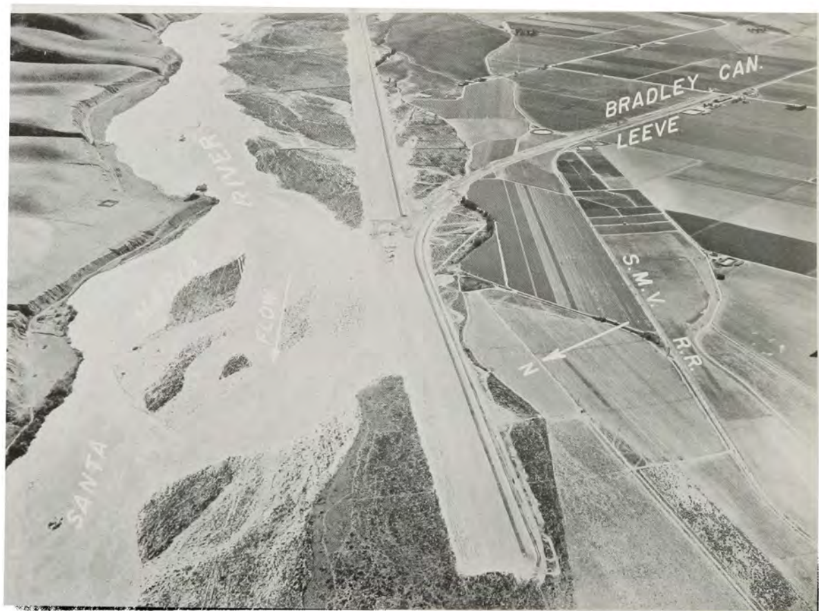
Upstream view of nearly completed Santa Maria Valley levee (December 1959).
