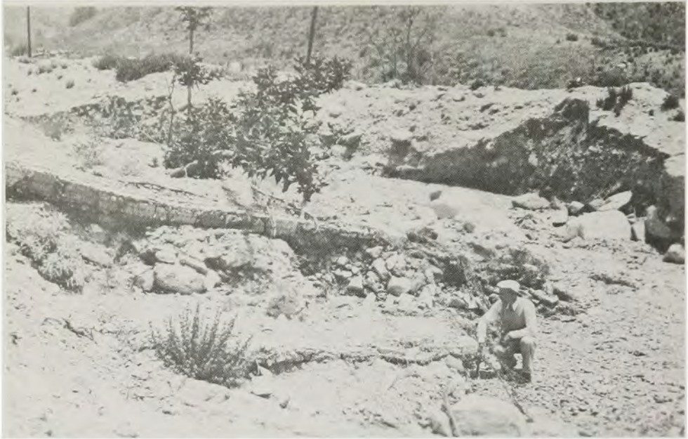
Debris left in Dunsmuir Canyon by the 1934 Flood, which destroyed the east half of the check dam.
