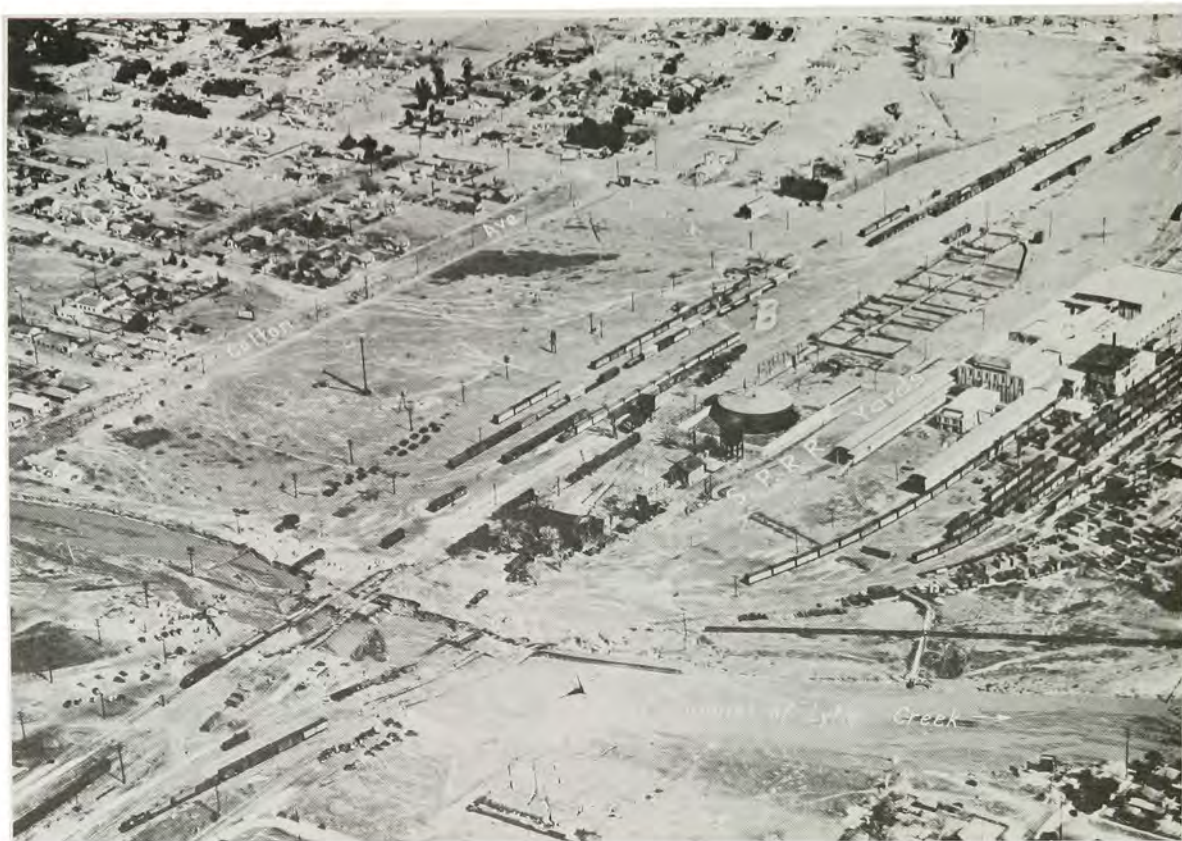
West channel of Lytle Creek at Colton, Calif., after the flood of March 1938, showing damage to transcontinental railroads and urban property.
