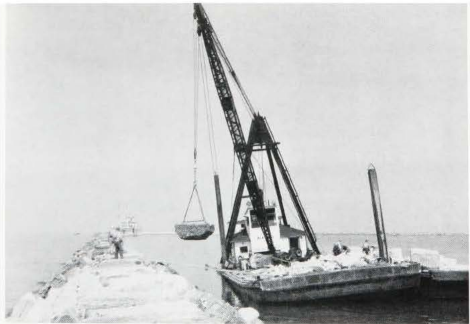
Repairs to West Arrowhead Breakwater, Oswego Harbor, New York, 1959
