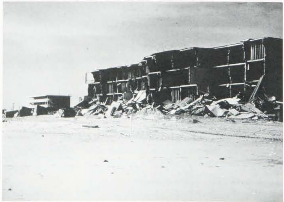
Storm Damage at Ocean City, Maryland, 1962
