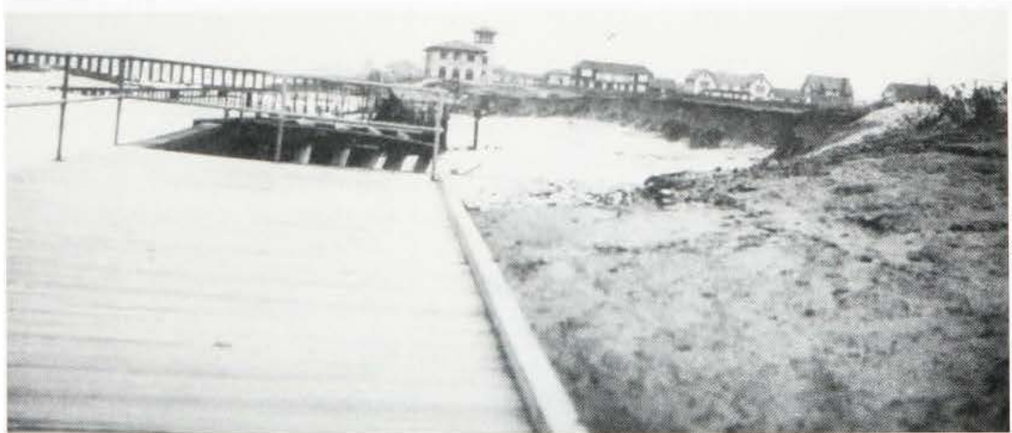
Beach Erosion at Cape May, New Jersey, 1935
