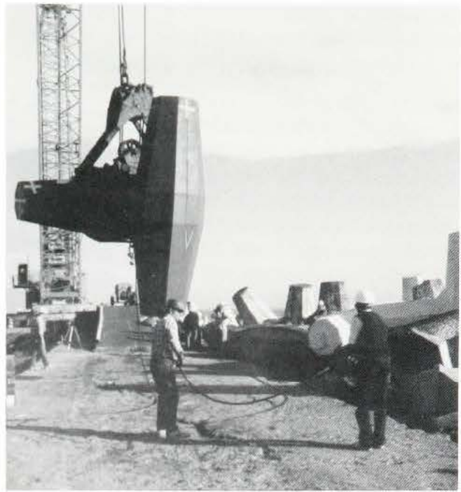
Use of Dolos for Construction at Crescent City, California, 1986
