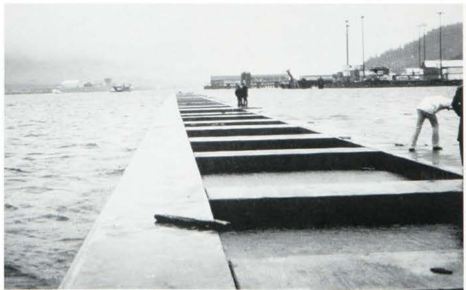
Floating Breakwater at Ketchikan, Alaska
