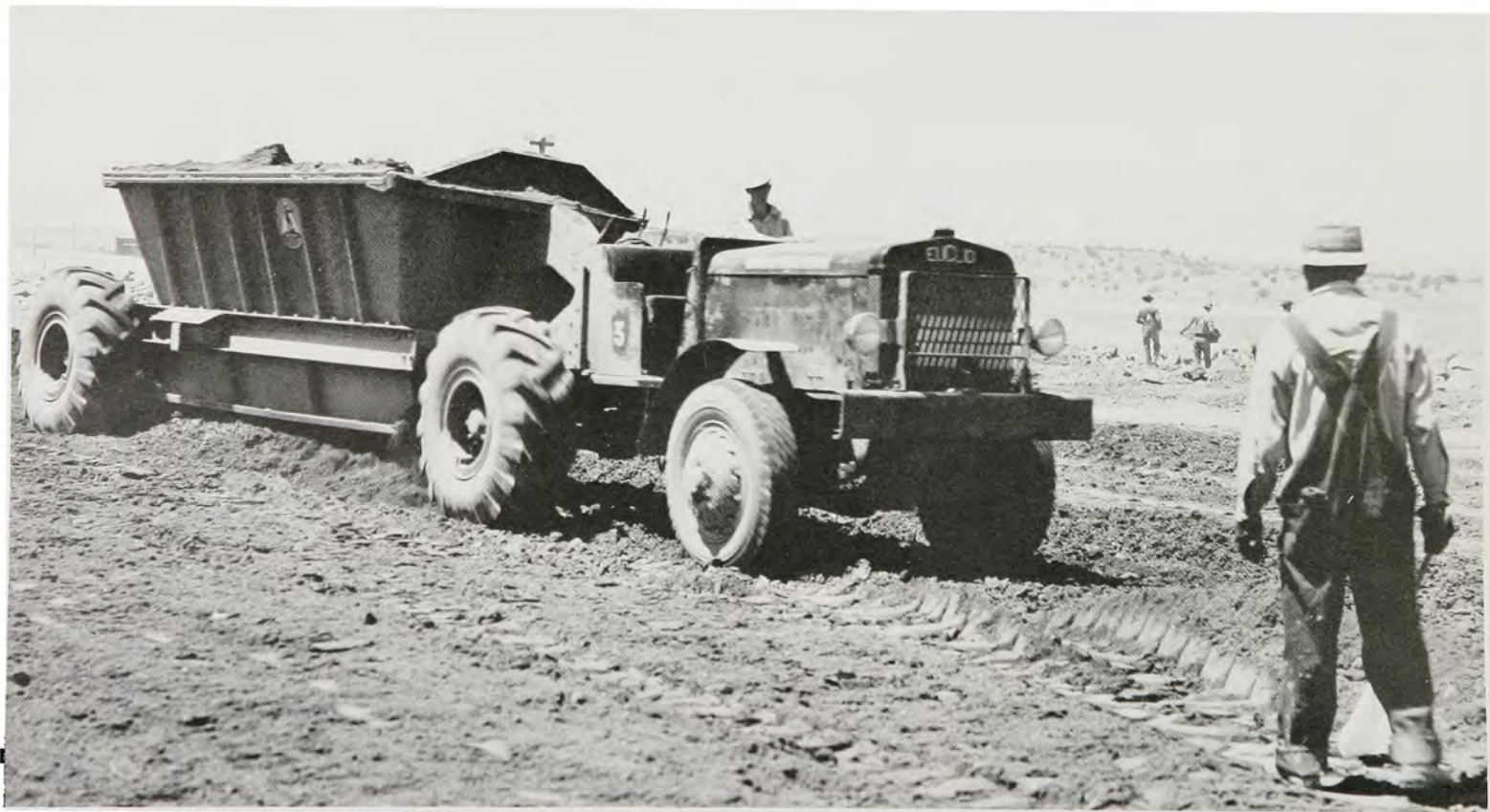
Plate No. 11. Dump Truck at South Dike, 1938
