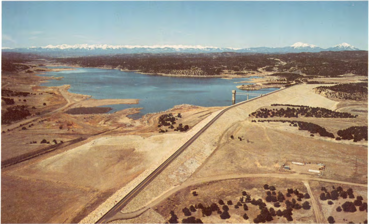
Plate No. 26. View of Trinidad Dam at Base of Sangre de Cristo Range, Colorado, 1985
