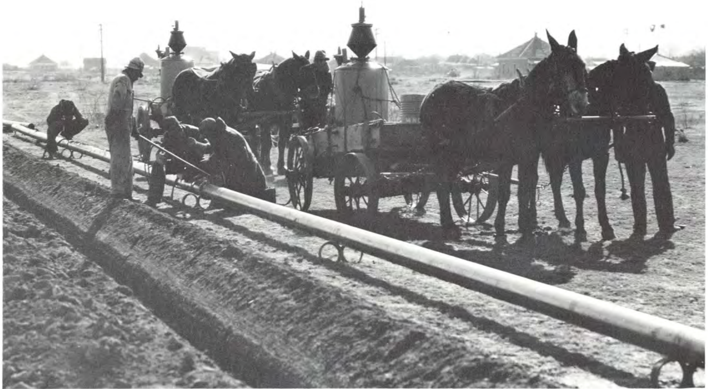
Plate No. 13. Welding Pipe for Gas Line, 1936
