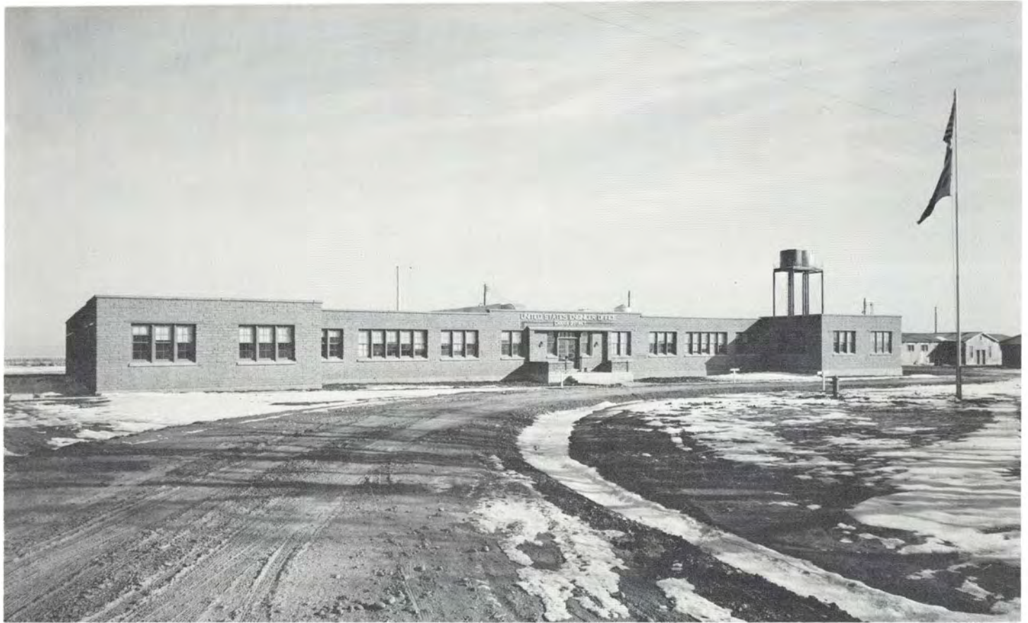
Plate No. 17. Caddoa District Headquarters, Caddoa Reservoir, 1940
