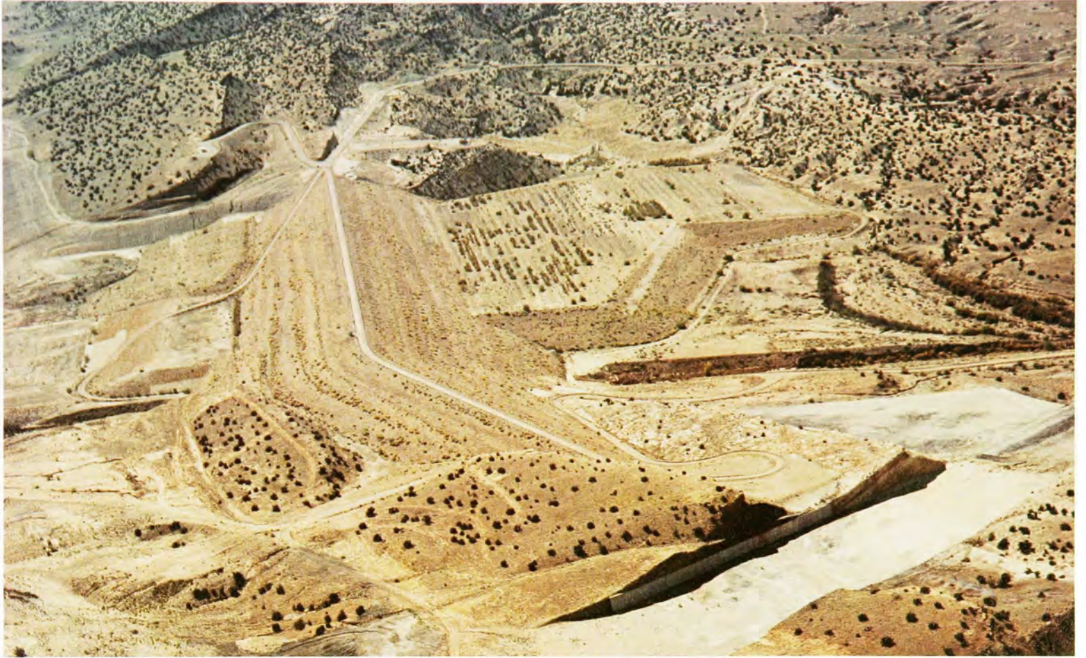
Plate No. 29. Aerial View of Galisteo Dam, South of Santa Fe, New Mexico, 1985
