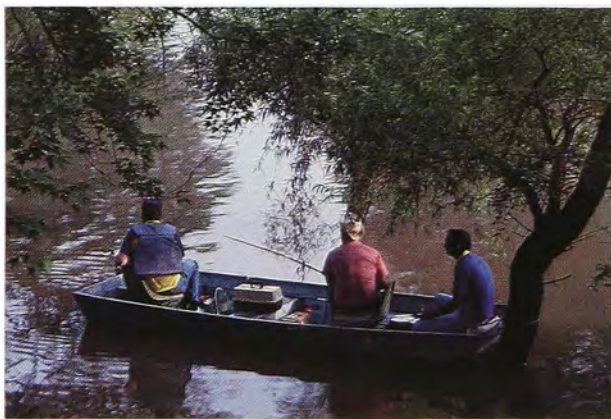
Fall River Dam in Greenwood County, Kansas: upper left, under construction, 1947, and completed, right. Lower left: fishing is a delight at Wister Lake on the Poteau River in eastern Oklahoma. The scenic and historic Wister area has been inhabited for thousands of years and contains numerous archaeological treasures.
