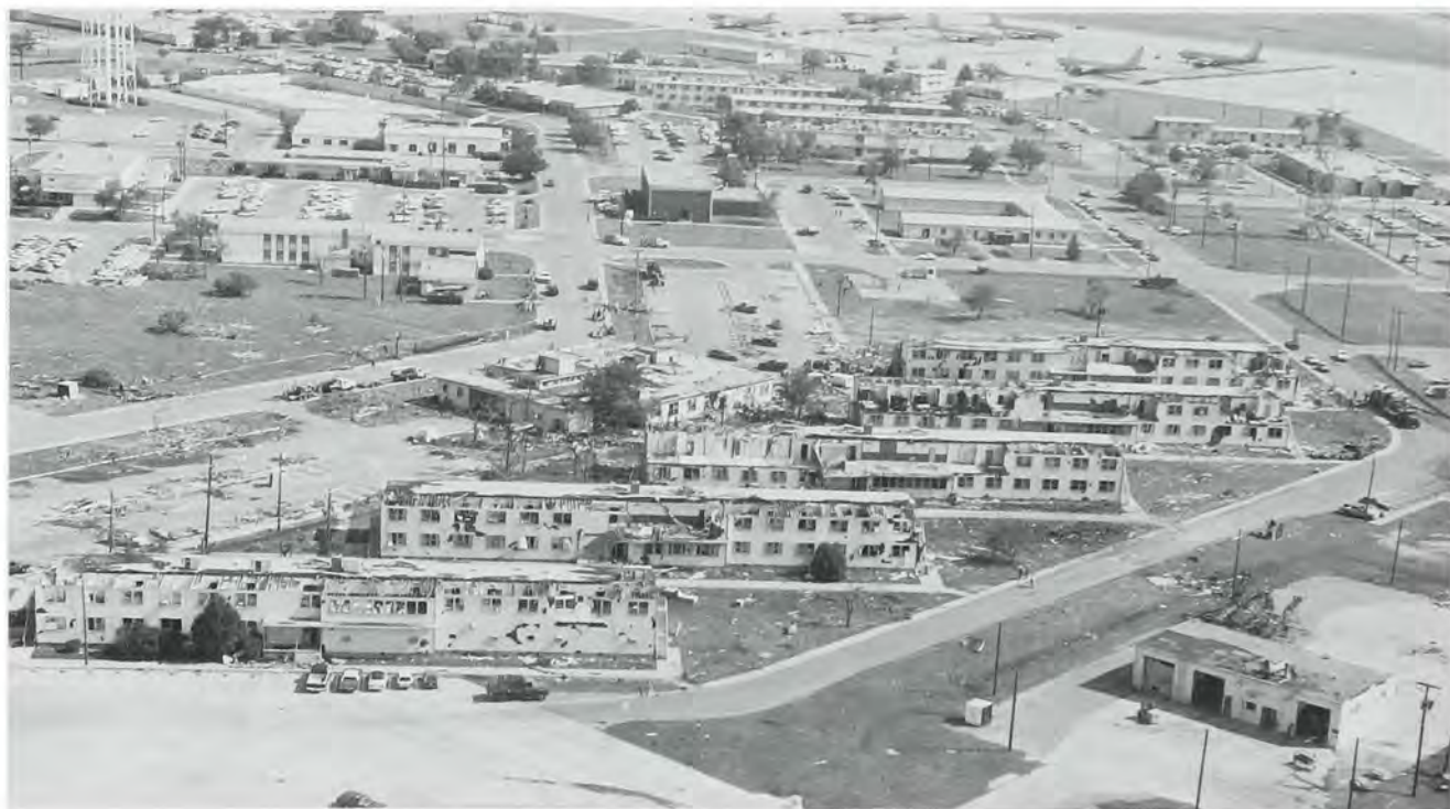
Tulsa District took the lead in repairing $14 million in damage at Altus Air Force Base from the 1982 tornado.
