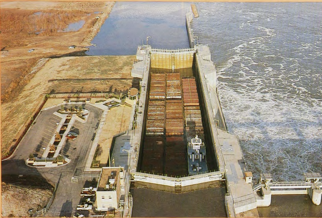
The McClellan-Kerr Arkansas River Navigation System: a 445-mile-long water stairway that rises 420 feet from the Mississippi River to Catoosa. Left, locking through Kerr Lock and Dam.
