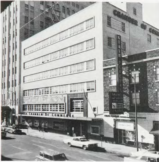
Tulsa Chamber of Commerce Building
