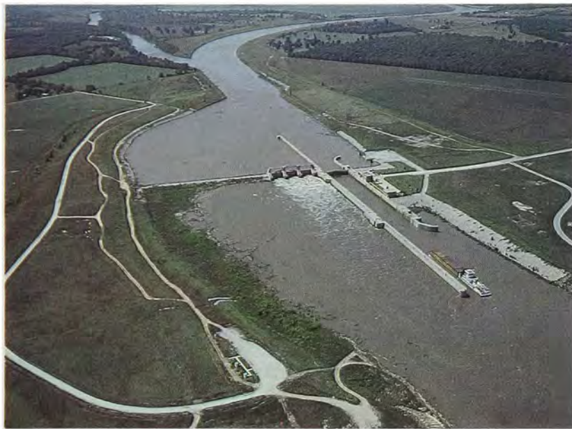
Top photo: Chouteau Lock and Dam. Bottom, Newt Graham Lock and Dam.
