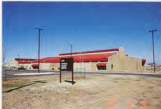
Among new construction projects: The physical fitness center and swimming pool at Fort Sill, shown here in exterior and interior photos.
