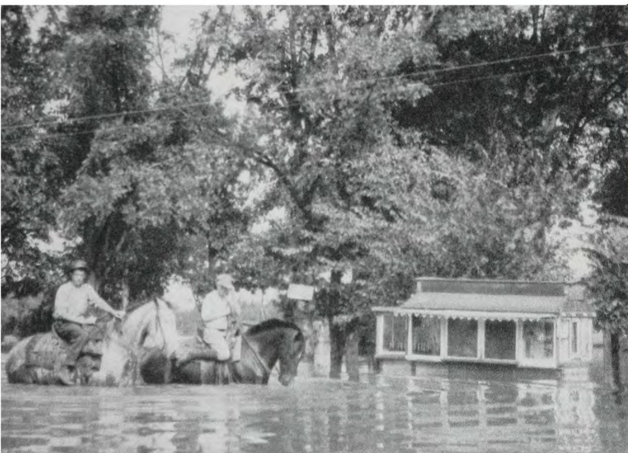
The Corps' number one peacetime problem was flooding, such as (bottom row, far left): the 1904 floods at Halstead and on the Walnut River in southeastern Kansas, and (near left) Bartlesville's 1912 flood. Above, Tulsa World cartoons poked gentle fun at the political possibilities of the 1908 flood.
