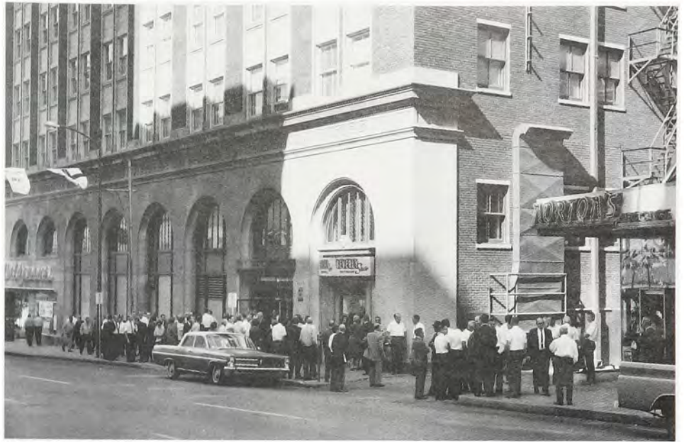
9 East Fourth Building
