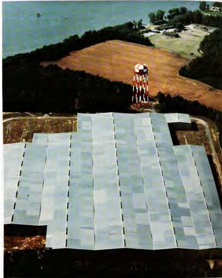
The fixed-bed Bay Hydraulic Model is molded in concrete to replicate the bathymetry of the Bay.
