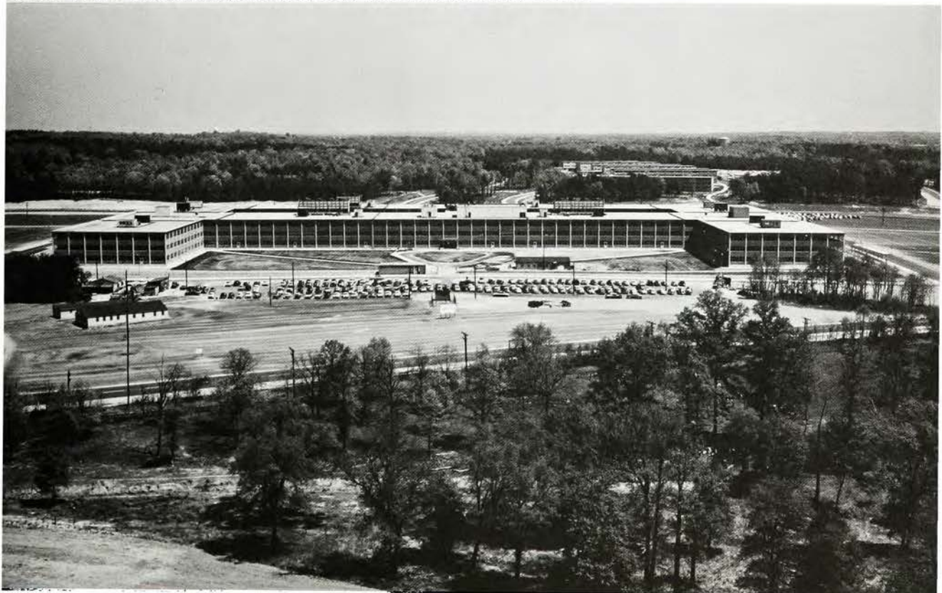
Operations Building, National Security Agency, Fort George G. Meade, Maryland, May 3, 1957.
