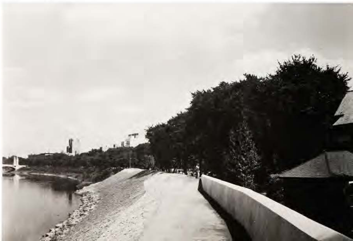
Upstream end of the levee designed to protect Wilkes-Barre from the Susquehanna's potentially dangerous flood waters, August 30, 1938. U.S. Army Corps of Engineers.—National Archives
