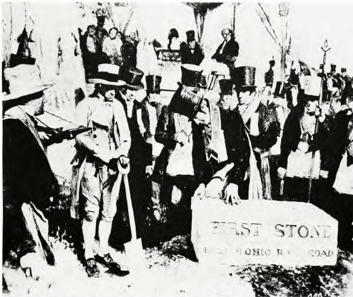
Ground breaking ceremony for the Baltimore and Ohio Railroad, July 4, 1828.—Library of Congress.
