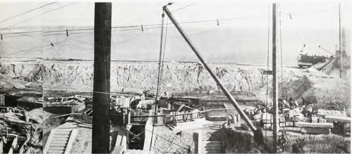
Hawkins Point during construction of gun emplacements in the spring of 1898. U.S. Army Corps of Engineers—National Archives.
