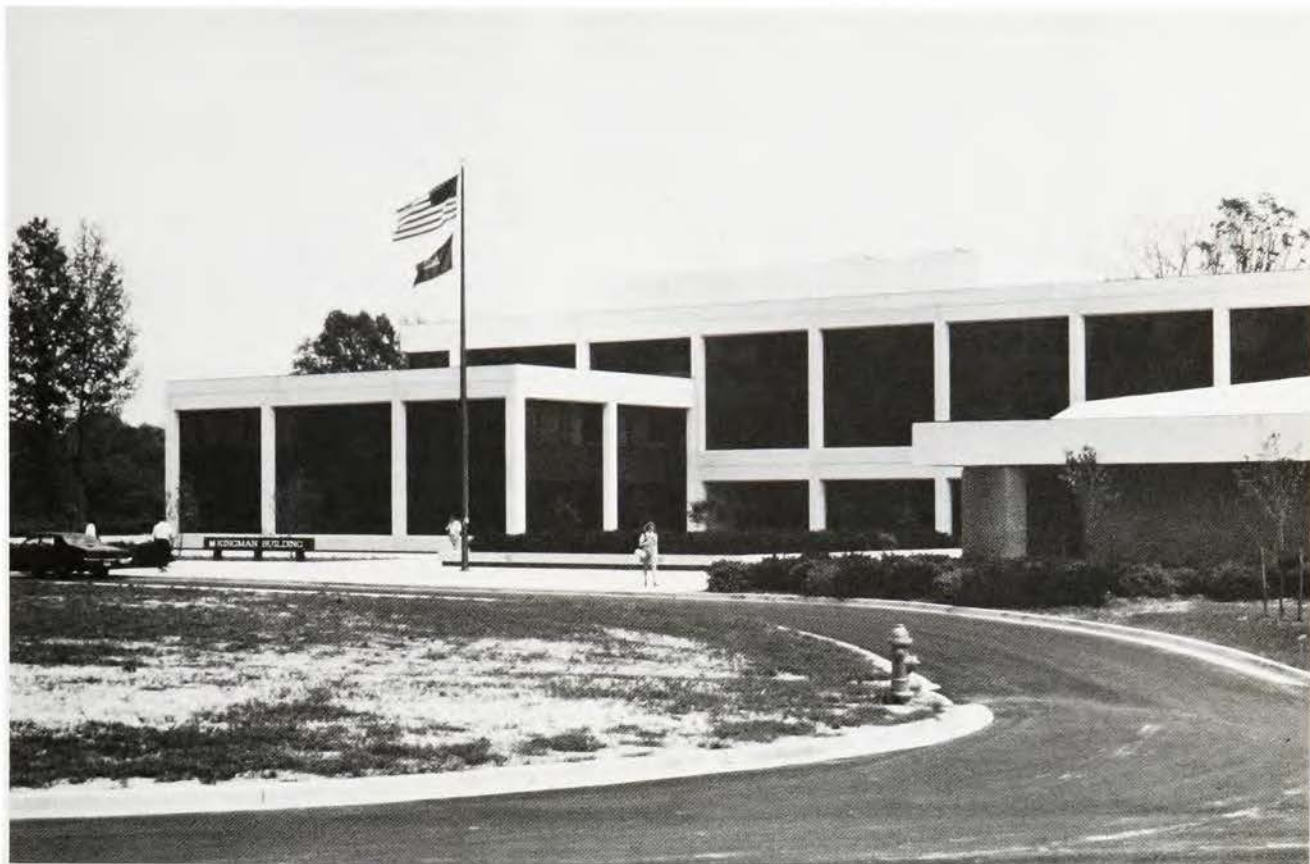
Kingman Building, Main Entrance
