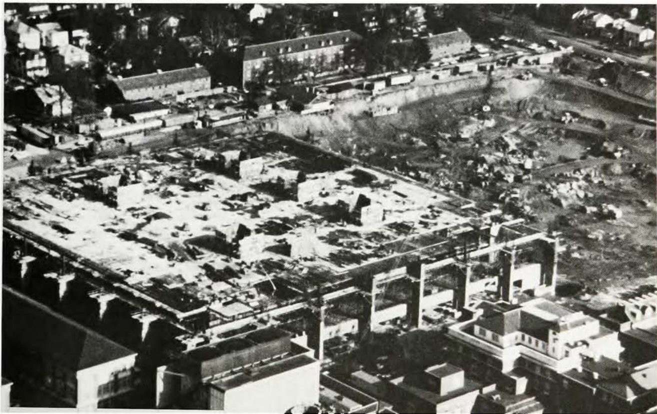
Construction of Walter Reed Army Medical Center
