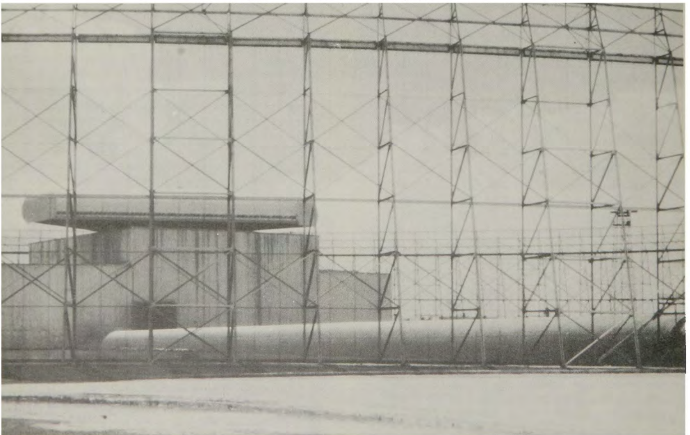
ZAR Radio Frequency Shielding Fence, Kwajalein.
