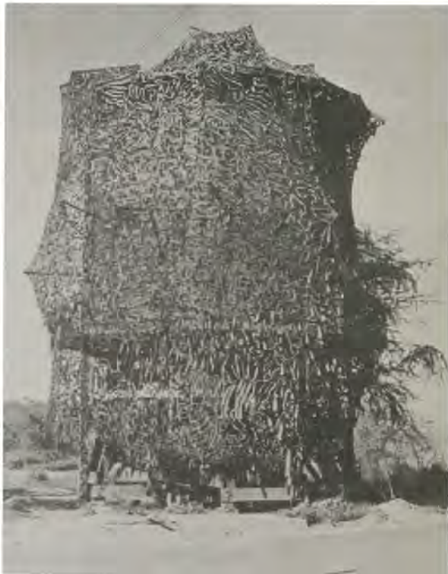
Camouflaged water tower on Kauai, early 1943.
