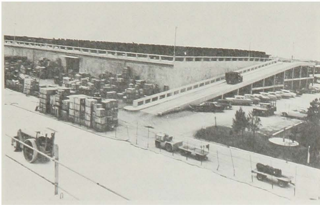
On-roof storage facilities at Machinato Service Area, Okinawa.
