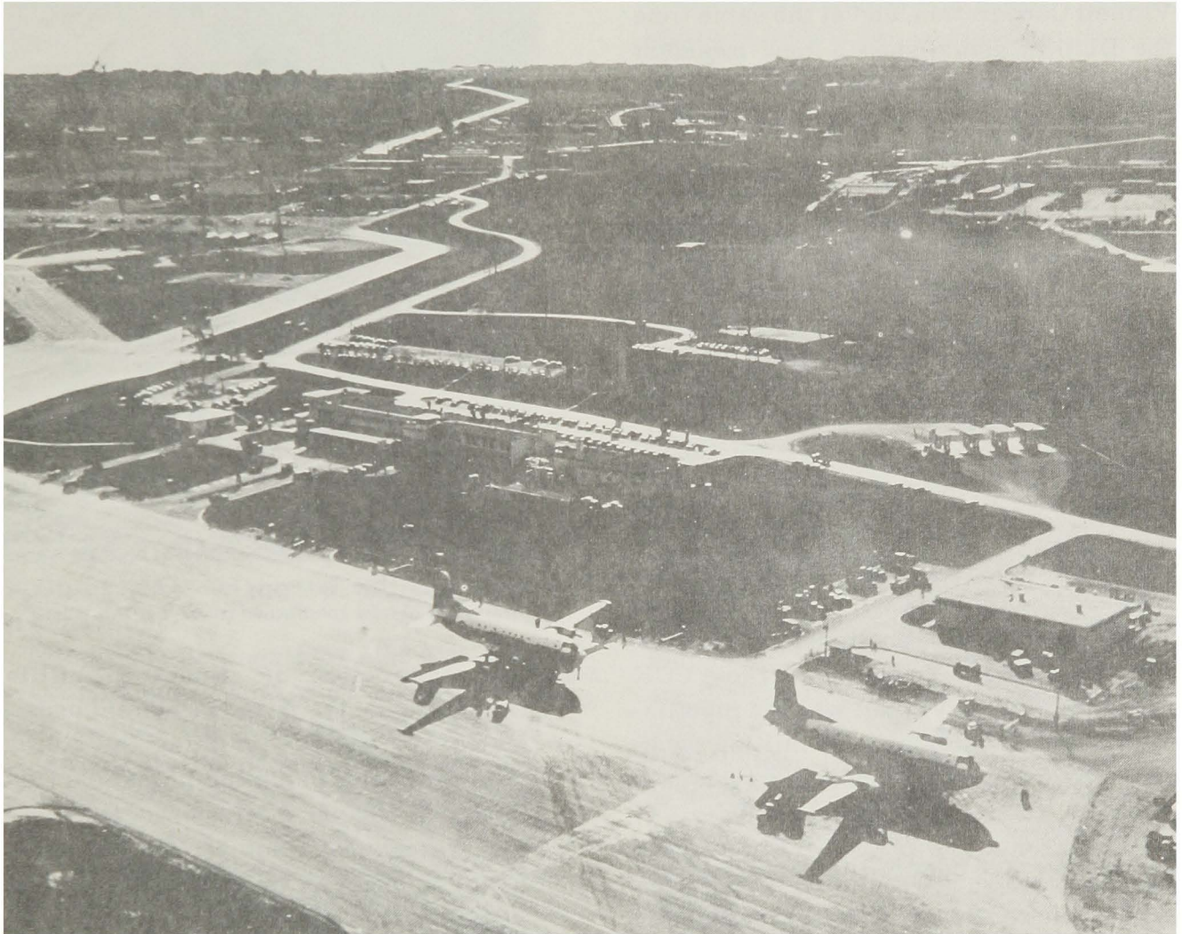
Airfield construction at CCK, Taiwan, around 1967.
