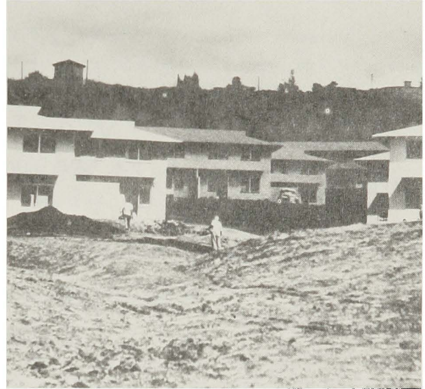
Capehart housing units built at Fort Shafter, Hawaii, January 1959.
