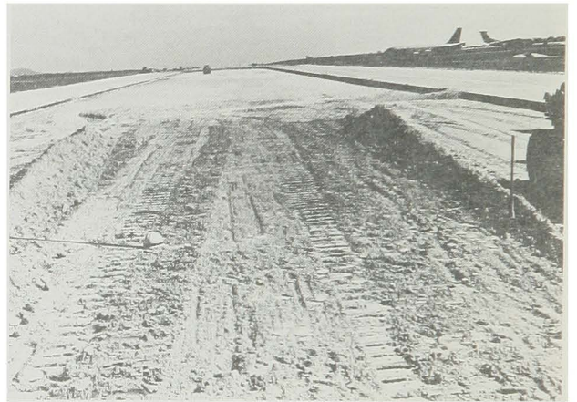
66-S airfield construction at Kadena Air Base.
