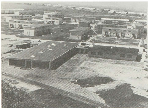
Addition to school built at Wakkanai, Japan, 1968.
