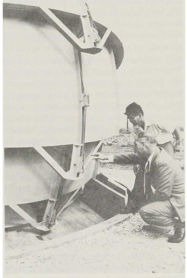
Close-up of the cable and pulley system which operates the Nike "clamshell" cover.
