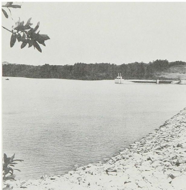
Reservoir at Tengan Dam, completed in 1968.
