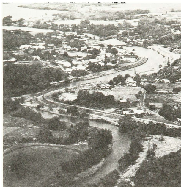
Flood control improvements built at Hanapepe, Kauai, Hawaii.
