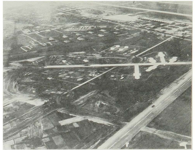
Paving of Kunsan Air Base, Korea, under 68-S, autumn 1968.
