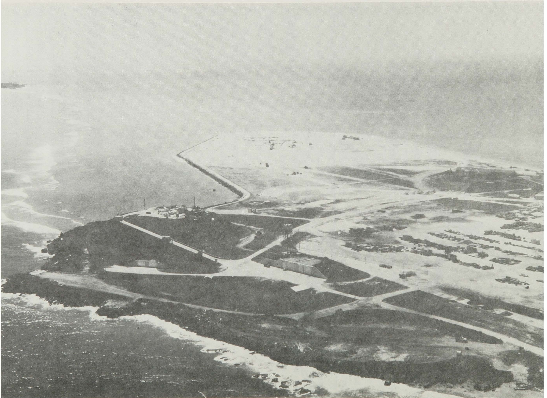
View of launch facilities constructed for Nike-Zeus on the western end of Kwajalein.
