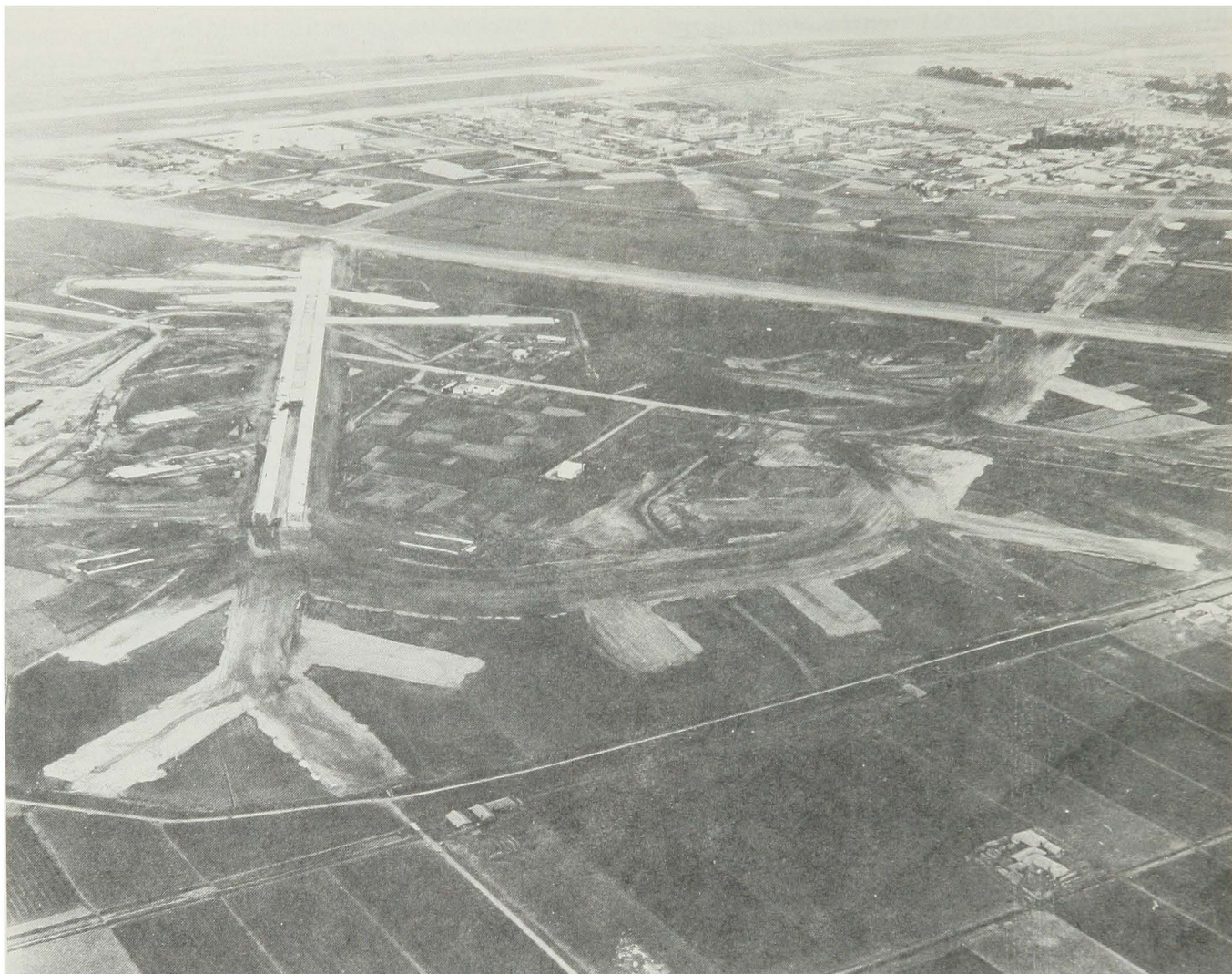
Paving at Kunsan Air Base, Korea, in late 1968.
