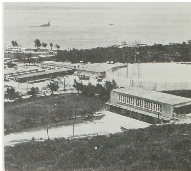
Water treatment plant at Ishikawa, Okinawa.
