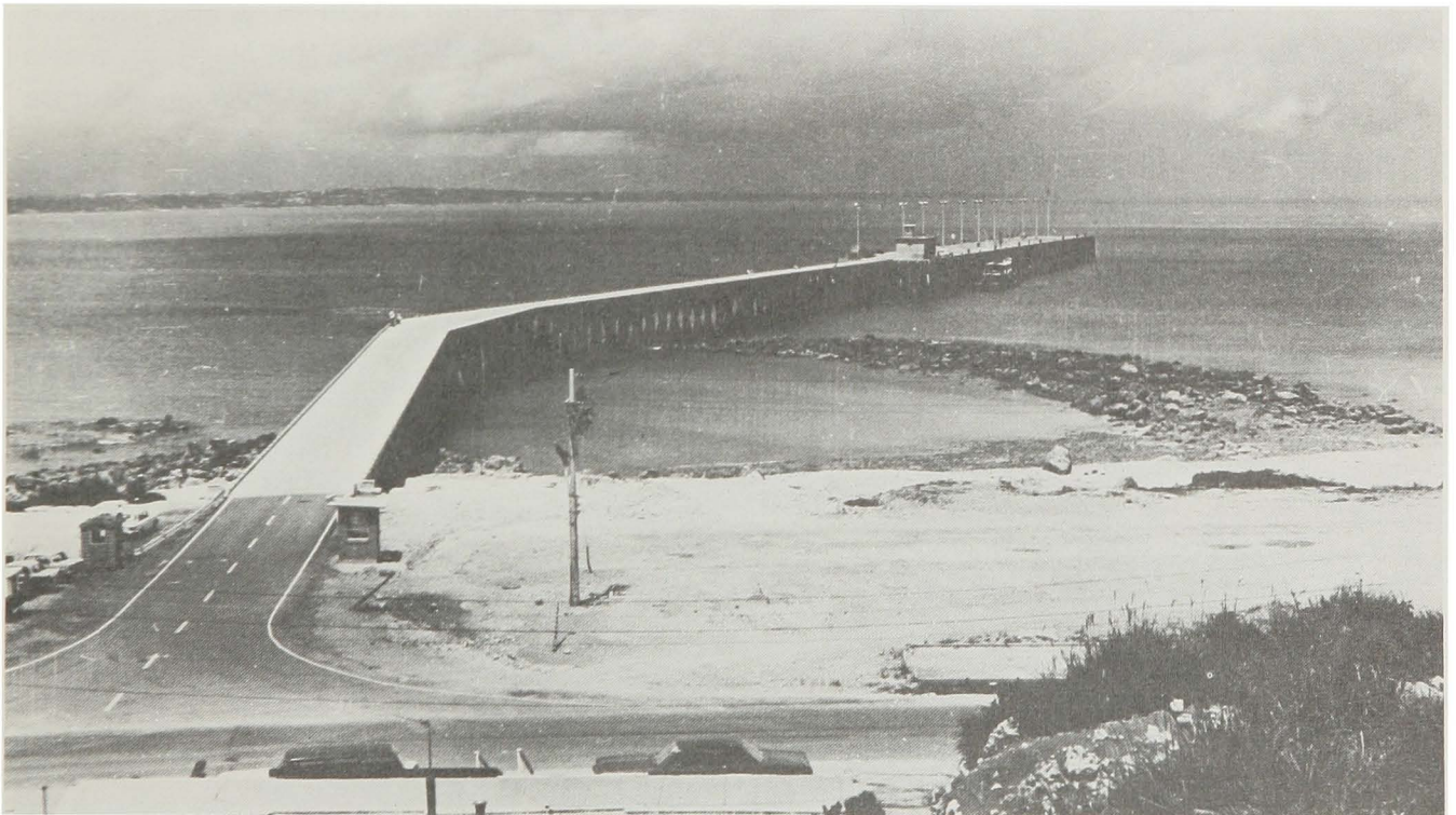
The completed pier at Tengan.
