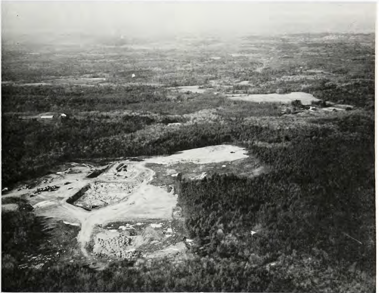
SHARPNER'S POND AFTER SUSPENSION OF WORK, MARCH 1970
