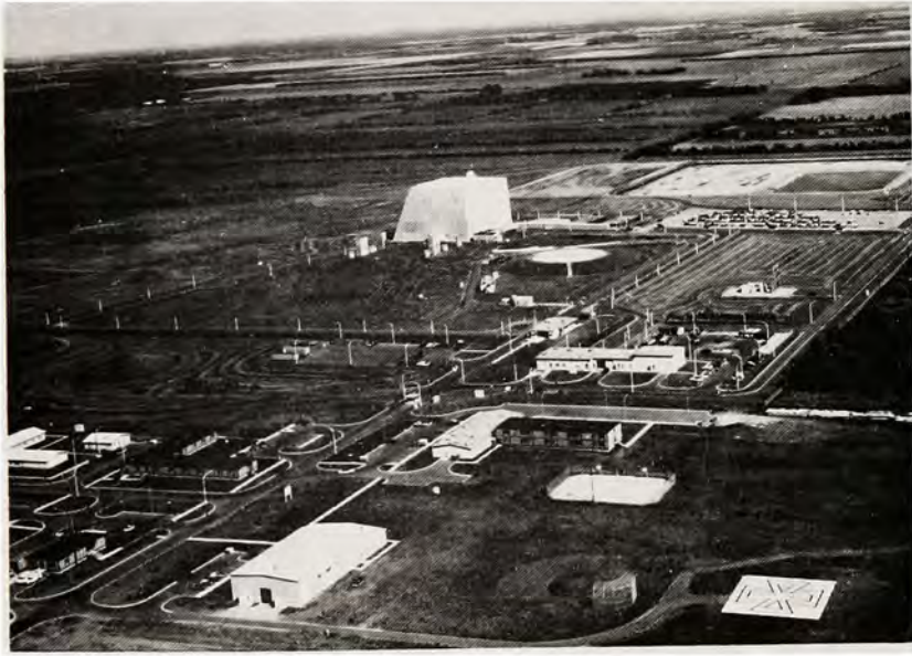
THE PERIMETER ACQUISITION RADAR SITE BEING CONSTRUCTED NEAR GRAND FORKS, NORTH DAKOTA. In the foreground are the nontactical and support facilities, in the center the Perimeter Acquisition Radar Building, the intake and exhaust stacks of the Power Plant, the circular buried Heat Sink and in the background the waste disposal systems.
