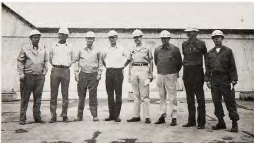
TRANSFER OF THE FIRST OF THE MAJOR TACTICAL BUILDINGS OF THE NORTH DAKOTA SAFEGUARD BALLISTIC MISSILE DEFENSE SYSTEM, the Perimeter Acquisition Radar Building, from control of the Huntsville Division to the Safeguard System Command on August 21, 1972. From left to right: S.N. Purinton, PAR Project Manager, M-KA; G.W. Gilfillan, Division Manager, Missile and Space Division, M-K; A.D. (Doc) Poteat, Resident Manager, M-KA; Paul C. Steidl, PAR Resident Manager; Colonel Lochlin W. Caffey, Contracting Officer and Deputy Division Engineer, Huntsville; Brigadier General Bates C. Burnell, Huntsville Division Engineer; Barney L. Trawicky, Chief, Construction Division, Huntsville; and Colonel John L. Lillibridge, Grand Forks Area Engineer.
