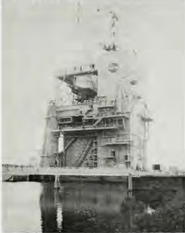
TEST STAND B2, "Main Propulsion Test Article" stand extensively remodeled at NSTL.
