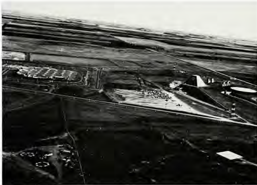
TACTICAL FACILITIES OF THE SAFEGUARD BALLISTIC MISSILE DEFENSE SYSTEMS' MISSILE SITE RADAR site constructed near Grand Forks, North Dakota. Right foreground is the Helipad; right is the circular underground heat sink; to its left the intake and exhaust stacks of the underground power plant; the turret of the partially buried Missile Site Control Building; to the left the Spartan and Sprint Missile Fields; and the mounded earth covered Missile Assembly Building.
