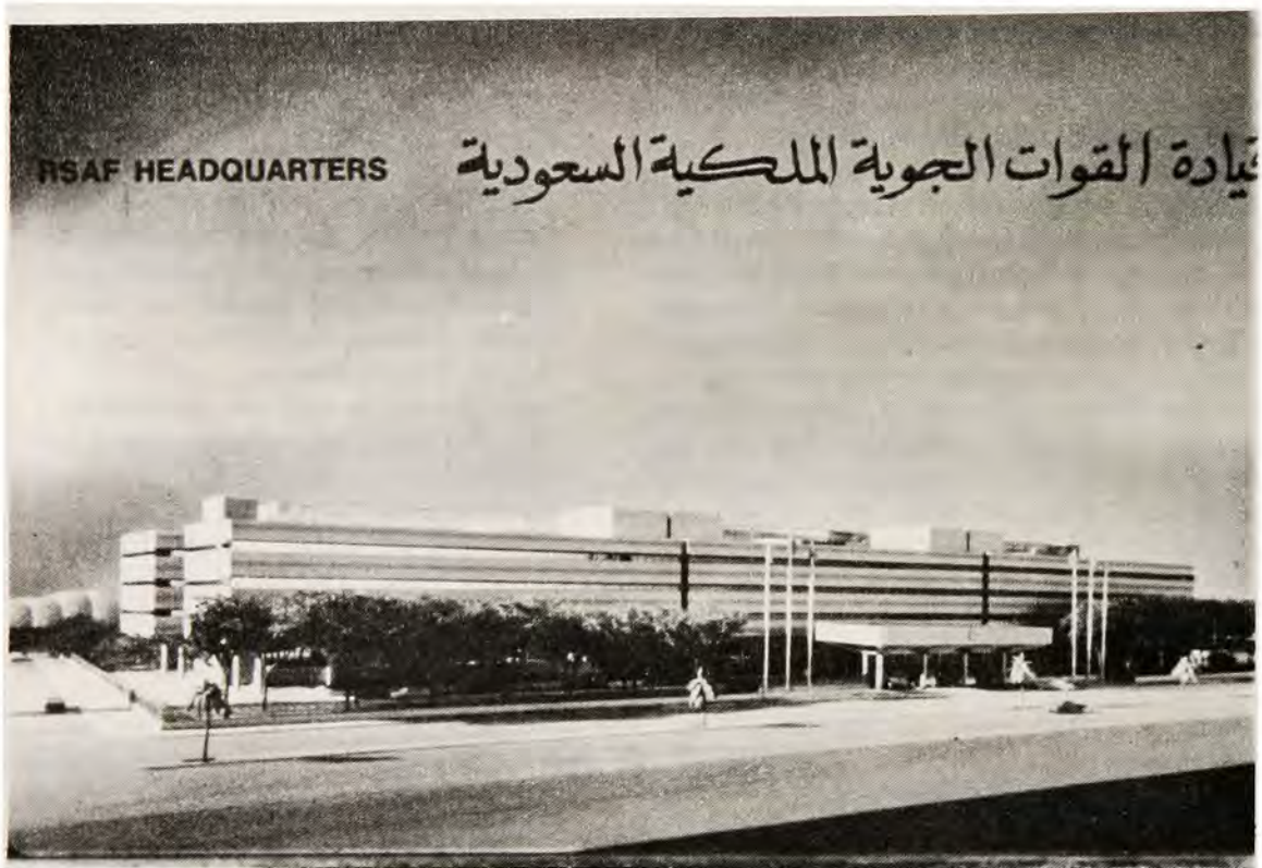
Royal Saudi Air Force Headquarters (RSAF) as constructed by the Corps.
