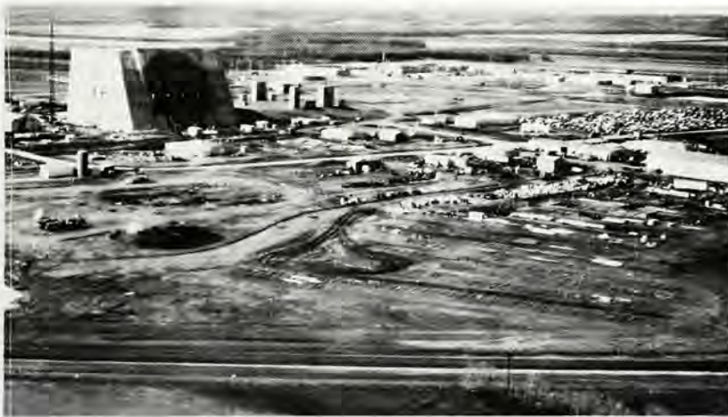
PAR FACILITIES of the SAFEGUARD Ballistic Missile Defense near Grand Forks, North Dakota, as they appeared on April 19, 1972. At the upper left is the PAR control building with its associated power plant to the right. In the background are some of the support facilities of the installation. In the center and on the right are temporary contractor buildings and workers' automobiles.
