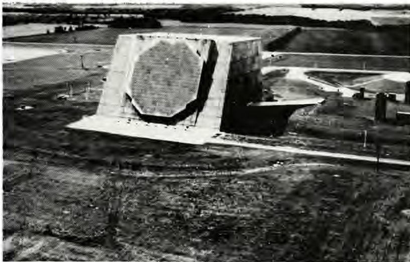
THE NORTH SIDE or face of the PARB with the intake and exhaust stacks of its underground power plant on the right.
