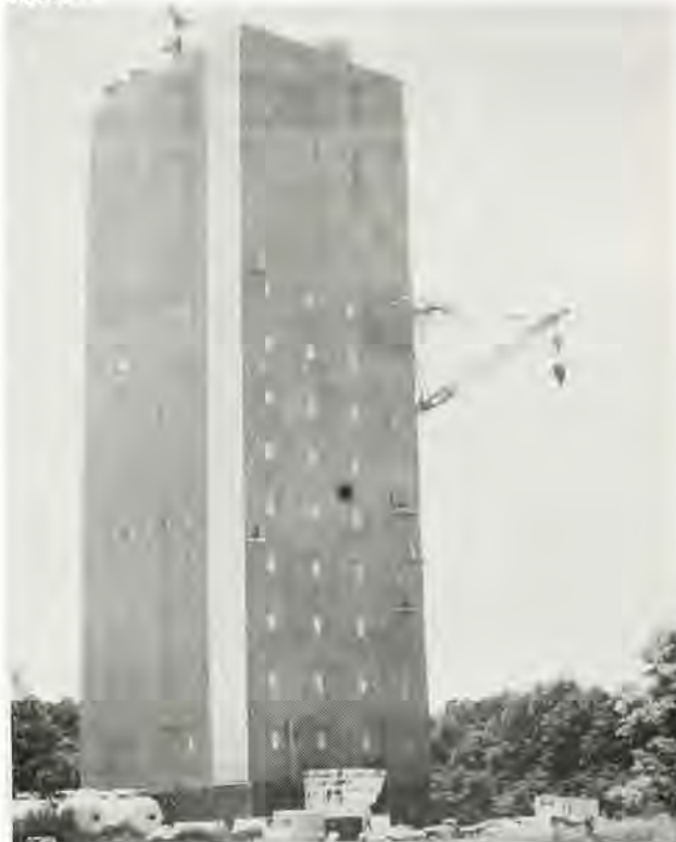
"SPACE SHUTTLE MATED GROUND VIBRATION TEST FACILITY" (Building 4450 Marshal Test Center) converted for Space Shuttle Testing.
