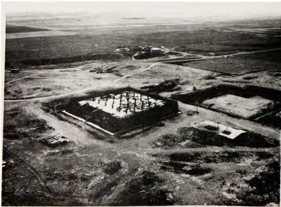
THE MALMSTROM PERIMETER ACQUISITION RADAR site as it appears looking from the southwest after completion of Phase I construction and clean-up. The control building is center with the straw covered base slab of the power plant on the right. In the background is the water reservoir and tank.
