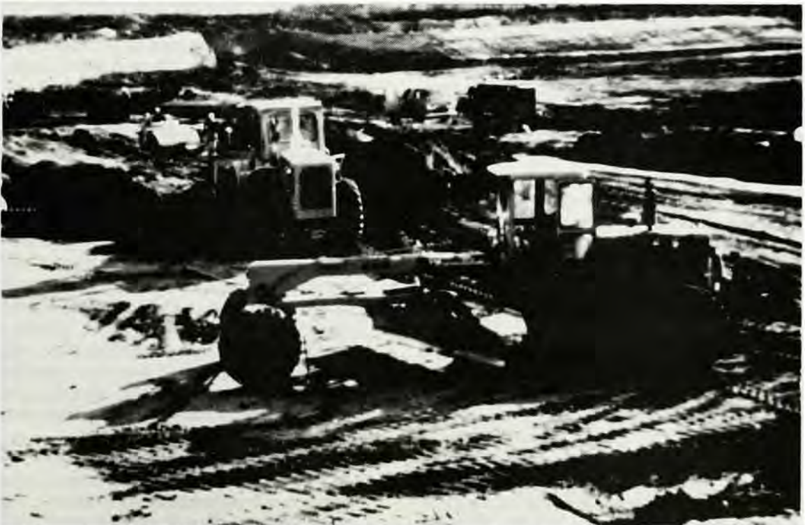
Grand Forks North Dakota SAFEGUARD construction start up 15 May 1970.
