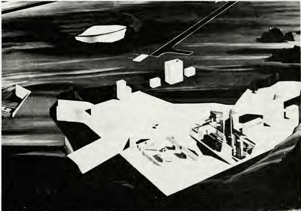
BMD POWER PLANT CUTAWAY. Underground entrance on left, heat sink at upper left, cooling towers upper right, and intake and exhaust stacks in center of rendering.
