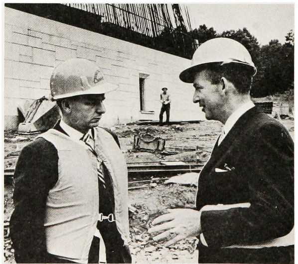
Brig. Gen. Frederick J. Clarke (Right) with Sen. Robert C. Byrd of West Virginia During Construction of the Roosevelt Bridge, 1961.
