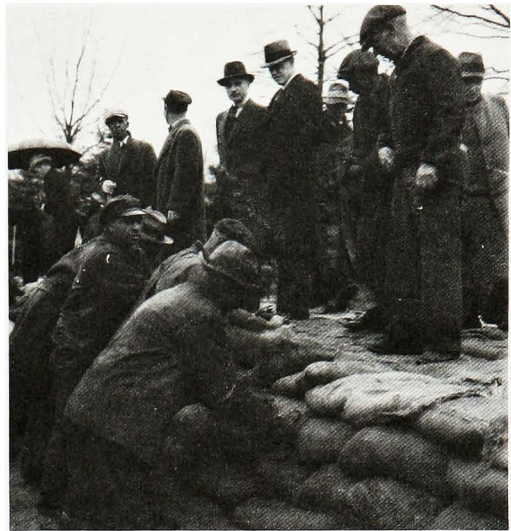
Lt. Col. Francis C. Harrington and Harry Hopkins (Center, Above) Watching Workmen Erect an Emergency Levee, Washington, 1936.
