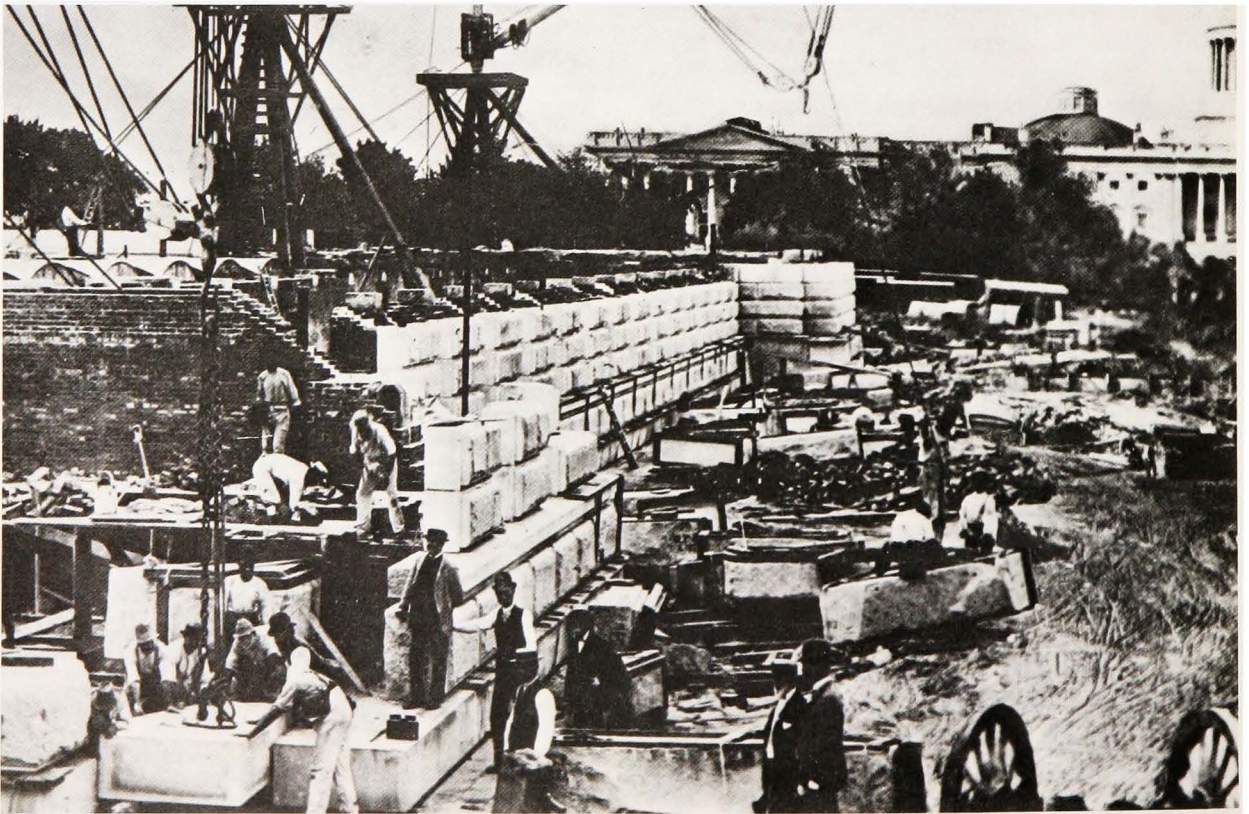
Building the Library of Congress.
