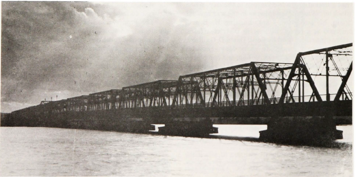
The Railroad Bridge, 14th Street.
