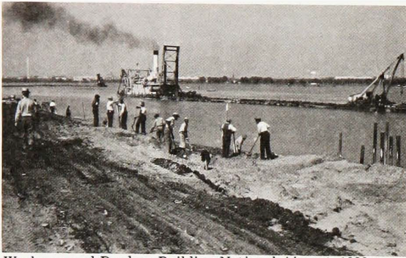
Workmen and Dredges Building National Airport, 1939.
