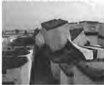
Figure 5. Collapsed JLIST Containers
