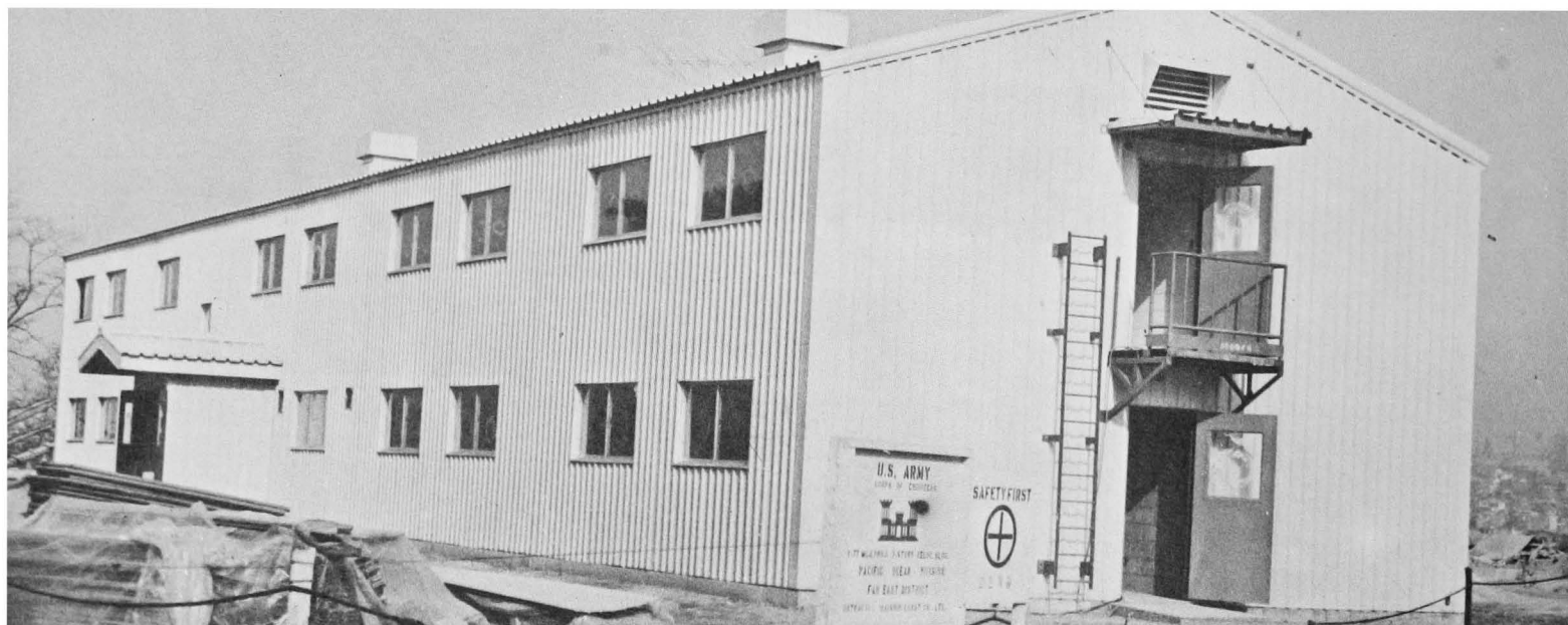
A two-story relocatable building, Yongsan
