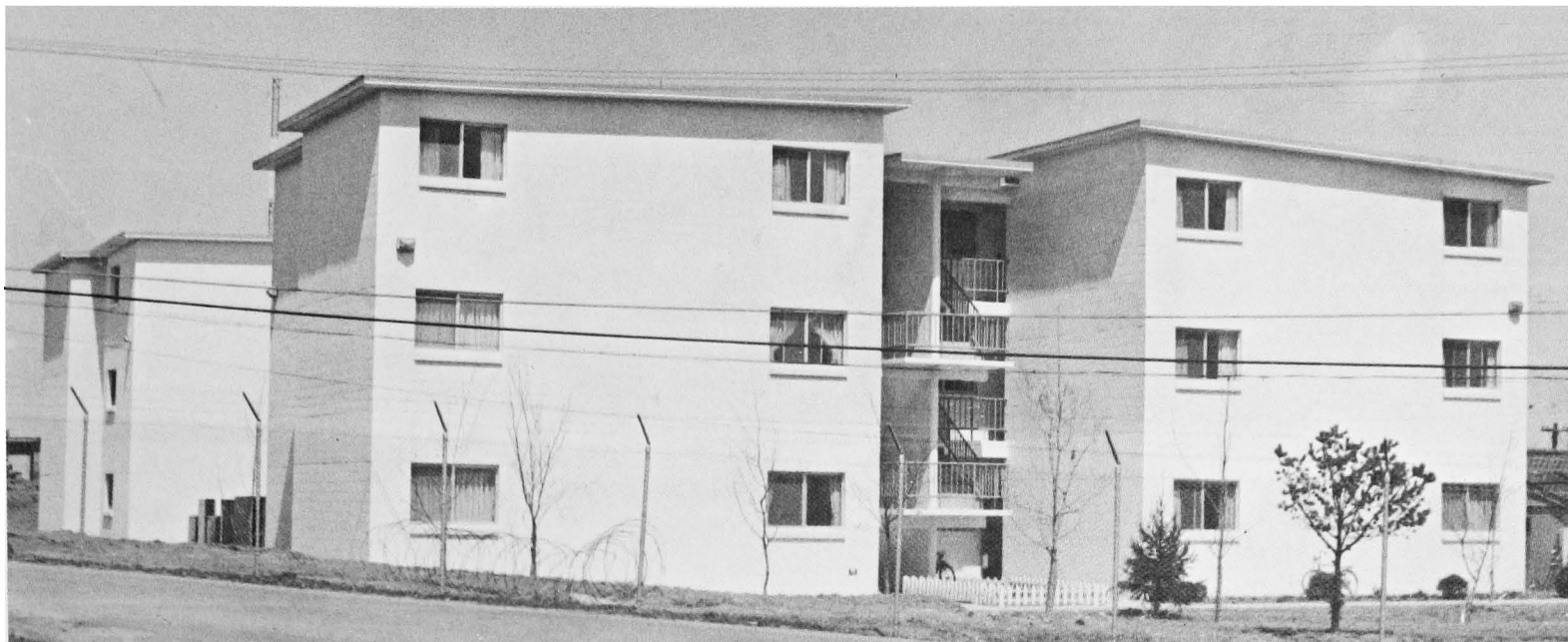
Centrally air conditioned 60 man BOQ at Camp Humphreys
