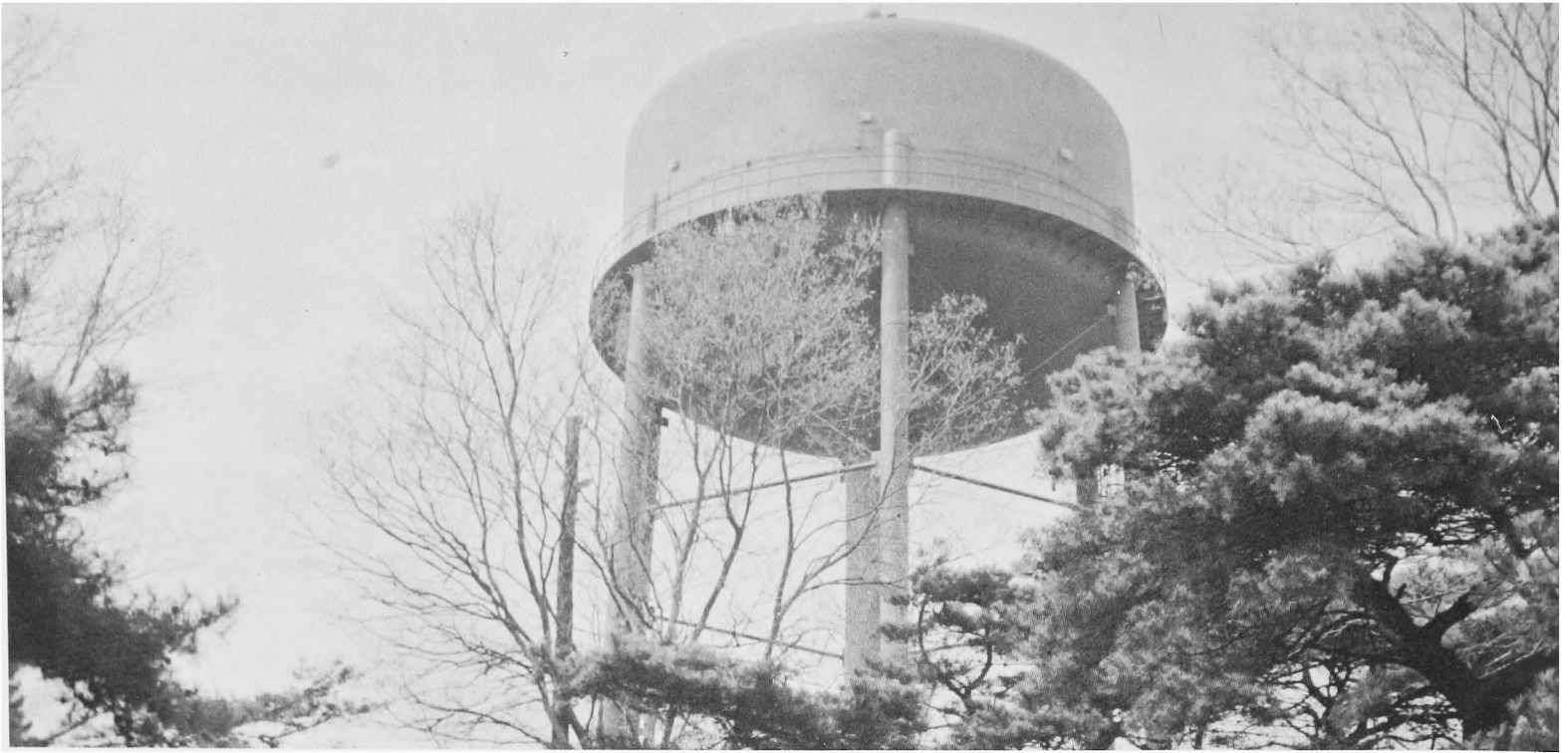
500,000 gallon water storage tank, Kunsan Air Base
