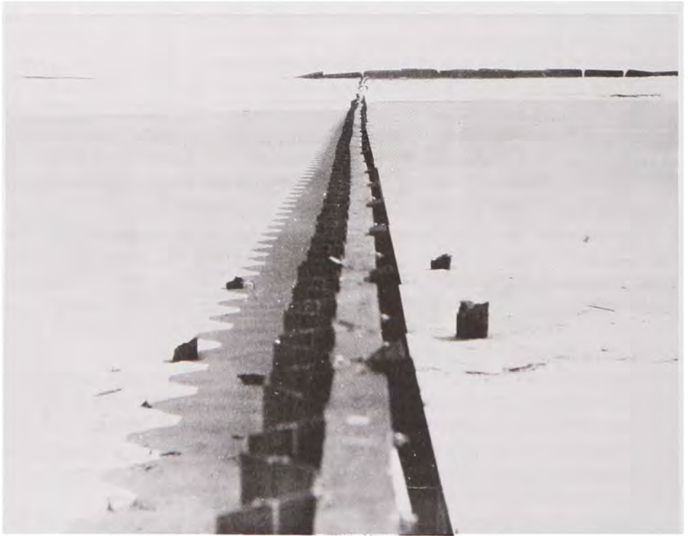
Groin No. 1 built by the MacDougald Company to help protect Fort Screven from beach erosion, looking east toward the ocean as of 12 February 1931. Notice the construction of interlocking steel sheet piles bolted to a frame of creosoted wood. The remains of the old Quartermaster Corps seawall can be seen in the distance. (Savannah District, Corps of Engineers)
