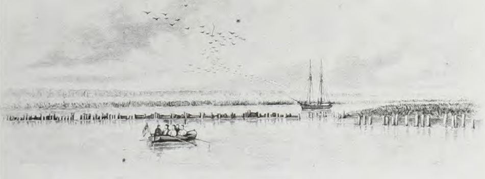
REBEL OBSTRUCTIONS IN THE NORTH CHANNEL OF THE SAVANNAH RIVER, GA., A FEW DAYS BEFORE THE CAPTURE OF FORT FISHER.
