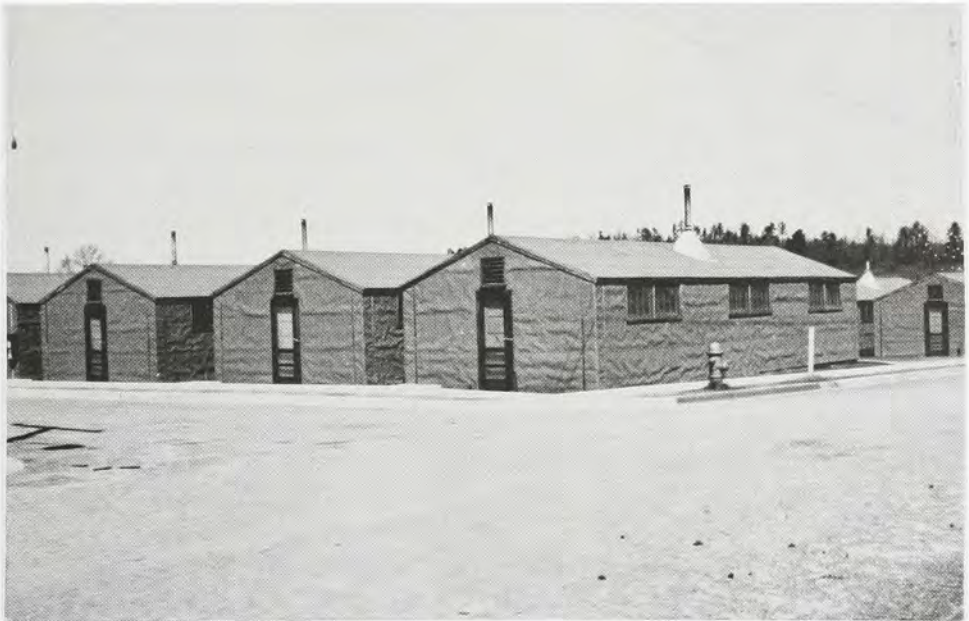
Enlisted men's hutments at Camp Toccoa, April 1944. These buildings show one type of temporary construction used by the Corps of Engineers during World War II. They had concrete floors, 90-weight composition roofs, and walls of siding insulated with gypsum board covered with tar paper. (Savannah District, Corps of Engineers)
