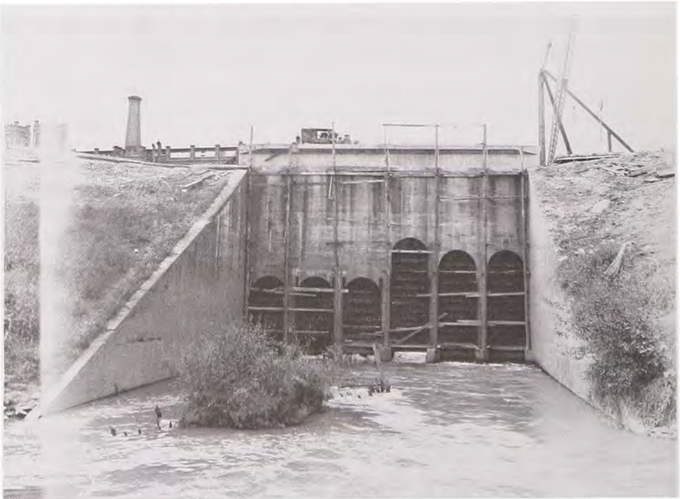
Sibley Mill Gates on the Augusta Levee as of 26 October 1939 and prior to improvement. (Savannah District, Corps of Engineers)
