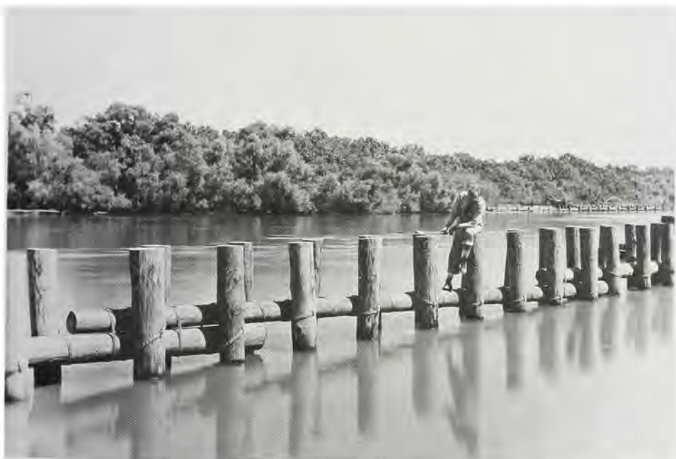
An example of a permeable pile dike built on the Altamaha River by contract with the C. Y. Thomason Company. Such structures were used for channel contraction. 3 October 1940. (Savannah District, Corps of Engineers)
