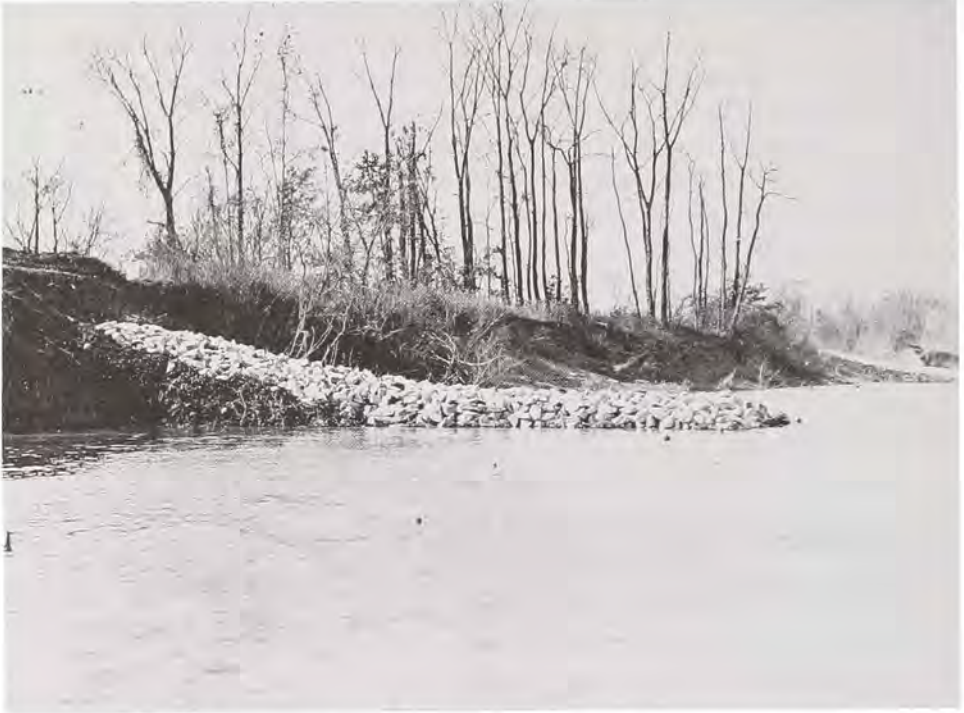
A spur dam on the Savannah River below Augusta in 1924. This type of construction was used by the Corps of Engineers in the early 20th century for contraction of river channels and protection of river banks. (Savannah District, Corps of Engineers)
