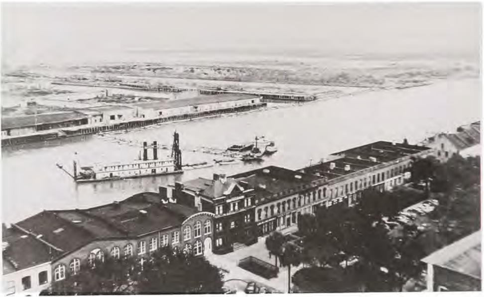
The U.S. pipeline dredge Henry Bacon at work in Savannah Harbor in the early 1950s. Notice the long pipeline leading to spoil sites on Hutchinson Island. (Savannah District, Corps of Engineers)
