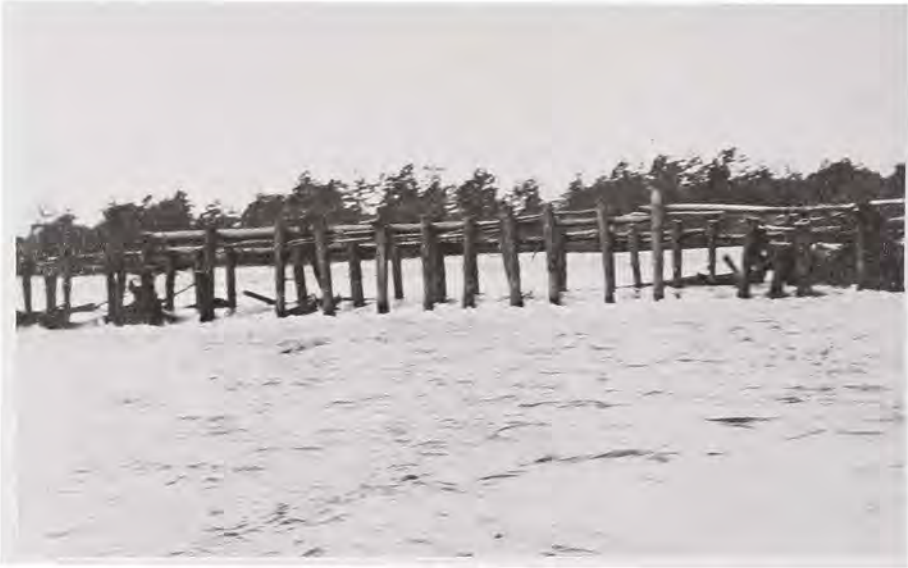
A May 1914 view of an earlier closing dam built by the Corps of Engineers at Jacks Suck, a cut off across an oxbow of the Altamaha River, as seen from the down stream side. (Savannah District, Corps of Engineers)
