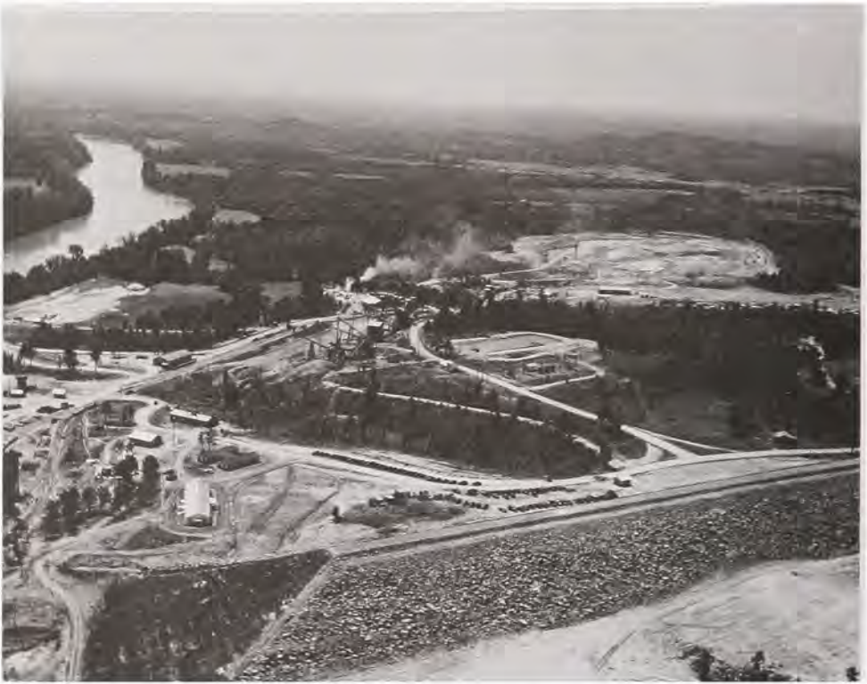
Clark Hill construction. This view of the construction site at the Clark Hill Dam shows the embankment on the Georgia side of the river (foreground), the reservoir (center), the quarry (far right), the aggregate storage piles (left center), and the construction buildings. 1948. (Savannah District, Corps of Engineers)
