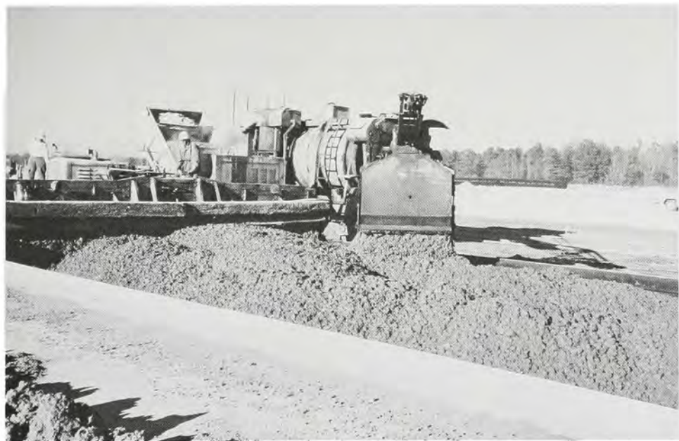
Paving operations for the SAC Airfield at Robins Air Force Base, 16 December 1958. (Savannah District, Corps of Engineers)
