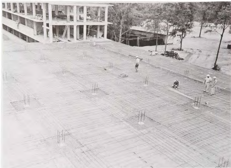
Construction of Airmen's Dormitories, Hunter Air Force Base, 20 May 1953. (Savannah District, Corps of Engineers)
