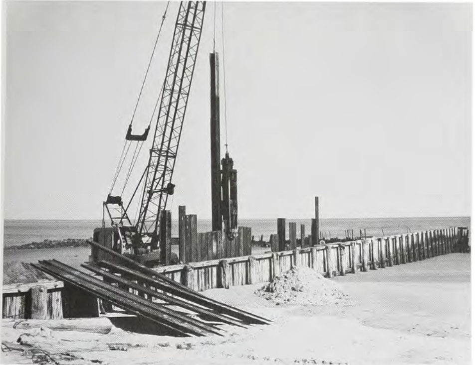
View of the construction of a groin in the beach erosion control program on Tybee Island, Georgia. (Savannah District, Corps of Engineers)
