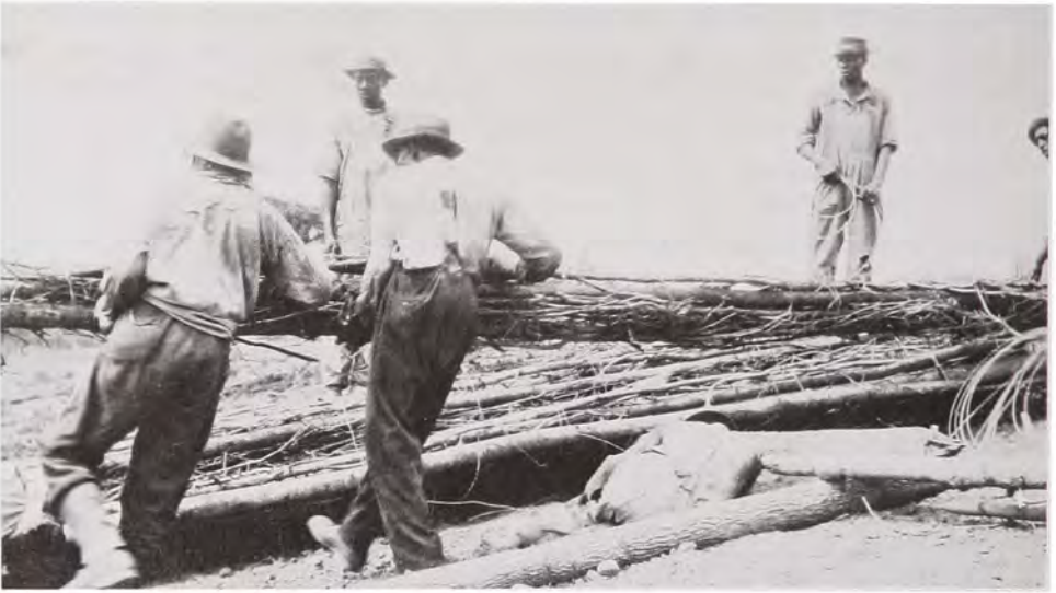
Workers constructing brush mattresses of fascines for use in bank protection works on the Savannah River below Augusta in July 1923. This particular mattress was composed of two layers of fascines and measured 21 feet by 200 feet. There were 358 fascines used in this mattress which took 13 men six hours to build. (Savannah District, Corps of Engineers)
