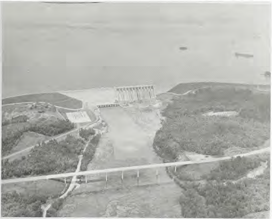
Aerial view of the Hartwell Dam showing the new highway bridge that had to be constructed across the Savannah River below the dam. Note the twelve taintor gates in the main spillway section, the powerhouse to the left of the spillway, the switchyard to the extreme left, and the impounded reservoir behind the dam. (Savannah District, Corps of Engineers)
