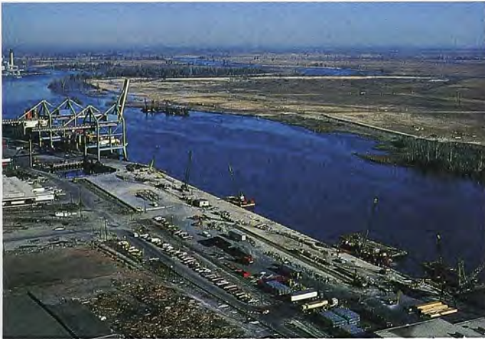
B. construction getting under way in 1980
