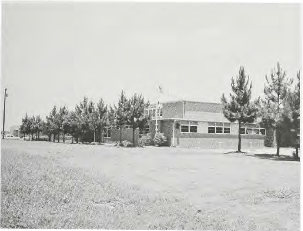
The U.S. Army Reserve Training Center Armory, Columbus, Georgia, 29 June 1960. (Savannah District, Corps of Engineers)
