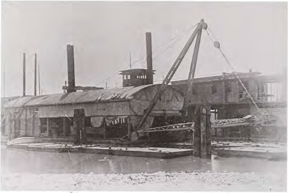
The U.S. pipeline dredge Macon, seen here in November 1921, was part of the government plant used in the improvement of the rivers of the Altamaha System. (Savannah District, Corps of Engineers)
