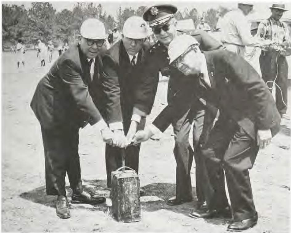
Four participants stand ready for the detonation exercise that signalled the start of construction of the West Point Dam project. Left to right: Congressman George Andrews (Ala.); Congressman John J. Flynt, Jr. (Ga.); Major General George H. Walker, South Atlantic Division Engineer; and Schaefer Heard, who initiated the process which brought the project into being. April 1966. (Savannah District, Corps of Engineers)
