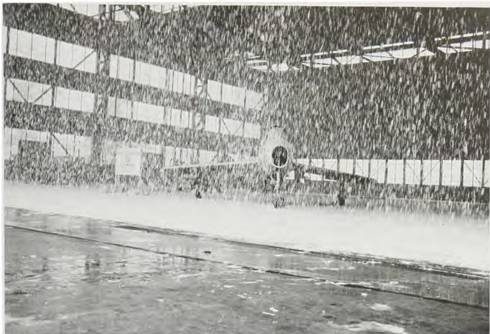
Testing the Foam-Water Fire Protection System constructed at Robins Air Force Base, 26 May 1956. (Robins Air Force Base, Office of History)
