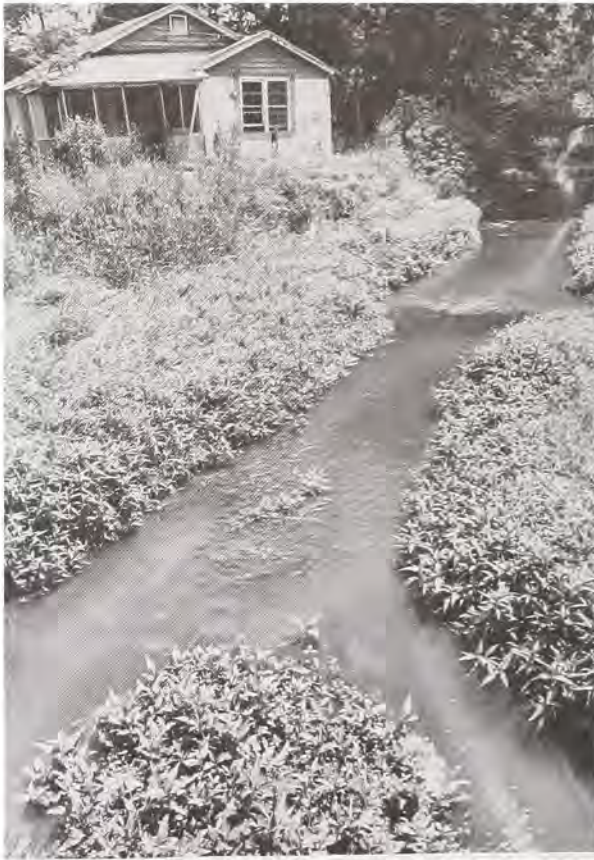
A view along the Oates Creek Flood Control project area in Richmond County, Ga. (Savannah District, Corps of Engineers)
