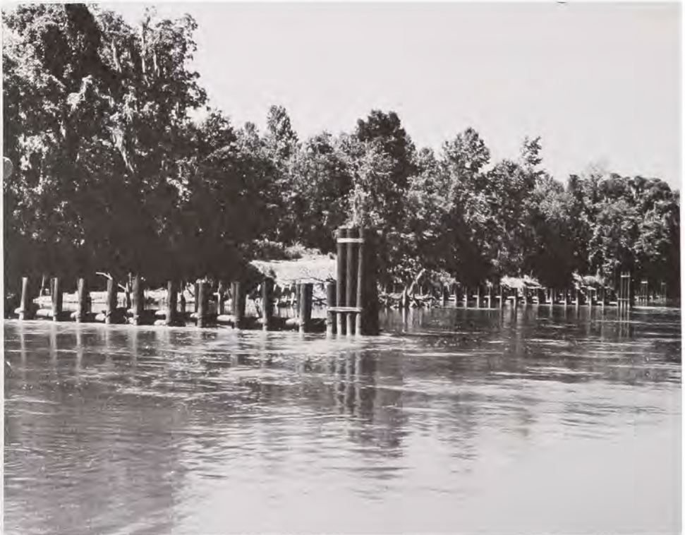
Completed pile dikes on the Savannah River. 18 August 1959. (Savannah District, Corps of Engineers)
