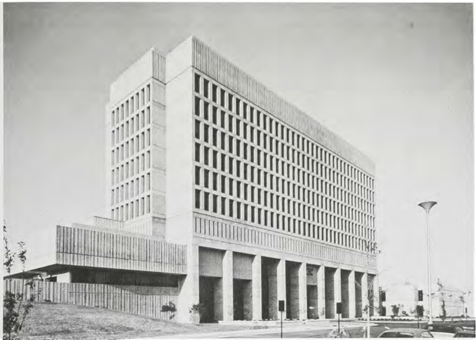
Moncrief Army Hospital at Fort Jackson, one of the new hospitals built by the Corps of Engineers at various Army installations as part of the "new look" on Army posts. (Savannah District, Corps of Engineers)
