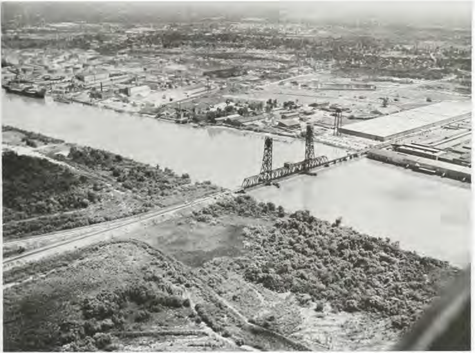
Aerial view of the Seaboard Air Line Railroad Bridge in July 1960 as seen from the South Carolina side of the Savannah River. (Savannah District, Corps of Engineers)
