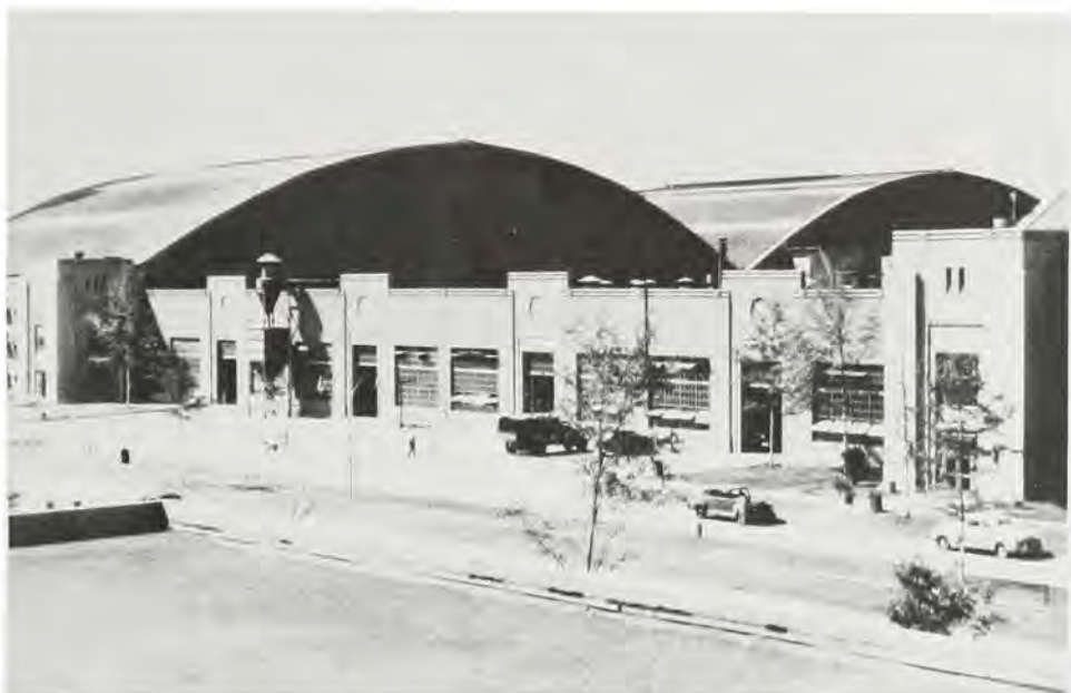
The completed Aircraft Repair Building at Robins Field, (Building 125, Robins Air Force Base) as seen from First Street, 18 June 1943. (Robins Air Force Base, Office of History)
