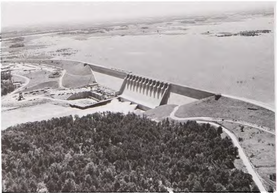
This view from the South Carolina side of the Savannah River shows construction on the Hartwell Dam almost completed. Notice the cofferdam still in place to keep water away from the powerhouse construction area. The reservoir is being impounded behind the dam and is flowing through the sluice gates. 1961. (Savannah District, Corps of Engineers)
