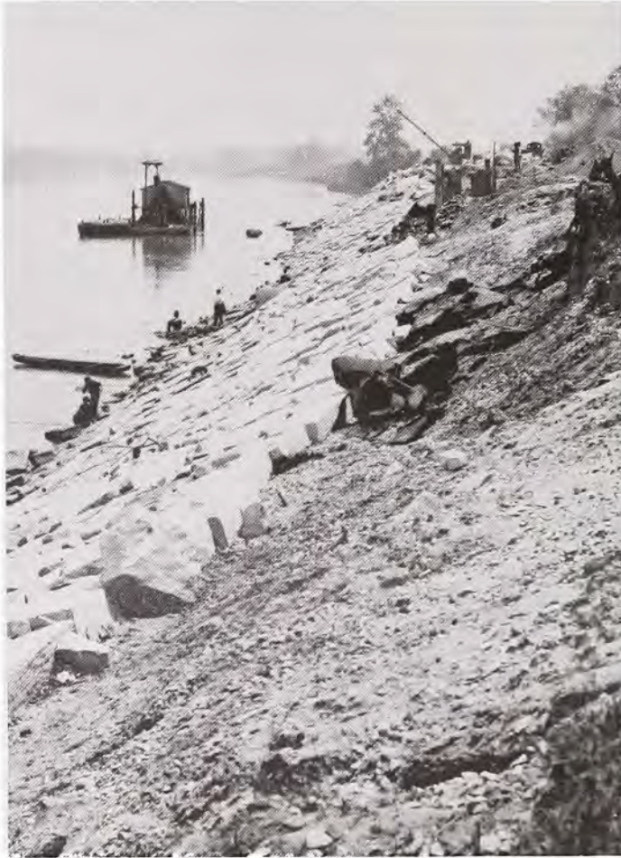
Bank revetment under construction on the Savannah River at Augusta between Center Street and East Boundary Street c. 1913. This project was carried out by contract with the Corps of Engineers. (Savannah District, Corps of Engineers)
