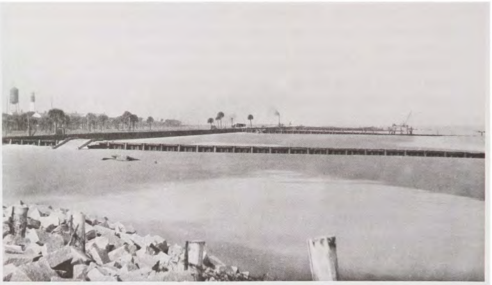
General view of the first bulkhead and groins built in the 1930s to protect Fort Screven from beach erosion. The MacDougald Company under contract with the Corps of Engineers completed the construction in January 1931. The derrick-rig shown is working on groin No. 3. (Savannah District, Corps of Engineers)
