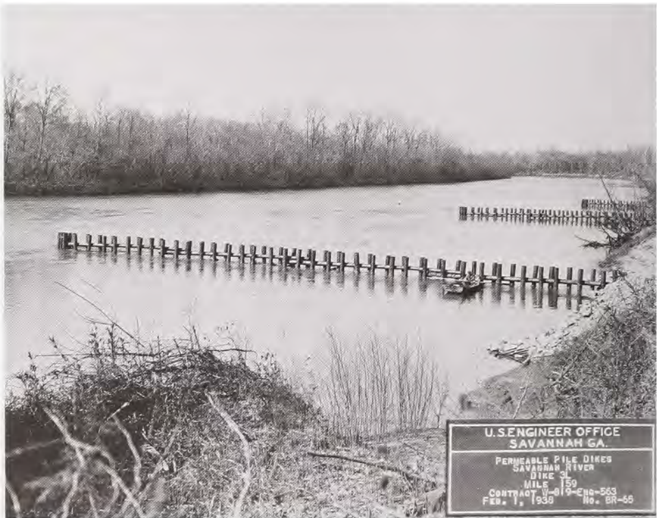
A permeable pile dike on the Savannah River below Augusta, one of the types of channel contraction works used by the Corps of Engineers in the Savannah District as of 1 February 1938. (Savannah District, Corps of Engineers)
