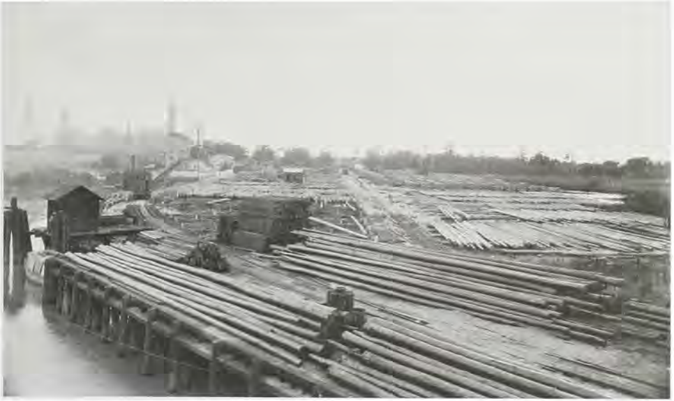
The wharf and yard of the Savannah Creosoting Company in the upper reaches of Savannah Harbor in 1924. A large part of the yard was leased to the Mead and Manucy Company whose piles are shown in the picture. The Savannah Sugar Refining Corporation is seen in the distance at the left. (Savannah District, Corps of Engineers)
