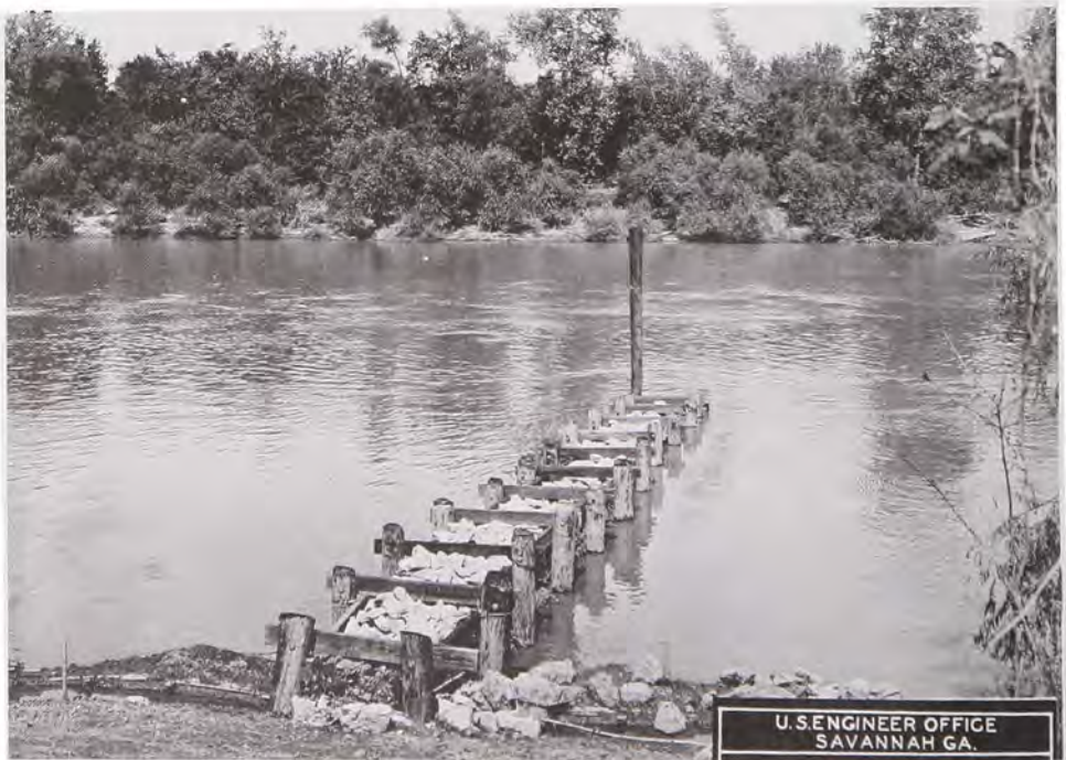
A completed pile dike used for channel contraction Augusta. Note the inner core of brush fascines topped by a layer of rip rap stone, 21 September 1935. (Savannah District, Corps of Engineers)
