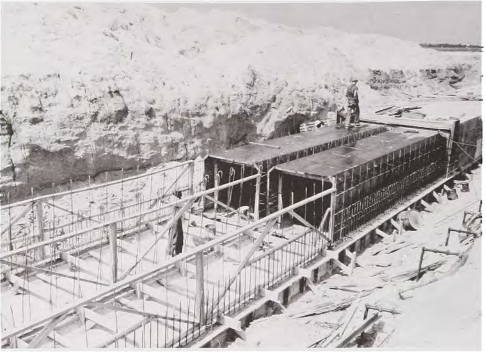
Construction of double 6ft. by 6ft. culverts as part of the extension and enlargement of runways at Robins Air Force Base to accommodate the SAC wing, 18 July 1958. (Savannah District, Corps of Engineers)
