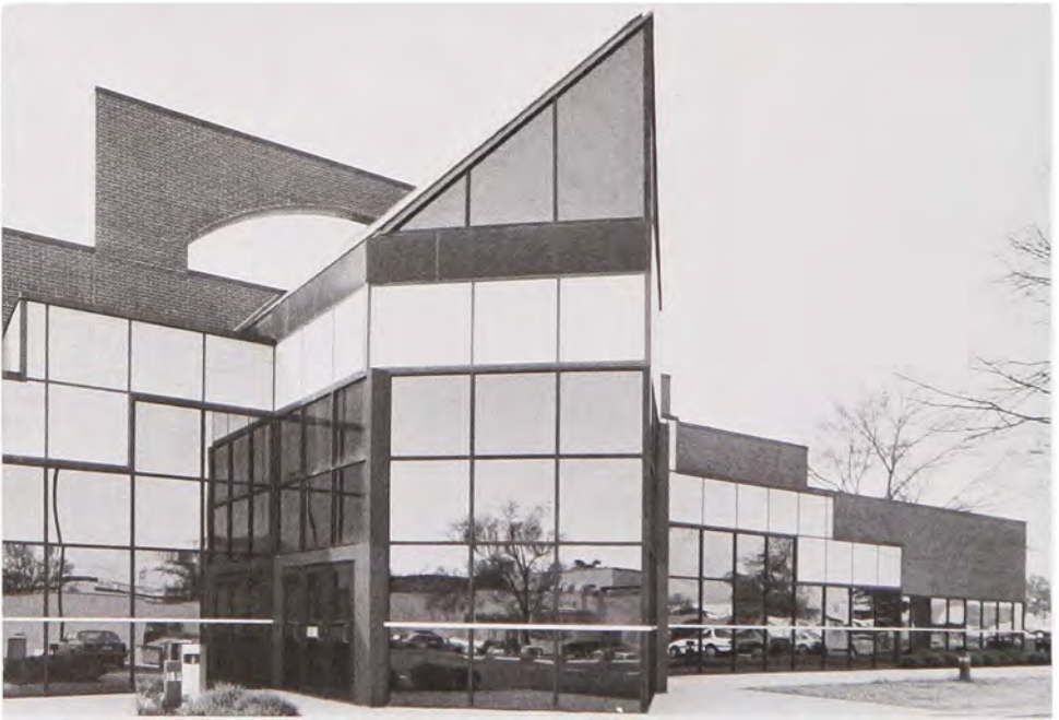
Dining facility for Robins Air Force Base personnel completed by the Savannah District in 1989. (Savannah District, Corps of Engineers)
