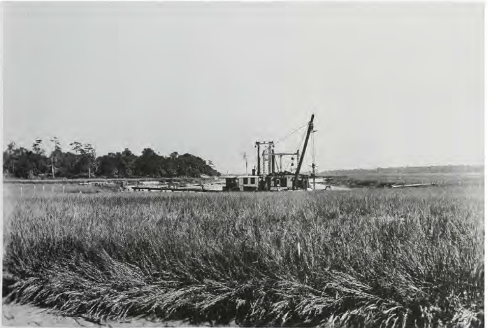
Dredging a land cut on the Intracoastal Waterway as part of the project to deepen the channel to 12 feet. 12 October 1940. (Savannah District, Corps of Engineers)
