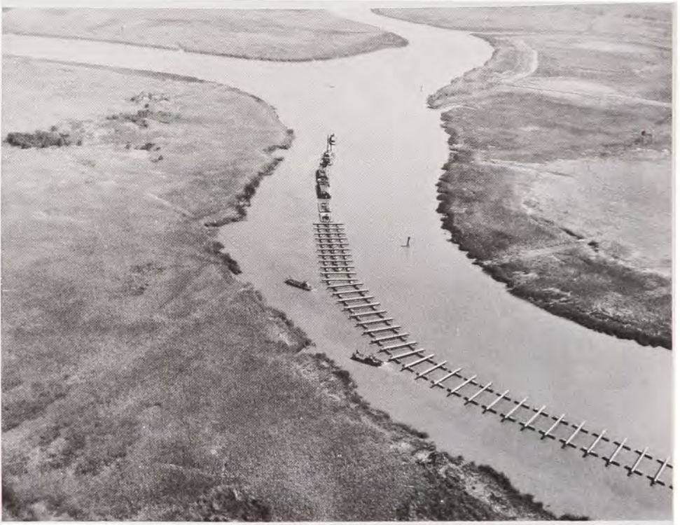
Commercial tow of sections of a pipeline and dredge on the Intracoastal Waterway near Wilmington Island, Georgia, 17 March 1966. (Savannah District, Corps of Engineers)
