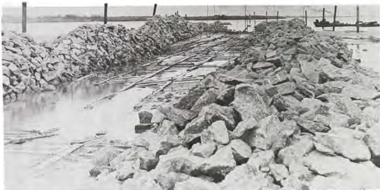
Placement of lumber mattresses bordered on each side with rip rap stone. 8 February 1940
