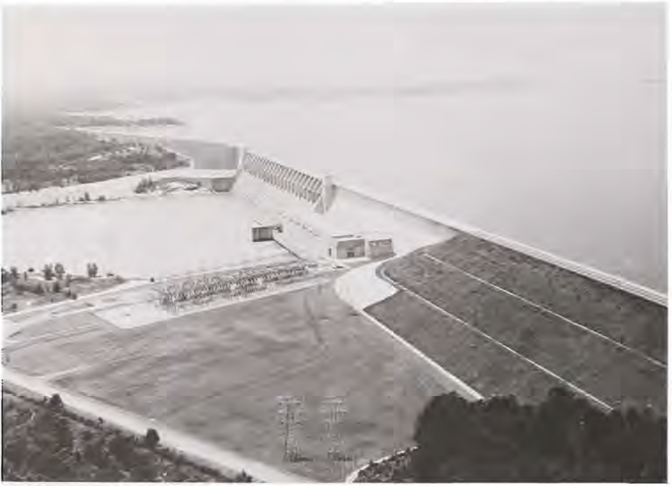
Clark Hill Dam after construction was completed. This view shows the completed dam, the earthen embankments on either side of the concrete dam, the powerhouse, the switchyard, and the impounded lake. 1965. (Savannah District, Corps of Engineers)
