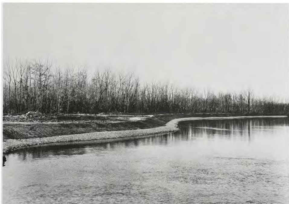
Completed bank protection at Canoe Cut on the Savannah River below Augusta. 5 December 1940. (Savannah District, Corps of Engineers)
