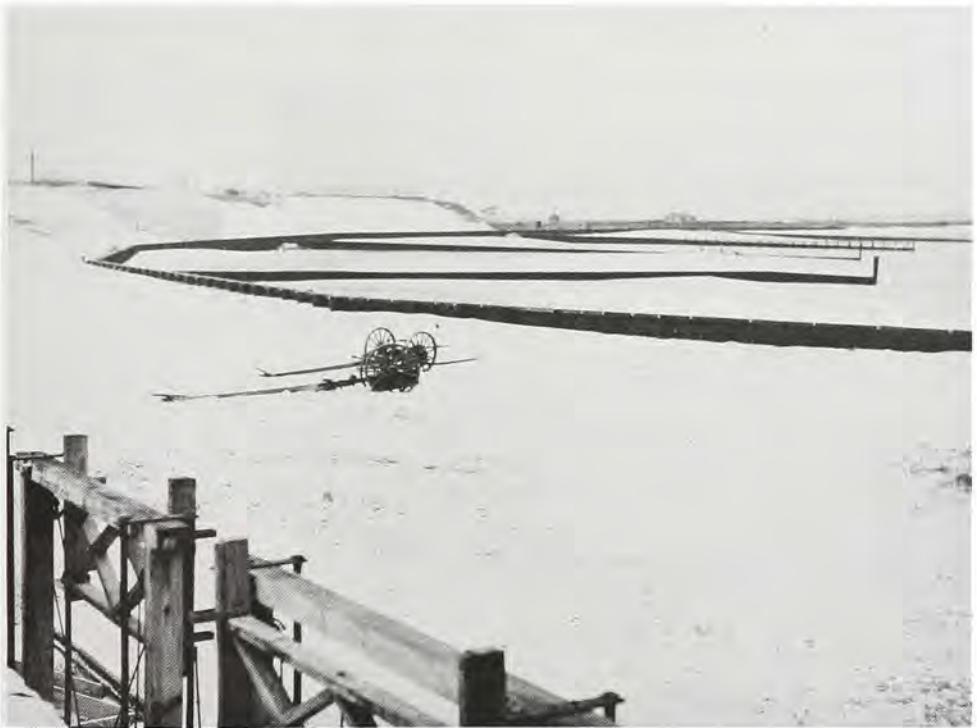
Wooden bulkhead and groins built by the W. P. A. under Corps of Engineers supervision to further protect Fort Screven from beach erosion. The photo was taken from the target butts at the Fort on the north end of Tybee Island on 22 June 1937. (Savannah District, Corps of Engineers)
