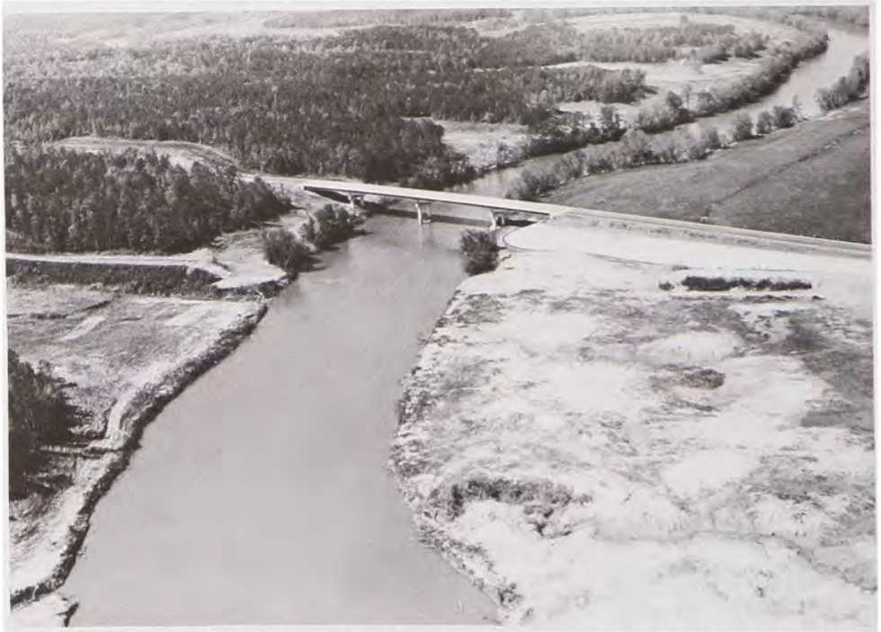
This Chattahoochee River bridge was named the "Prize Bridge" in the Medium Span Low Clearance category in the 1974 competition sponsored by the American Institute of Steel Construction, Inc. The bridge was built in connection with the West Point Dam project which required the relocation of Georgia Highway 219. March 1974. (Savannah District, Corps of Engineers)
