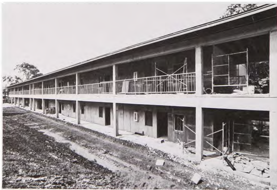
New barracks under construction by the Savannah District for Army Rangers at Camp Merrill. (Savannah District, Corps of Engineers)
