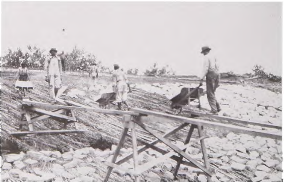
Workers placing stone on brush mattresses as part of the shore protection works on the Savannah River below Augusta in July 1923. (Savannah District, Corps of Engineers)
