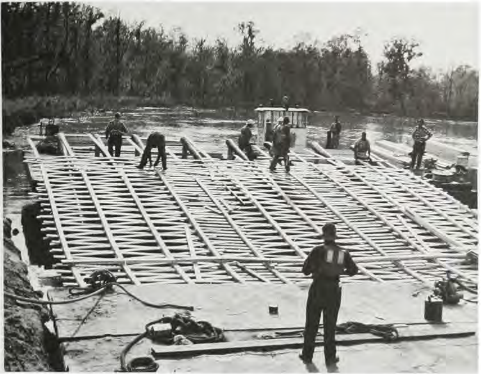
Contractors weaving lumber mattresses for shore protection works on the Savannah River below Augusta. 16 December 1959. (Savannah District, Corps of Engineers)
