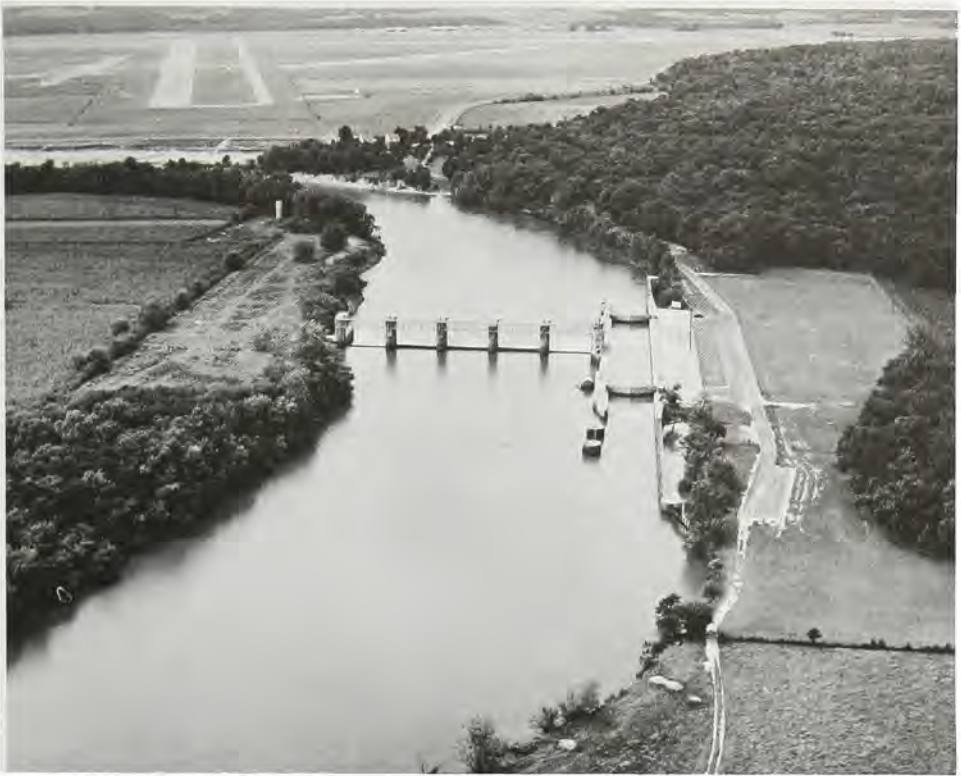
New Savannah Bluff Lock and Dam on the Savannah River looking downstream. The structure was completed in 1937. (Savannah District, Corps of Engineers)
