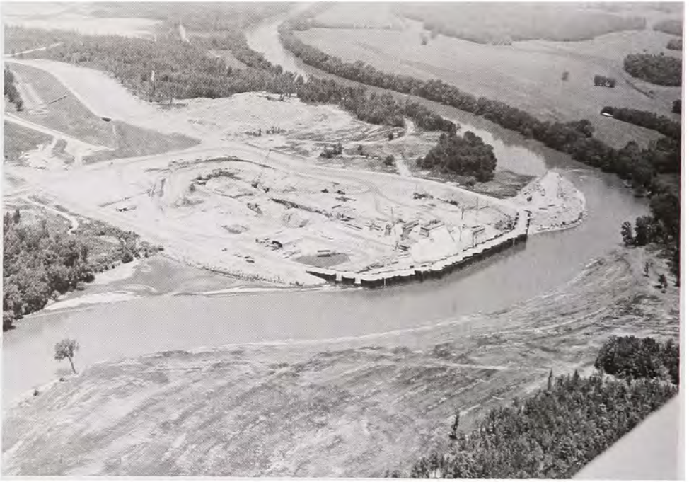
Aerial view showing construction underway on the West Point Dam on the Alabama side of the Chattahoochee River. Note the natural river channel, the diversion channel, and the cofferdam built around the construction area. (Savannah District, Corps of Engineers)
