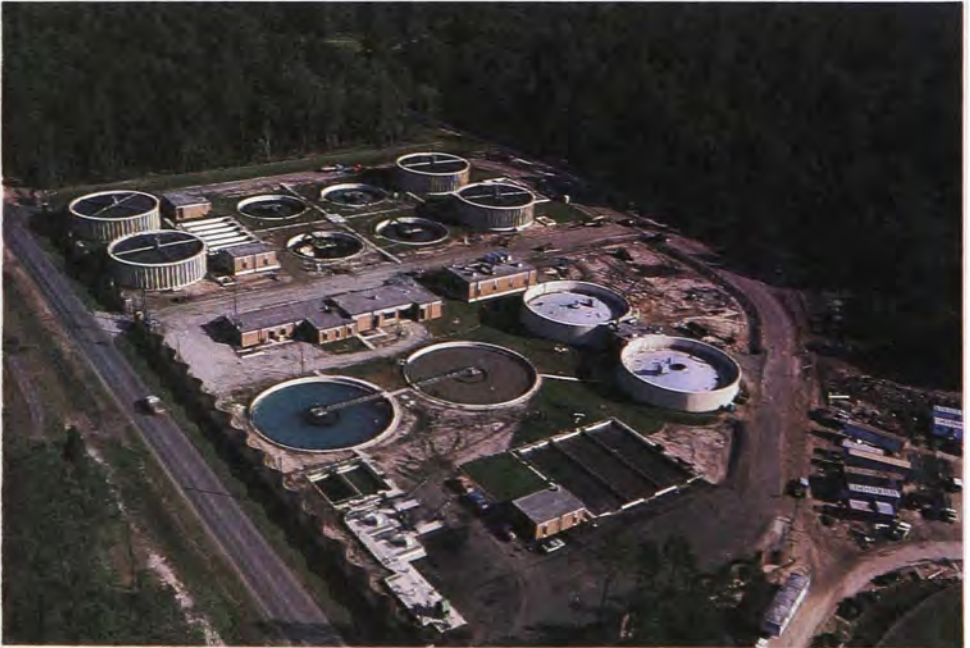
The Fort Stewart sewage treatment plant dedicated in November 1985. (Savannah District, Corps of Engineers)
