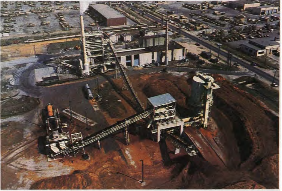
The wood burning plant built at Fort Stewart in 1984, designed to burn waste wood to supply energy needs throughout the post. (Savannah District, Corps of Engineers)
