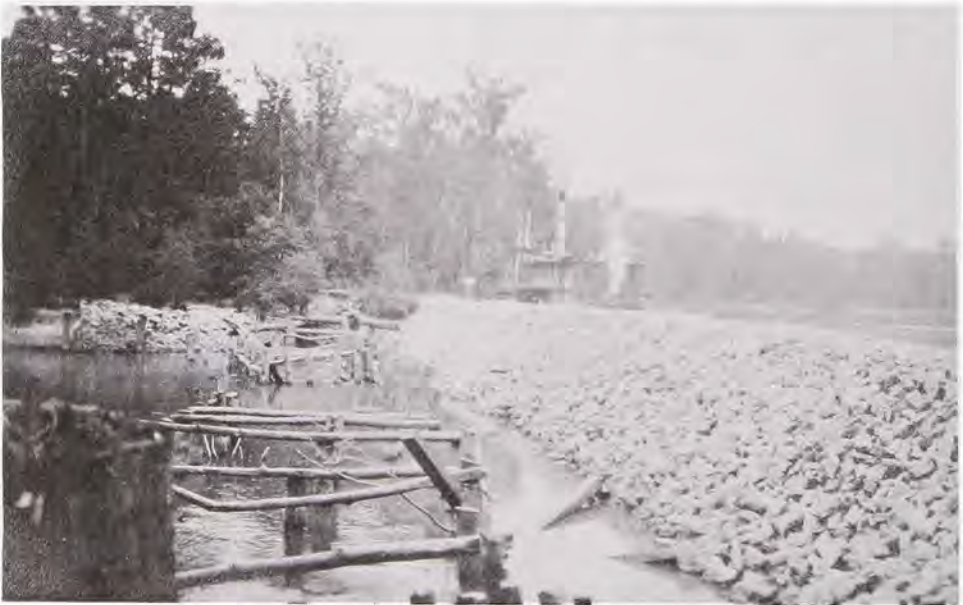
The earlier closing dam at Jacks Suck on the Altamaha River was replaced by a rock closing dam completed by the Corps of Engineers in 1916. Note the remains of the original closing dam. The main channel of the Altamaha River is seen to the right looking upstream, and Jacks Suck is to the left of this photograph taken 28 April 1916. A snagboat can be seen beyond the closing dam. (Savannah District, Corps of Engineers)
