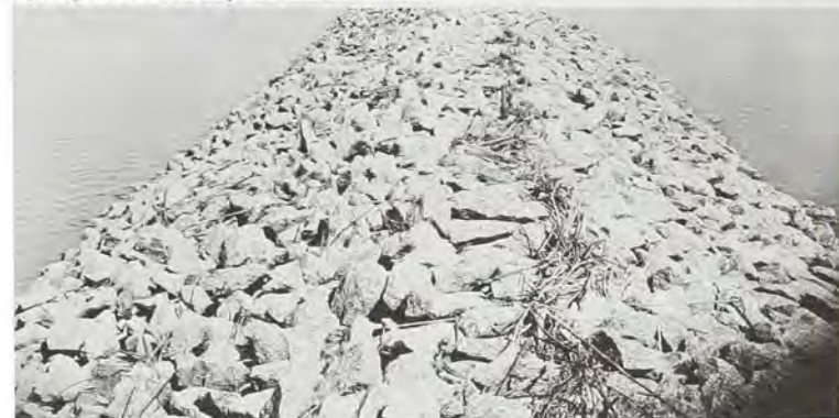
Completed Fig Island Training Wall in Savannah Harbor. 11 October 1940
