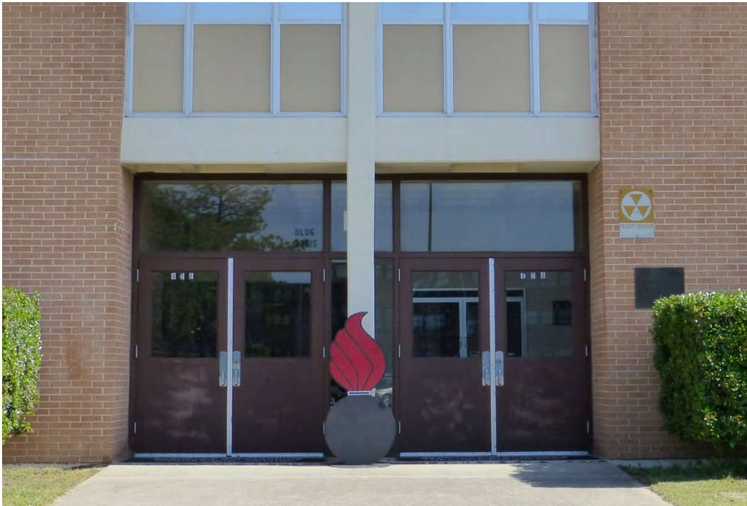
Figure 57. Two sets of metal doors with pane and transoms above separated by exposed concrete structure, Building 29815, Hazen Hall (ERDC-CERL, 2015).
