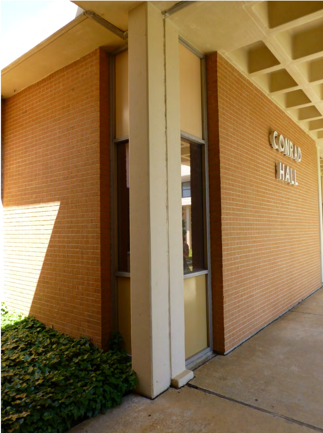
Figure 64. Exposed concrete structural element, located at the corner of the building and framing the corner window system, Building 29807, Museum (Conrad Hall) (ERDC-CERL, 2015).
