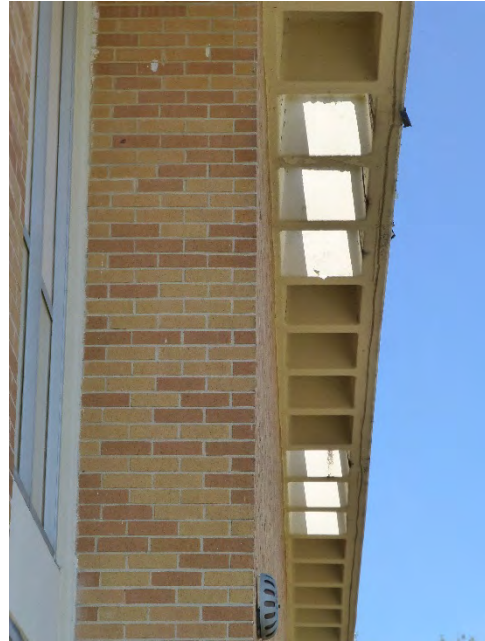
Perforated concrete waffle overhang.
