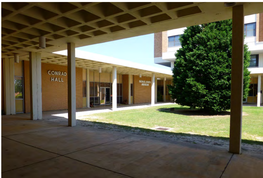
Figure 246. Looking at the main entry into Building 29807, Conrad Hall on the east elevation (ERDC-CERL, 2015).
