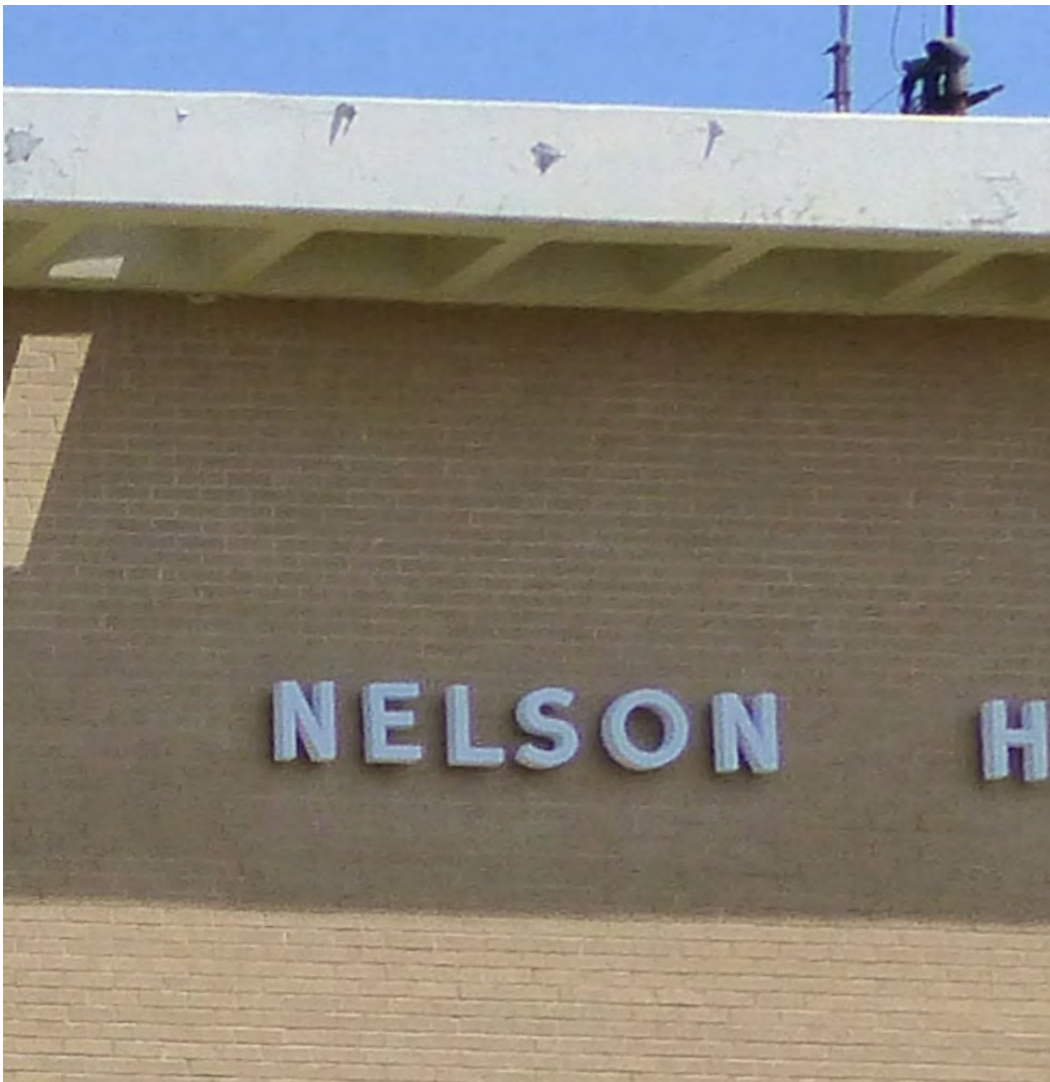
Figure 80. Example of the uniform lettering, Building 29801, Nelson Hall (ERDC-CERL, 2015).
