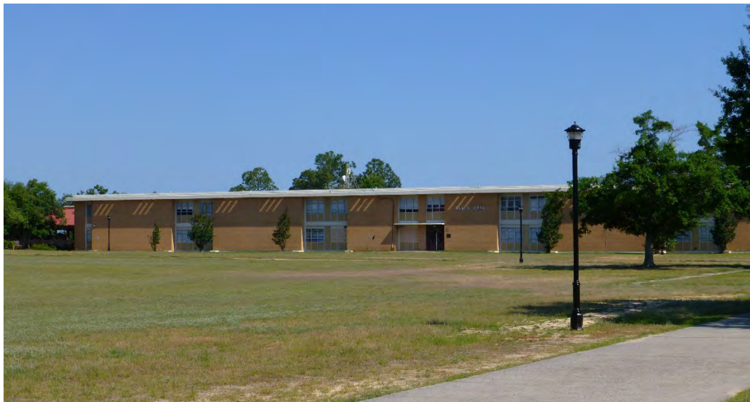
Figure 343. South elevation of Building 29813, Allen Hall (ERDC-CERL, 2015).
