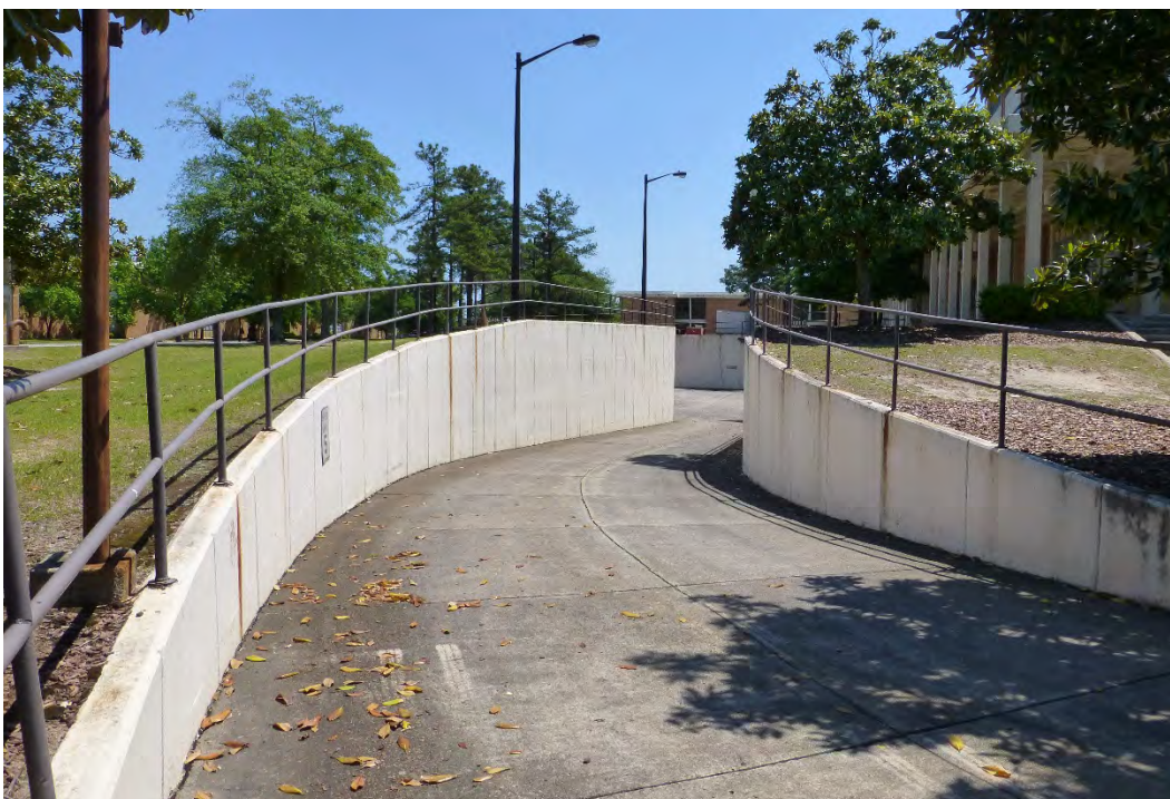
Figure 87. Curved poured-in-place concrete retaining wall system topped with metal pipe handrails, Building 29808, Signal Towers (ERDC-CERL, 2015).
