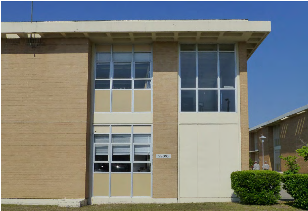
Figure 50. Example of three window systems: bright-aluminum framed awning windows with insulated panels, bright-aluminum framed fixed-pane windows, and concrete panel inserts, Building 29816, Fisher Hall (ERDC-CERL, 2015).
