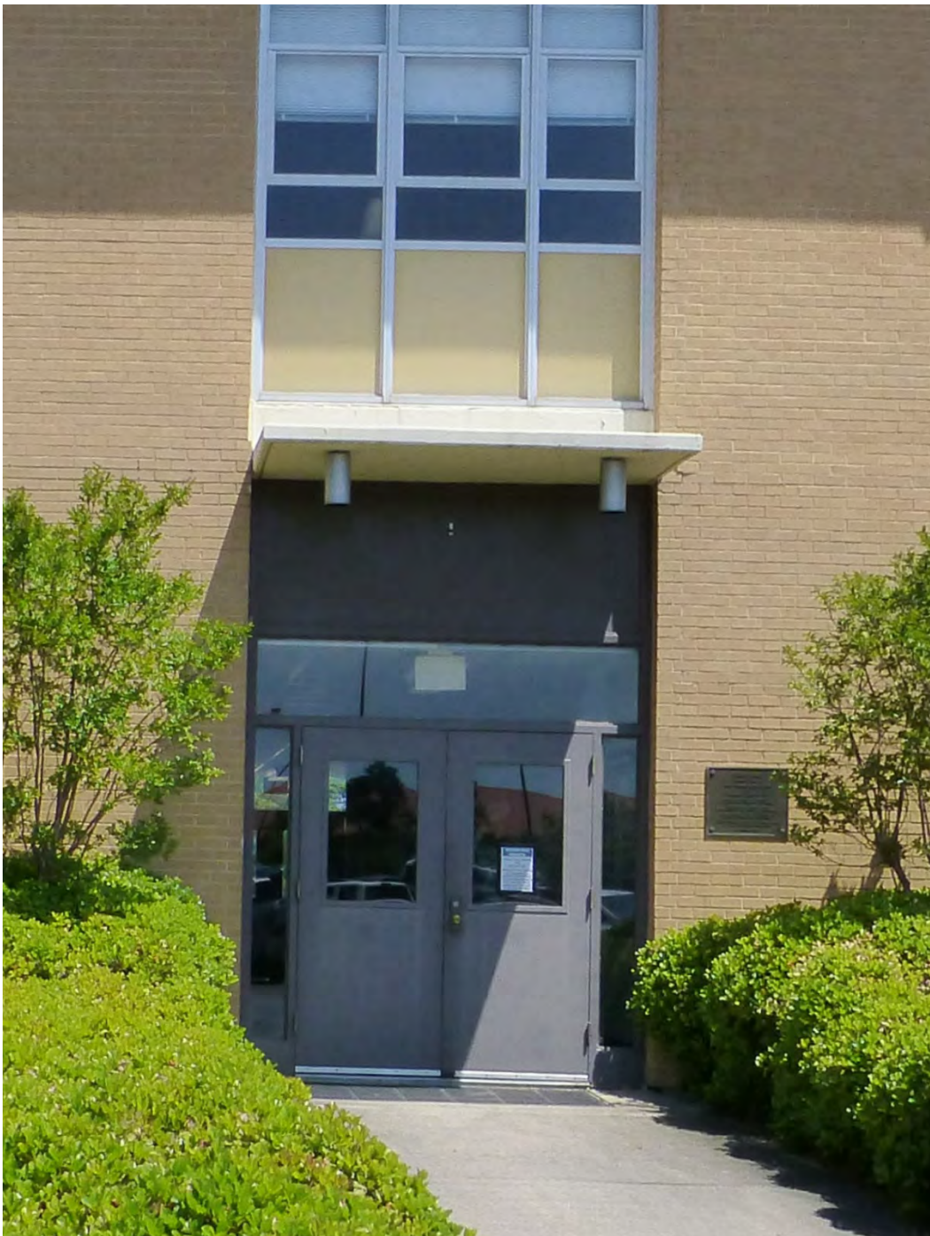
Figure 67. Flat concrete canopy above a set of metal entry doors on Building 29801, Nelson Hall (ERDC-CERL, 2015).
