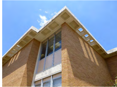
Overhanging eaves (waffle construction) with perforated waffles casting a "light pattern" on the second floor of the brick walls.
