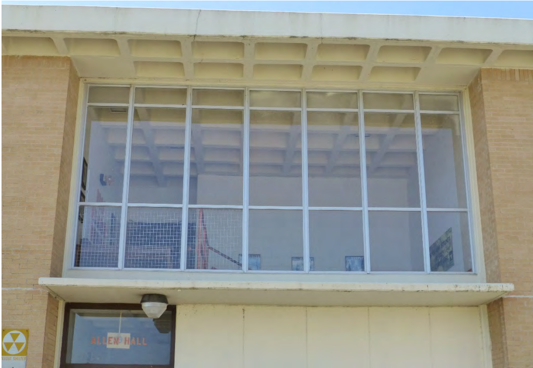
Figure 49. Bright-aluminum fixed-pane window system above entry bay, Building 29813, Allen Hall (ERDC-CERL, 2015).
