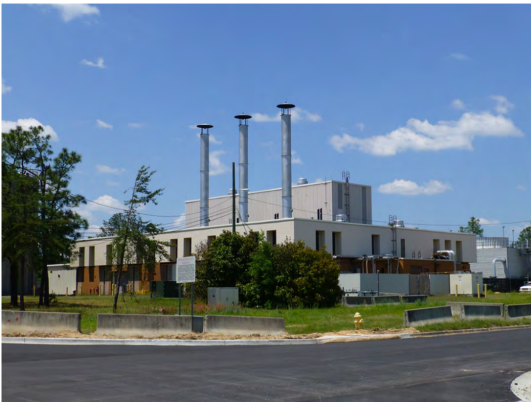
Figure 460. Building 25910 Heating/AC Plant was constructed in 1966 and designed by Sewell and Associates (ERDC-CERL 2015).
