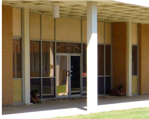
Bright-aluminum and plate-glass doors and sidelights with insulated panels.
