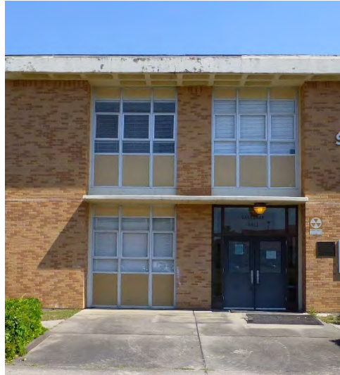
Main entry on the south elevation with groups of three windows, flat concrete canopy, and metal entry doors.
