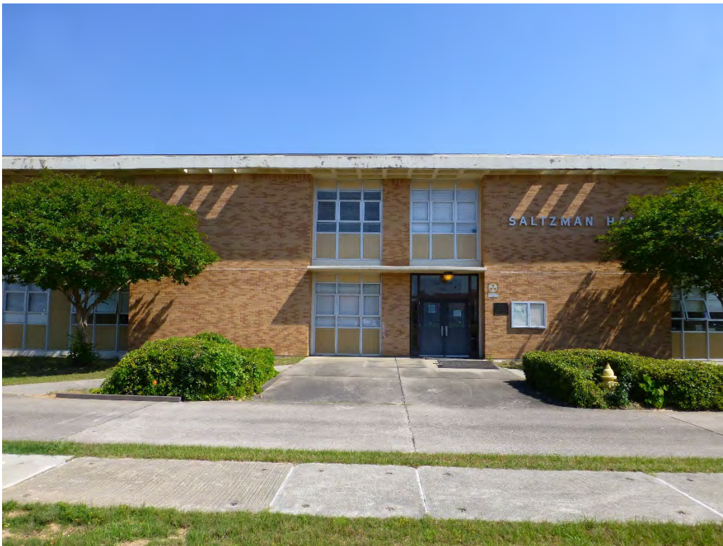
Figure 314. Main entry bay on the south elevation of Building 29811, Saltzman Hall (ERDC-CERL, 2015).
