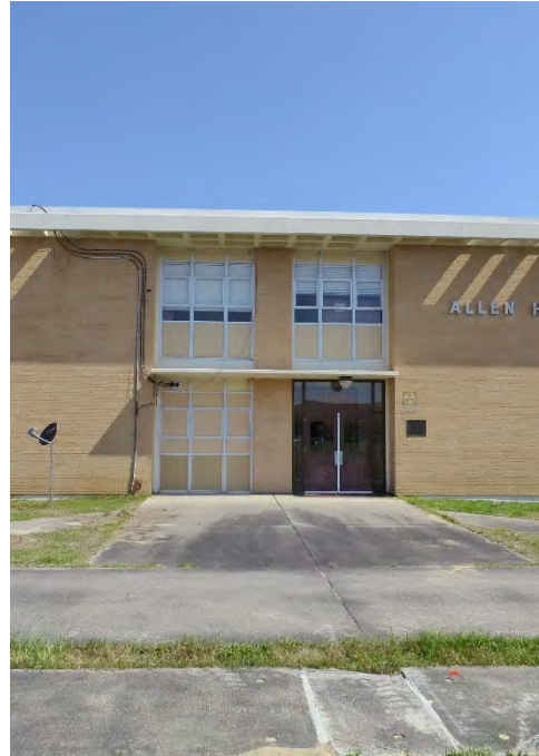
Main entry on the south elevation with groups of three windows, flat concrete canopy, and metal entry doors.
