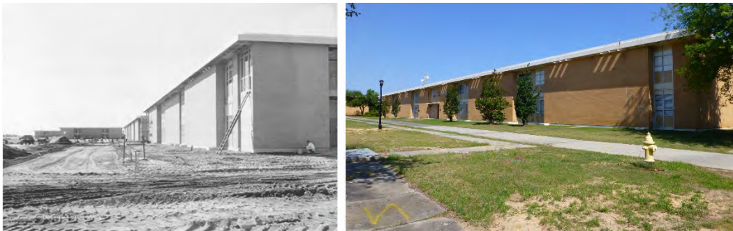
Figure 362. Southeast oblique – comparison of the original design and materials for Building 29811 and construction in 1966 [left] to the current condition of the south elevation of Building 29813, Allen Hall [right] (ERDC-CERL, 2015).
