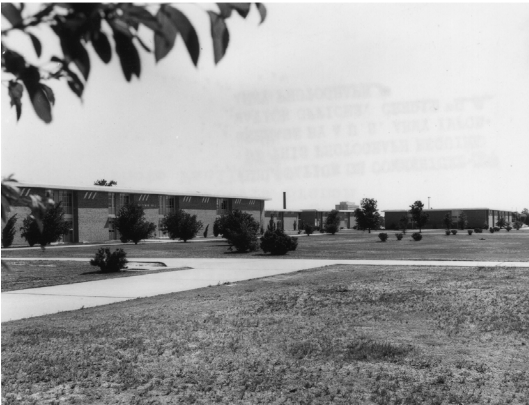
Figure 19. General view of the campus, showing landscaping and looking northeast towards Saltzman Hall (Building 29811) on the left, Allen Hall (Building 29813) middle, and Allison Hall (Building 29817) right, April 1978 (National Archives at College Park, MD).
