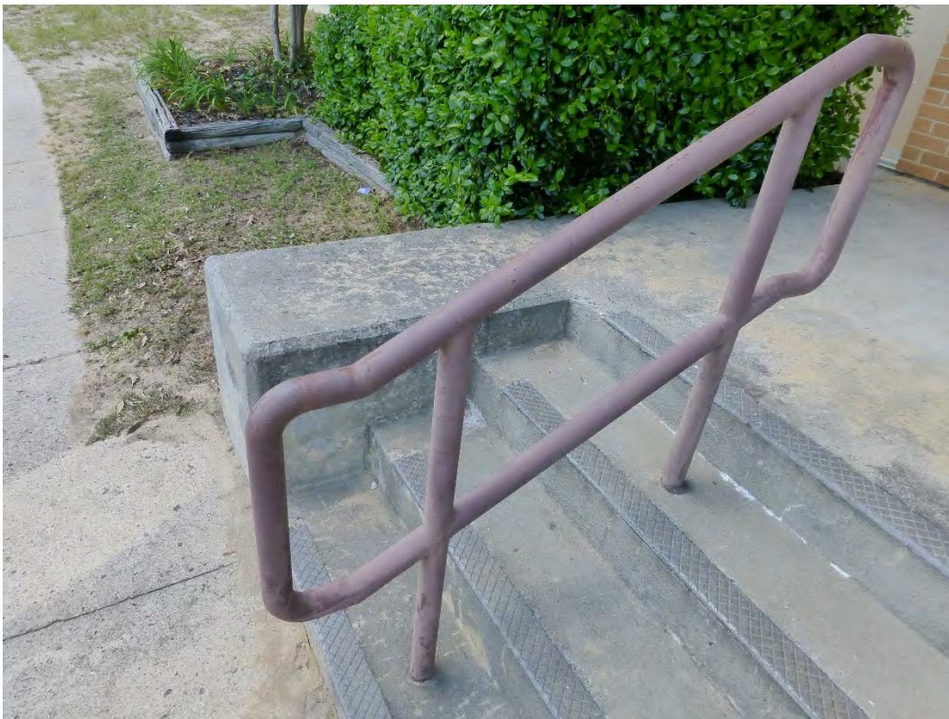
Figure 86. Example of the metal pipe handrail located near the entries for Building 25810, Brant Hall (ERDC-CERL, 2015).
