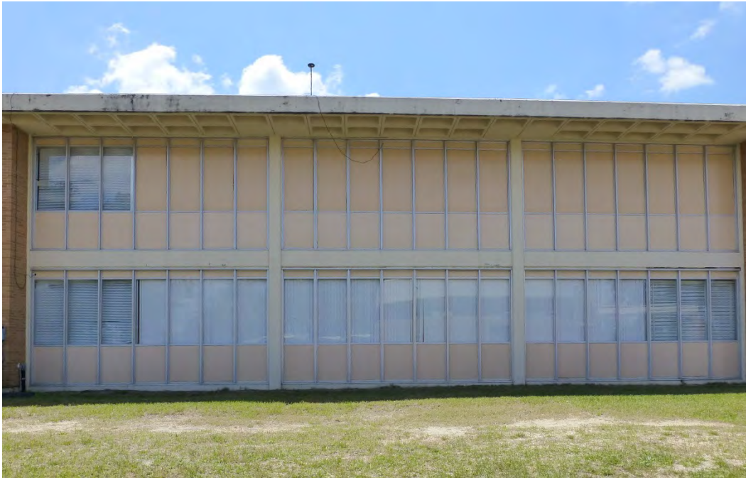
Figure 47. Modified window pattern with the removal of the original awning window and the addition of the newer insulated panel, Building 25810, Brant Hall (ERDC-CERL, 2015).
