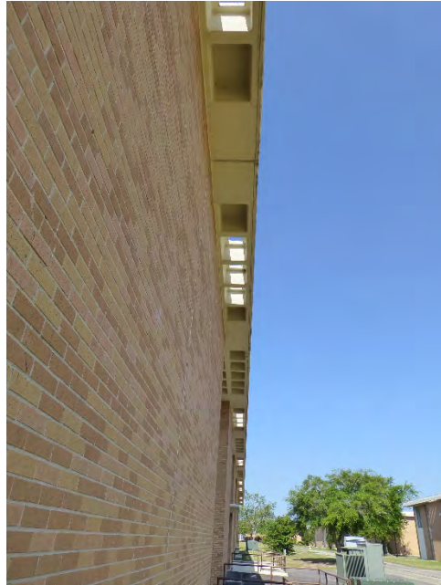
Perforated concrete waffle overhang.
