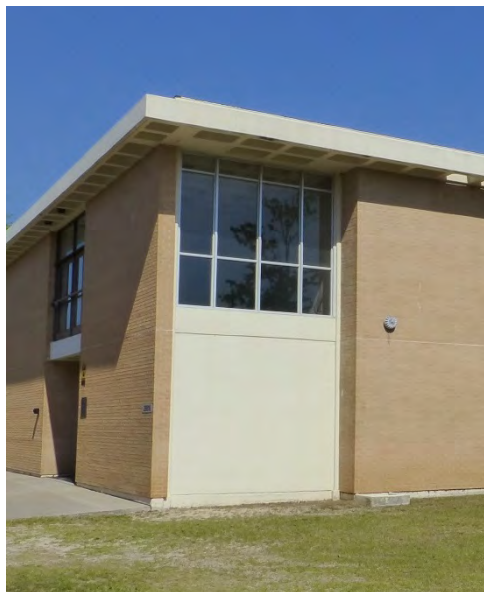
Window bay with concrete panels and bright-aluminum three-pane fixed windows.
