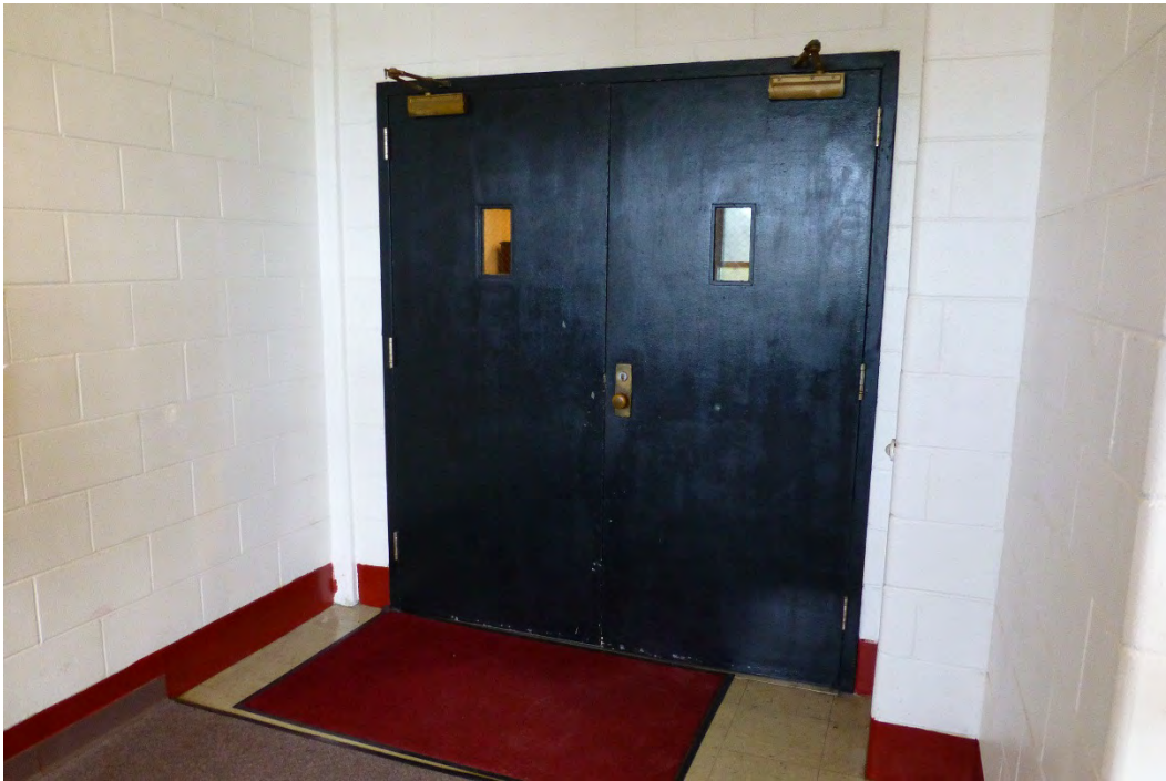
Figure 151. Typical metal security doors with one small pane, leading from the stairwell into the central hall (ERDC-CERL, 2015).
