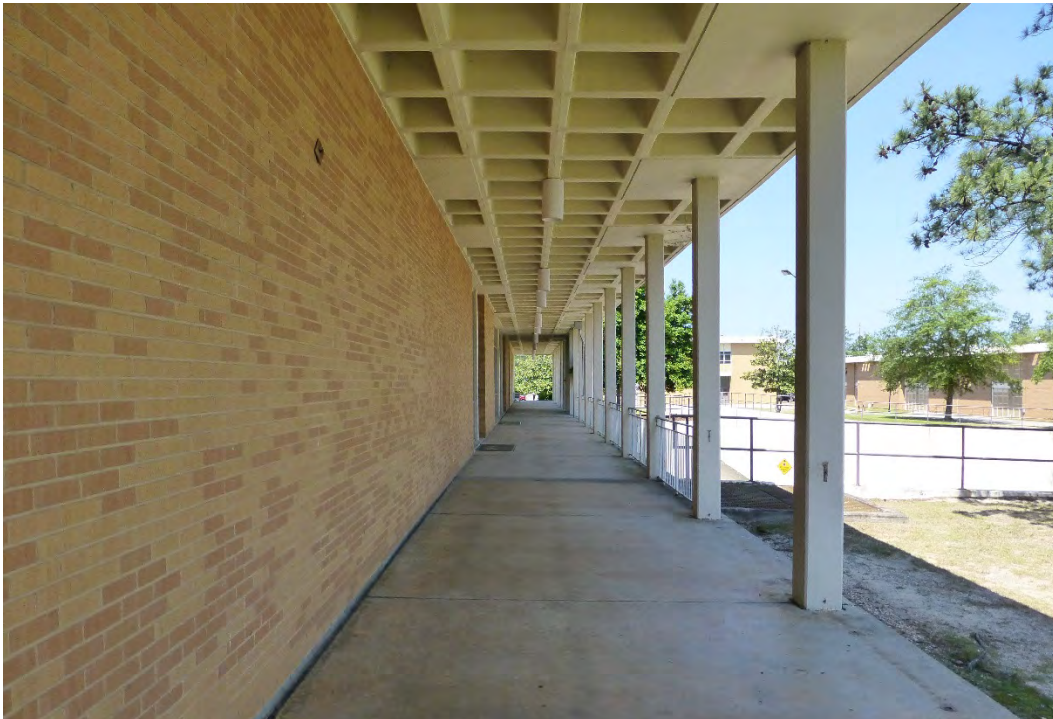
Figure 261. First-floor concrete waffle canopy structure that surrounds Building 29808, Signal Towers, and connects it to Buildings 29805 and 29807 (ERDC-CERL, 2015).
