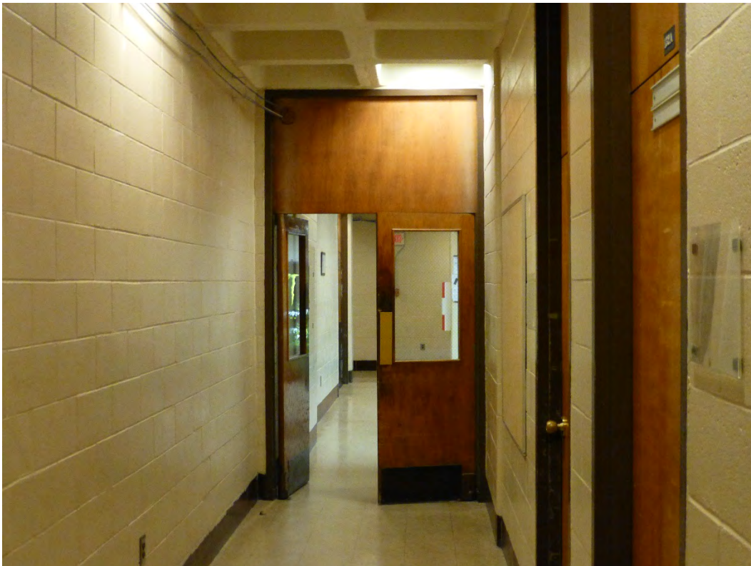
Figure 152. Typical interior wood doors with large pane and wood transom, located in the hallway [left] and typical wood door with wood transom leading into room off hallway [right] (ERDC-CERL, 2015).
