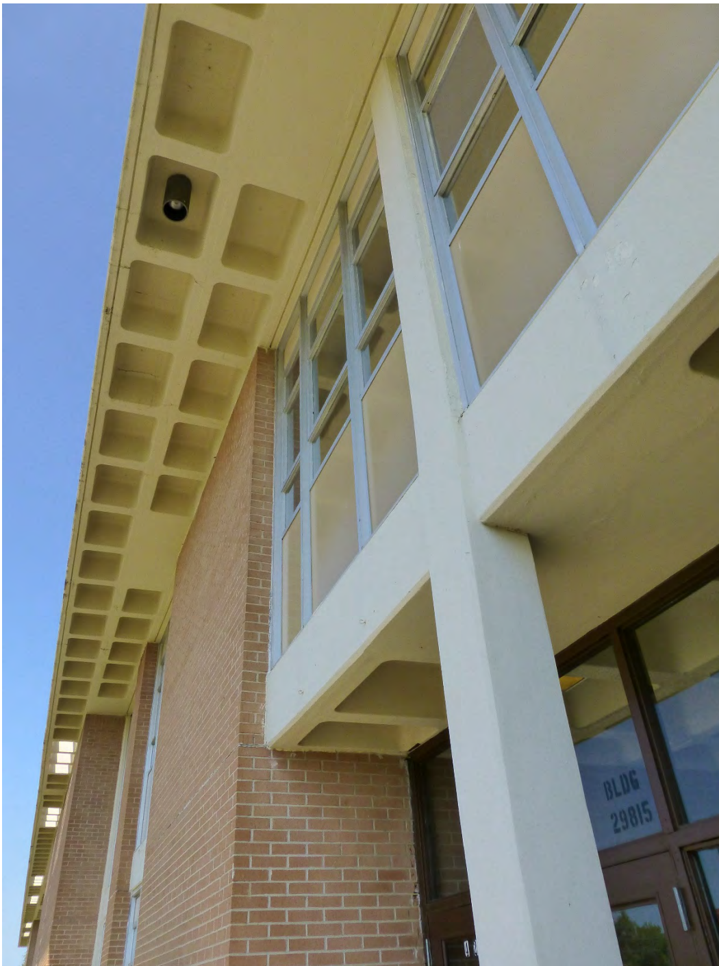
Figure 63. Close-up of the exposed concrete structural system framing the doors and window bays, Building 29815, Hazen Hall (ERDC-CERL, 2015).
