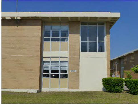
Window bays consisting of bright-aluminum three-pane awning-style windows sandwiched between insulated panels and bright-aluminum three-pane fixed windows above concrete panels.
