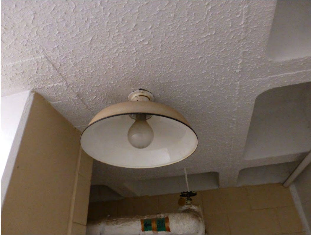
Figure 145. Typical original ceiling-mounted pendant light fixture (ERDC-CERL, 2015).
