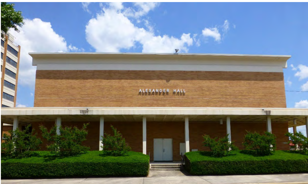
Figure 27. Rectangular massing, Building 29805, Alexander/Olmsted Halls (ERDC-CERL, 2015).
