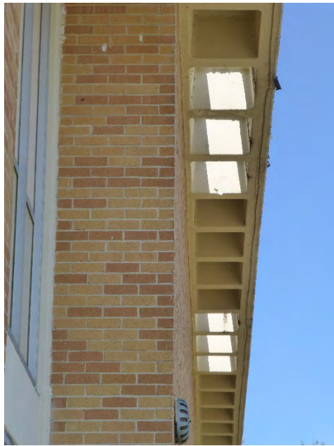
Perforated concrete waffle overhang.
