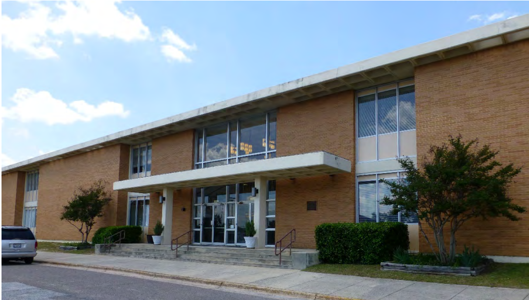
Figure 175. Building 25810, Brant Hall, south [front] elevation (ERDC-CERL, 2015).
