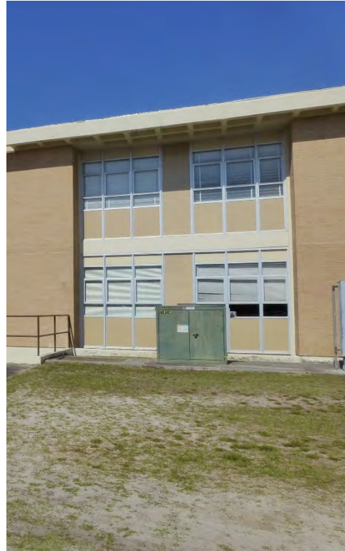
Large window bay with six windows separated by insulated panel.
