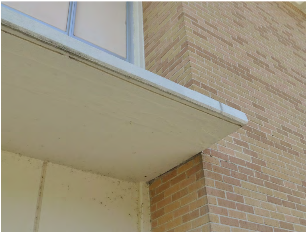
Figure 70. Close-up of the concrete canopy detail, Building 29817, Allison Hall (ERDC-CERL, 2015).
