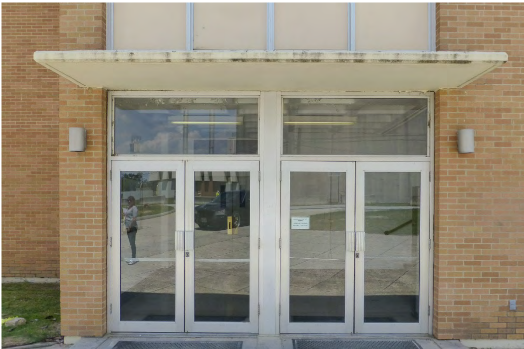
Figure 71. Wall-mounted light fixtures flanking either side of an entry, Building 25810, Brant Hall (ERDC-CERL, 2015).
