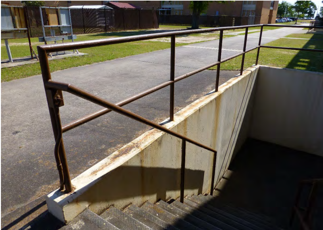
Figure 85. Example of typical poured-in-place concrete retaining walls and metal handrails framing the exterior basement access points, Building 29813, Allen Hall (ERDC-CERL, 2015).
