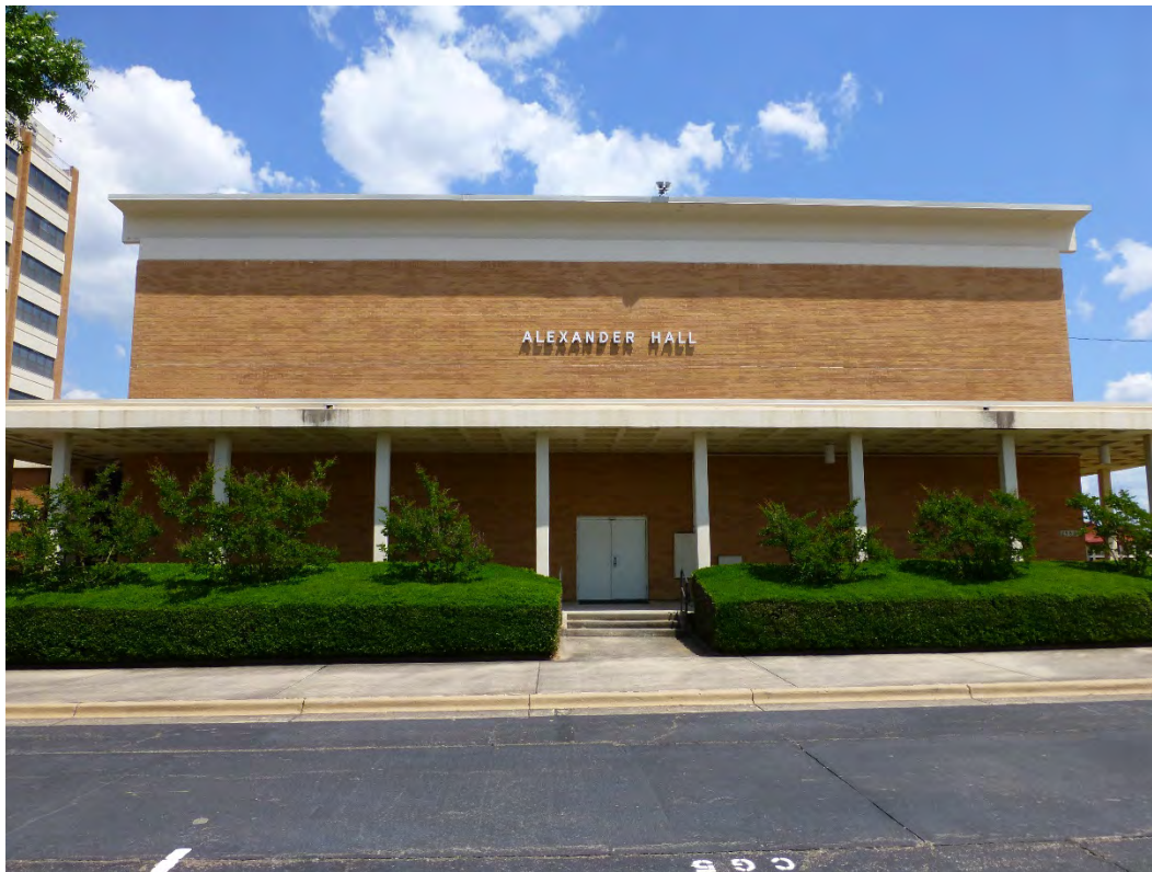
Figure 225. West elevation of Building 29805, Alexander/Olmstead Halls (ERDC-CERL, 2015).
