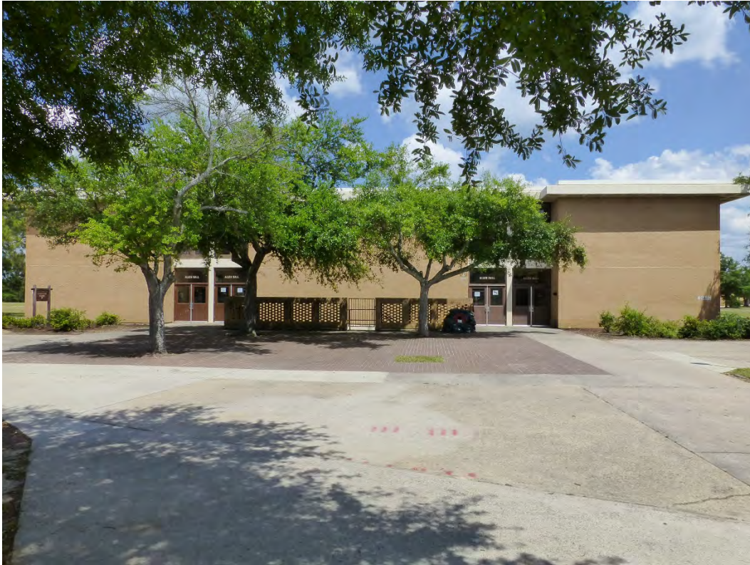
Figure 346. West elevation of Building 29813, Allen Hall (ERDC-CERL, 2015).
