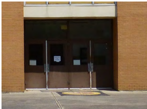
Recessed metal doors with a pane and a fixed transom above.
