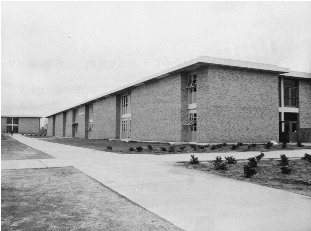
Figure 318. Building 29811, Saltzman Hall, March 1967 (National Archives at College Park, MD).
