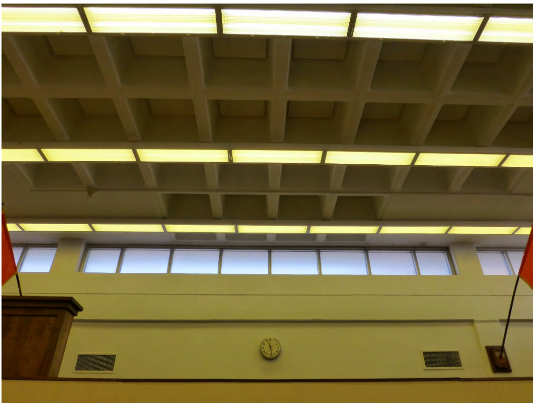
Figure 52. Bright-aluminum fixed-pane clerestory windows, Building 29807, Museum/Conrad Hall (ERDC-CERL, 2015).
