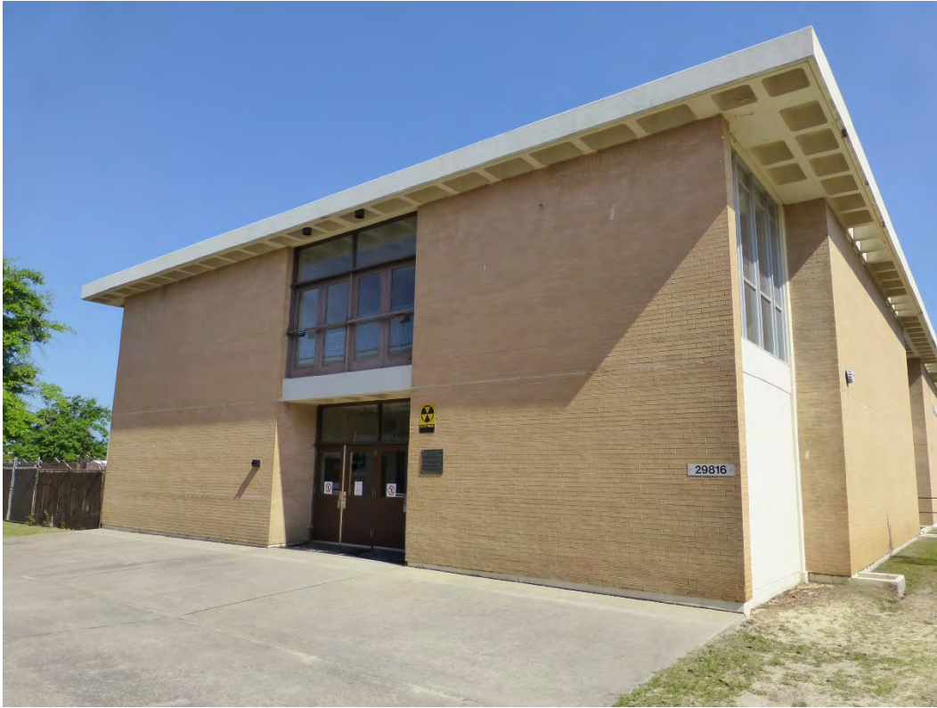
Figure 388. South elevation of Building 29816, Fisher Hall (ERDC-CERL, 2015).
