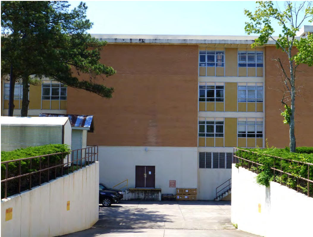
Figure 88. Poured-in-place concrete retaining walls framing driveway to walkout basement for Building 29810, Burkhardt Hall (ERDC-CERL, 2015).
