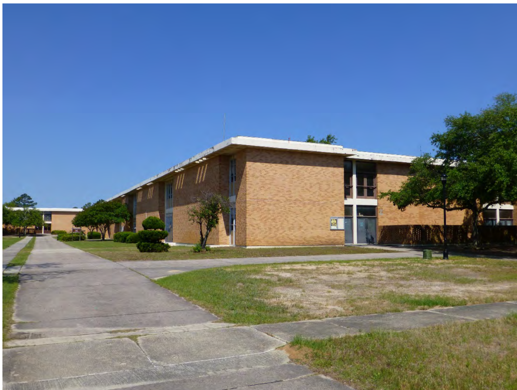
Figure 312. Southeast corner of Building 29811, Saltzman Hall, (ERDC-CERL, 2015).
