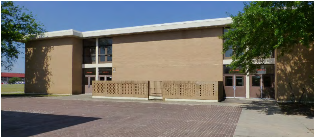
Figure 90. Example of the decorative perforated brick wall, Building 29813, Allen Hall (ERDC-CERL, 2015).
