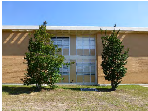
Window pattern; window bay with six bright-aluminum awning-style windows sandwiched by insulated panels and separated by an insulated panel. Exposed concrete structural system divides the first and second-floor window groups.
