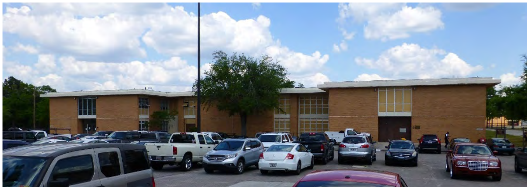
Figure 216. West elevation of Building 29803 [left] and Building 29802 [right] (ERDC-CERL, 2015).
