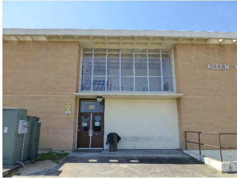
Entry bay on north elevation with concrete panels, metal doors, flat concrete canopy, and fixed windows framed with bright-aluminum sashes.
