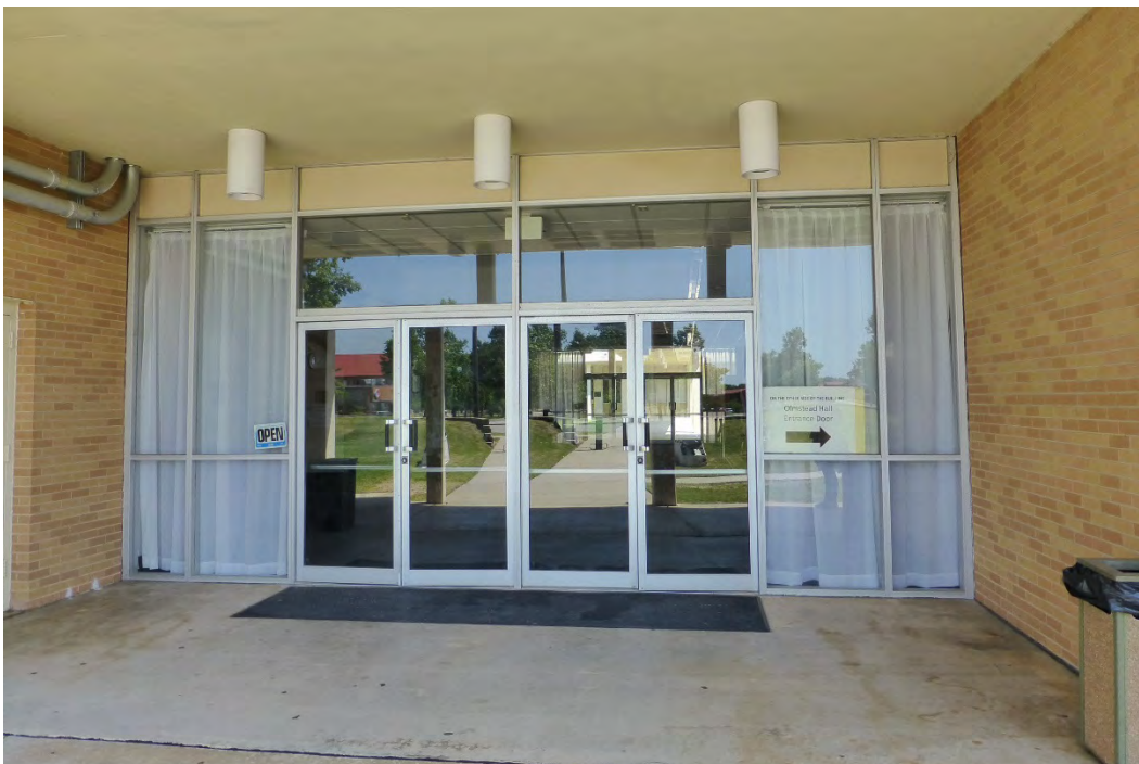
Figure 74. Ceiling-mounted light fixtures placed under the recessed ceiling of the entry into Building 29805, Alexander/Olmsted Halls (ERDC-CERL, 2015).
