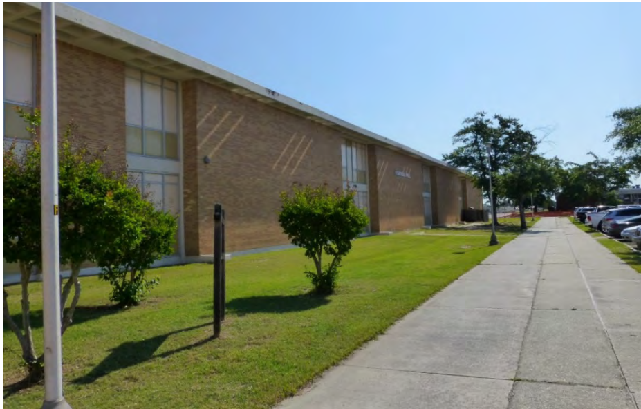
Figure 117. Looking east down the sidewalk running in front of Building 29819, Stansell Hall (ERDC-CERL, 2015).
