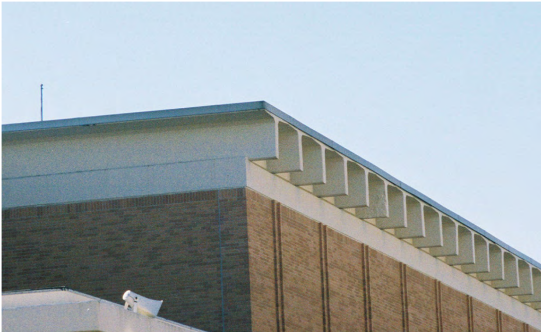
Figure 40. Building 29805, Alexander/Olmsted Halls, constructed with precast concrete T-beams (ERDC-CERL, 2015).
