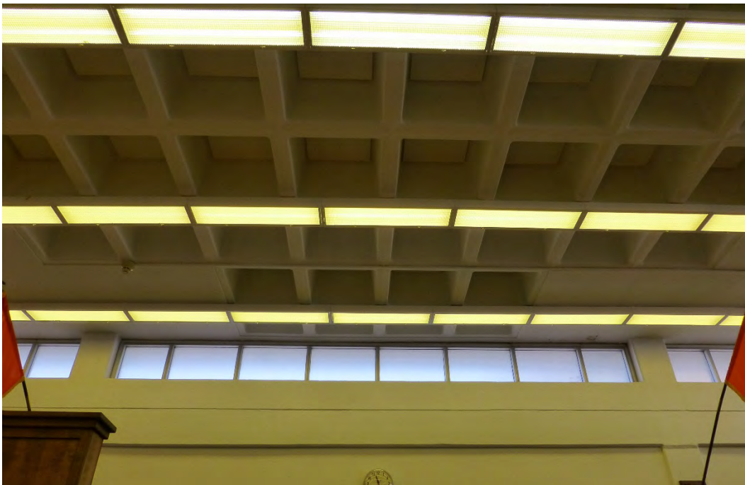
Figure 249. Building 29807, exposed waffle ceiling and clerestory windows (ERDC-CERL, 2015).
