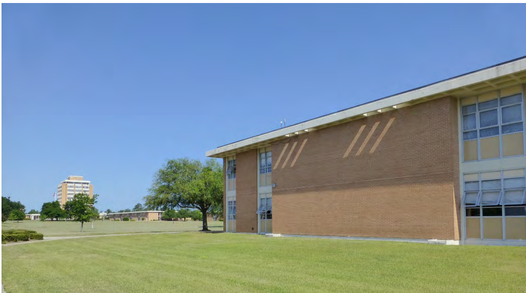
Figure 116. Looking west from Chamberlain Avenue toward the Signal School Campus with Building 29815, Hazen Hall, on the right and the tall Building 29808, Signal Towers, in the background (ERDC-CERL, 2015).
