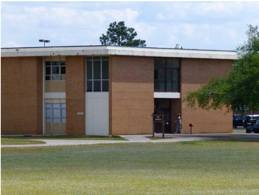
Figure 373. West elevation of Building 29815, Hazen Hall (ERDC-CERL, 2015).
