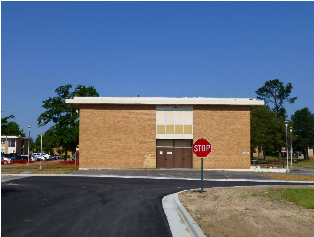
Figure 442. East elevation of Building 29819, Stansell Hall (ERDC-CERL, 2015).
