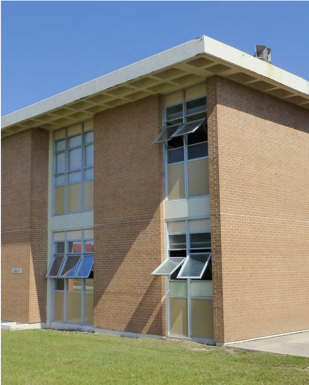
Figure 46. Typical window bay system with bright-aluminum frames, three-pane awning windows, and insulated panels, Building 29813, Allen Hall (ERDC-CERL, 2015).
