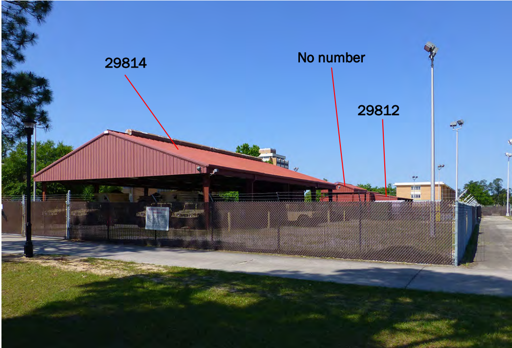
Figure 458. Building 29814 (left) is a covered training area, constructed in 1997; there is an unnumbered covered training area in the middle, constructed circa 2000; and 29812 on the right is a covered training area constructed in 2001 (ERDC-CERL 2015).
