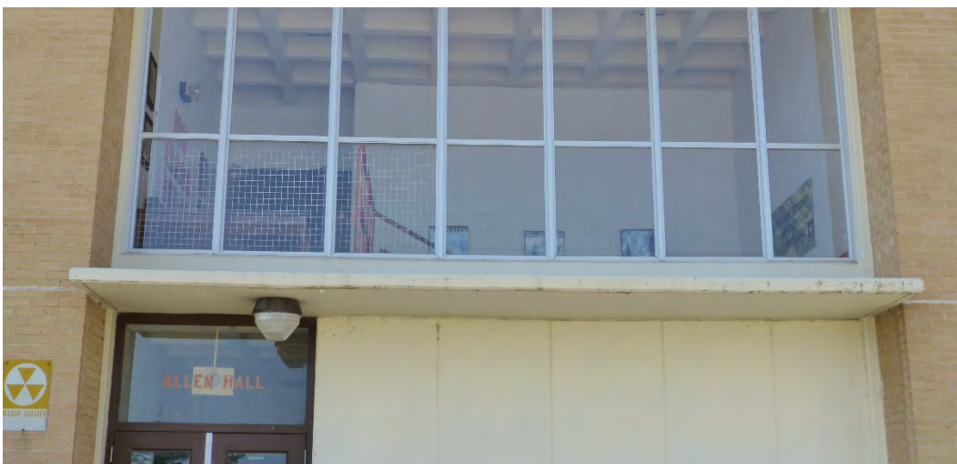
Figure 69. Flat concrete canopy extending over entry doors and a bay of concrete panels on Building 29813, Allen Hall (ERDC-CERL, 2015).
