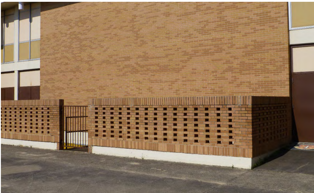
Figure 91. Close-up of the perforated brick wall showing the same type of brick used as the building's brick-veneer exterior wall, Building 29817, Allison Hall (ERDC-CERL 2015).
