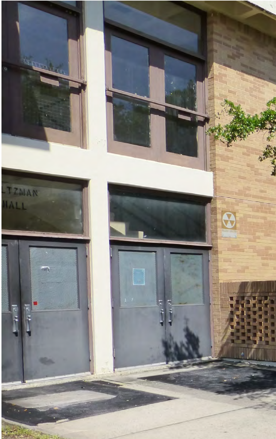
Figure 62. Exposed concrete structure dividing the first and second-floor doors and separating the sets of doors vertically, Building 29811, Saltzman Hall (ERDC-CERL, 2015).
