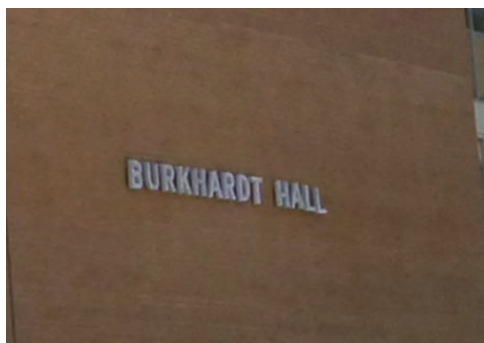
Lettering on the north and south elevations.
