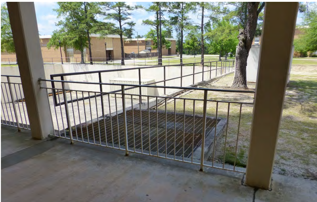
Figure 89. Metal balustrade placed between concrete supports surrounding Building 29808, Signal Towers (ERDC-CERL, 2015).
