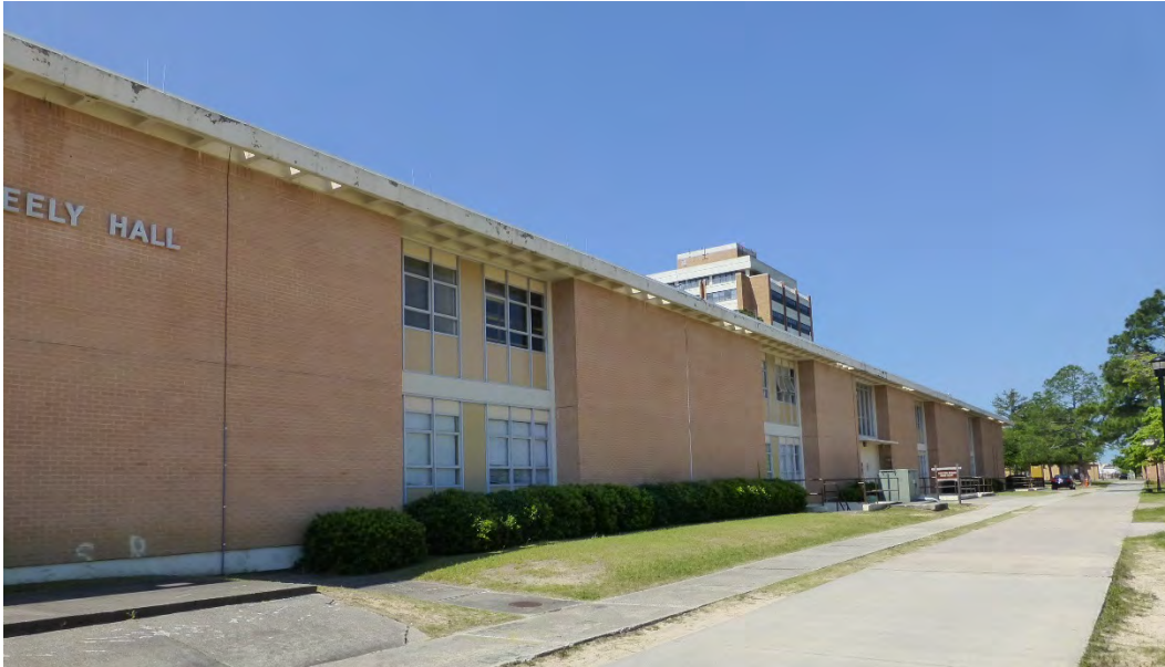
Figure 274. North elevation of Building 29809, Greely Hall (ERDC-CERL, 2015).
