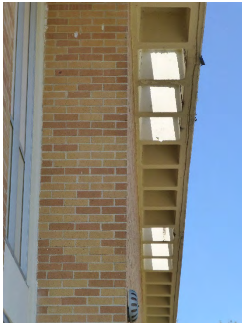
Perforated concrete waffle overhang.
