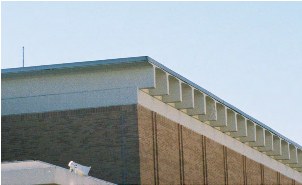
Figure 236. Roof detail of Building 29805, Alexander/Olmstead Halls (ERDC-CERL, 2004).
