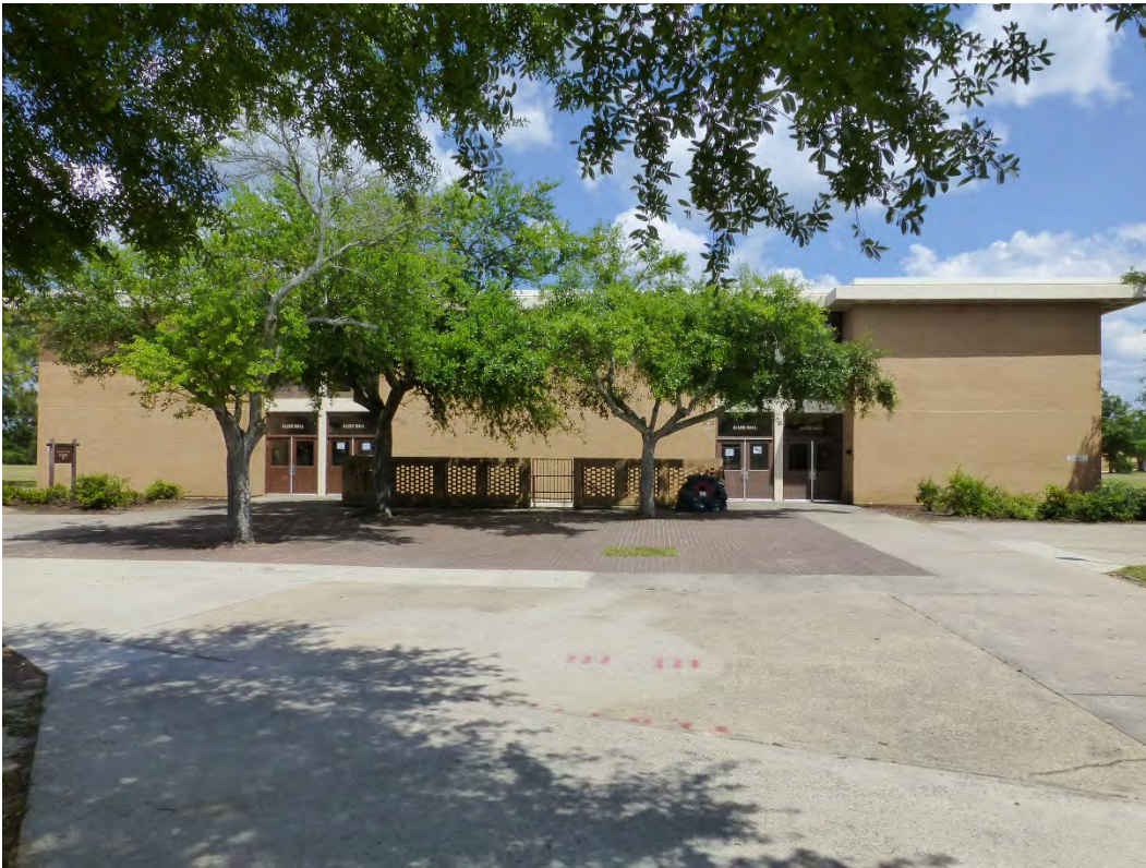
Figure 106. West side of Building 29813, Allen Hall, looking at the brick plaza and three trees (ERDC-CERL, 2015).
