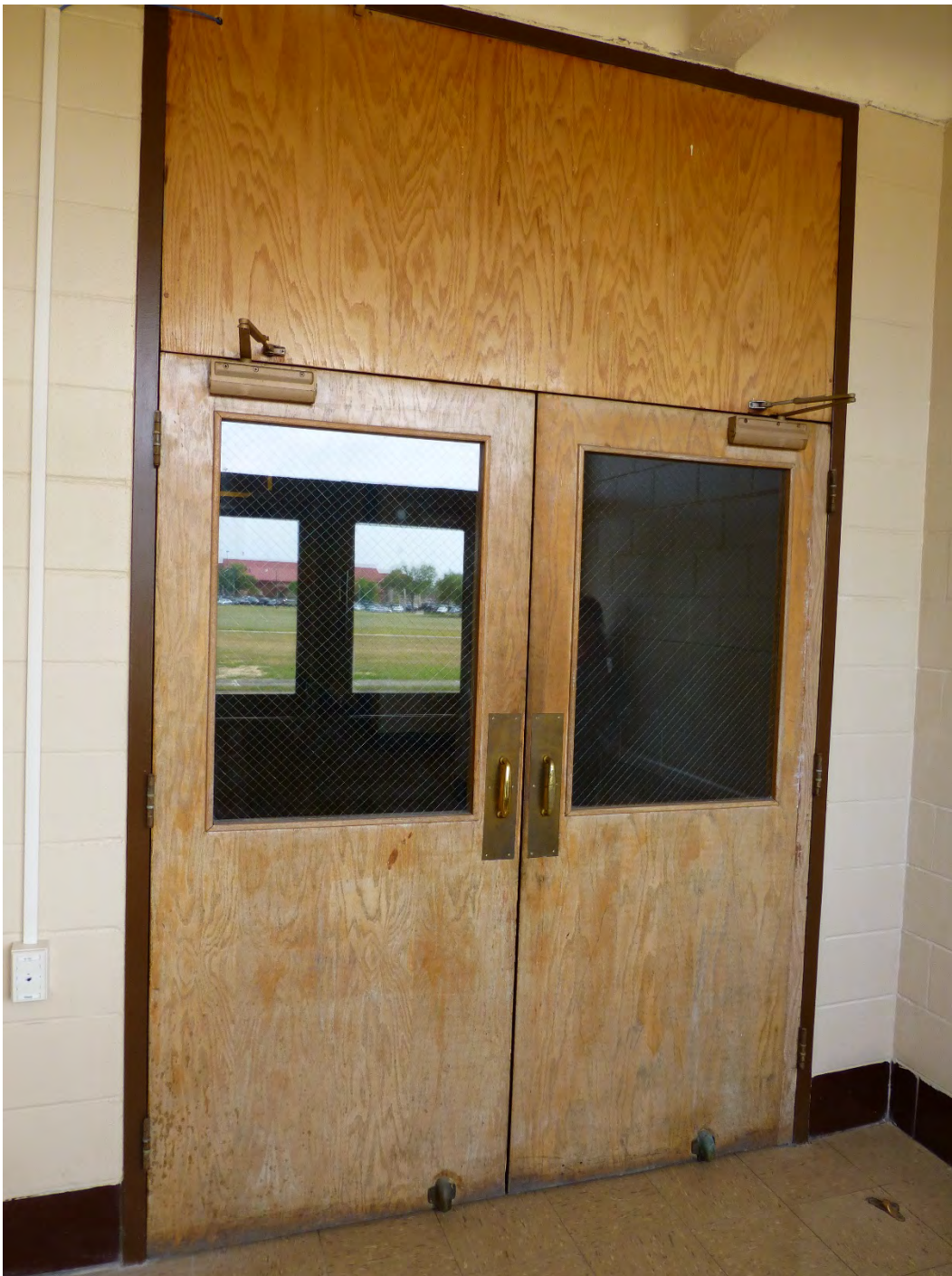
Figure 153. Typical wood doors with a large pane and wood transom, leading from stairwell into the central hallway (ERDC-CERL, 2015).
