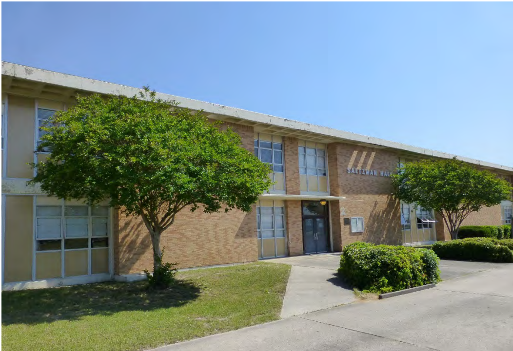
Figure 102. South entry of Building 29811, Saltzman Hall, with two original crabapple trees flanking either side of the entry (ERDC-CERL, 2015).
