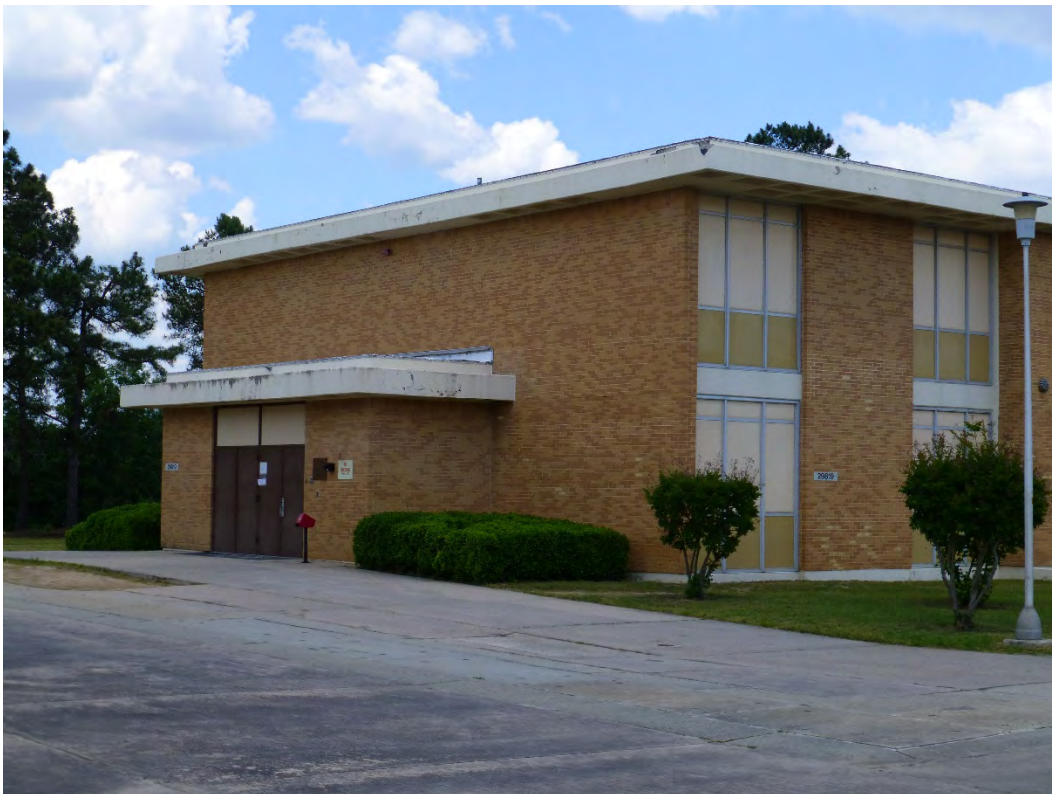
Figure 443. Southwest oblique of Building 29819, Stansell Hall (ERDC-CERL, 2015).
