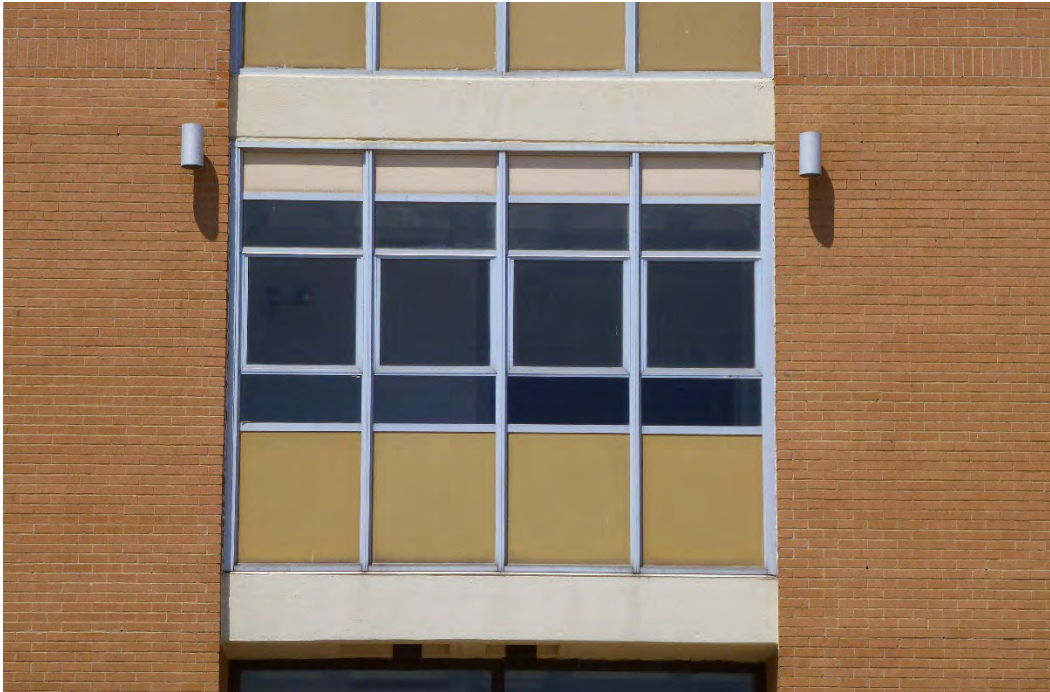
Figure 44. Typical four-bay window system designed with bright-aluminum frames, three-pane awning windows, and insulated panels, Building 29810, Burkhardt Hall (ERDC-CERL, 2015).
