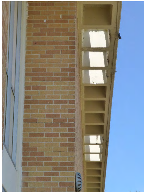
Concrete overhang with perforated waffle.
