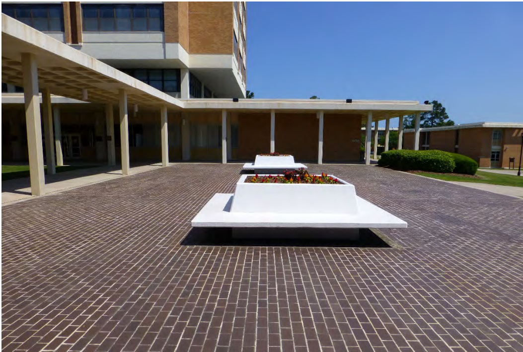
Figure 260. Brick plaza connects Buildings 29805, 29807, and 29808 (ERDC-CERL, 2015).
