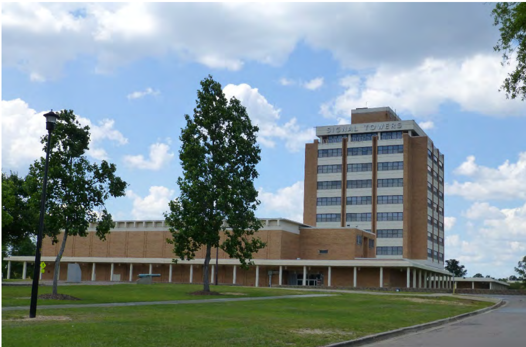
Figure 226. South elevation of Building 29805, Alexander/Olmstead Halls (ERDC-CERL, 2015).
