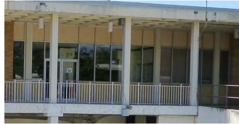
Fixed-pane windows sandwiched between insulated panels and framed in bright-aluminum framing.
