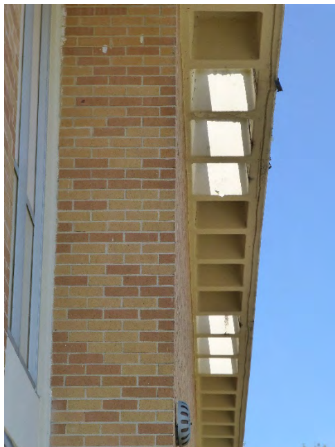
Perforated concrete waffle overhang.
