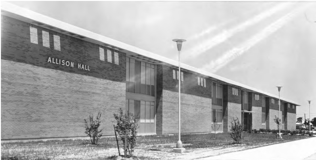
Figure 407. South elevation of Building 29817, Allison Hall, May 1970 (Signal Corps Historian Office).
