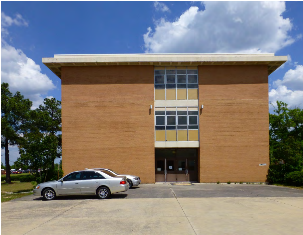
Figure 303. West elevation of Building 29810, Burkhardt Hall (ERDC-CERL, 2015).
