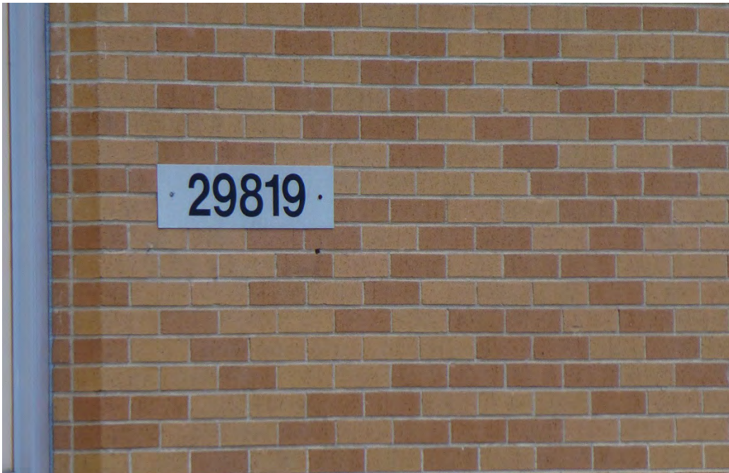
Figure 35. Close-up of an example of the brick veneer exterior walls, Building 29819, Stansell Hall (ERDC-CERL, 2015).
