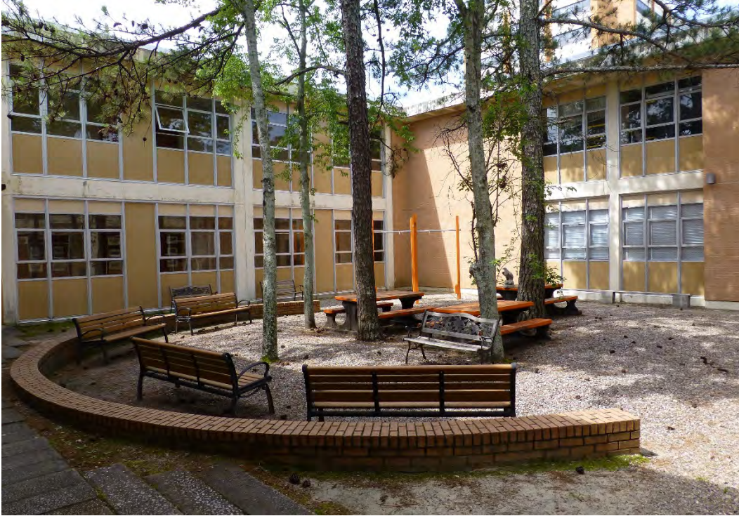
Figure 95. Interior view of the west courtyard in Building 29809, Greely Hall, showing the designed landscape plan of the trees and the curved brick-sitting wall (ERDC-CERL, 2015).
