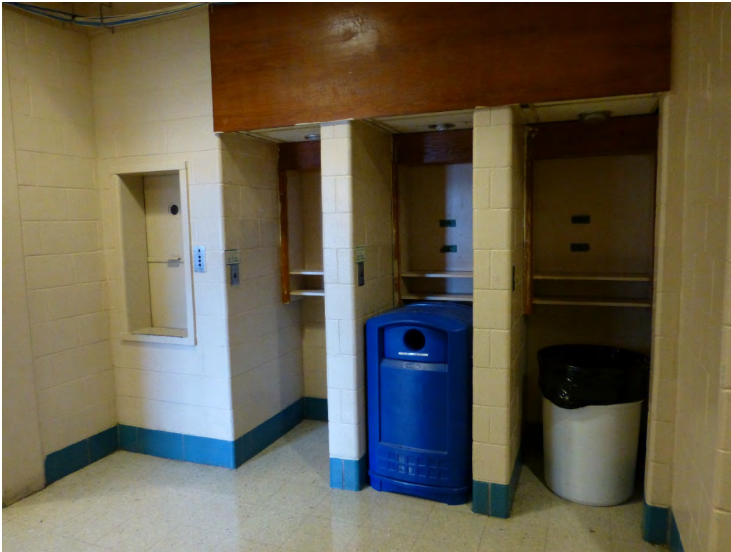
Figure 160. Example of an original telephone alcove, which is no longer being used for its original purpose (ERDC-CERL, 2015).
