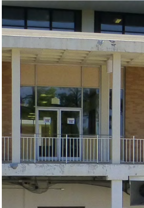
Bright aluminium and plate-glass entry doors.
