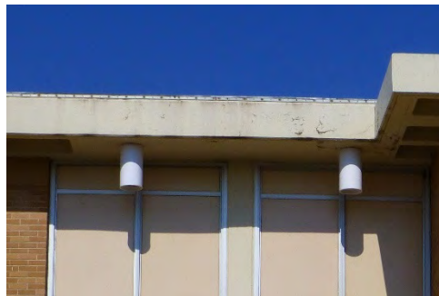
Ceiling-mounted light fixture under the waffle overhang on the east and west elevations.
