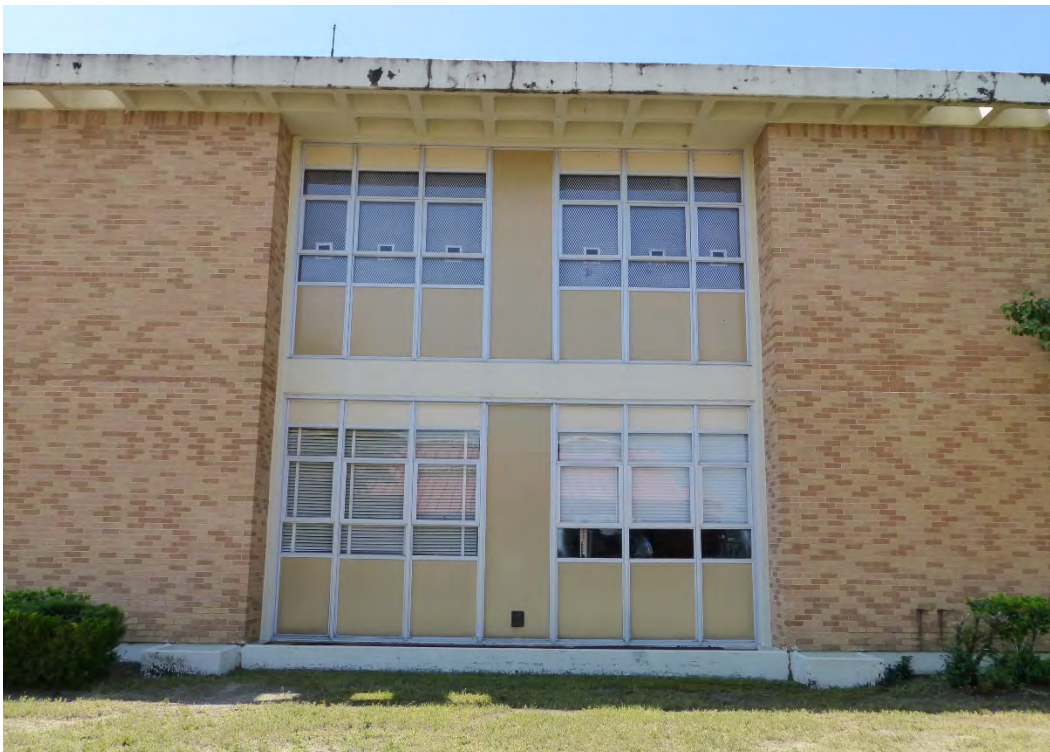
Figure 45. Typical seven-bay window system with bright-aluminum frames, six three-pane awning windows separated by insulated panels and sandwiched by insulated panels, Building 29811, Saltzman Hall (ERDC-CERL, 2015).
