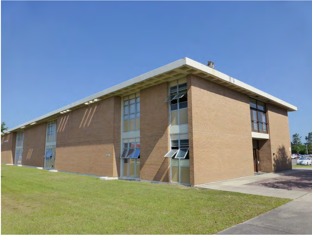
Figure 372. East elevation of Building 29815, Hazen Hall (ERDC-CERL, 2015).
