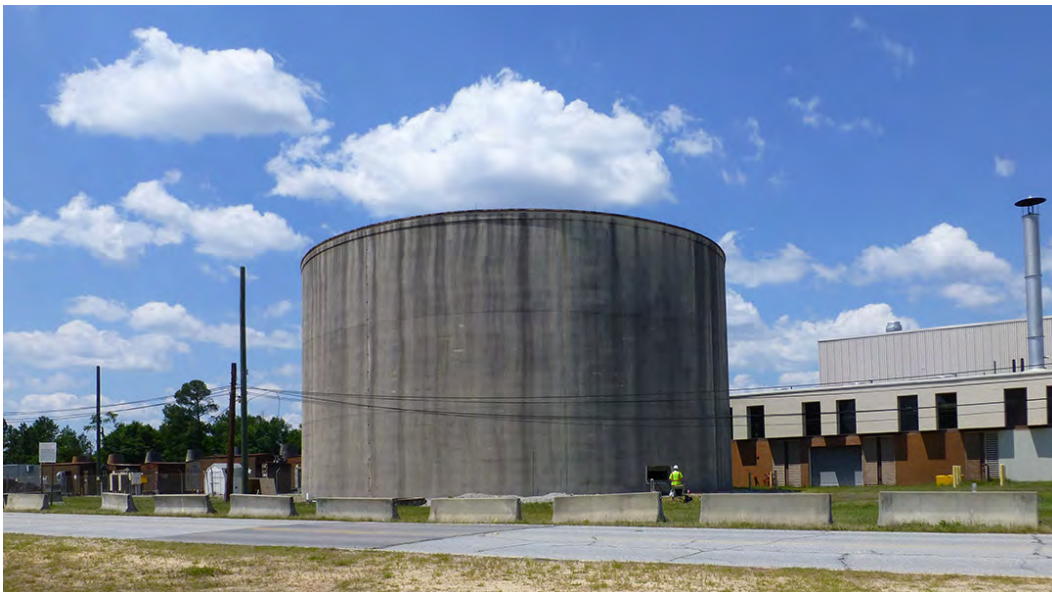
Figure 462. Building 25912 Water Storage Tank was constructed in 2000 (ERDC-CERL 2015).
