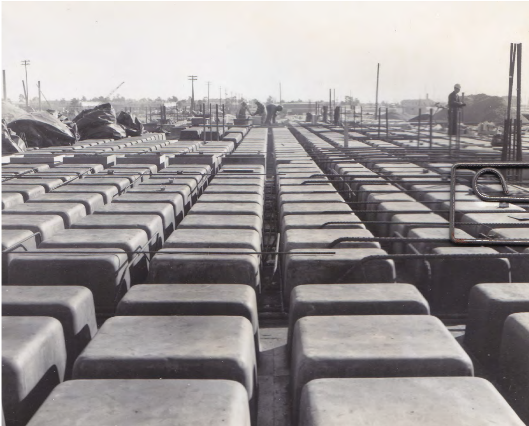
Figure 11. Forms for the concrete waffles at Fort Gordon, 1963 (Fort Gordon DPW).
