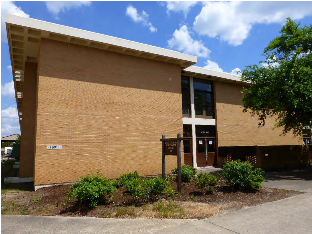
Figure 38. Typical concrete waffle overhang on the classroom buildings, Building 29813, Allen Hall (ERDC-CERL, 2015).
