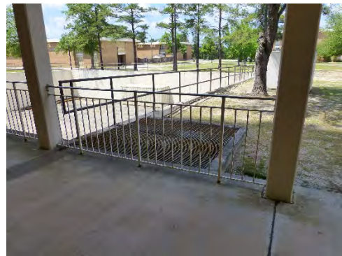
Metal handrail encompassing covered walkway around the building.
