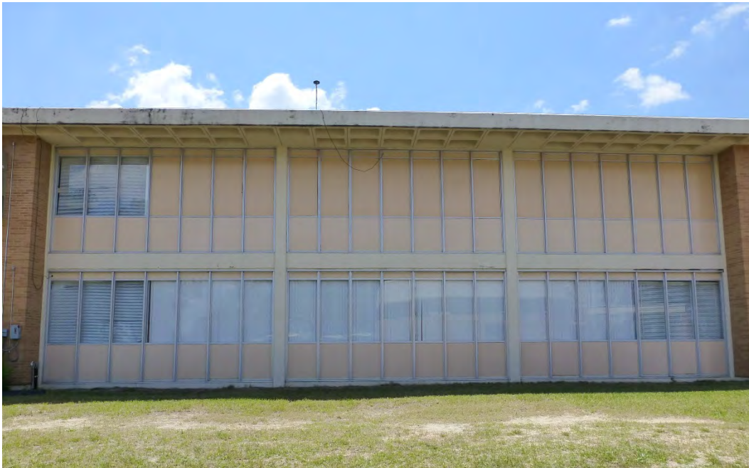
Figure 177. Building 25810, Brant Hall, east elevation of the east wing (ERDC-CERL, 2015).
