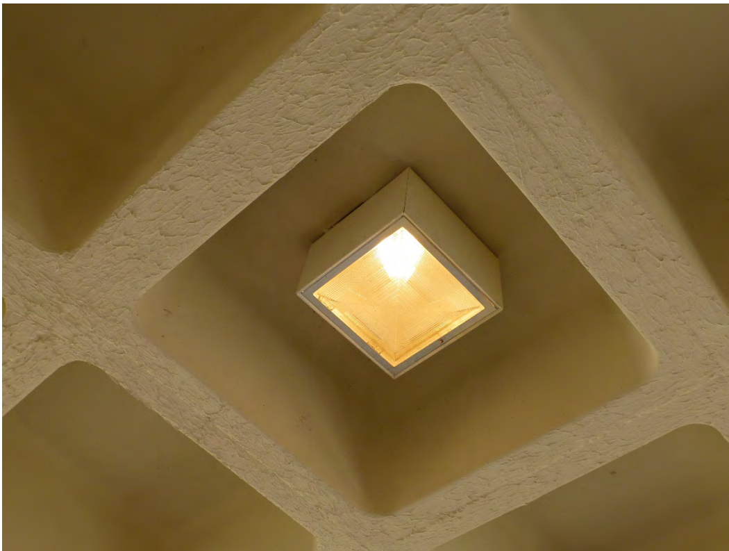
Figure 142. Replacement in-kind, square, ceiling-mounted light fixture set within the waffle ceiling (ERDC-CERL, 2015).
