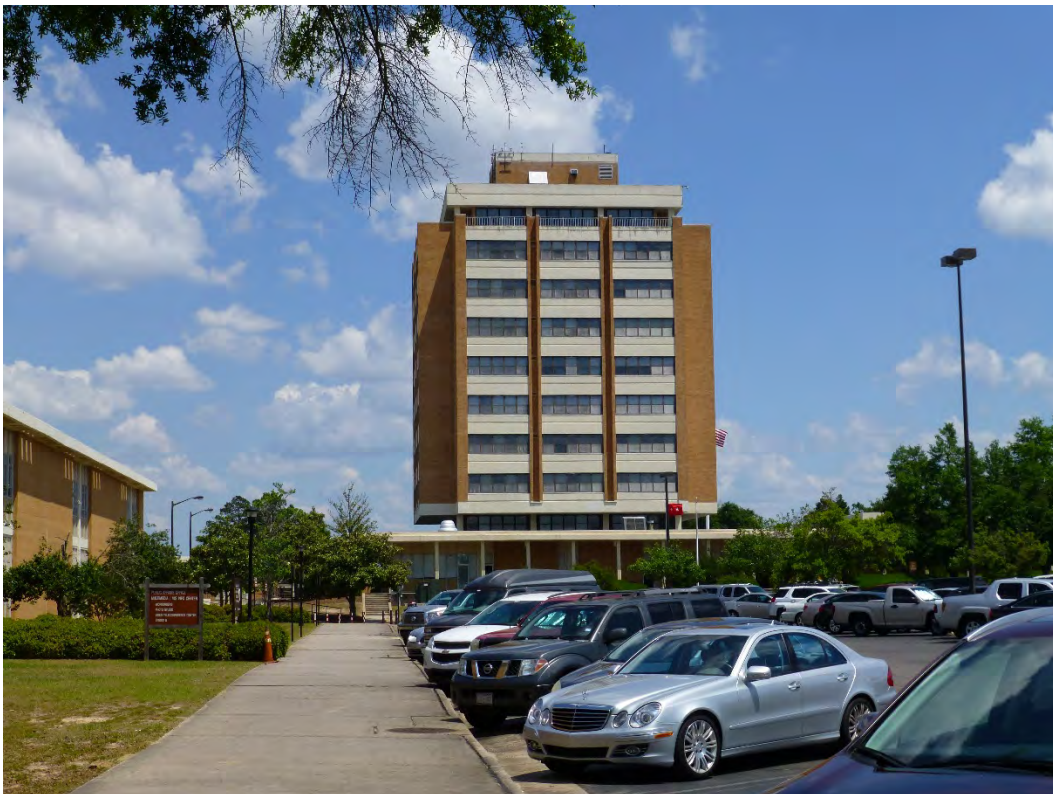
Figure 259. West elevation of Building 29808, Signal Towers (ERDC-CERL, 2015).
