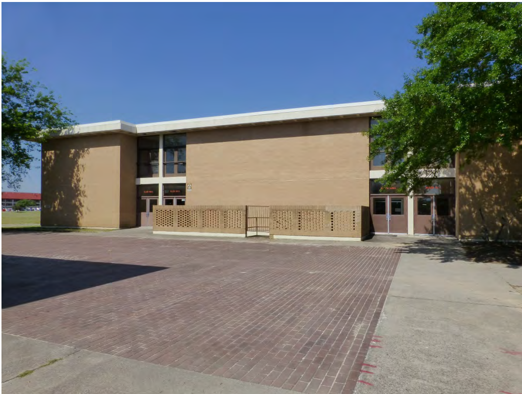
Figure 345. East elevation of Building 29813, Allen Hall (ERDC-CERL, 2015).
