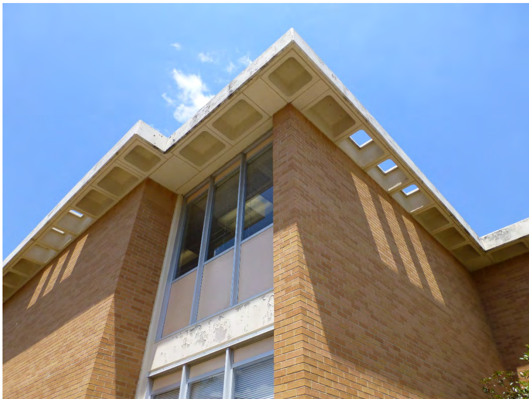
Figure 36. Concrete waffle ceiling structure that extend out to form an overhang, Building 25810, Brant Hall (ERDC-CERL, 2015).
