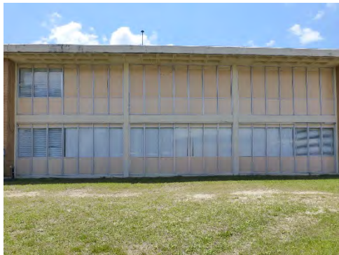
Groups of windows; bright-aluminum frame with fixed panes and insulated panels divided by concrete columns and beam. *Note: the removal of the second-floor windows replaced with new panel inserts.
