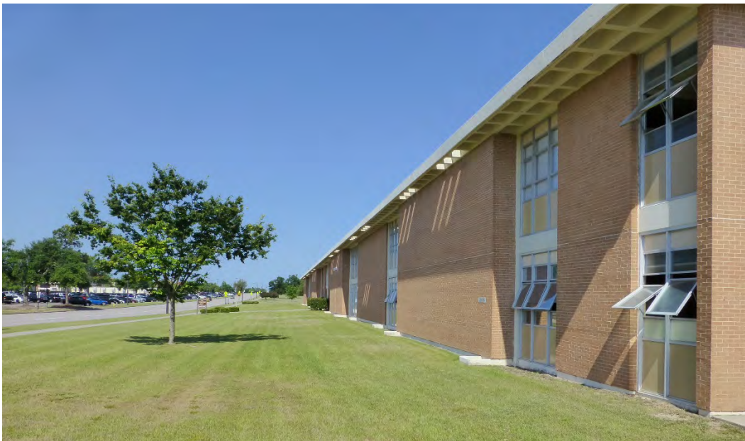
Figure 371. South elevation of Building 29815, Hazen Hall (ERDC-CERL, 2015).
