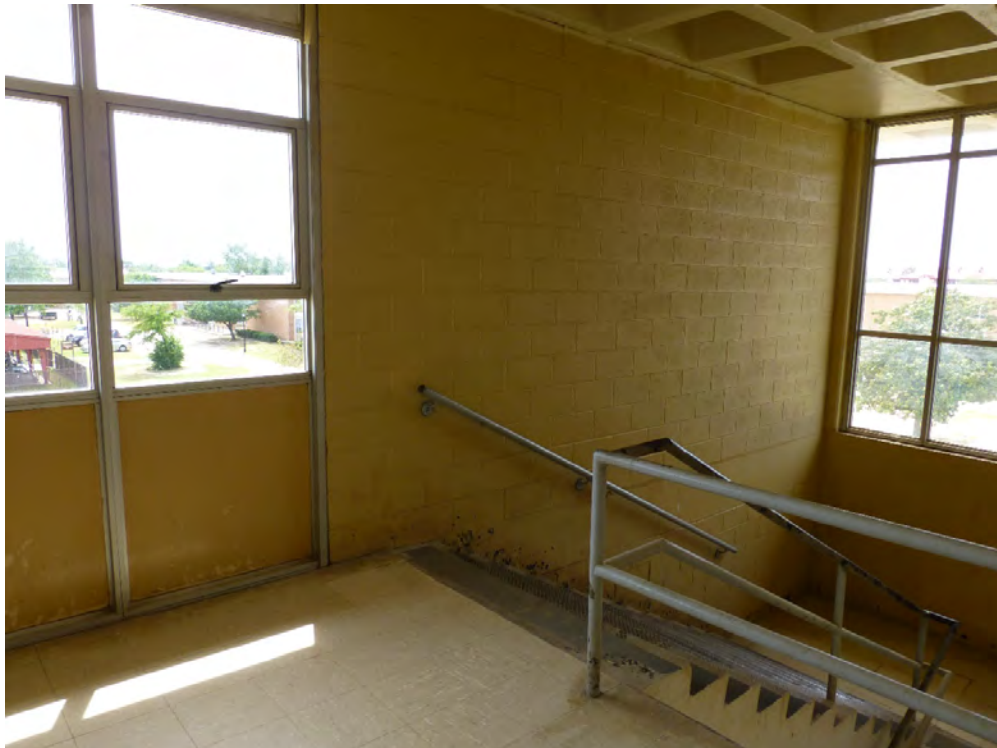
Figure 137. Typical stairwell (ERDC-CERL, 2015).
