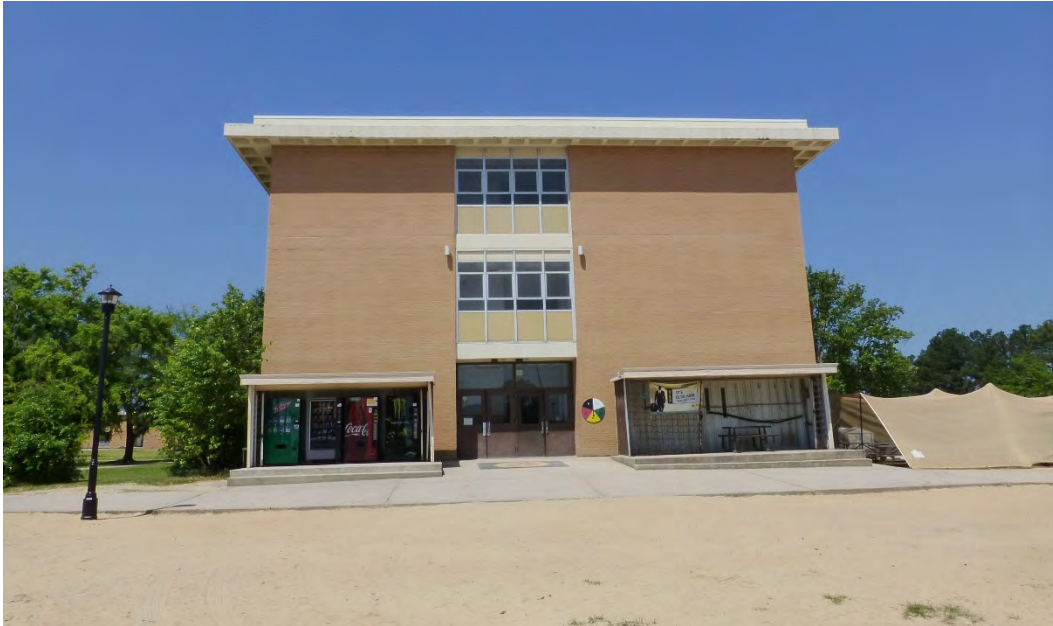
Figure 301. East elevation of Building 29810, Burkhardt Hall (ERDC-CERL, 2015).
