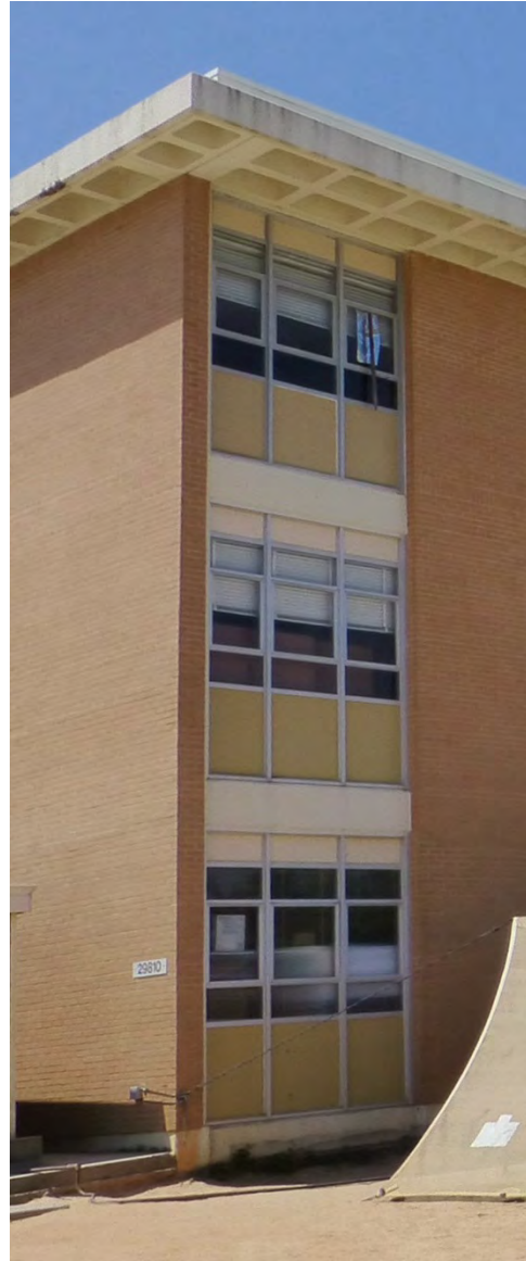
Windows are bright-aluminum framing a three-pane awning-style window sandwiched between insulated panels.
