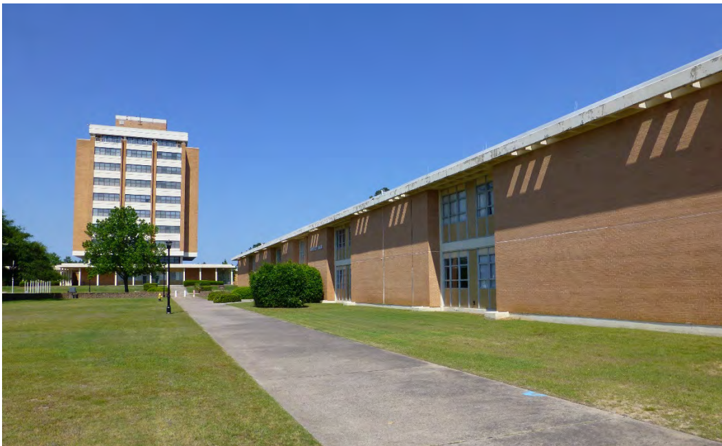
Figure 115. View looking west with Building 29809, Greely Hall, on the right and Building 29808, Signal Towers, in the background (ERDC-CERL, 2015).
