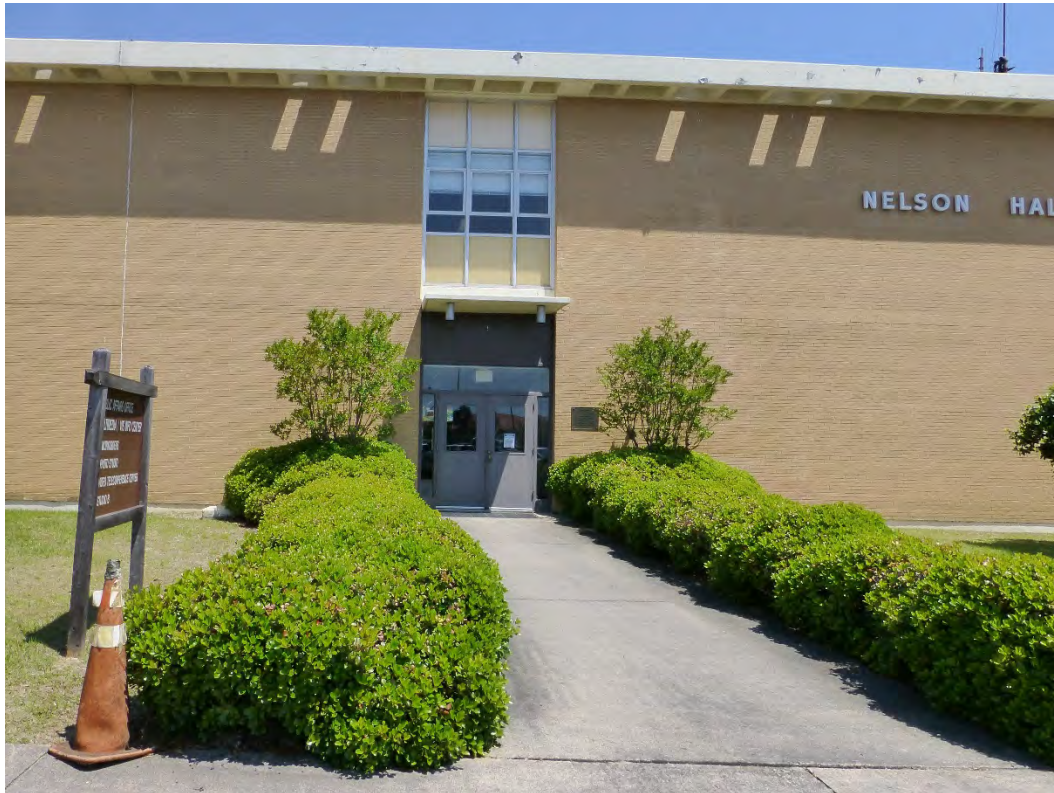
Figure 191. South elevation of Building 29801, Nelson Hall (ERDC-CERL, 2015).
