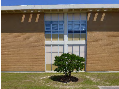
Window bays on the south elevation and “light pattern” cast from the perforated waffle roof overhang.
