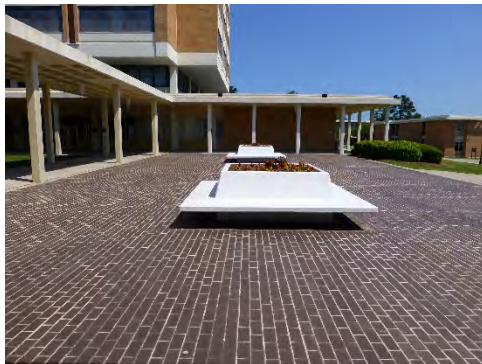
Brick plaza connecting Buildings 29805, 29807, and 29808.
