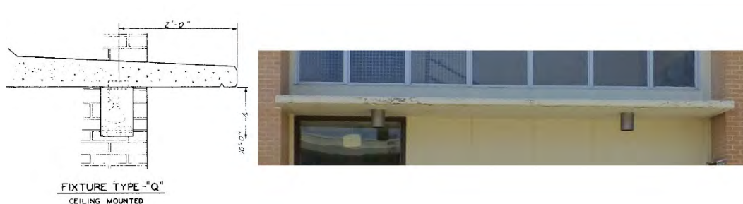
Figure 298. Ceiling-mounted light fixture under flat concrete canopy – comparison of the original design and material from 1966 [left] to the current condition of the ceiling-mounted light fixture [right] (ERDC-CERL, 2015).
