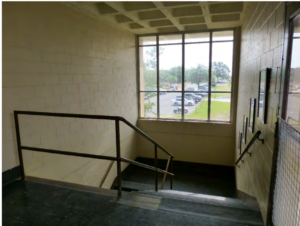
Figure 135. Interior view of the south stairwell in Building 29816, showing concrete switchback stairs, metal handrails, exposed concrete walls, and exposed concrete waffle ceiling (ERDC-CERL, 2015).
