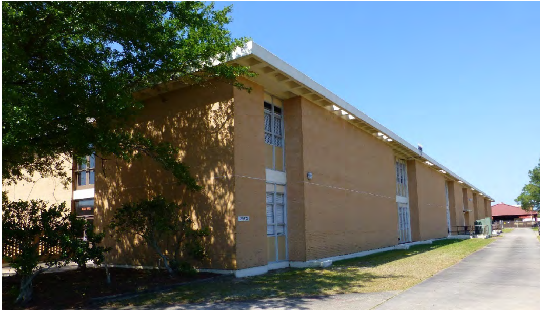
Figure 34. Brick veneer exterior walls, Building 29813, Allen Hall (ERDC-CERL, 2015).
