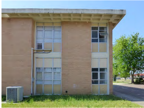
Window bays consisting of bright-aluminum three-pane awning-style windows sandwiched between insulated panels.
