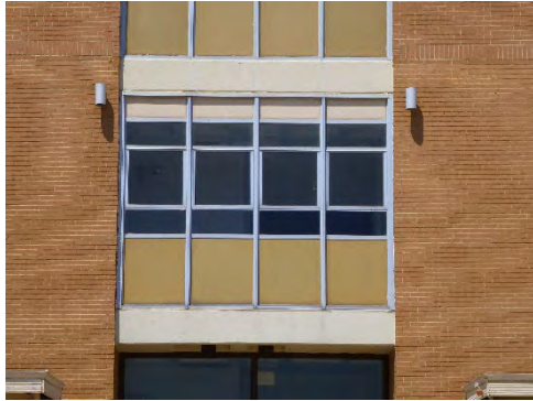
Group of four bright-aluminum-framed, three-pane awning-style windows are sandwiched between insulated panels that are located on the 2 nd and 3 rd floors of the east and west elevations above the entries.
