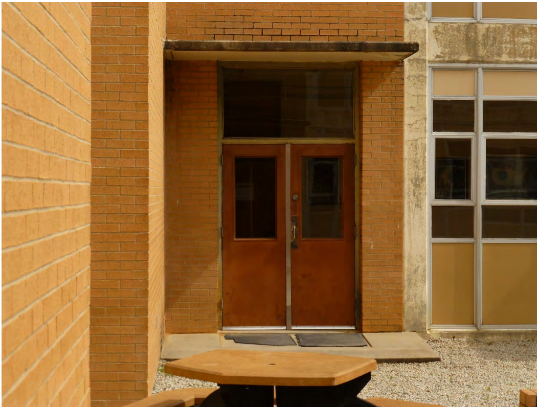
Figure 61. Typical doors located on the north and south walls entering the courtyards, Building 29811, Saltzman Hall (ERDC-CERL, 2015).
