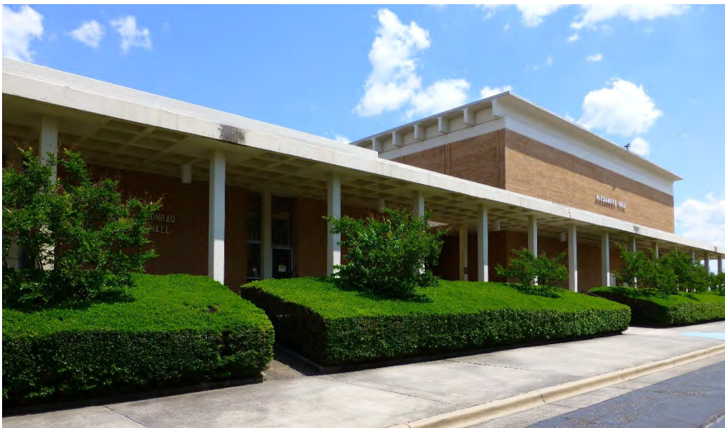
Figure 248. West side of Building 29807 with single entry doors and the concrete waffle canopy that connects to Buildings 29805 and 29808 (ERDC-CERL, 2015).
