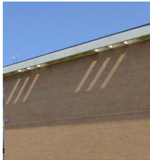
“Light pattern” created by the perforated concrete waffle overhang.
