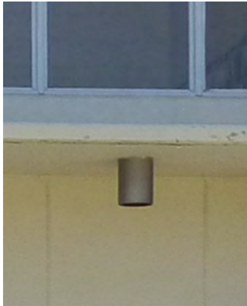
Ceiling-mounted light fixture under flat canopies.
