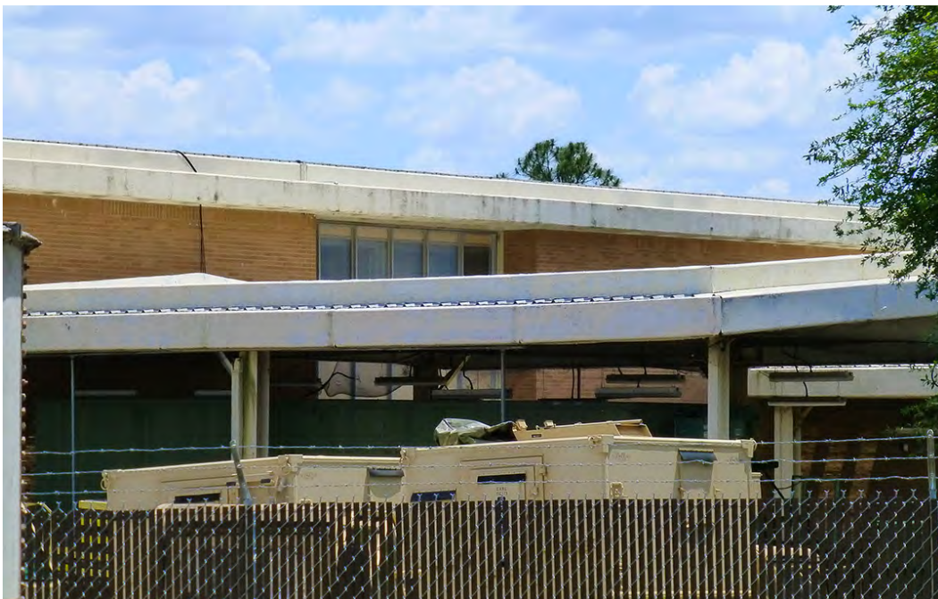
Figure 457. Buildings 25812 and 25813 are covered storage areas to the west of Building 25810 (ERDC-CERL).
