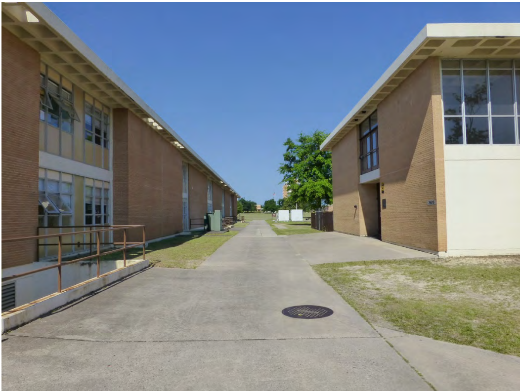
Figure 114. View looking west with Building 29815, Hazen Hall, on left and Building 29816, Fisher Hall, on right (ERDC-CERL, 2015).
