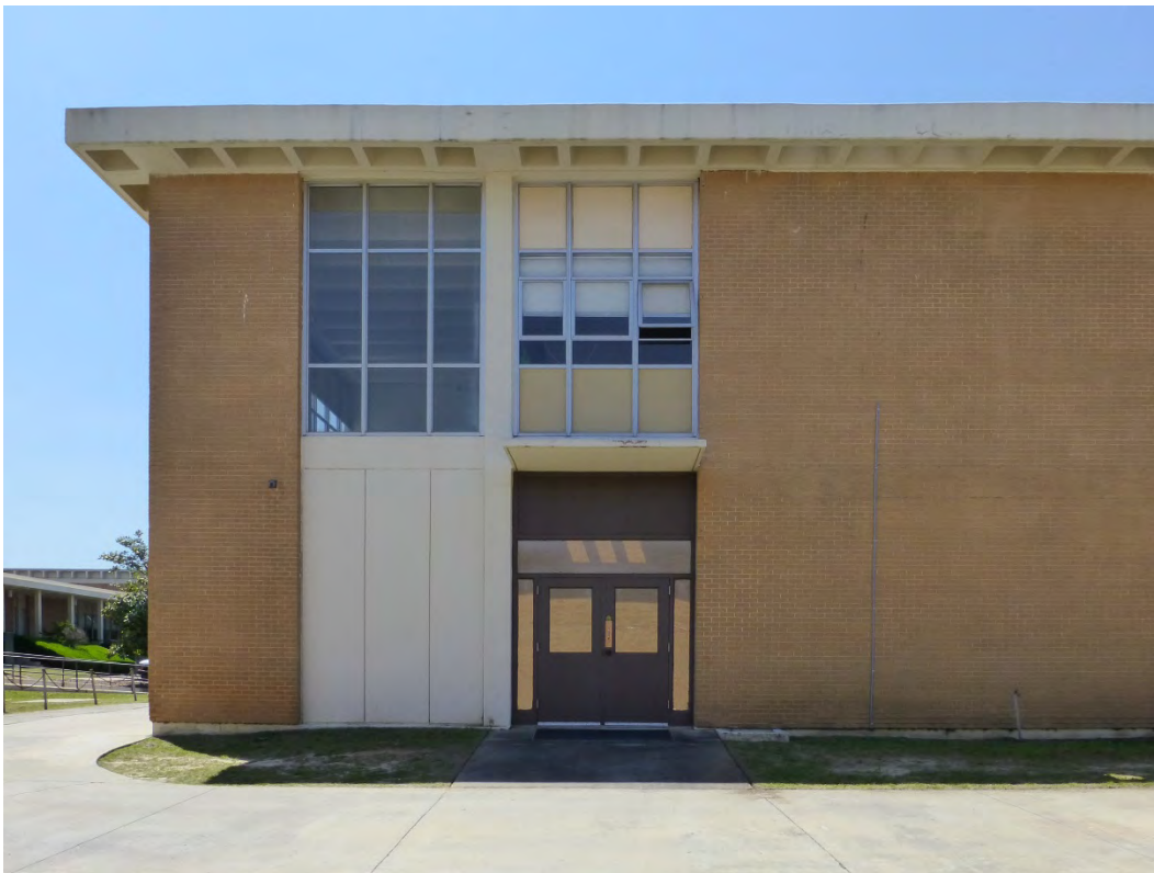
Figure 193. Left side of the north elevation of Building 29801, Nelson Hall (ERDC-CERL, 2015).
