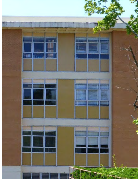
Window pattern; groups of three separated by insulated panel insert. Windows are bright-aluminum framing a three-pane awning-style window sandwiched between insulated panels. Exposed concrete beam structure system divides each floor.
