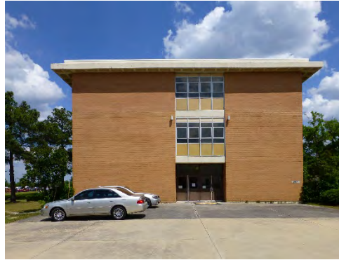
Main entries on the east and west elevations.
