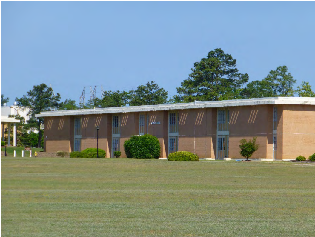
Figure 273. South elevation of Building 29809, Greely Hall (ERDC-CERL, 2015).
