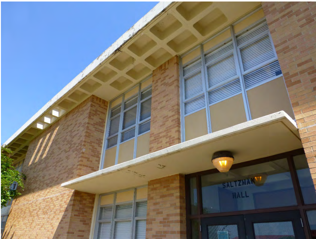
Figure 68. Flat concrete canopy extending over doors and a bay of windows on Building 29811, Saltzman Hall (ERDC-CERL, 2015).
