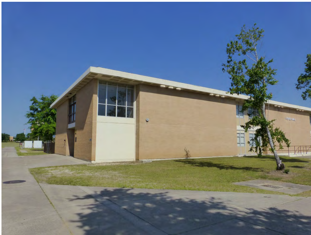
Figure 387. Southeast oblique of Building 29816, Fisher Hall (ERDC-CERL, 2015).
