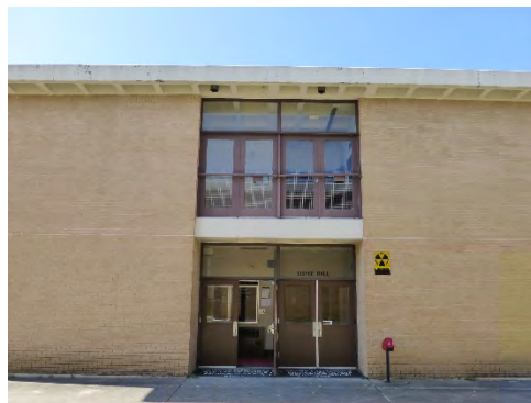
Metal doors with pane and transom on first floor and metal and plate glass doors on second floor, separated by exposed concrete structural system.
