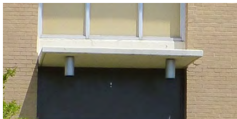
Concrete canopy with ceiling-mounted bronze light fixtures.
