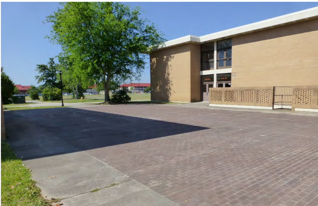
Figure 105. East side of Building 29813, Allen Hall, looking at the brick plaza where all the original trees have been removed (ERDC-CERL, 2015).
