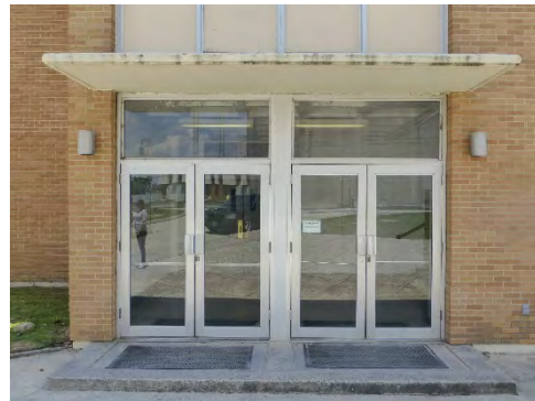
Bright-aluminum and plate-glass doors with transoms protected by a flat concrete canopy.
