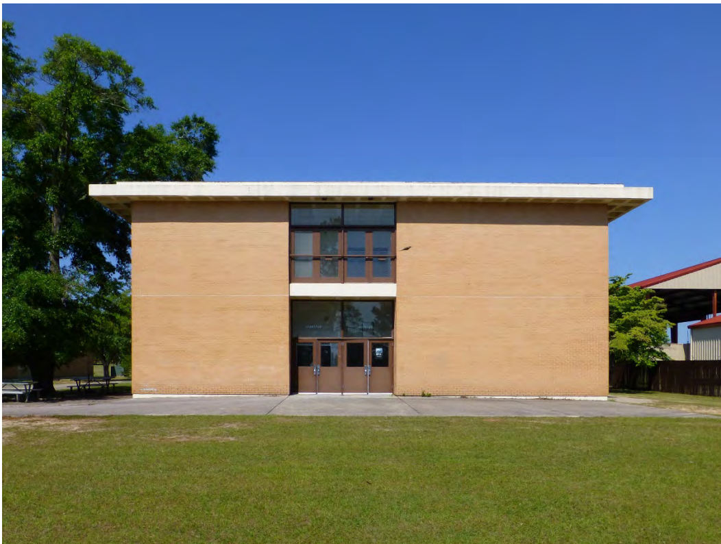
Figure 424. East elevation of Building 29818, Johnston Hall (ERDC-CERL, 2015).
