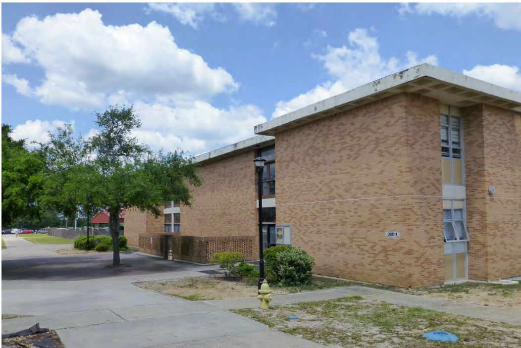
Figure 316. West elevation of Building 29811, Saltzman Hall (ERDC-CERL, 2015).
