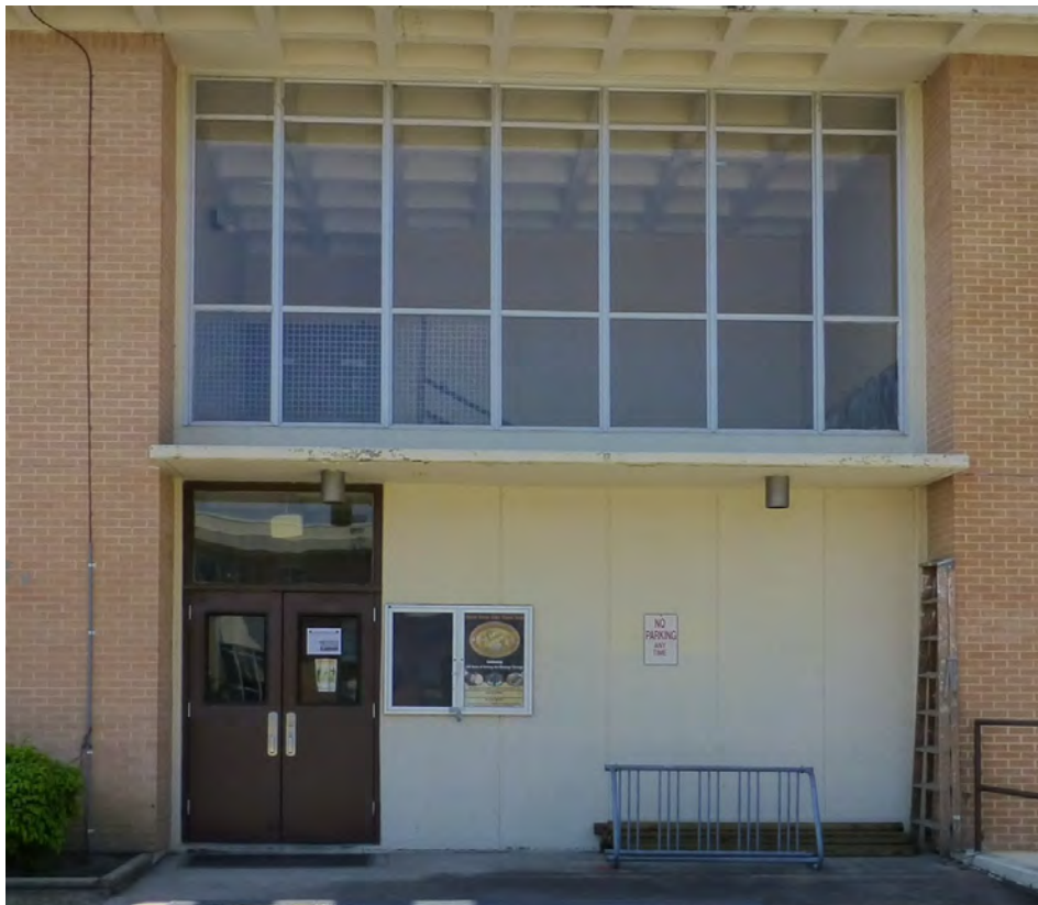
Figure 58. Metal doors with pane and transom above, Building 29809, Greely Hall (ERDC-CERL, 2015).
