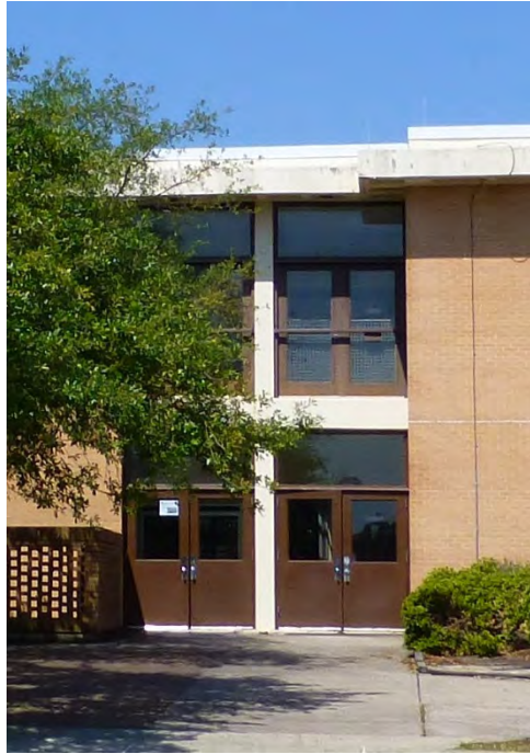
Metal doors with pane and fixed transom on the first floor and paired metal and plate-glass doors on the second floor.
