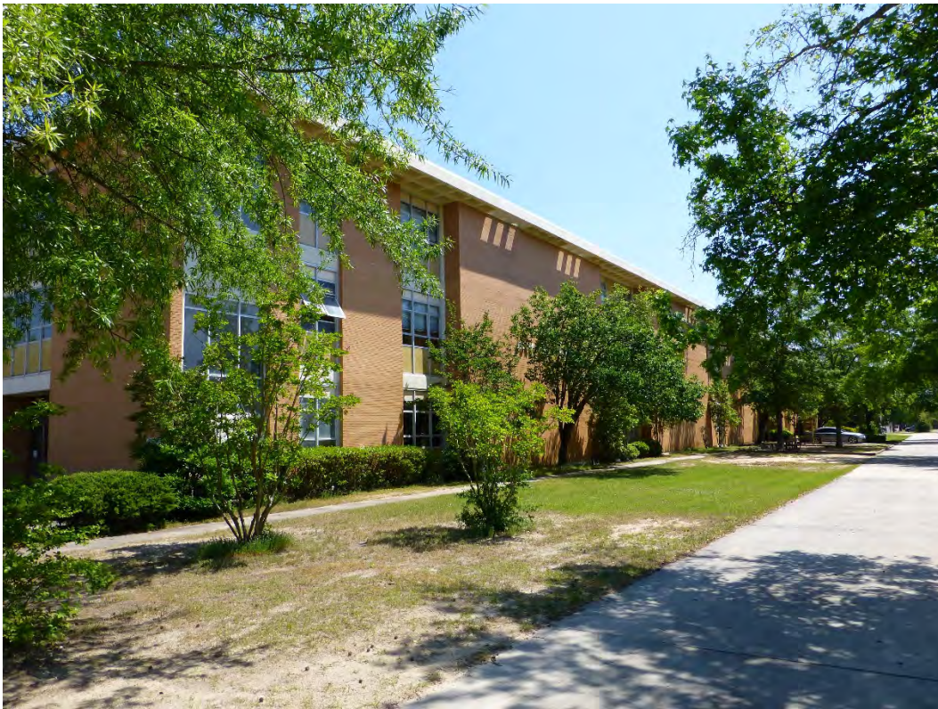
Figure 302. South elevation of Building 29810, Burkhardt Hall (ERDC-CERL, 2015).
