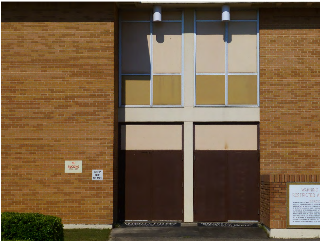
Figure 60. Metal doors with an insulated panel placed in the transom above, Building 29816, Fisher Hall (ERDC-CERL, 2015).
