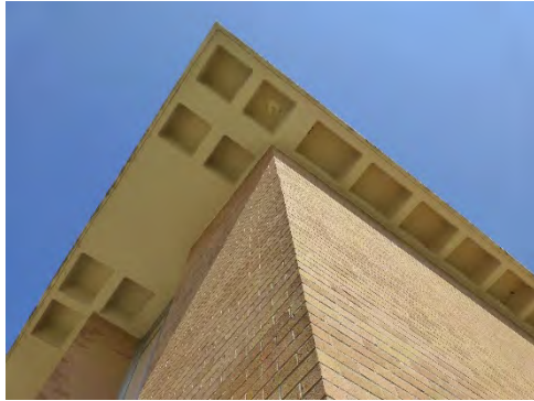
Concrete waffle overhang.
