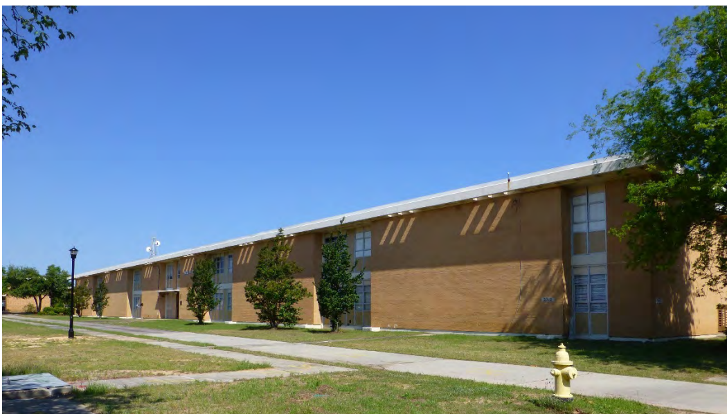
Figure 31. Two-story classroom Building 29813, Allen Hall (ERDC-CERL, 2015).
