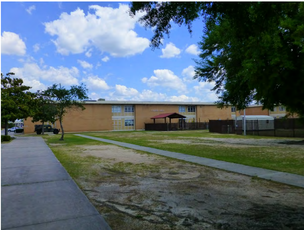
Figure 391. West elevation of Building 29816, Fisher Hall (ERDC-CERL, 2015).
