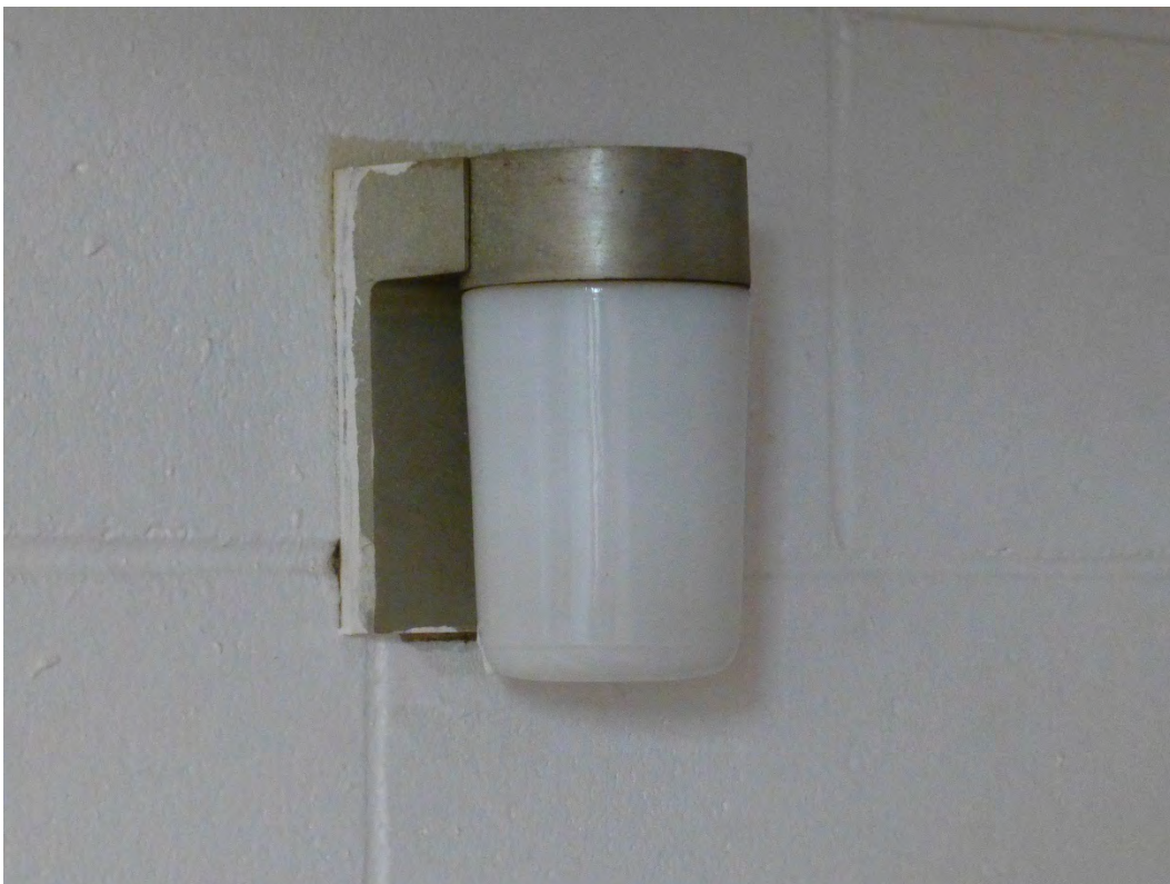
Figure 144. Typical original wall-mounted light fixture (ERDC-CERL, 2015).
