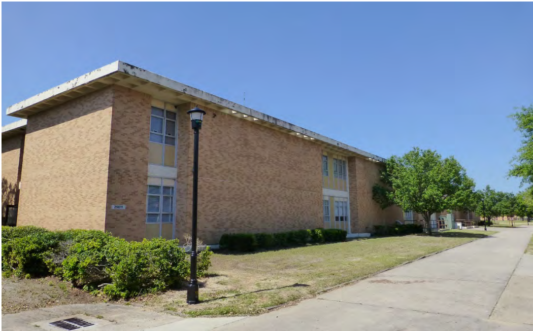
Figure 30. Two-story classroom building, Building 29811, Saltzman Hall (ERDC-CERL, 2015).
