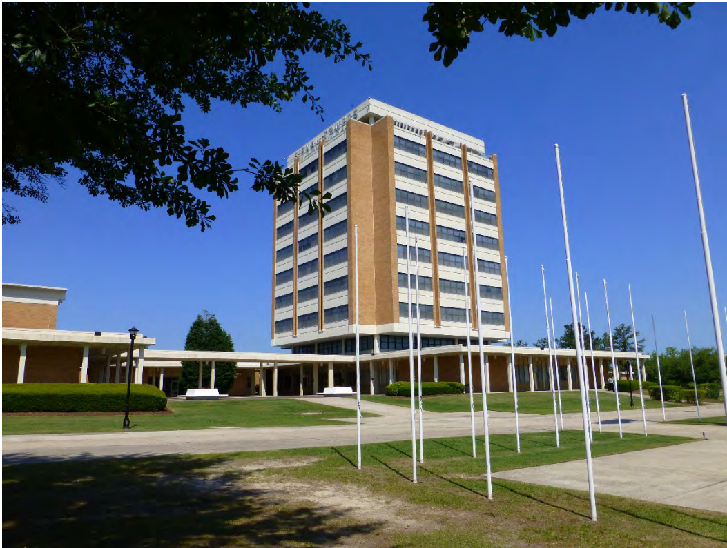
Figure 258. Southeast oblique of Building 29808, Signal Towers (ERDC-CERL, 2015).
