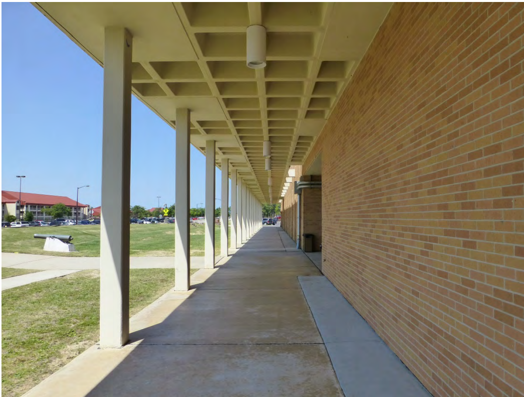
Figure 66. Extensive wrap-around concrete waffle canopy connects the main administration buildings: Building 29805, Alexander/Olmsted Halls; Building 29807, Museum (Conrad Hall); and Building 29808, Signal Towers (ERDC-CERL, 2015).
