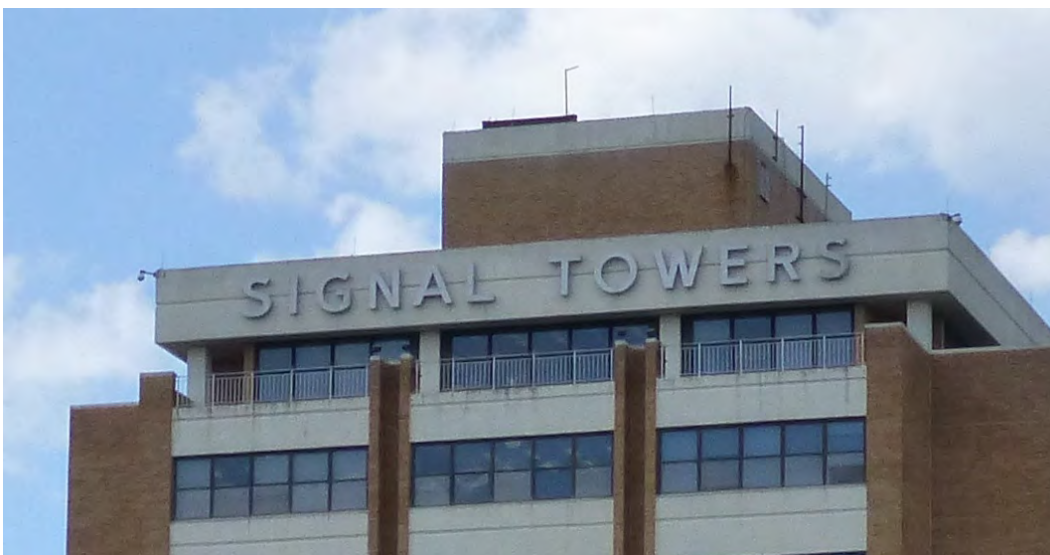
Figure 83. The larger scale of the lettering located at the top of Building 29808, Signal Towers (ERDC-CERL, 2015).
