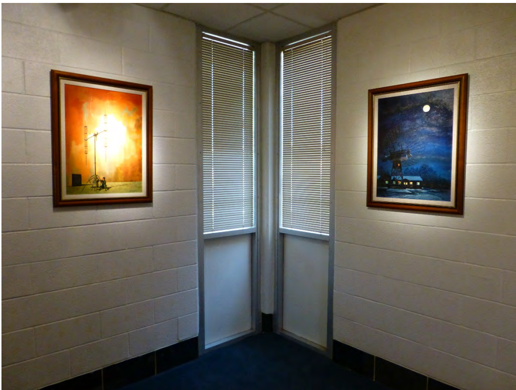
Figure 250. Building 29807, close-up of corner window detail (ERDC-CERL, 2015).
