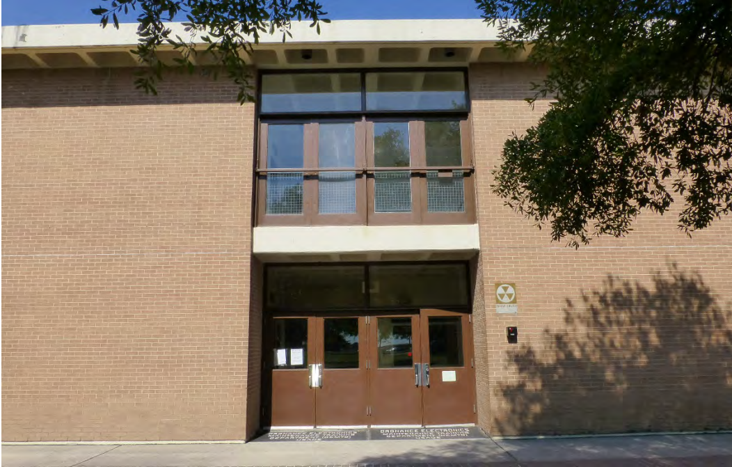
Figure 59. Entry bay that consists of two sets of metal doors with pane and transom on the first floor and two sets of metal and plate-glass doors with transoms above on the second floor, Building 29815, Hazen Hall (ERDC-CERL, 2015).
