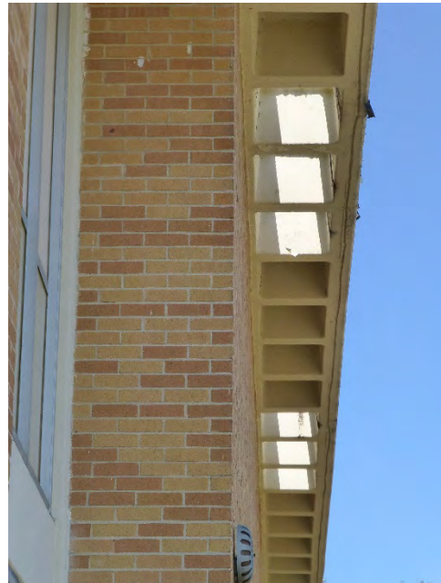
Perforated concrete waffle overhang.
