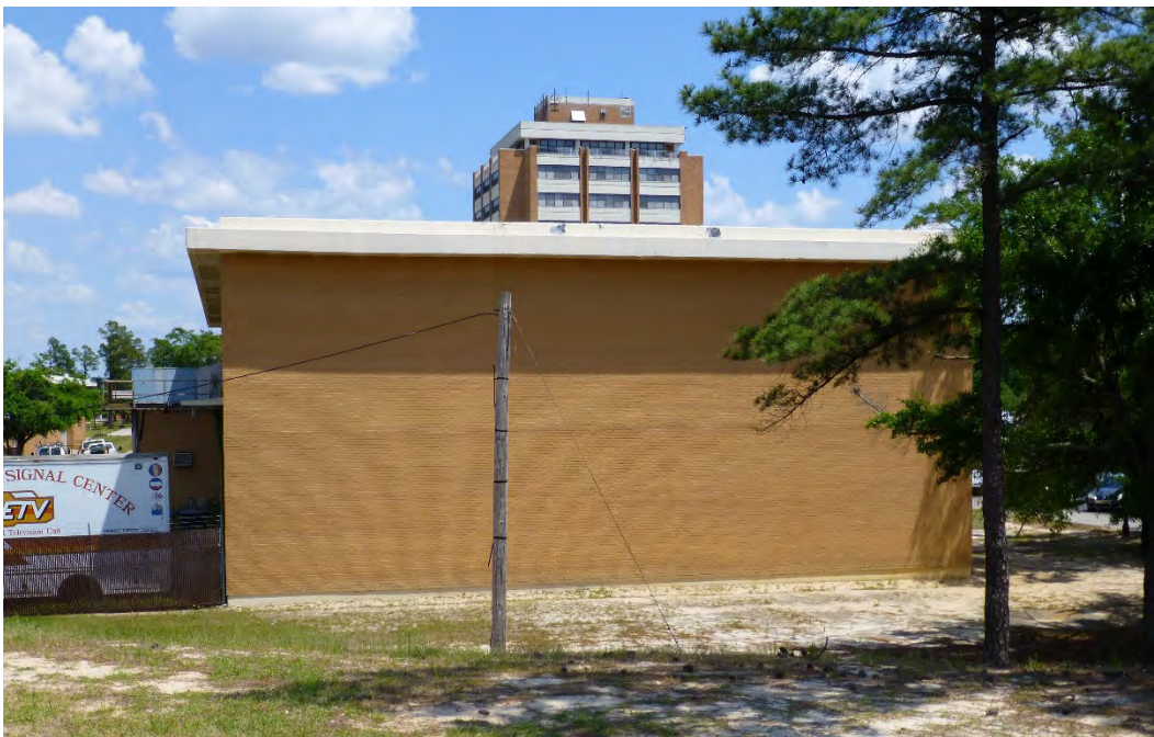
Figure 194. West elevation of Building 29801, Nelson Hall (ERDC-CERL, 2015).
