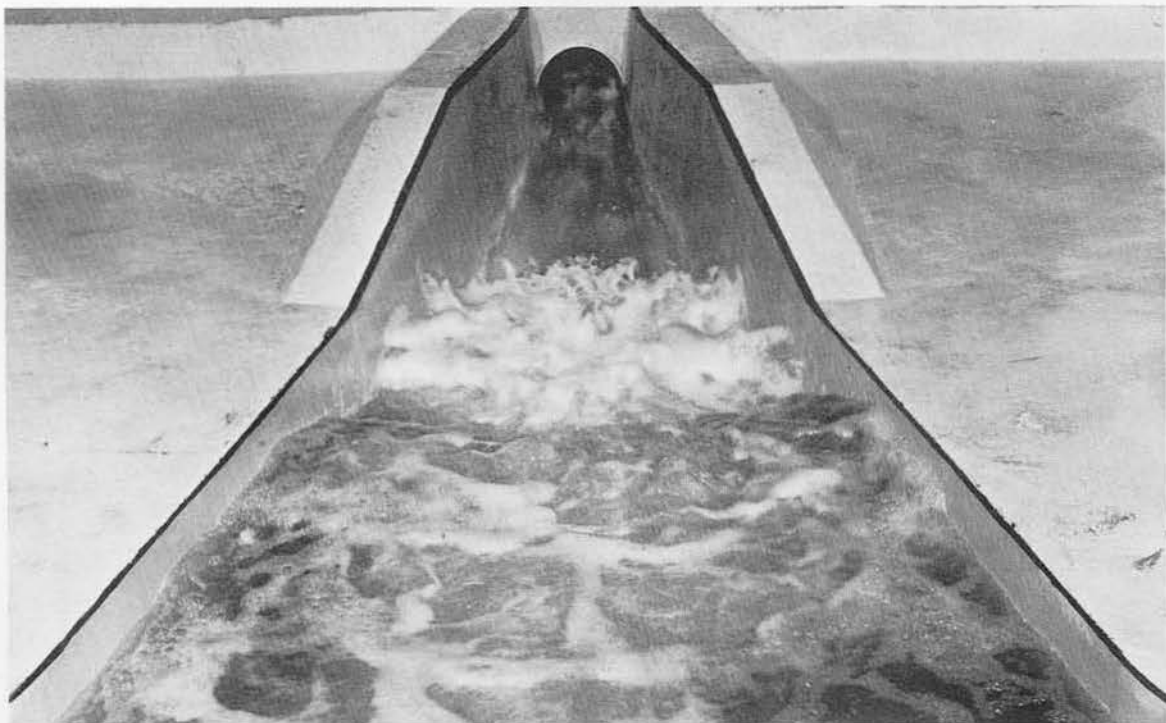
Photograph 13. Discharge, 12,500 cfs; pool elev, 592.0; TW elev, 398.0 Flow in stilling basin, type 8 design, center gate open, side gates 1/4 open
