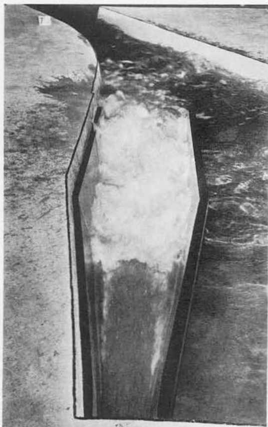
Photograph 19. Flow through original design stilling basin with 7.5-ft end sill Discharge, 10,800 cfs Tailwater elev, 926.8 (normal)
