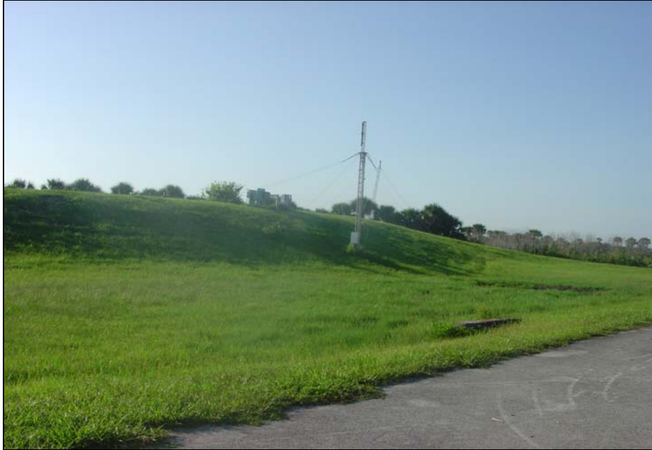
Figure 2-9: Site 7—Universal Camera Site 13 on KSC
