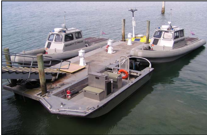
Figure 1-3: Existing Boat Dock in Trident Turning Basin at CCAFS
