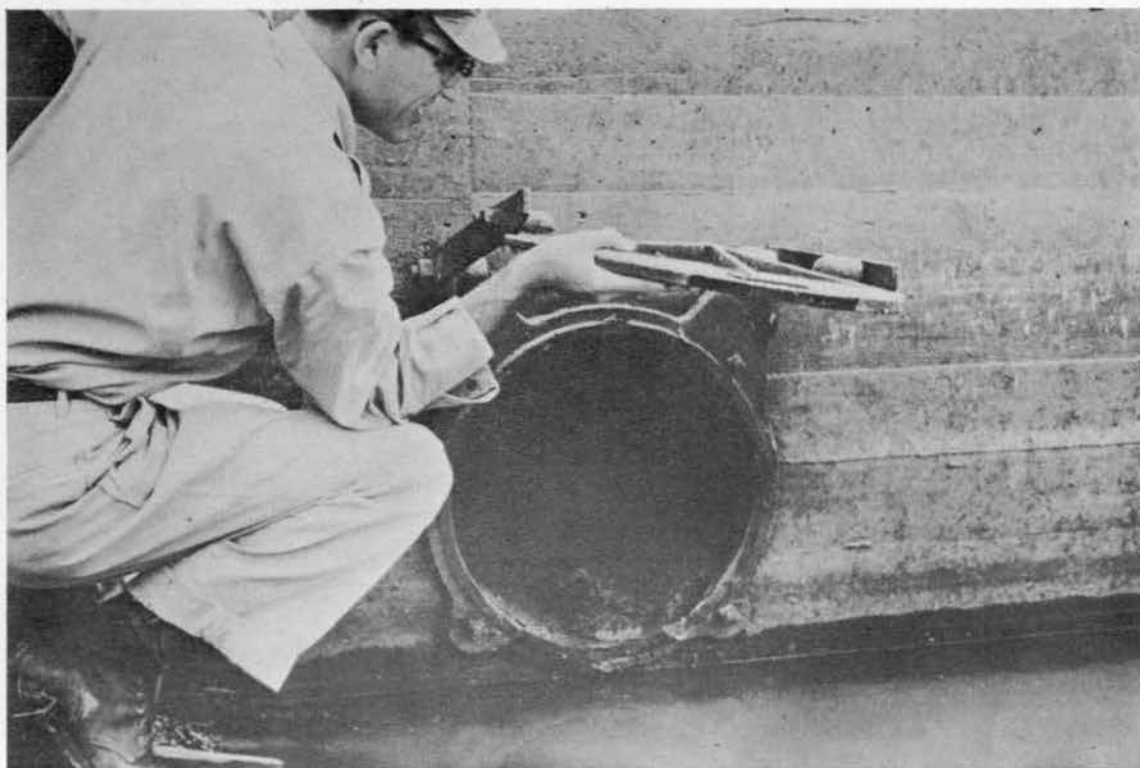
Fig. 8. Mud behind 18-in. flap gate (July 1955)
