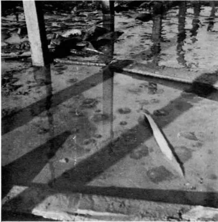
Numerous sand boils upstream of conduits (9 June 1951)
