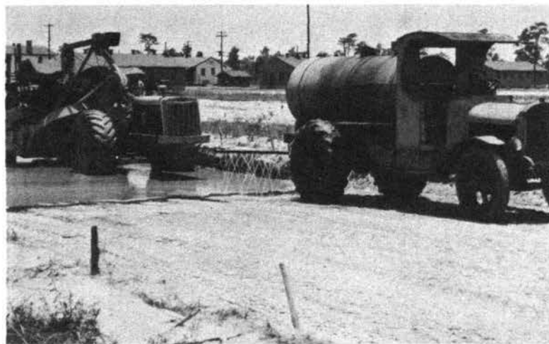
Sprinkling operation during tracking
