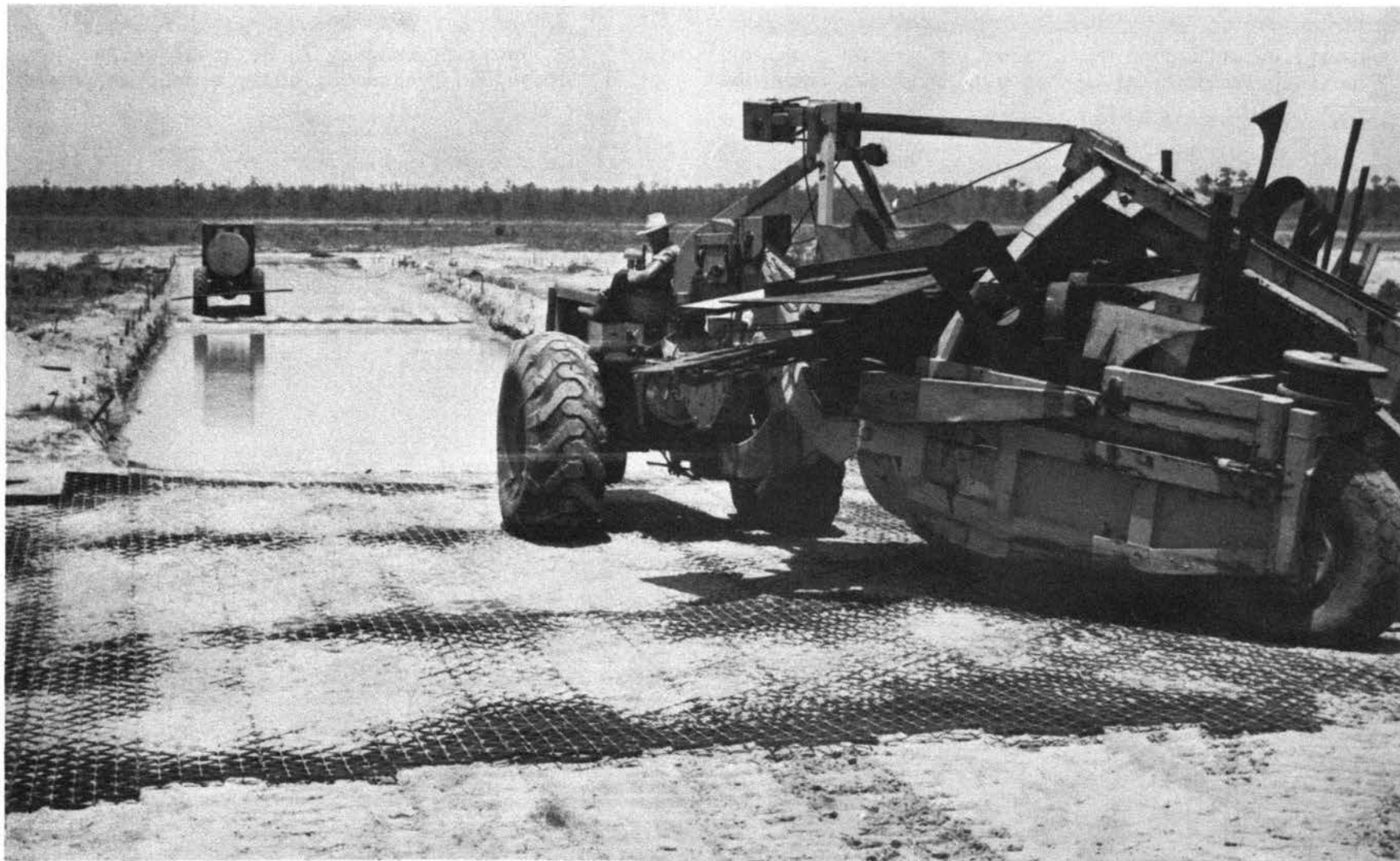
Photograph 5. Tournapull loaded to 15,000 lb per wheel entering ponded area of Section 2
