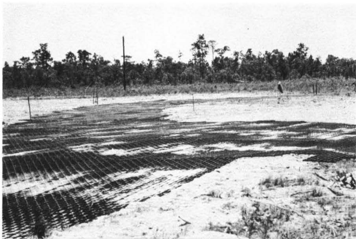
Photograph 8. Landing mat turnaround at south end of Section 2
