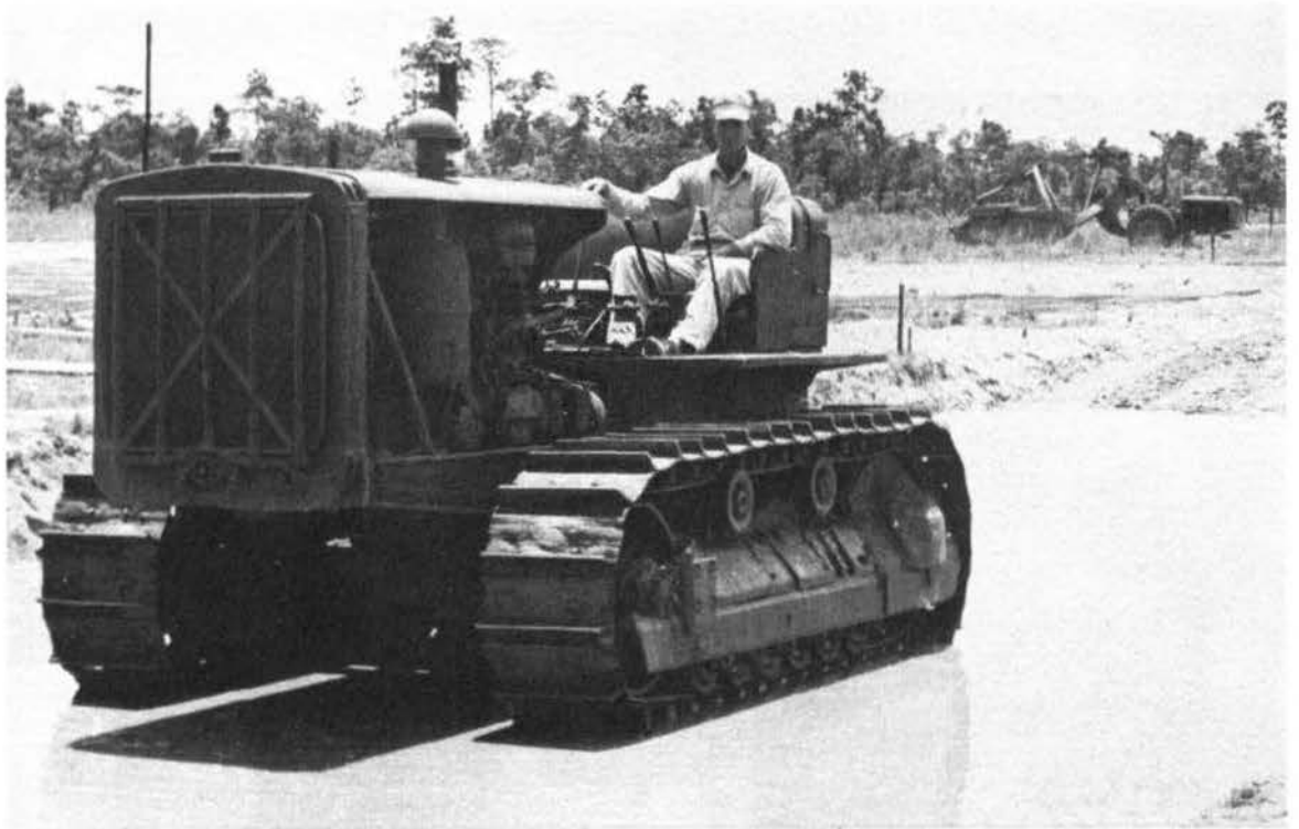
Photograph 3. RD-8 tractor in ponded area of Section 1
