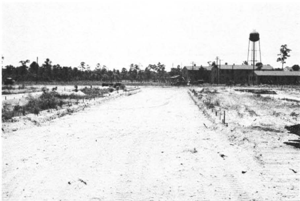
Photograph 7. Section 3 after grading
