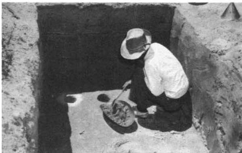
Excavating hole for field density determination
