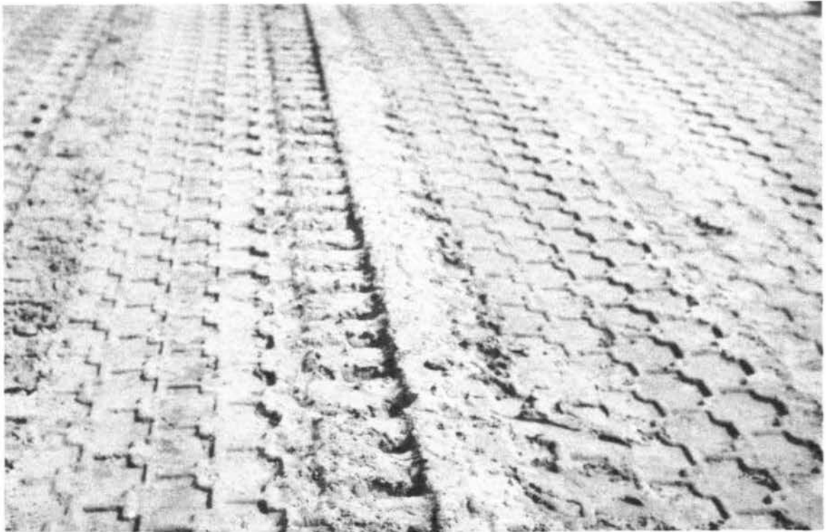
Photograph 10. Tire marks of 60,000-lb wheel load in sprinkled area of Section 3
