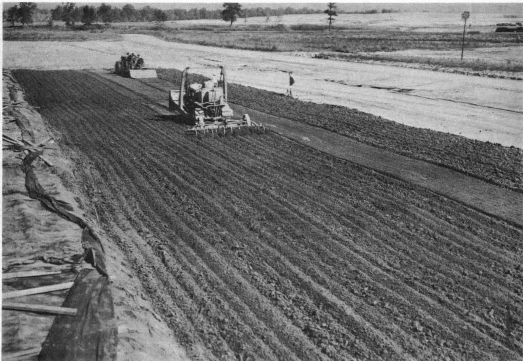
Killifer plow and Seaman pulvimixer plowing material prior to compaction
