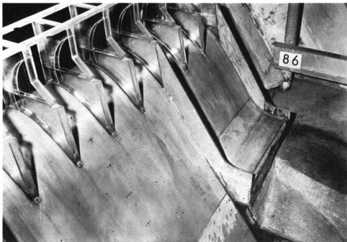
Photograph 65. Details of the type A center training wall
