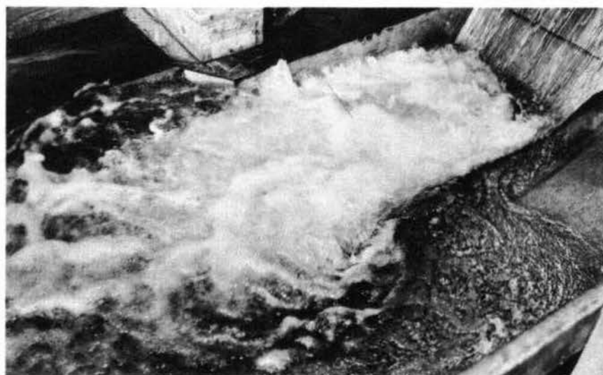
Photograph 59. Flow conditions of basin with: gates 1 through 5 open full; crest dischg, 300,000 cfs; penstocks closed; pool elev, 468.6; tailwater elev, 212.6
