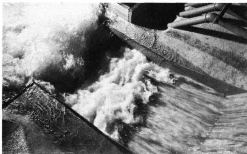
Photograph 43. Flow conditions of basin with: gates 1 through 5 open full; crest dischg, 300,000 cfs; penstocks closed; pool elev, 468.6; tailwater elev, 212.6
