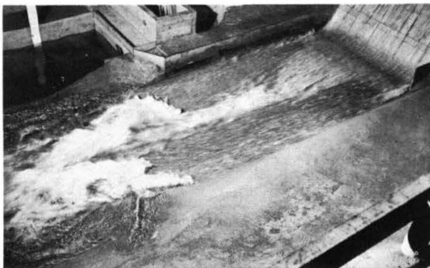
Photograph 21. Jet action of bucket. Gates 1 through 5 open 14 ft; crest dischg, 108,000 cfs; penstock dischg, 7,000 cfs; pool elev, 466.0; tailwater elev, 179.2
