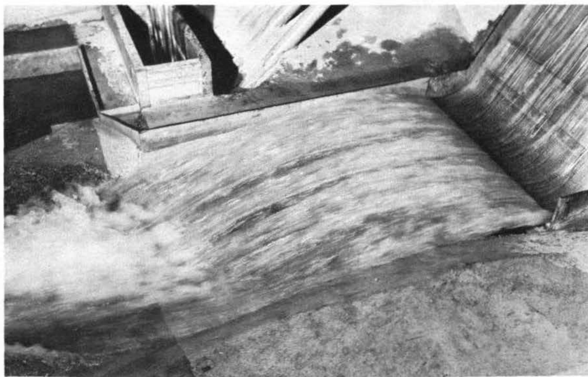
Photograph 8. Flow conditions below bucket of original design with contour area altered on the left bank. Spillway gates 1 through 5 open 14 ft. Crest dischg, 108,000 cfs; penstock dischg, 7,000 cfs; pool elev, 466.0; tailwater elev, 179.2
