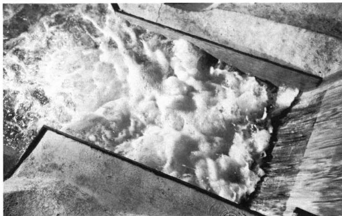
Photograph 35. Gates 1 through 5 open 28 ft; crest dischg, 193,000 cfs; penstock dischg, 7,000 cfs; pool elev, 466.0; tailwater elev, 196.0
