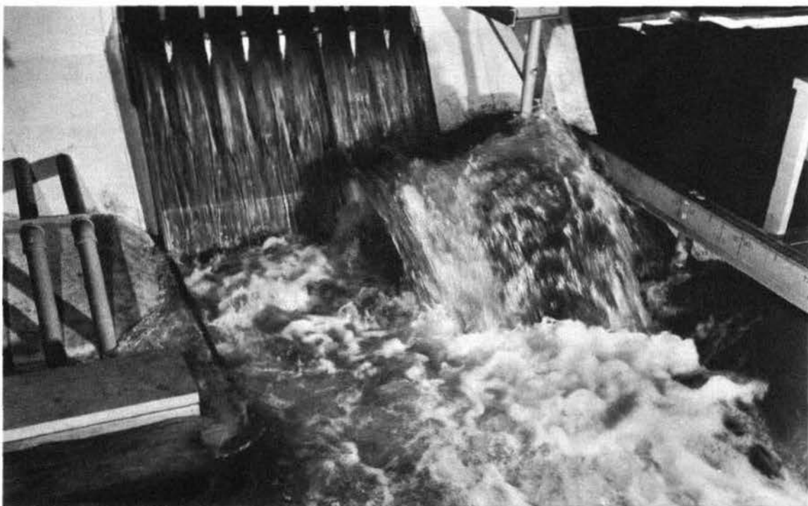
Photograph 50. Gates 1 through 8 open full; crest dischg, 567,000 cfs; penstocks closed; pool elev, 473.0; tailwater elev, 242.0
