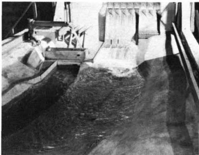
Photograph 1. Spillway gates 1 through 5 open 6 ft; crest dischg, 50,000 cfs; penstock dischg, 7,000 cfs; pool elev, 466.0; tailwater elev, 176.5
