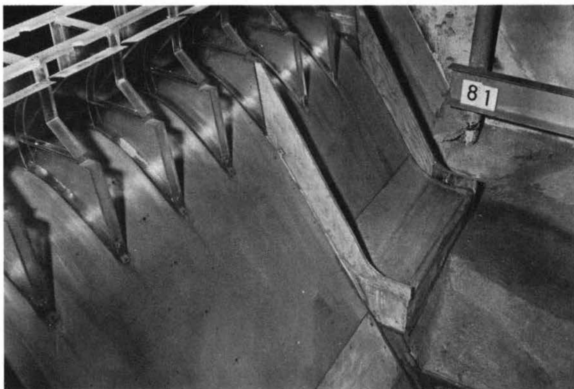
Photograph 67. Details of type C center training wall
