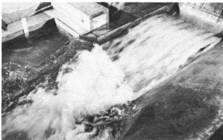
Photograph 25. Jet action of bucket. Gates 1 through 5 open 28 ft; crest dischg, 193,000 cfs; penstock dischg, 7,000 cfs; pool elev, 466.0; tailwater elev, 196.0
