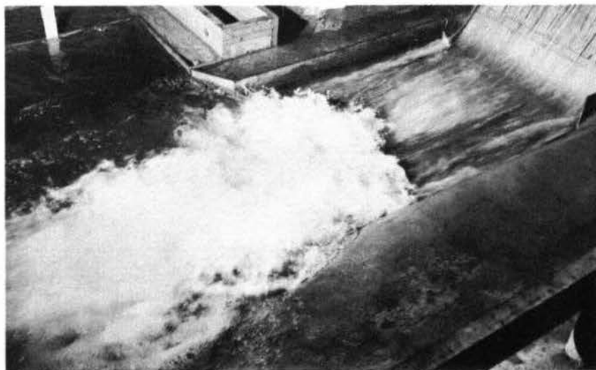
Photograph 23. Jet action of bucket. Gates 1 through 5 open full; crest dischg, 300,000 cfs; penstocks closed; pool elev, 469.4; tailwater elev, 212.6
